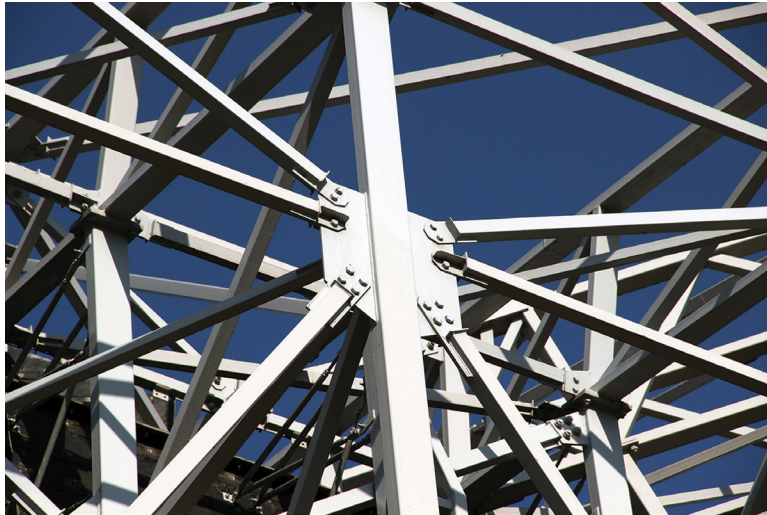
FIGURE 13-1 Much time and effort is invested in the design and analysis of loads and stresses on machine elements and structural components. Since that loading must be safely transferred to neighboring components, similar diligence must be exercised with regard to connections.
