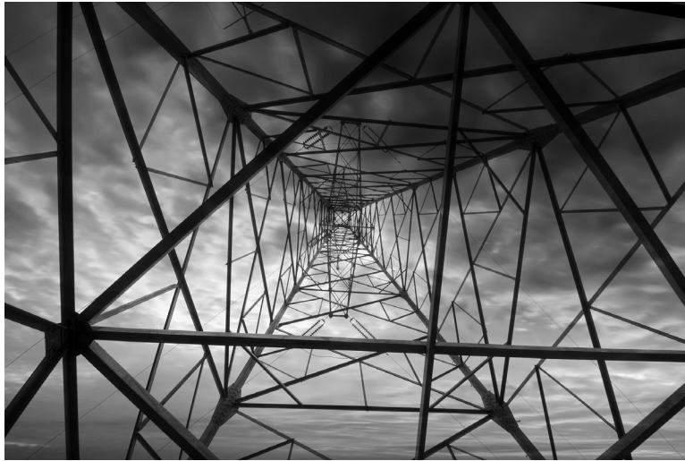
FIGURE 11–1 (See color insert.) Trusses are rigid networks of simple two-force members and provide the framework for many structures such as this tall tower. Each member of this tower is long relative to its cross section, so any that is loaded in compression is susceptible to buckling. Care must be taken to ensure that no single member of this structure buckles resulting in a sudden and catastrophic failure of the entire structure.
