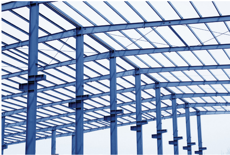
FIGURE 7-1 Elements loaded in bending require more analysis than those with simple axial loads, and proper calculation and design is critical. Look at all the beams in this building, and consider the serious responsibility of the designer to assure that, once completed, these beams can safely support the roof panels, the roofing material, and all other loading.
