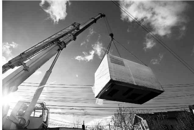
FIGURE 10-2 Crane boom loaded in bending and compression.
