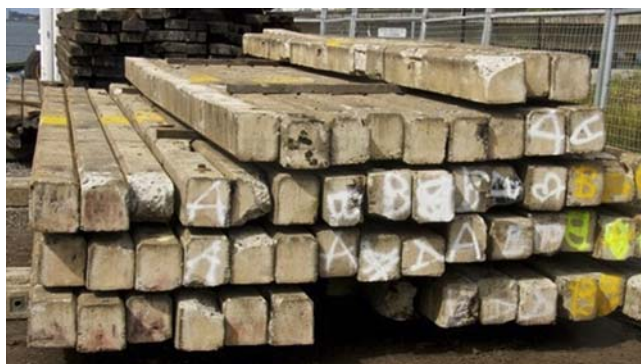
Figure 2.3 Piles in storage after demolition, showing no exterior evidence of internal corrosion. Even after the extended period (80+ years) of exposure in the marine atmosphere, the tidal zone and immersed, there were no signs of longitudinal cracking along the lines of reinforcement.
