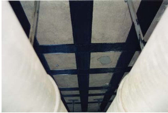
Figure 7.2 Wet lay-up of fabric on soffit affords efficient strengthening.
