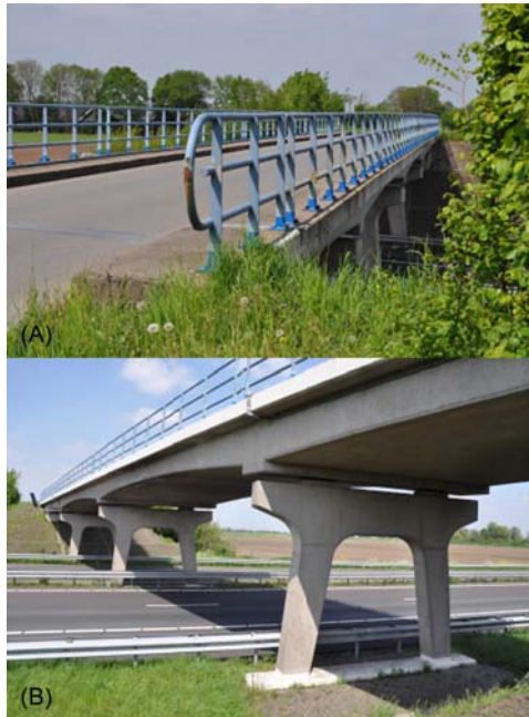
Figure 9.1 Photograph of viaduct Zijlweg: (A) top view; (B) bottom view.
