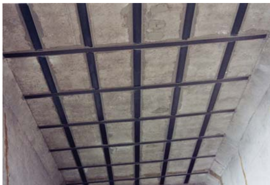
Figure 7.1 Adhesively bonded pultruded strips.
