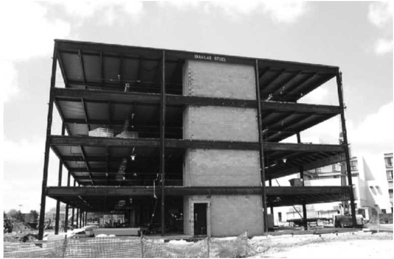
FIG. 2.3 This Steel Frame Building Uses Masonry Shafts for Elevators and Stairs to Resist Lateral Loads Due to Wind and Earthquakes
