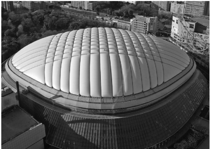
FIG. 1.6 The Fabric (membrane) Roof of the Tokyo Dome is Tensioned (inflated) by Air Pressure from Inside the Stadium © Gavin Hellier / Alamy
