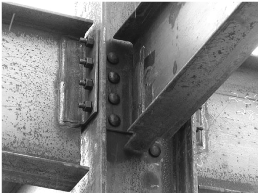
(a) Beam-to-Column Shear Connections
