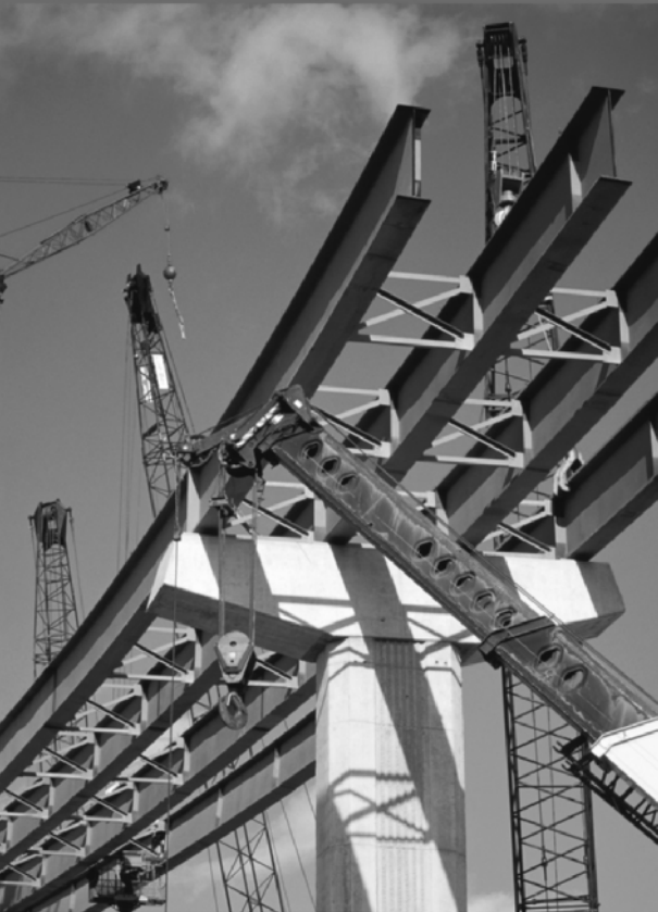
Bridge Construction on an Expressway
