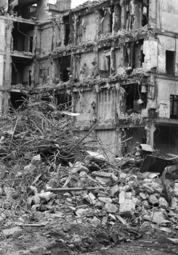
Earthquake-Damaged Building Ints Vikmanis/Shutterstock.com
