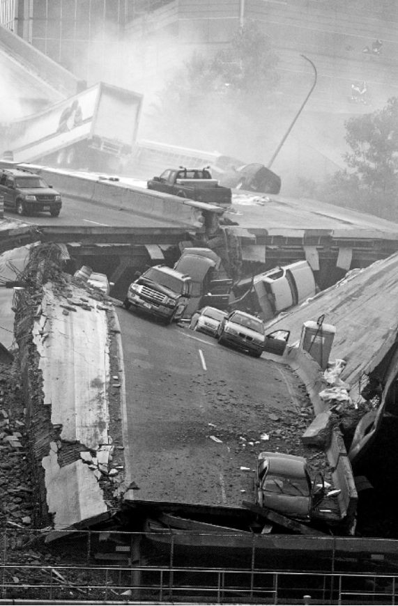
Interstate 35W Bridge Collapse in Minnesota (2007)
