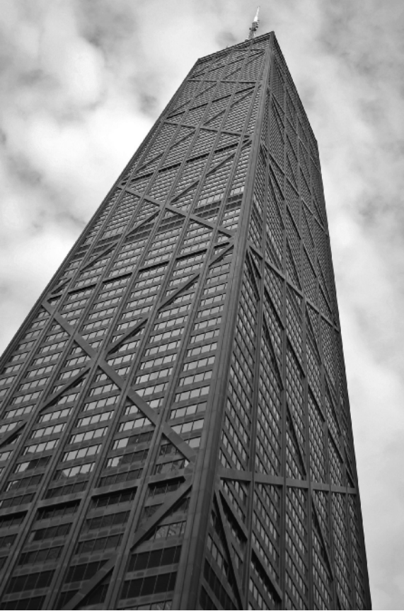
The John Hancock Building in Chicago with cross-bracing on its exterior to reduce horizontal movement due to strong winds
