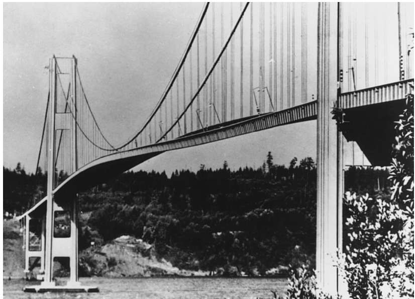
FIG. 1.5 Tacoma Narrows Bridge Oscillating before Its Collapse in 1940 Smithsonian Institution Photo No. 72-787. Division of Work & Industry, National Museum of American History, Smithsonian Institution
