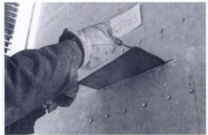
Figure 13. Placing the flat jack.
