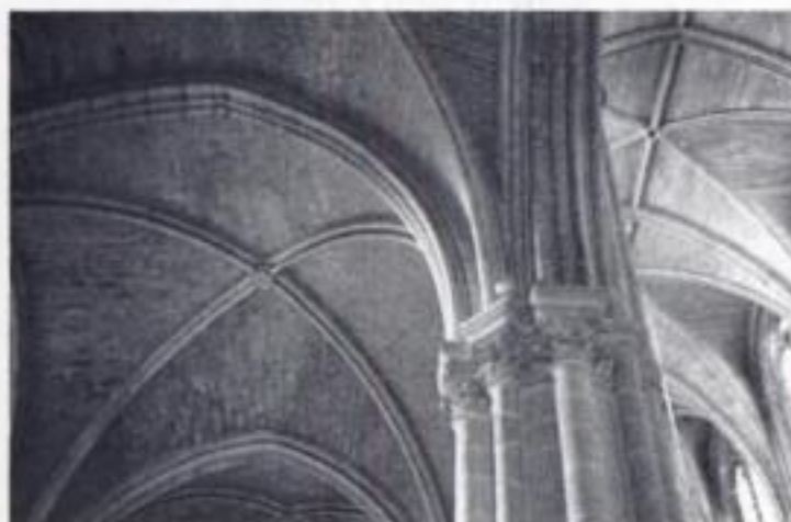
(b) Aisle vault
