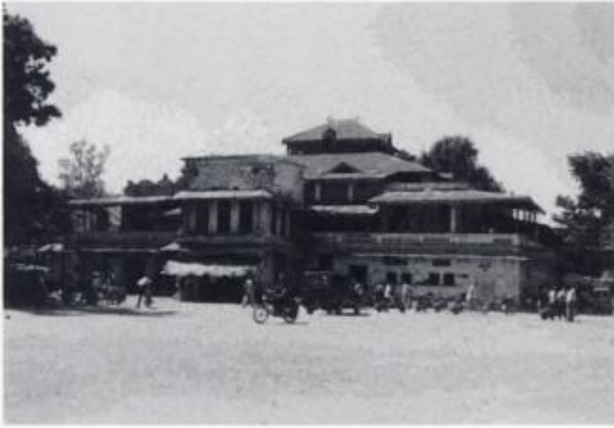
Figure 2. RTO building damaged during Jabalpur earthquake of 1997, India.
