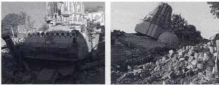
Figure 3. Wide spread damage was caused to temples all around the Gujarat during Bhuj earthquake causing complete failure.
