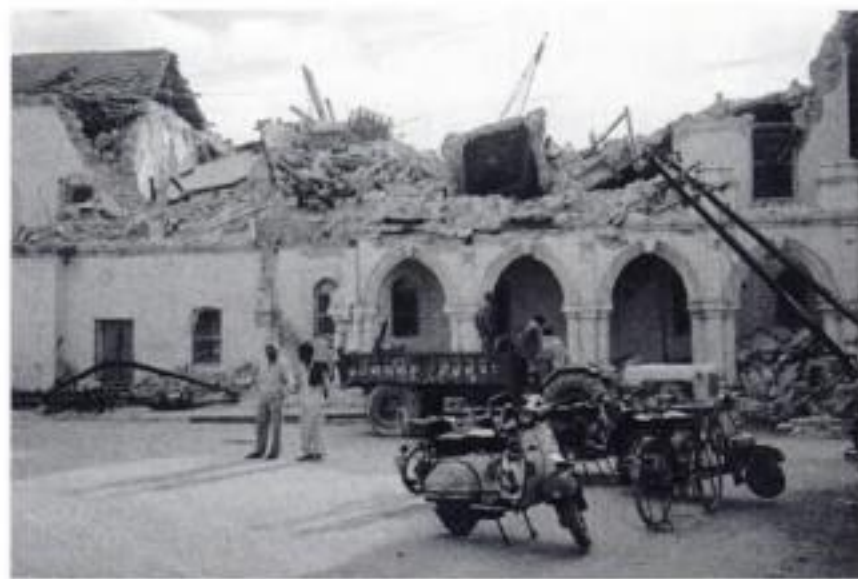
Figure 1. Monument at Bhuj damaged due to Gujarat Earthquake.
