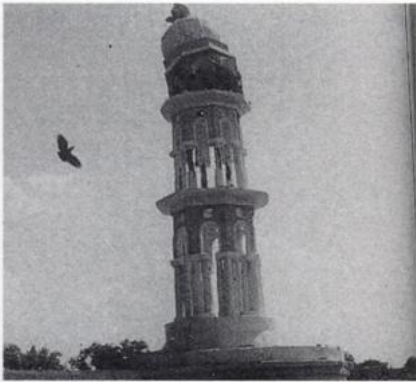
Figure 9. Partly broken and tilted minar of Idgah (the prayer place for muslims) during Jabalpur earthquake.
