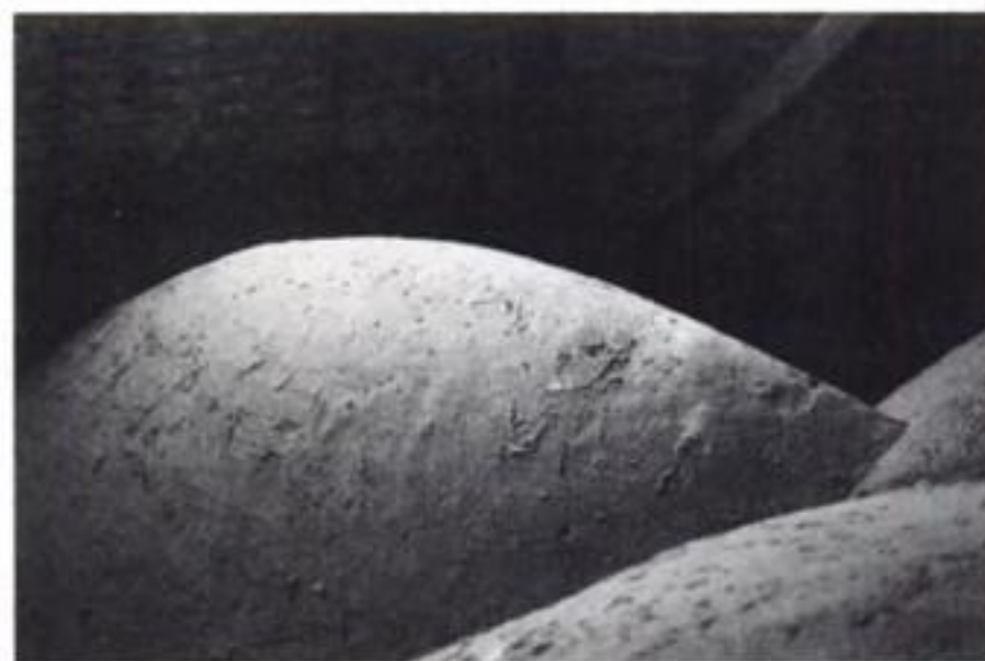
Figure 22. Extrados of a vault. The ridge line shows a characteristic profile.
