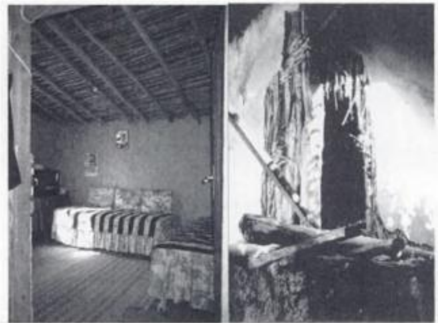
Figure 15, 16. Ridge roof construction without truss, and reed covering material. Adana, 2000 and Huğ House's wall detail, Mersin, 1998 (demolished in 1999).
