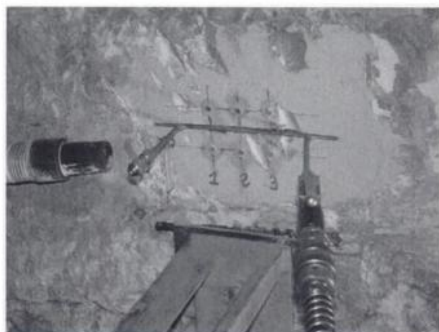
Figure 15. Flat-jack inside the slot.
