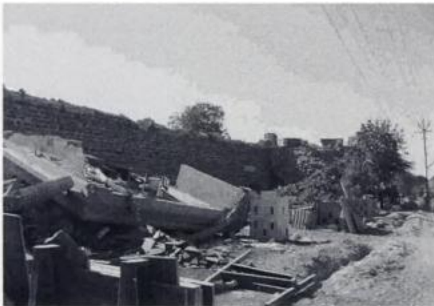
Figure 4. Collapse of wall of a Bhuj fort.
