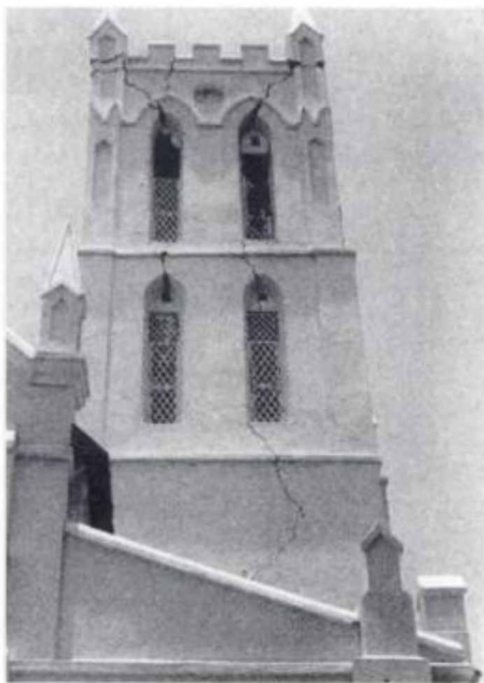
Figure 12. 125 years old St. Paul Cathedral Church cracked with partial collapse of tower.
