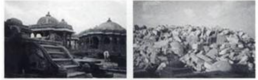
Figure 5. Chattris are very common in Gujarat area. Figure shows the view of Chattri before and after the Bhuj earthquake.
