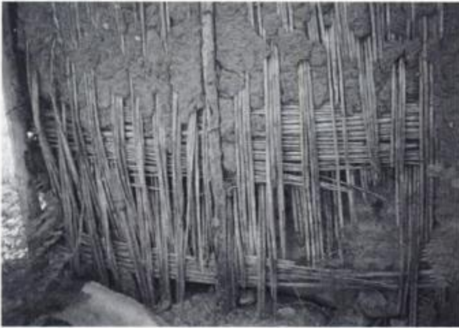
Figure 7. The detail of masonry bond of traditional Huğ House, 1998.
