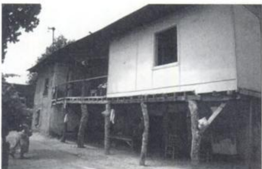
Figure 18. Two-storey Huğ House, Adana, 1999.
