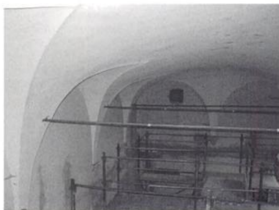
Figure 4. Image of the tie beams n. 2, 3, 4.
