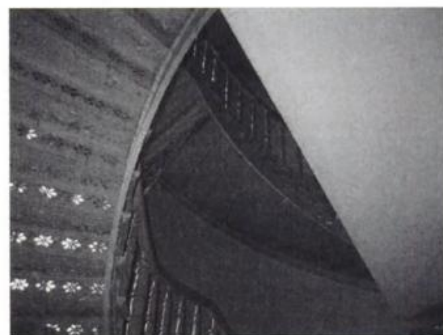
Figure 10. A steel staircase.
