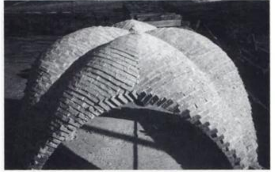
Figure 25. The extrados of the finished vault prototype.
