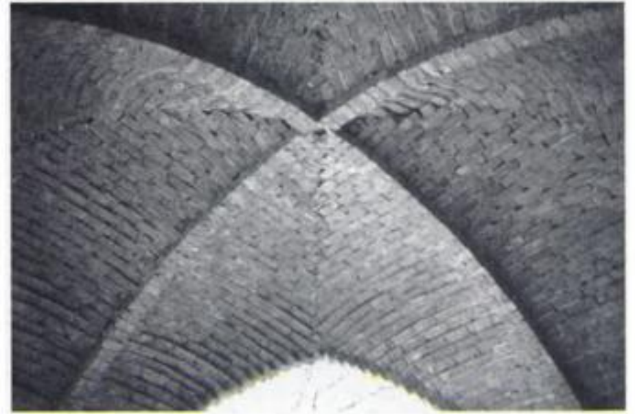
Figure 26. The intrados of the finished vault prototype.
