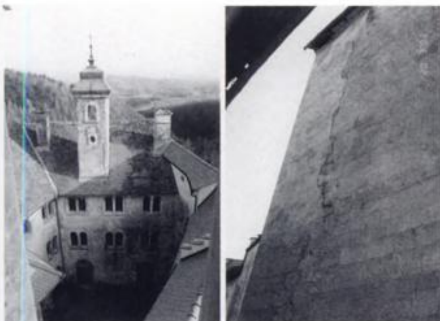
Figure 3. Left: Pisece Castle in Slovenia built at the first half of the 13th century as defense fortification against the Hungarian threat by archbishop of Salzburg. Right: Crack at the main tower.
