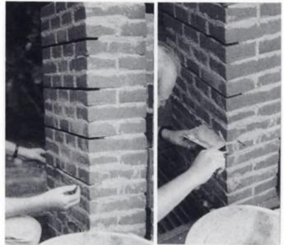
Figure 19. Application of CFRP strips in an experimental panel.
