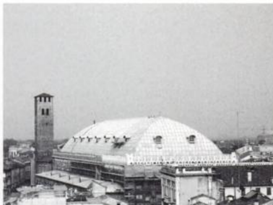
Figure 1. External view of the roof of the “Palazzo della Ragione” in Padua.
