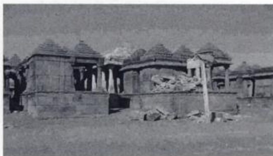
Figure 13. Collapse of Chattris made up of large block stone masonry during Bhuj earthquake.
