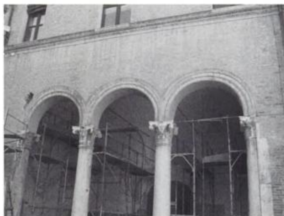
Figure 3. Image of the pavilion vault arcade under investigation.
