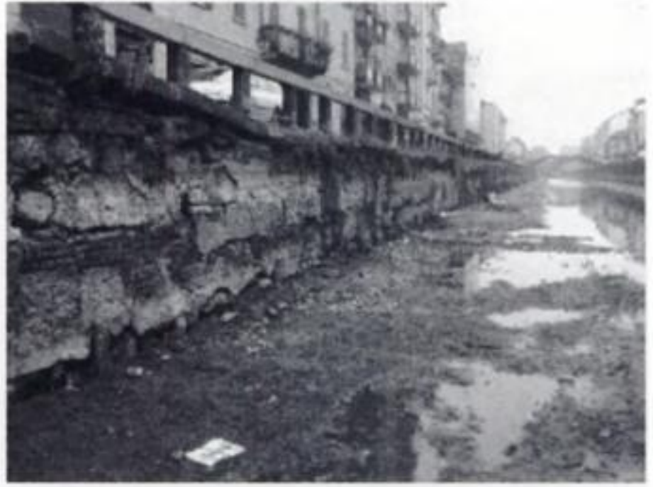
Figure 9. Example of today's sidewall.
