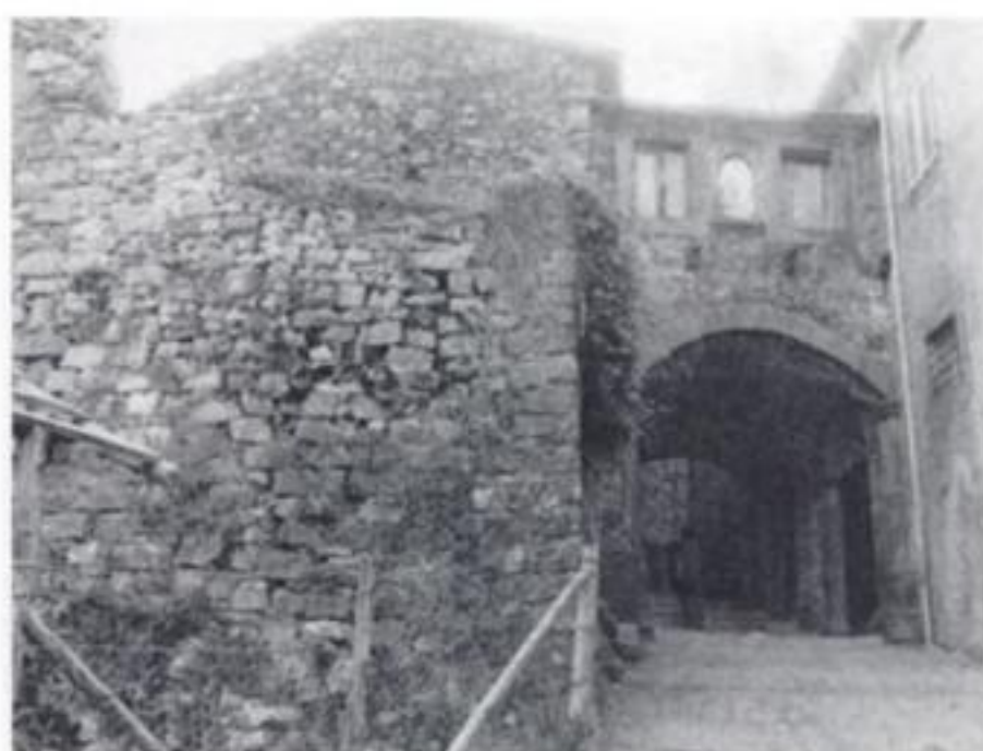
Figure 2. The habitable buttressing in the old town of Albiano.
