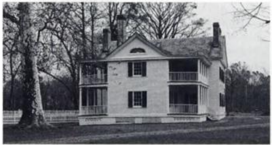
Figure 10. Mid-nineteenth century plantation house with clapboard over brick nogging.
