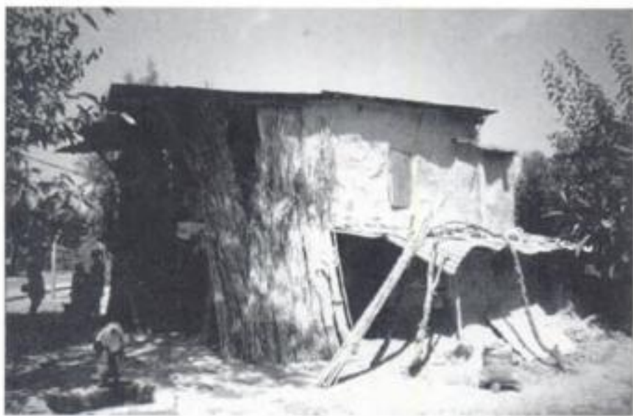
Figure 17. Two-storey Huğ House, Kayışh Village, Adana, 1999.
