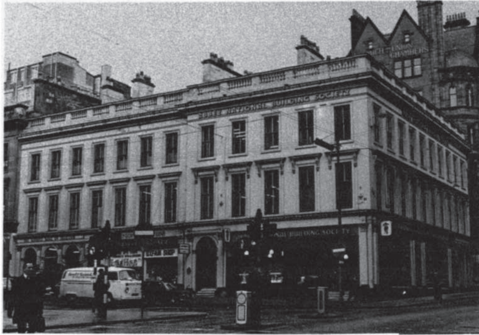
Figure 7.87 Abbey House, Glasgow: before redevelopment.
