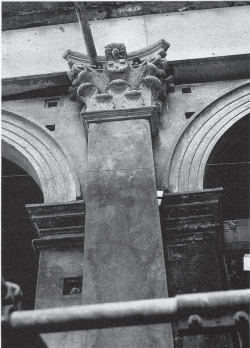
Figure 7.89 Abbey House, Glasgow: new glass reinforced concrete arcading.
