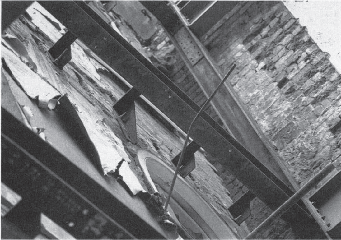
Figure 7.13 118–120 Colmore Row, Birmingham: new beam and facade-tie brackets in permanent positions.
