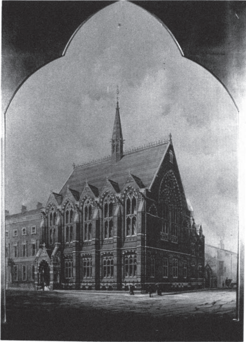
Figure 5.1 Church Institute, Leeds: before redevelopment.
