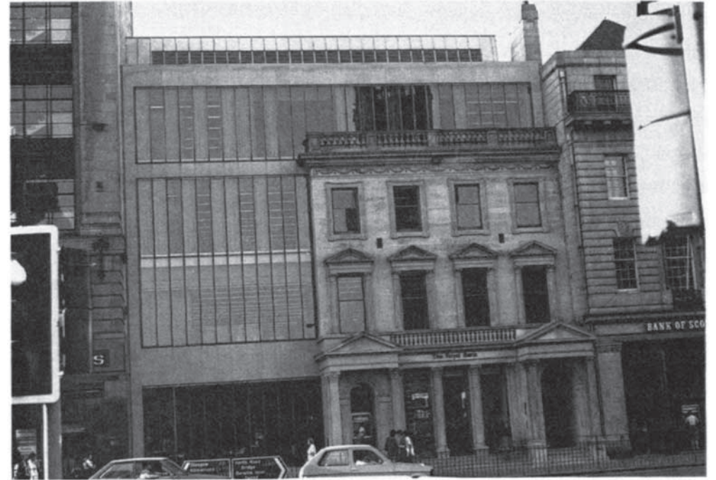
Figure 5.4 142–144, Princes Street, Edinburgh: after redevelopment.
