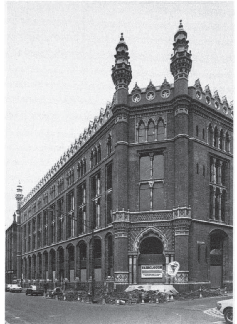
Figure 7.21 St Paul's House, Leeds: after redevelopment.
