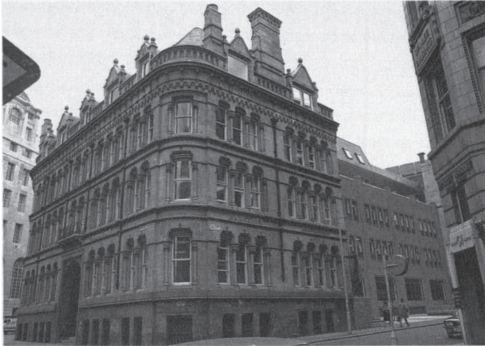
Figure 5.5 Barclays Bank, Manchester: after redevelopment.
