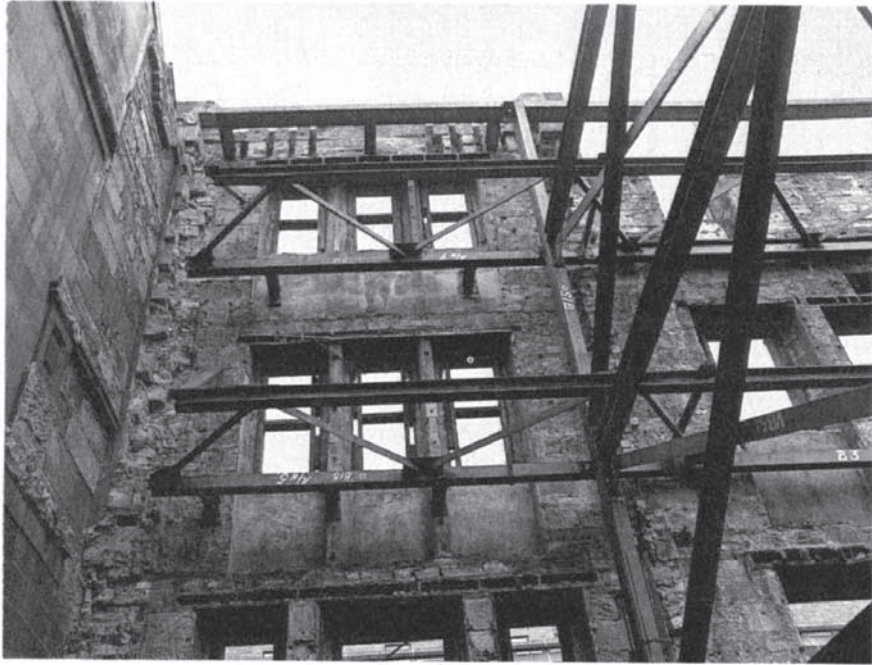
Figure 7.53 144 West George Street, Glasgow: view from rear showing temporary support system.
