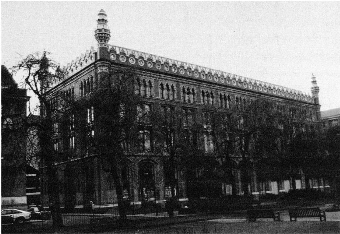
Figure 7.20 St Paul's House, Leeds: after redevelopment.
