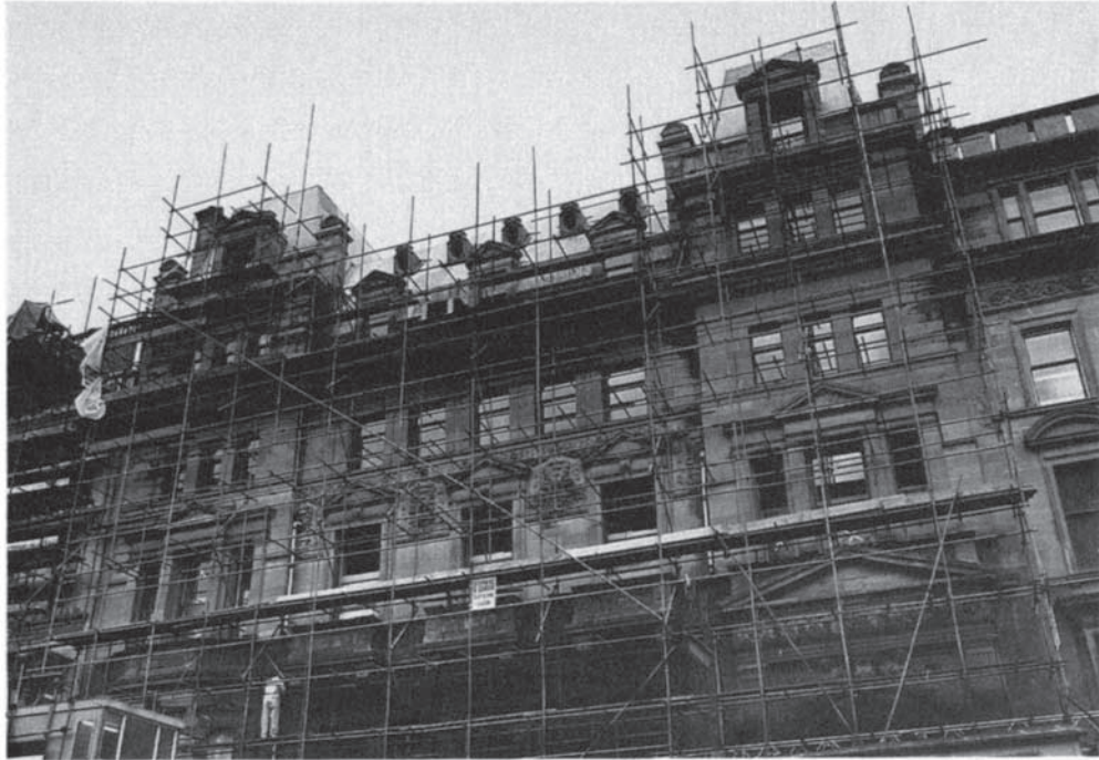
Figure 7.49 144 West George Street, Glasgow: front elevation near completion of the scheme.
