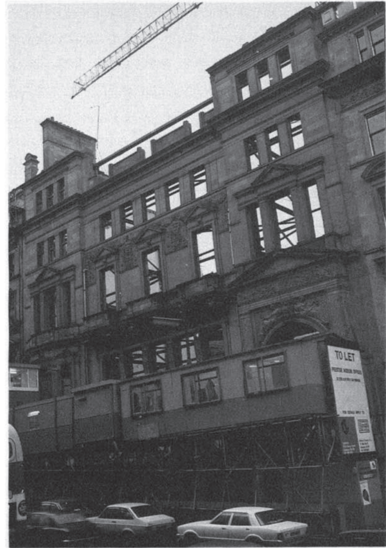
Figure 7.50 144 West George Street, Glasgow: front elevation after completion of interior demolition.
