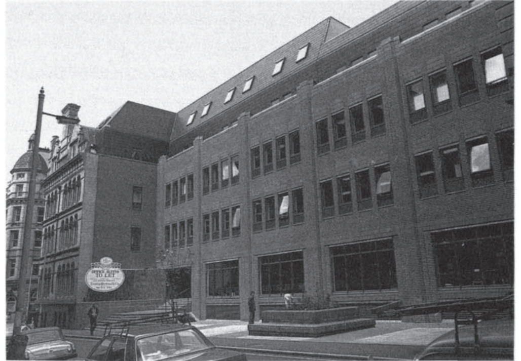
Figure 5.6 Barclays Bank, Manchester: after redevelopment.
