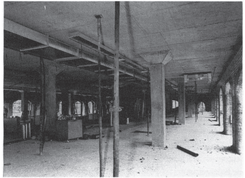
Figure 7.25 St Paul's House, Leeds: interior view after structural completion.
