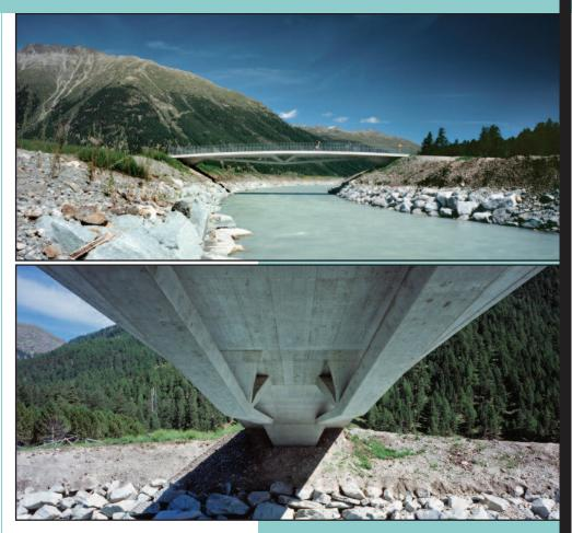
tension ties, the diagonals and the deck were cast. The cables were tensioned in three steps: 30% after three days, 75% after eight days and subsequent demoulding, 100% after 28 days following the casting of the edges. The behaviour of the structure was verified by simple deformation measurements before and after tensioning, demoulding and laying the deck paving: the measured and calculated vertical deformation values were very close.
