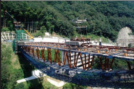
"This self-anchored composite truss bridge responds strongly to the desire of the Jury for projects that impact only lightly on their environment. By constructing the lower chord first as a stressed ribbon, very little disturbance was made to the site as the result of construction activities.
