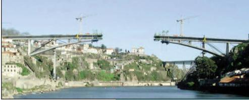
central span was built by typical cast-inplace segmental methods. A major achievement was a highly efficient monitoring system for the structural behaviour during construction, assessing support reactions, axial forces, bending moments, axial forces in the temporary stay cables etc. Three independent systems allowed to control all movements from the exact positioning of formwork to the removal of the temporary pillars.
