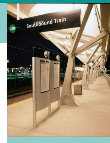
"The distinctive elements of this building are the thin high performance fibre-reinforced concrete shells forming a series of canopies.
