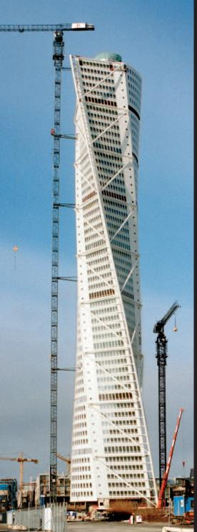
the façade. Prefabricated formwork and reinforcement elements were used for these slabs.
