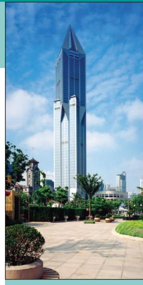
"The Jury were impressed by the fact that whilst the building shape is rotated through 45° at the 37th level it is done in a transitional way that avoids direct transfer structures.
