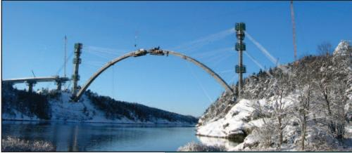
temporarily supported by cable stays from a temporary concrete tower on each side of the fjord; stays also reduced the transverse movement of the arch. To save construction time, the main span was erected in one prefabricated unit that was fabricated in smaller segments in Germany, then transported by barge to a location 10 km from the bridge. Here the units were assembled, transported to the site and within 12 hours installed by lifting from temporary crossbeams resting on top of the arch.
