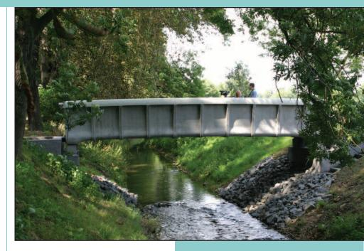
the joints between the segments stay closed in all load cases and the transmission of shear within the joints is secured.
