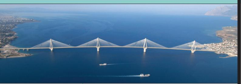
The Rion-Antirion cable-stayed bridge crosses the Gulf of Corinth near Patras in western Greece with a total length of 3 km including its two access viaducts. The three central spans measure 560 m each.
