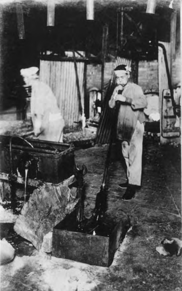
Figure 7.1 Production by the cylinder method.
