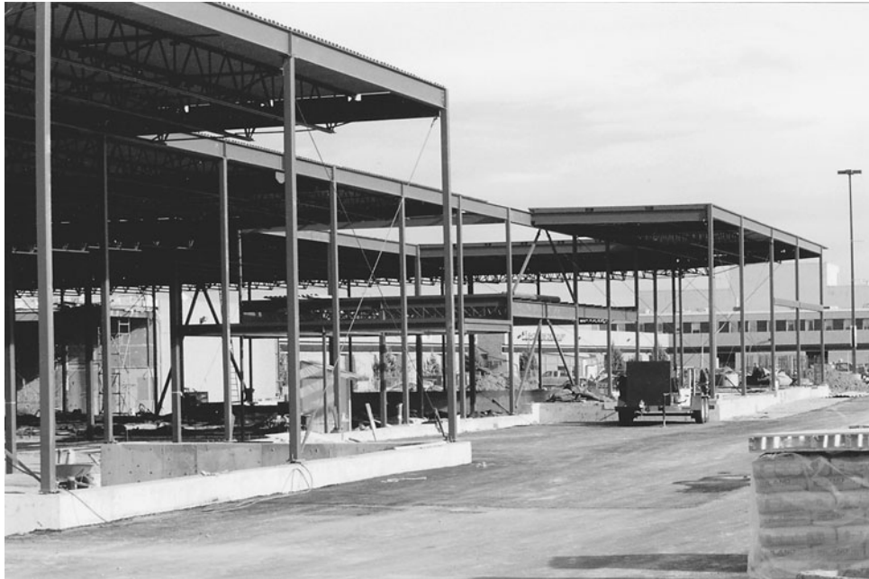
Figure 10-27 Typical Structural Steel Frame.
