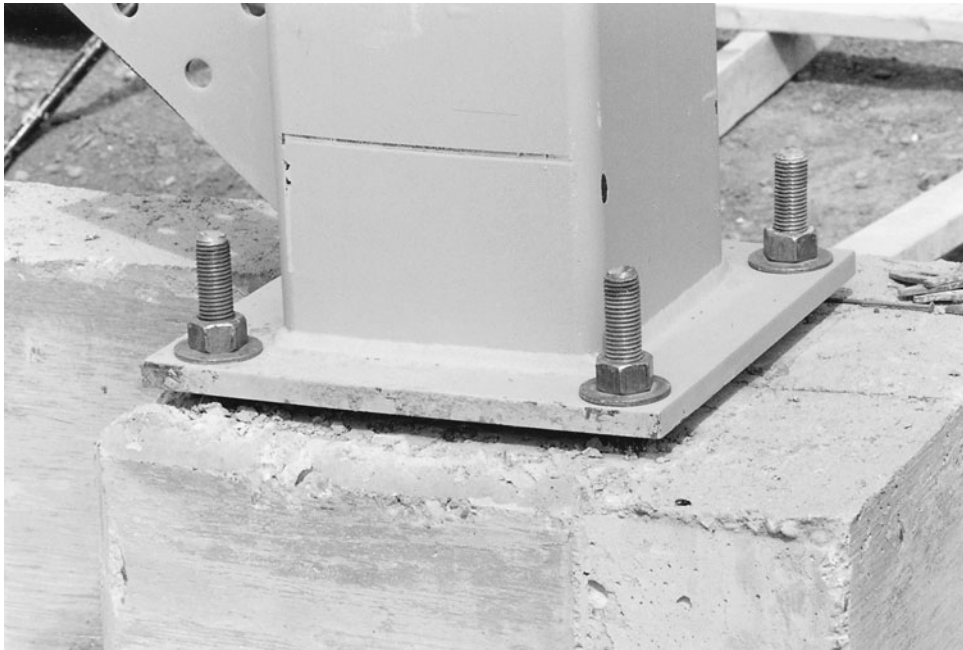
Figure 10-23 Column Base Plate Secured by Anchor Bolts.
