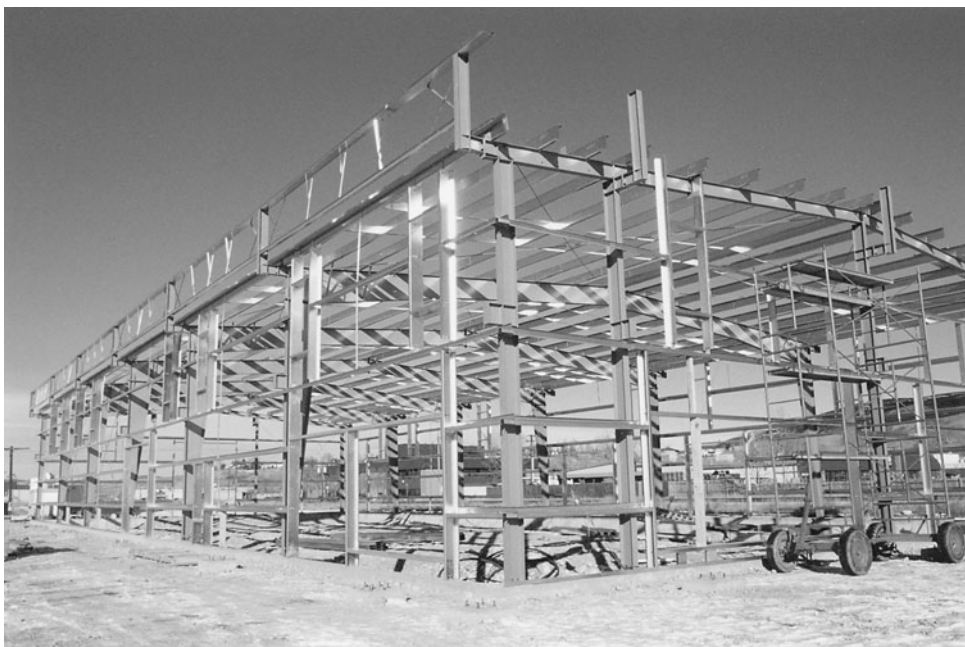
Figure 10-18 Cold-Formed Girts and Roof Purlins.
