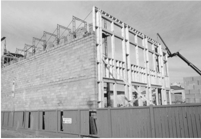
Figure 14-3 Load-Bearing Lightweight Concrete Block Curtain Wall.
