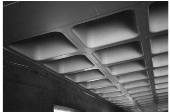
Figure 11-20 Underside of Waffle Slab.
