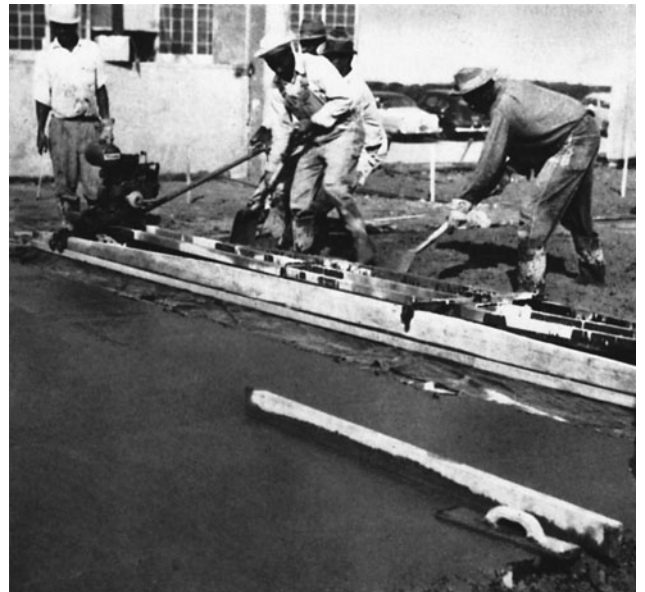
Figure 11-4 Power-Screeding a Slab-on-Grade Concrete Floor.
