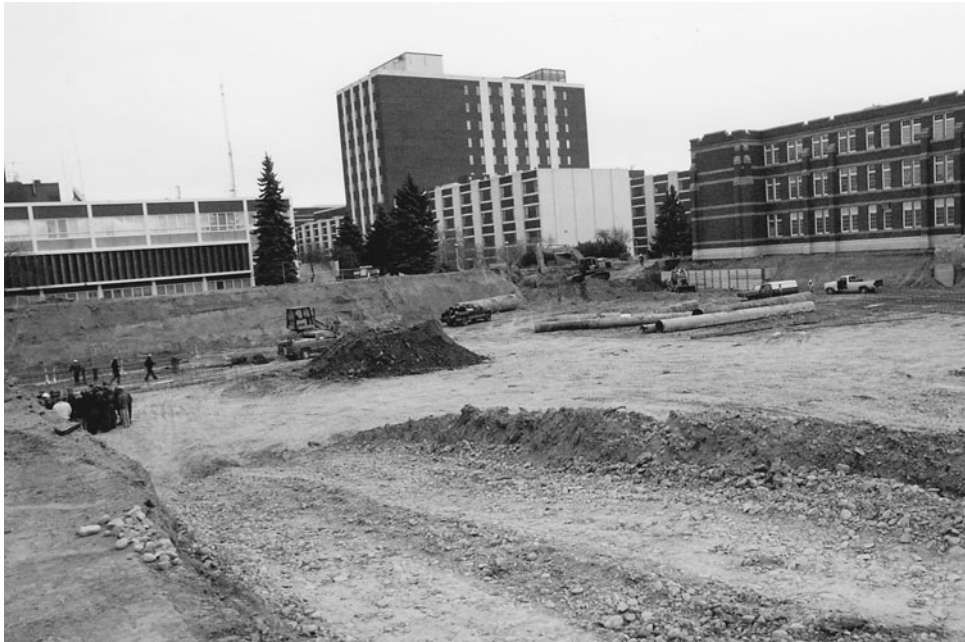
Figure 3-1 Access Ramp into Building Site Excavation.
