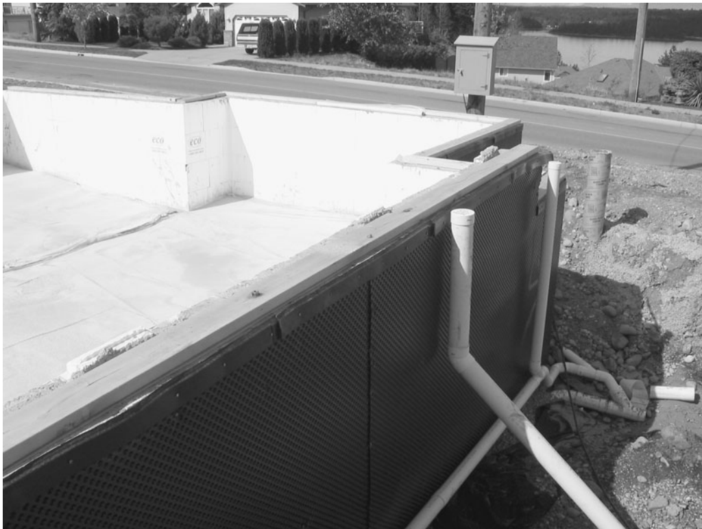
Figure 15-25 Expanded Polystyrene Block Wall with Protective Exterior Covering.
