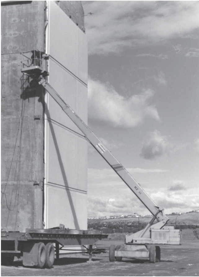
Figure 14-20 Plant-Cast Precast Concrete Wall Panels.
