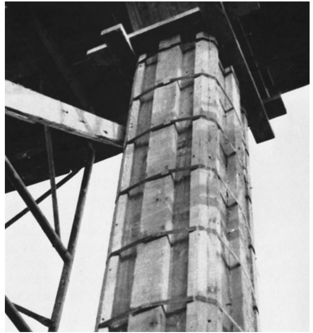
Figure 9-12 Steel-Banded Column Form. (Courtesy Acme Steel Co.)
