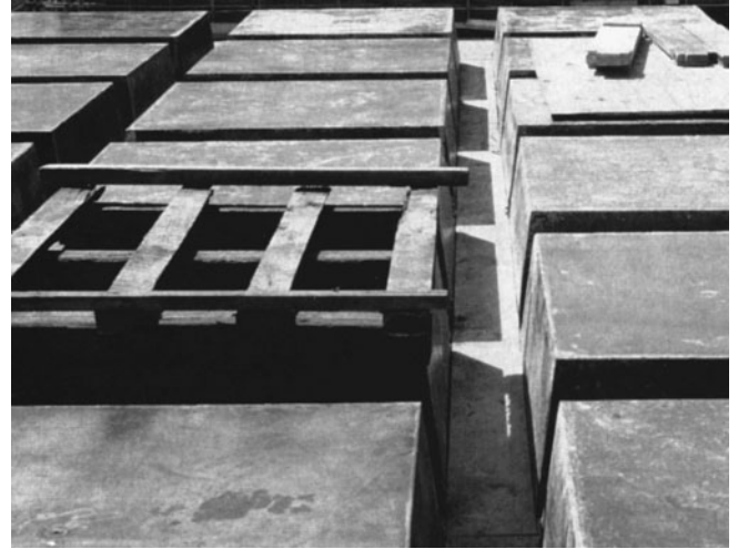
Figure 6-5 Metal Pan Forms.
