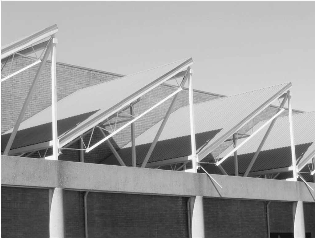
Figure 12-19 Unusual Joist Roof Framing.
