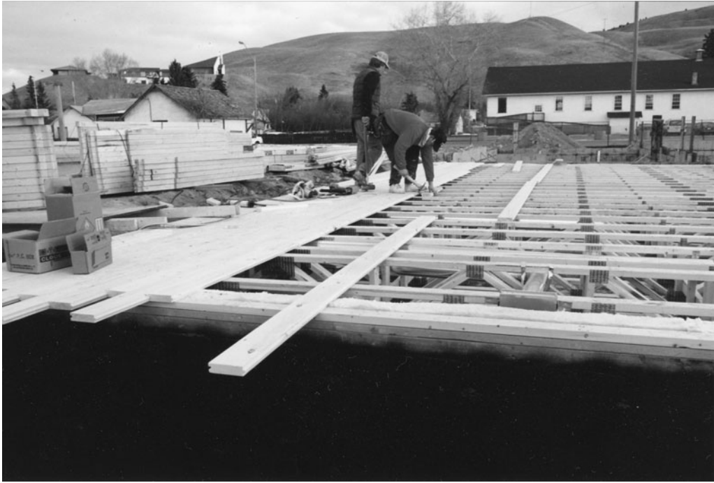
Figure 11-3 Plank Decking Applied to Open-Web Joists.
