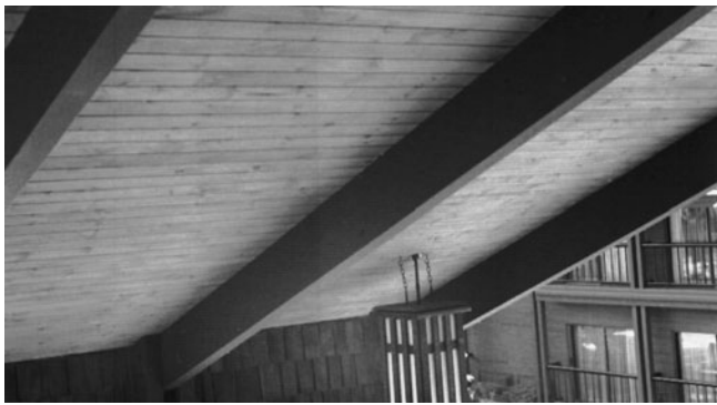
Figure 8-21 Decking on Main Beams.
