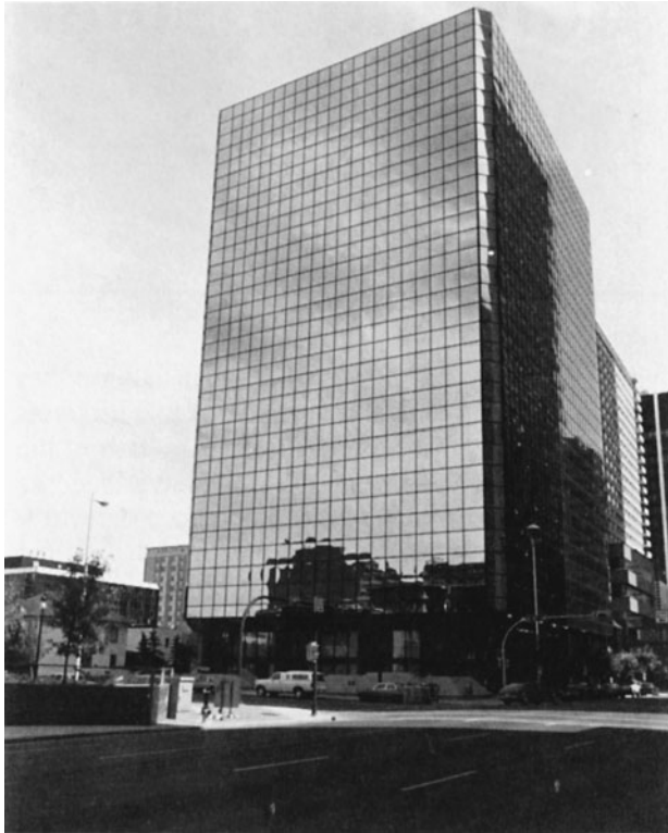
Figure 14-47 Reflective Glass Curtain Wall.
