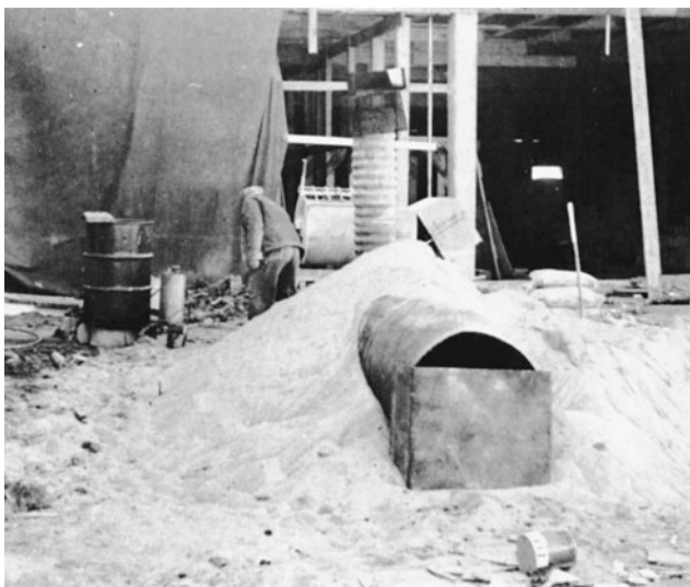
Figure 13-48 Keeping Mortar Sand Warm. (Reprinted with permission of Portland Cement Association.)
