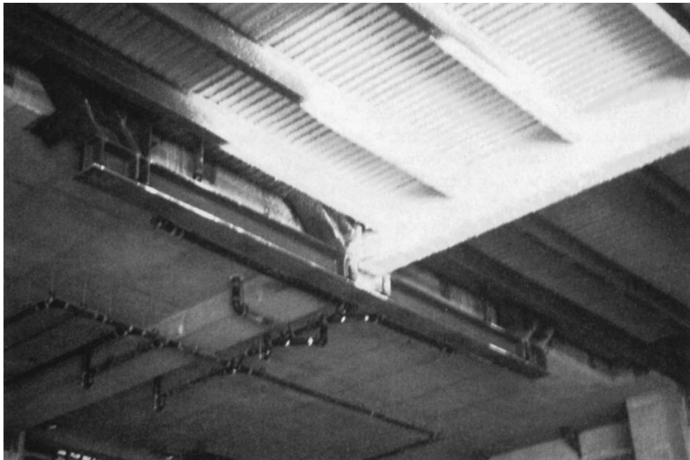
Figure 15-7 Structural Steel Beams and Decking Fire Protected with Sprayed-On Insulation.
