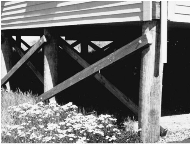
Figure 5-4 Driven Pressure-Treated Timber Piles Used in Sandy Soil.
