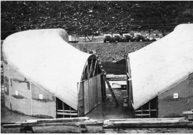
Figure 6-2 Intricate Formwork Can Be Achieved Using Plywood Sheathing.
