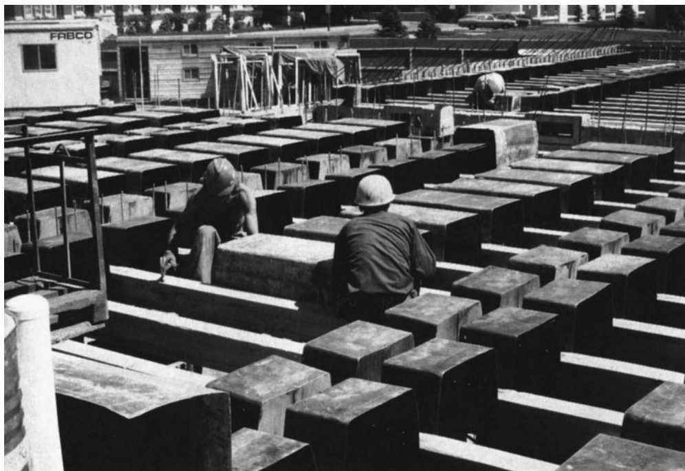
Figure 6-69 Ribbed Slab Floor Forms.
