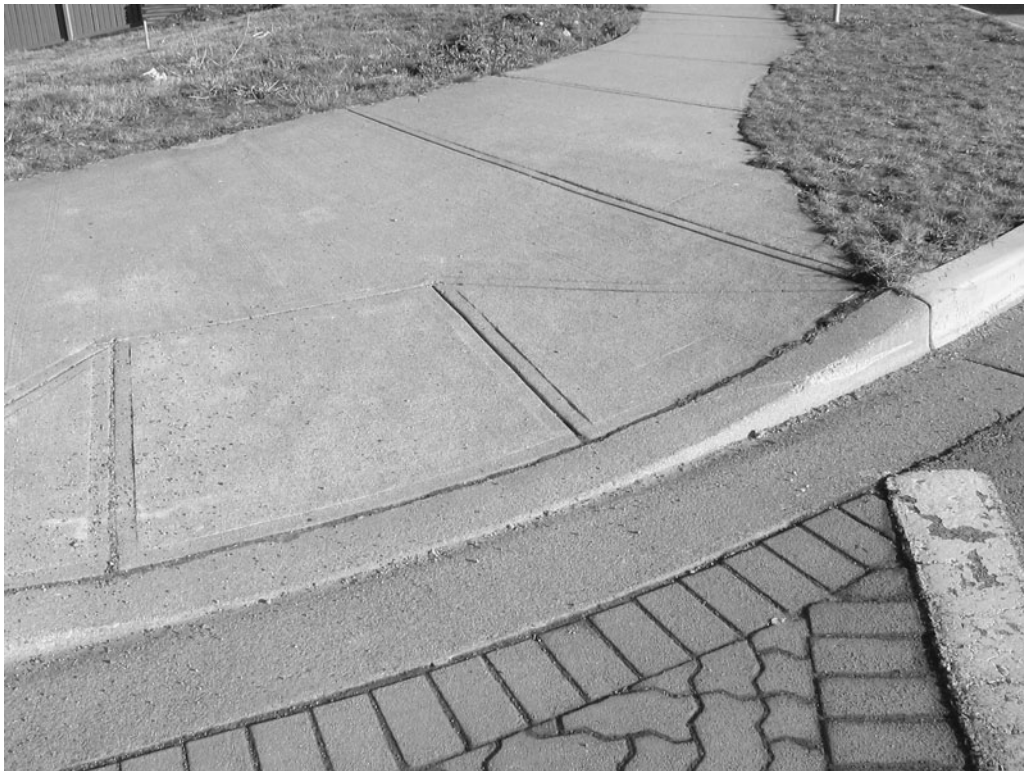
Figure 4-13 Curb Ramp at Street Intersection.
