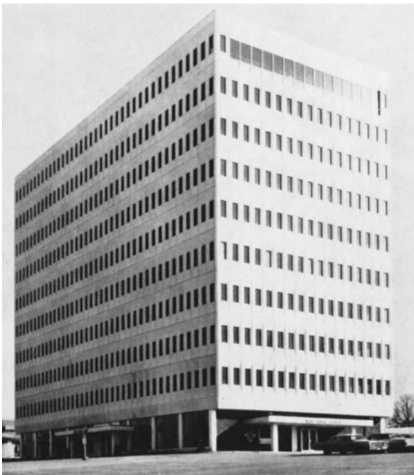
Figure 9-59 Walls Built from One Master Mold. (Reprinted by permission of Precast/Prestressed Concrete Institute.)
