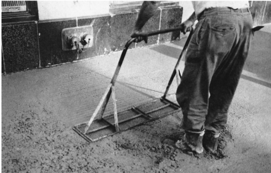
Figure 11-58 Consolidating and Leveling a Concrete Floor. (Reprinted with permission of Portland Cement Association.)
