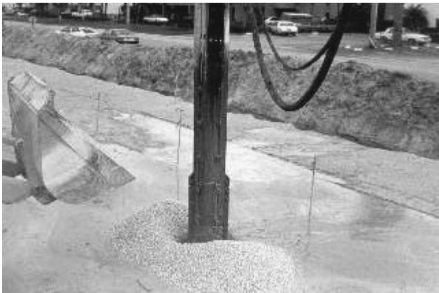
Figure 5-38 Vibrator Inserted in Soil. (Courtesy Hayward Baker Inc.)
