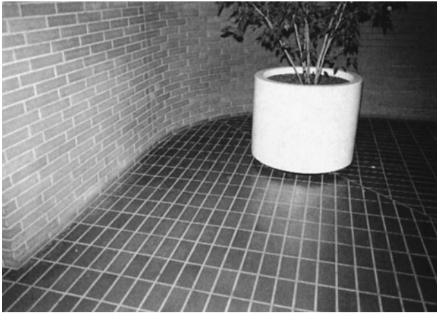
Figure 16-41 Brick and Tile Provide a Durable Interior Finish to Walls and Floors.
