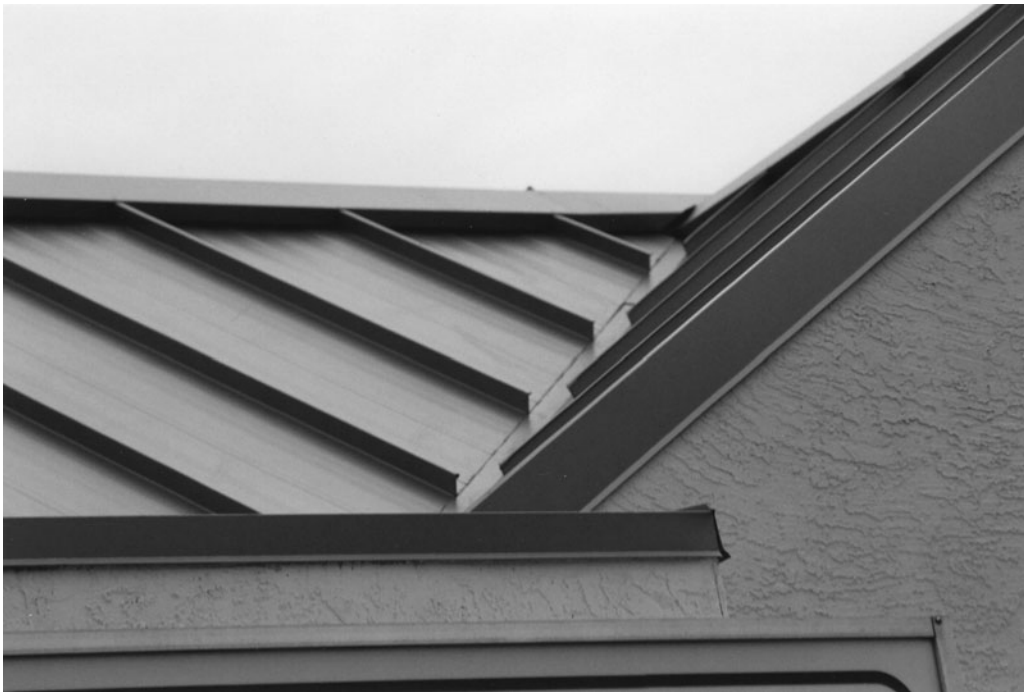
Figure 12-60 Standing Rib Metal Roof Membrane.
