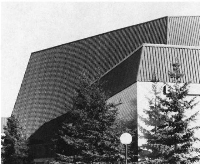
Figure 16-5 Prefinished Metal Siding Is Available in Different Colors and Is Easily Applied.
