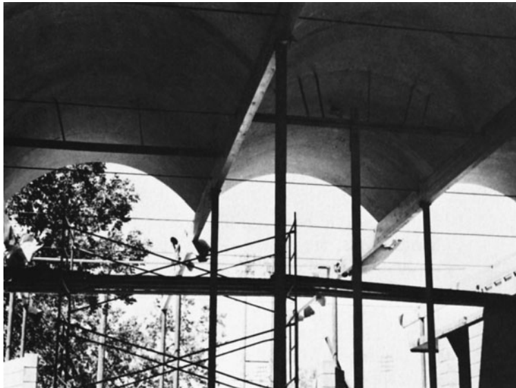
Figure 12-44 Valley Beams under Long-Barrel Shells. (Reprinted with permission of Council of Forest Industries of British Columbia.)
