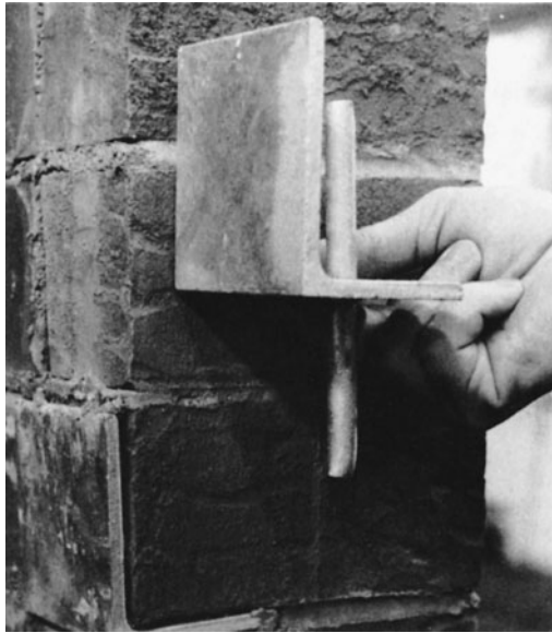
Figure 13-42 Weld Plate for Anchoring Brick Panels to a Structural Frame. (Reprinted by permission of International Masonry Institute.)
