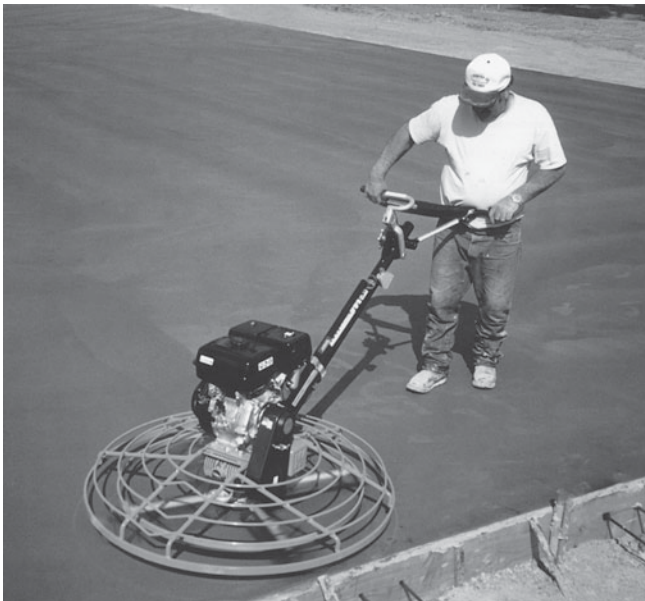
Figure 7-53 Power Trowel in Operation. (Reprinted by permission of Multiquip, Inc.)
