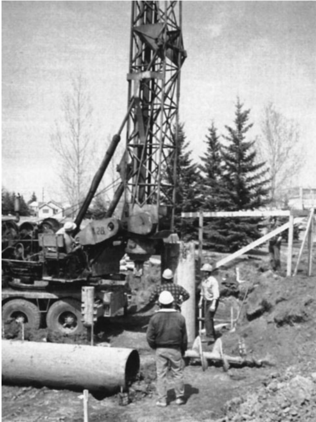
Figure 5-26 Steel Casing Being Used to Line Drill Caisson Shaft.
