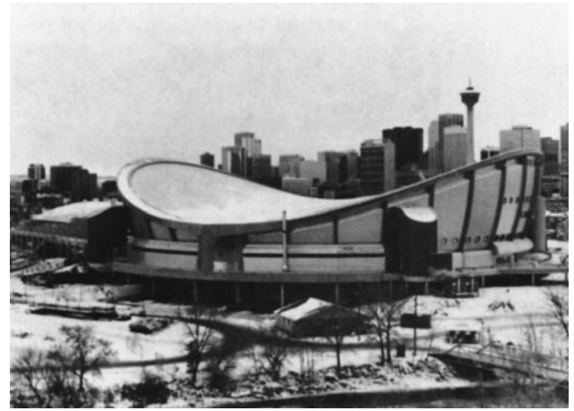
Figure 12-51 Sports Arena with Cable-Supported Roof.
