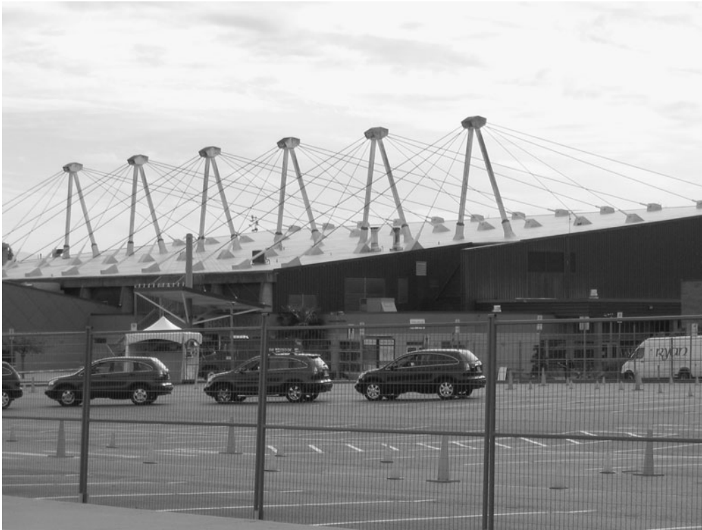
Figure 12-1 Cable-Supported Roof.
