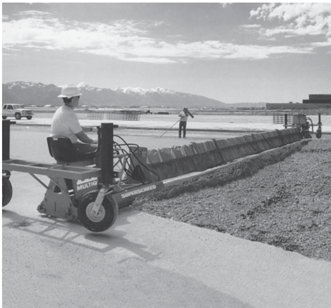
Figure 7-48 Power-Operated Strike-Off Bars. (Reprinted by permission of Multiquip, Inc.)
