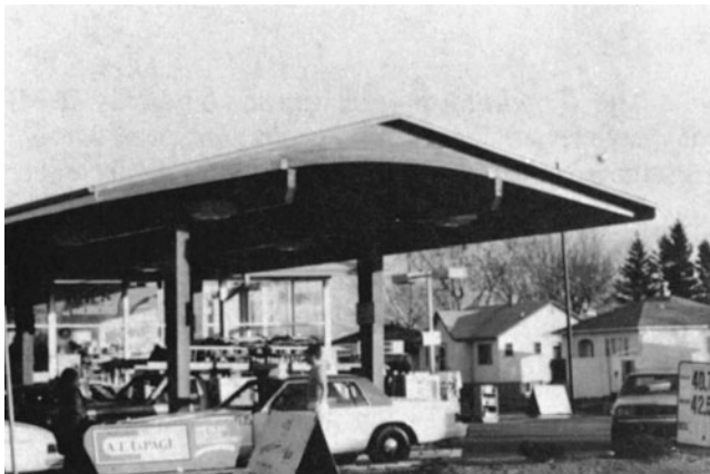
Figure 8-35 Symmetrically Tapered Beam.
