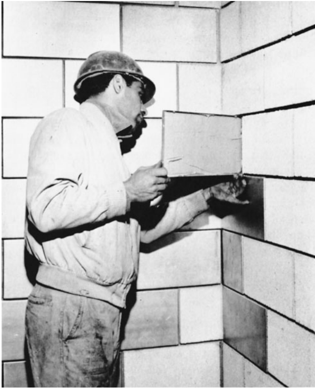
Figure 16-45 Steel Facing Units for Concrete Block.
