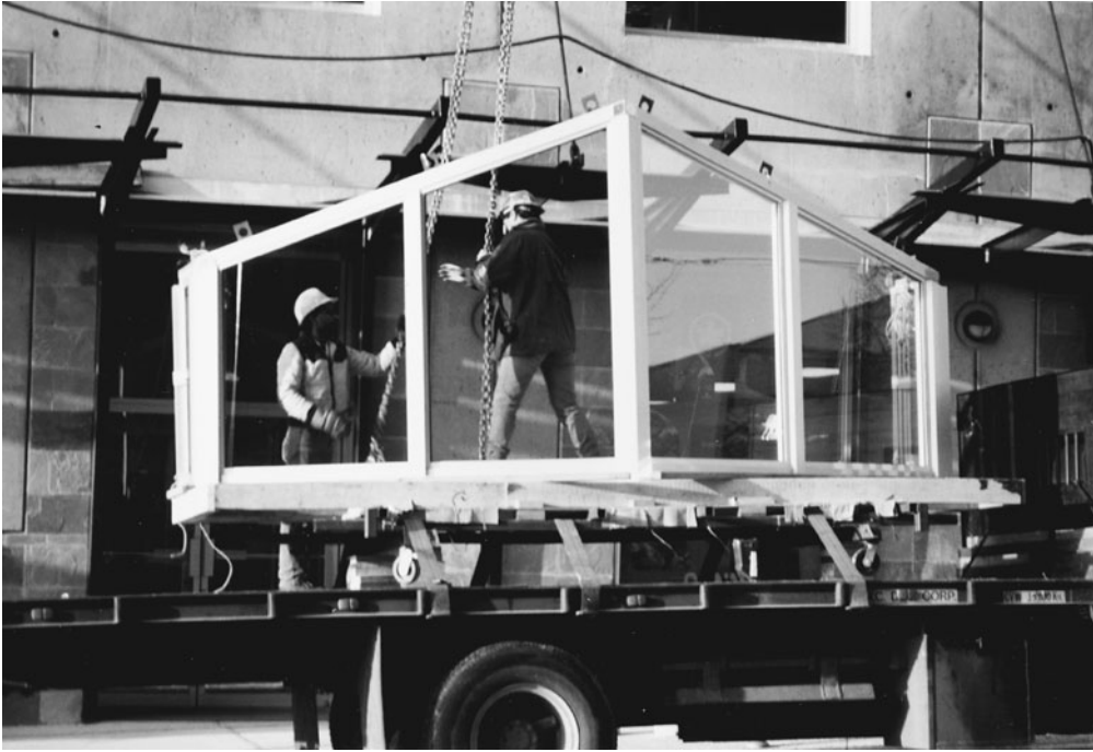
Figure 14-42 Prefabricated Aluminum Frames for Glass Curtain Wall.
