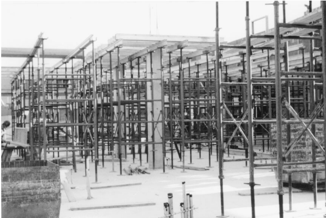
Figure 6-80 Scaffold-Type Shoring Used to Support Structural Slab Formwork.
