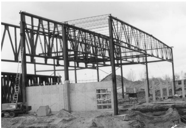
Figure 12-17 Open-Web Joists Serving as Purlins between Steel Trusses.
