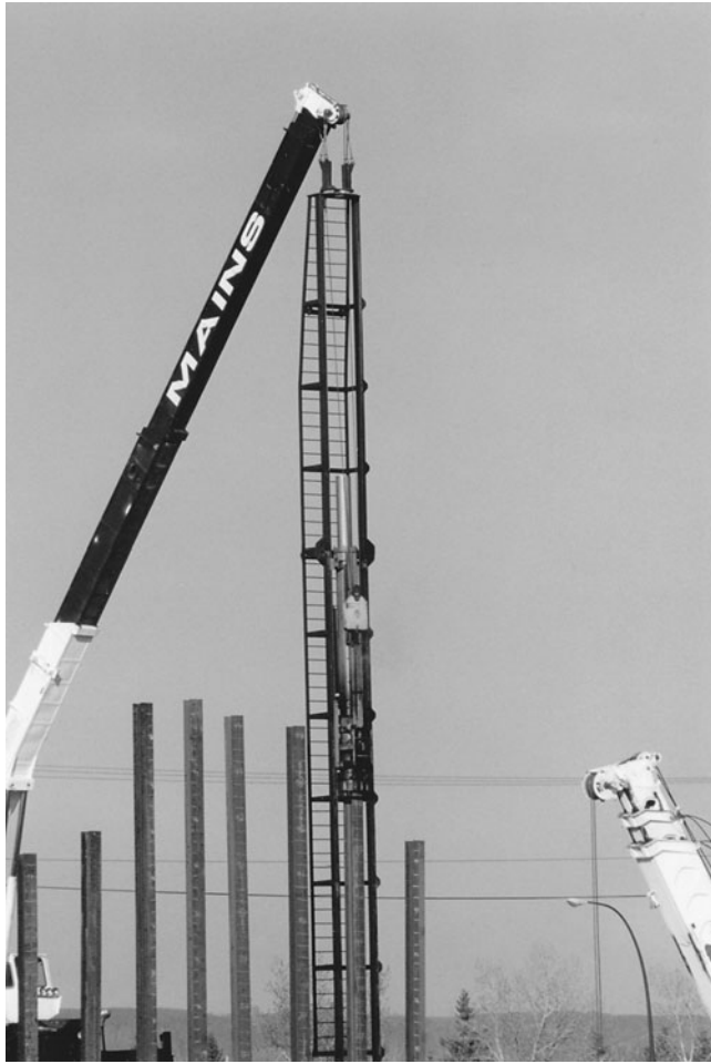
Figure 5-23 Diesel Hammer Driving Steel Bearing Pile.
