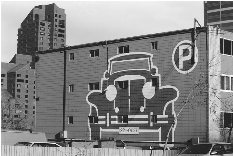
Figure 16-15 Painted Concrete Blocks as Exterior Finish.
