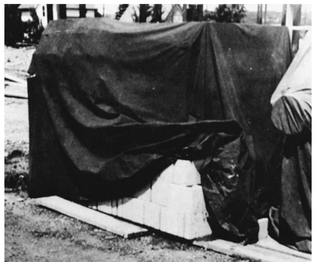
Figure 13-49 Heating Blocks Just Prior to Use. (Reprinted with permission of Portland Cement Association.)
