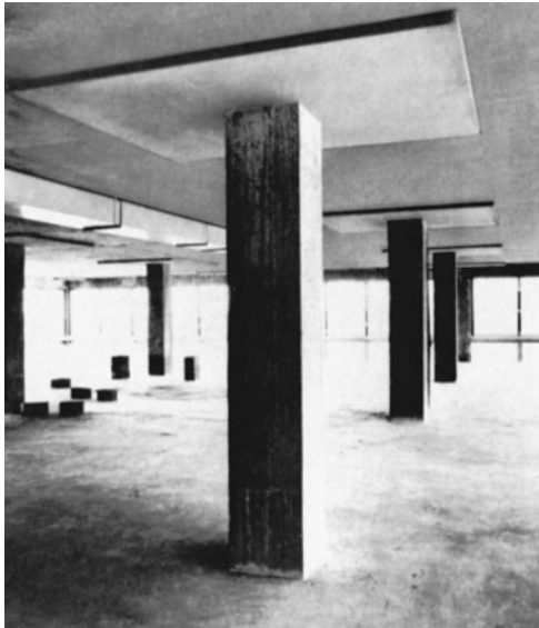
Figure 11-14 Flat-Slab Floor with Drop Panel. (Reprinted with permission of Portland Cement Association.)
