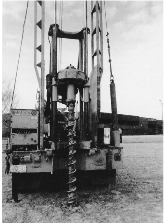
Figure 1-2 Truck-Mounted Drill Rig.
