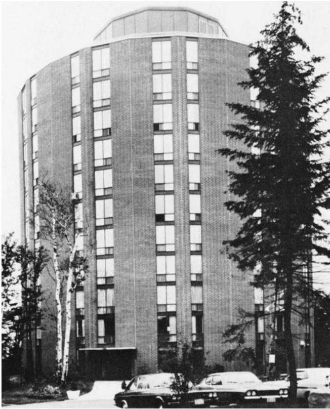
Figure 13-35 Typical Load-Bearing Brick Wall Structure. (Reprinted by permission of International Masonry Institute.)
