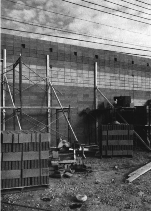
Figure 13-4 Temporary Bracing Supporting Masonry Wall.
