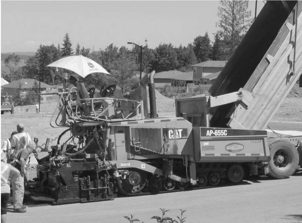
Figure 4-5 Paving Machine Being Loaded from Dump Truck.
