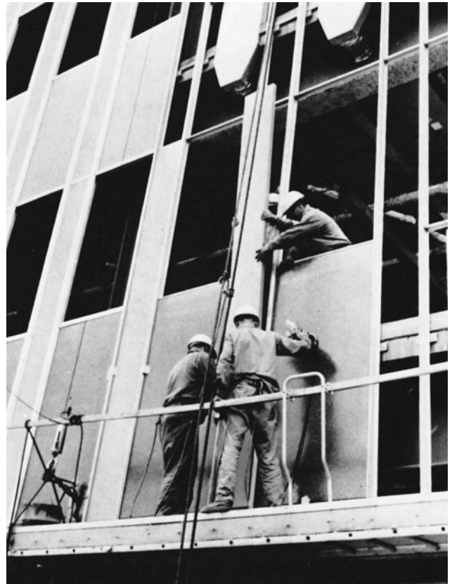
Figure 14-39 Curtain Wall with a Subframe.
