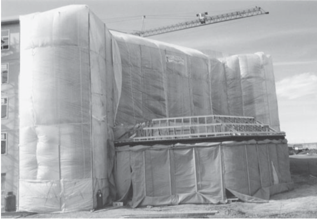
Figure 7-36 Reinforced Polyethylene Film Encloses Building.
