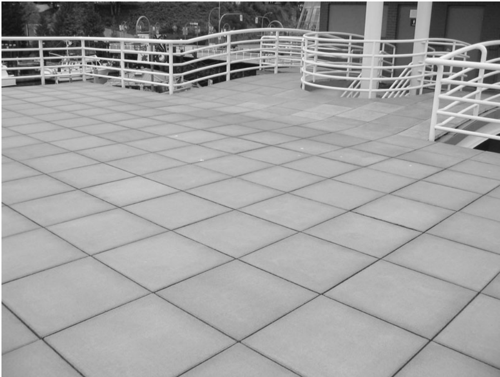
Figure 12-71 Patio Blocks Used as Insulation Protection.
