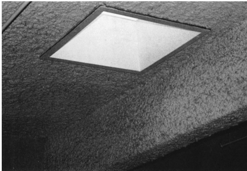
Figure 16-52 Sprayed Insulation Provides Acoustical Treatment to Exposed Concrete Ceiling.
