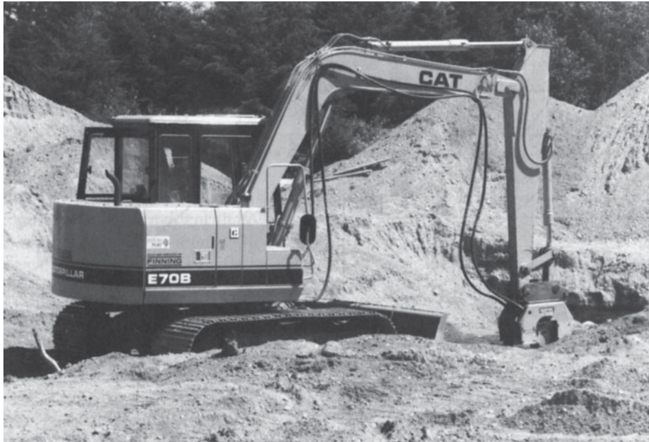
Figure 7-16 Compacting Subgrade.
