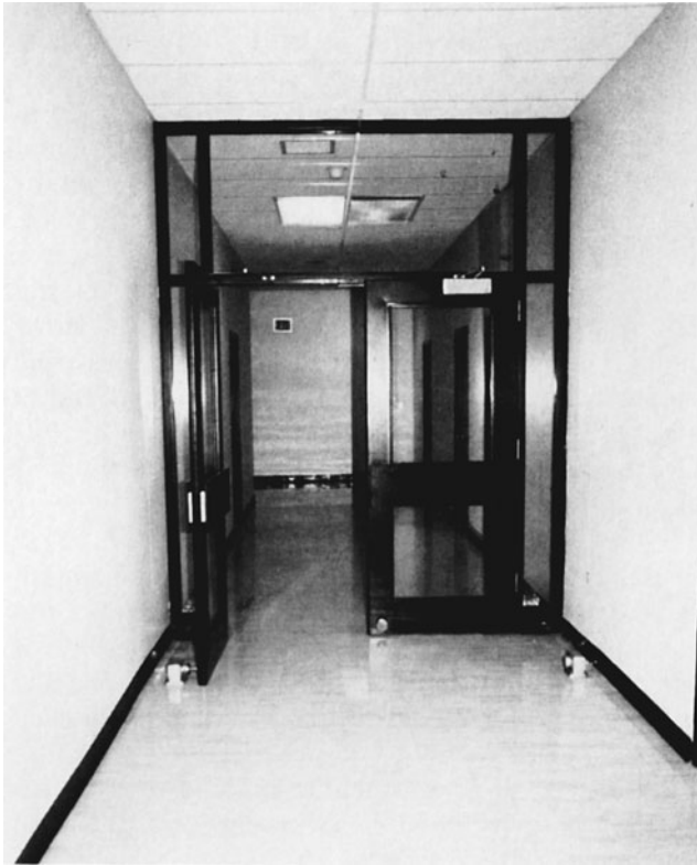
Figure 16-34 Walls Covered with Drywall and Vinyl Floors Provide Smooth, Durable Surfaces for Institutional Buildings.
