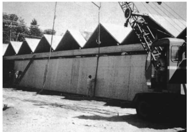
Figure 8-59 Folded Plate Roof of Stressed-Skin Panels.
