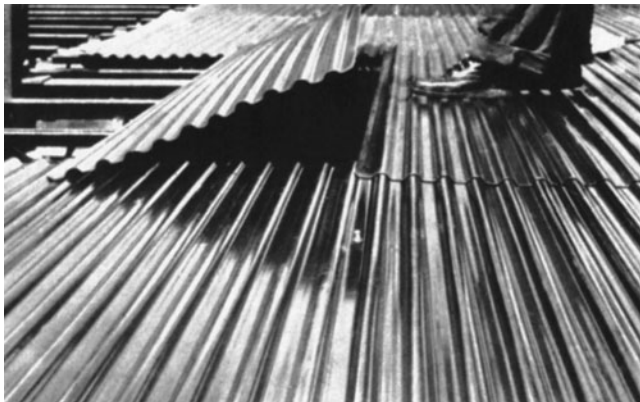
Figure 11-50 Corrugated Sheet Steel Decking.
