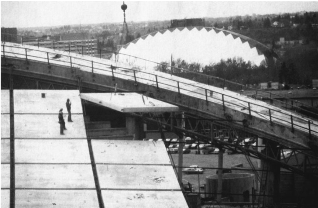
Figure 12-53 Precast Panels Being Placed on Supporting Cables.
