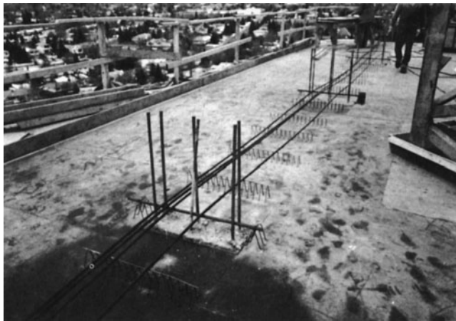
Figure 11-22 Posttensioning Cables Being Positioned on Chairs.
