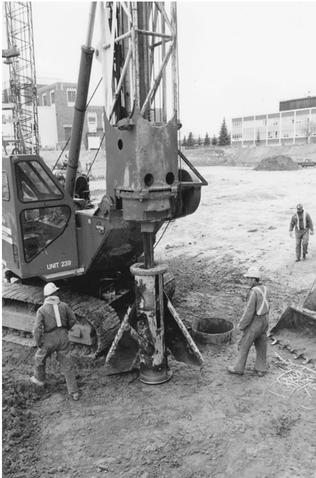
Figure 5-12 Belling Equipment for Pile Bottoms.
