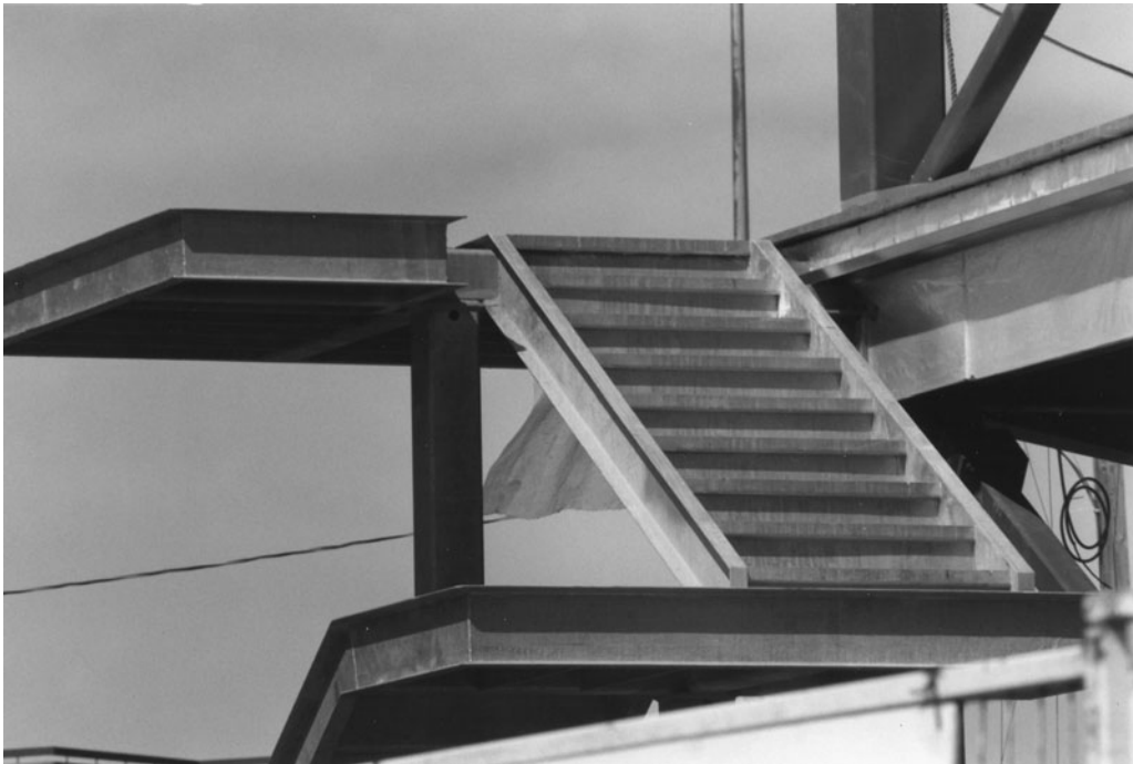
Figure 10-7(b) Channel Sections Used as Stair Stringers.
