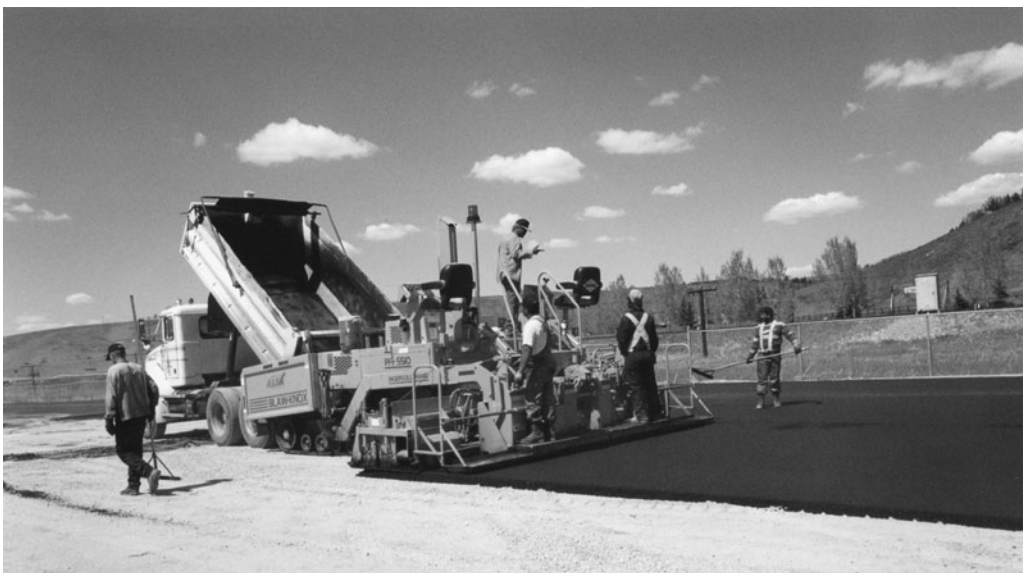
Figure 4-15 Hot-Mix Asphalt Surface Being Placed on Prepared Base.
