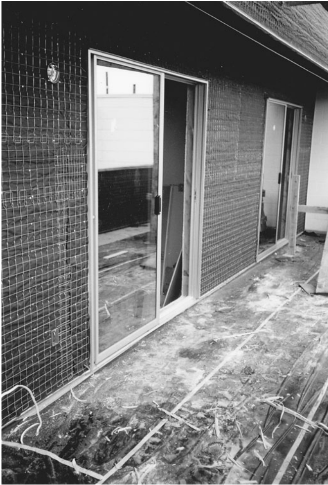
Figure 16-7 Exterior Wall Covered with Building Paper and Stucco Wire.
