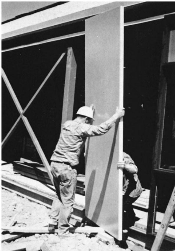
Figure 14-37 Steel Sandwich Panels Being Installed.
