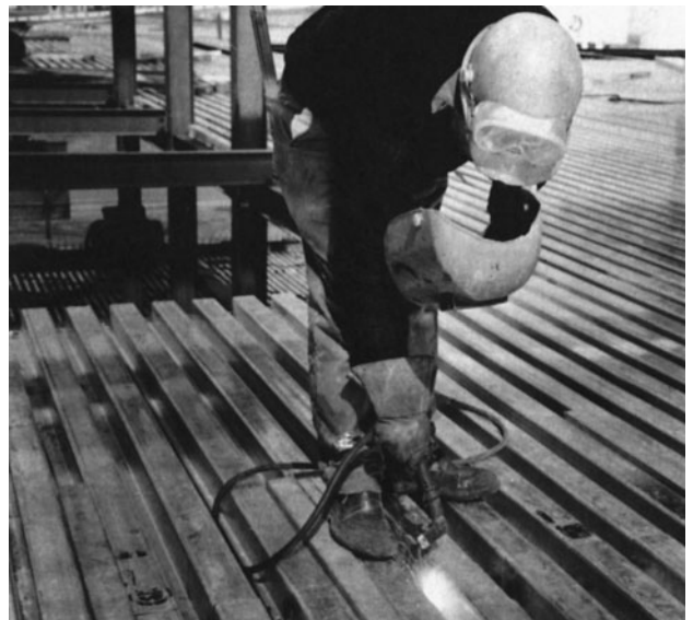
Figure 11-52 Spot-Welding Steel Deck. (Reprinted by permission of Bethlehem Steel Co.)
