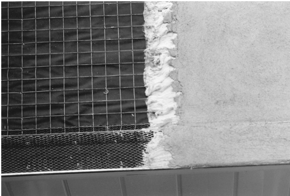
Figure 16-8 Synthetic Stucco Application.
