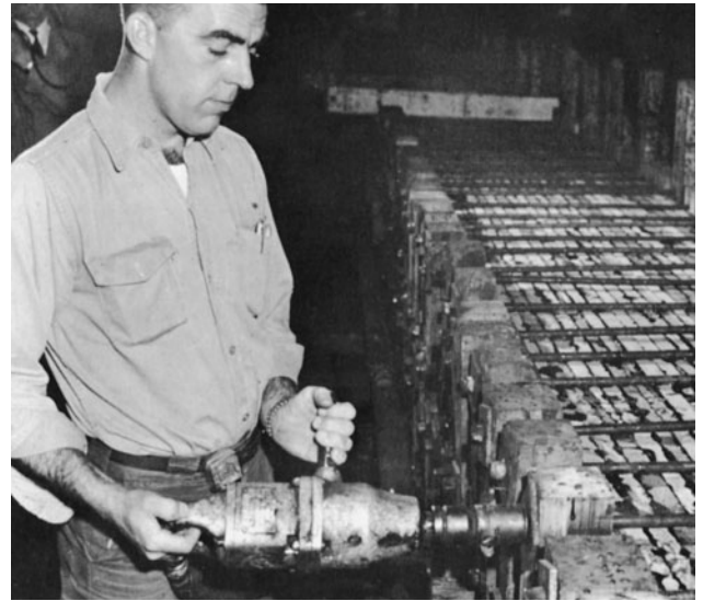
Figure 8-30 Tightening Clamp Bolts with an Air-Operated Impact Wrench. (Reprinted by permission of Canadian Wood Council.)
