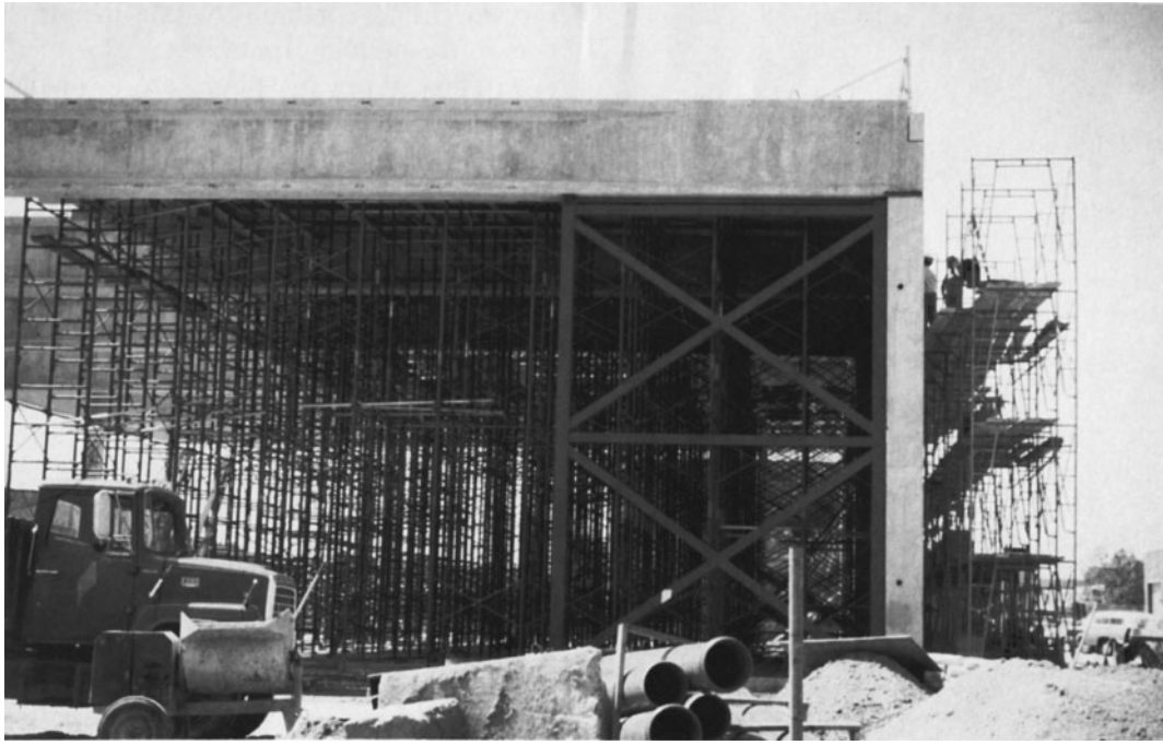
Figure 9-3 Structural Steel Cross-Bracing Provides Lateral Stability for Precast Concrete Structure.
