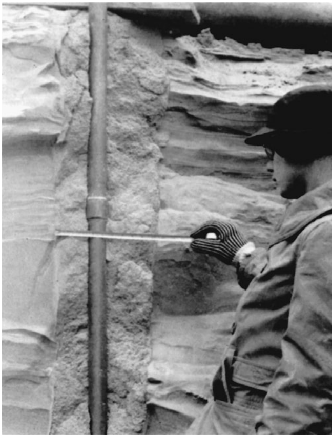
Figure 3-10 Properly Sanded Well-Point. (Reprinted by permission of Moretrench American Corporation.)
