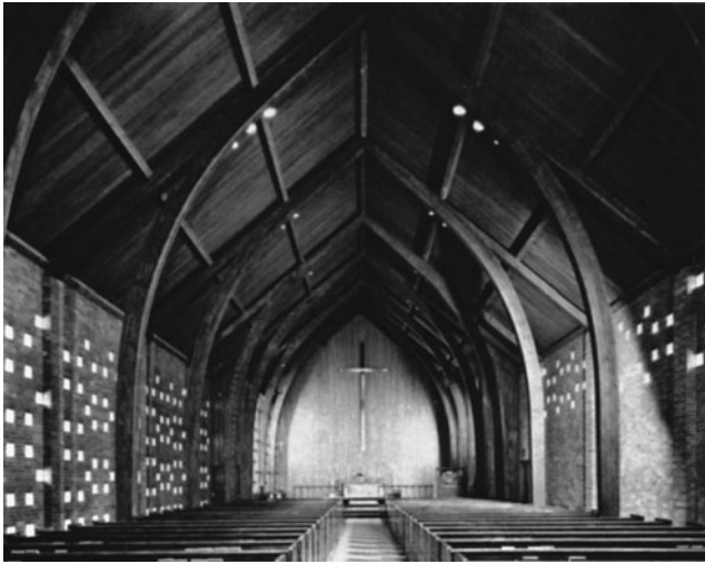
Figure 8-40 Arches with Straight Top End. (Reprinted by permission of American Institute of Timber Construction.)
