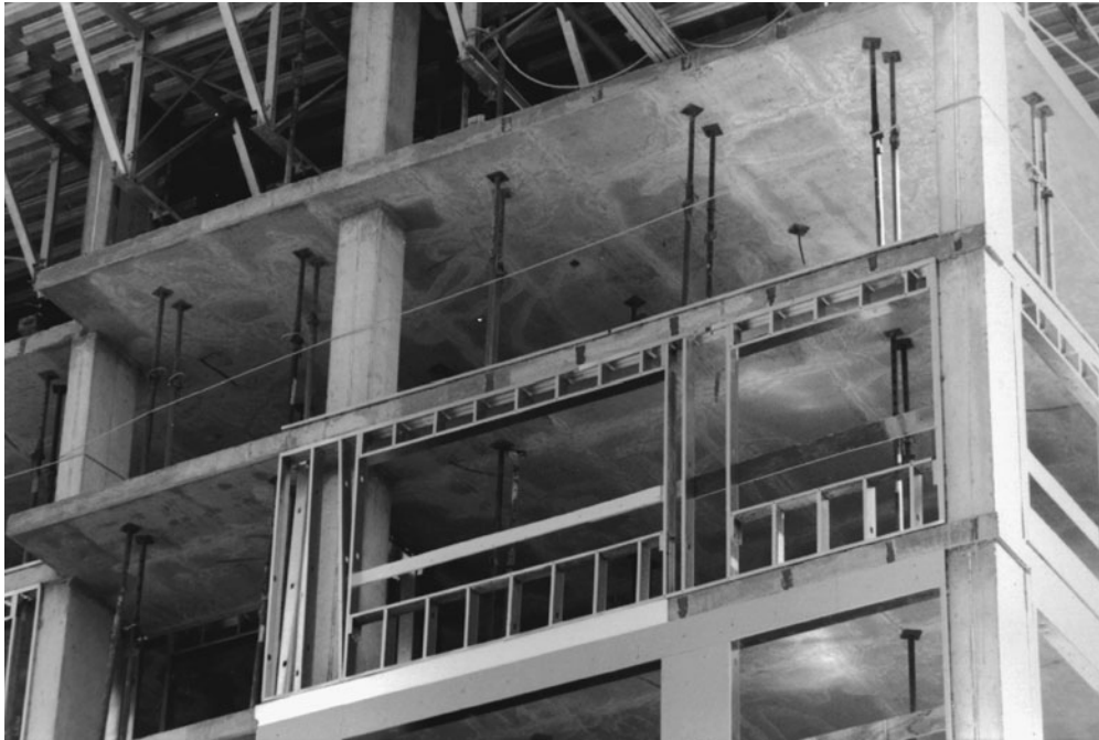
Figure 6-82 Reshoring in a Multistory Structure.
