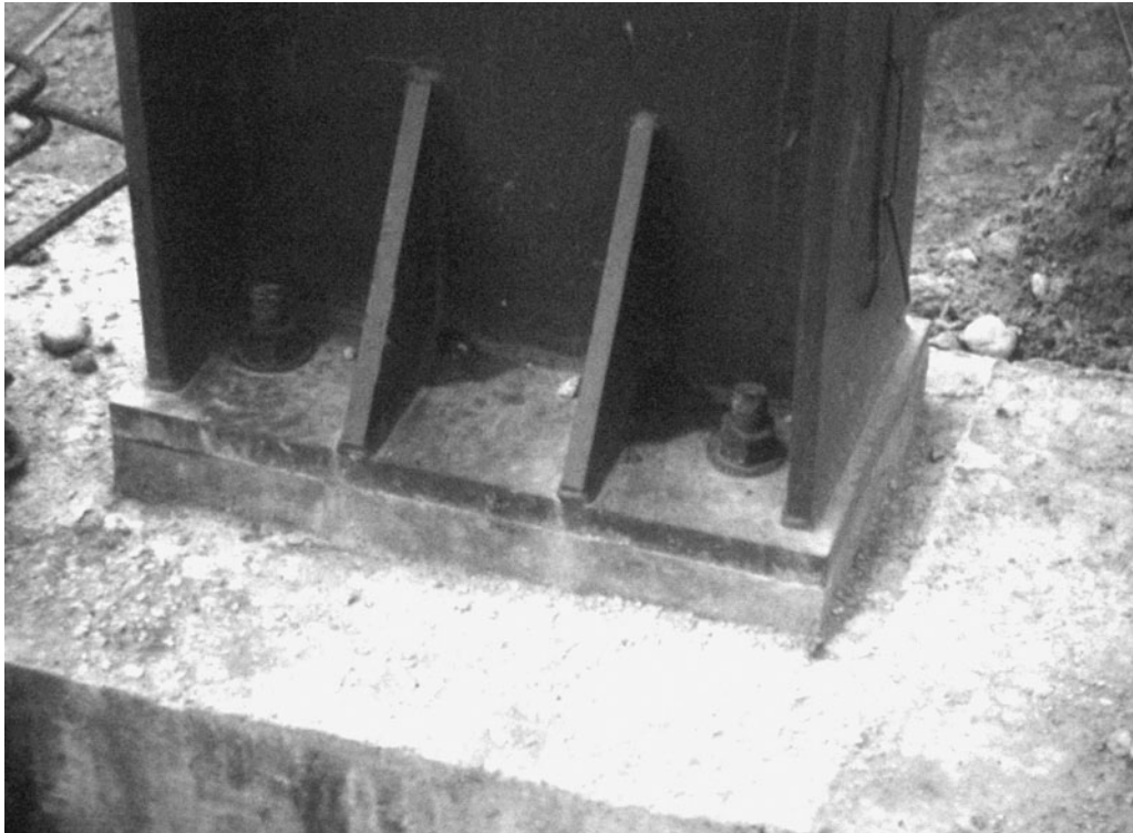
Figure 10-47 Grouted Column Base Plate.
