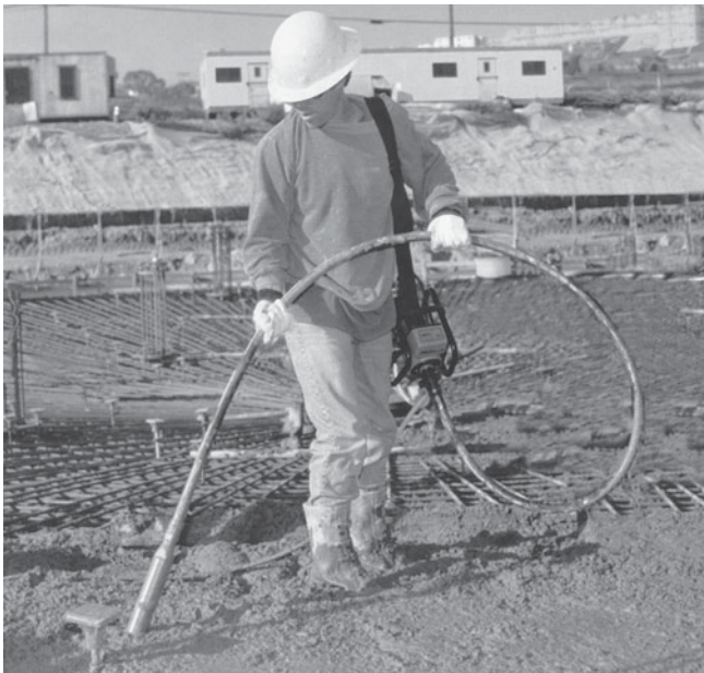
Figure 7-32 Gasoline-Powered Internal Vibrator. (Reprinted by permission of Multiquip, Inc.)
