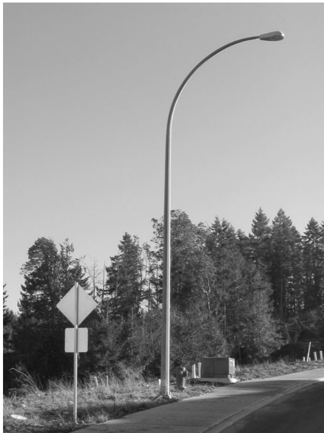
Figure 4-21 Cobra-Head-Style Street Light Standard.
