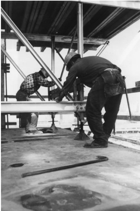
Figure 6-76 Flying Form Frame and Jacks. (Reprinted by permission of Aluma Enterprises, Inc.)
