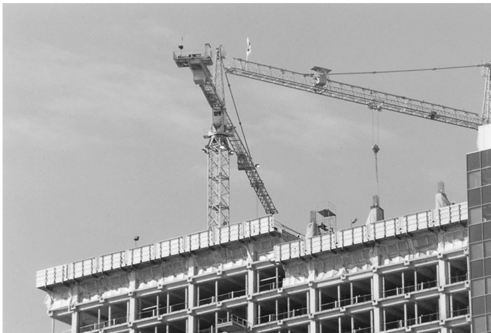
Figure 10-45 Tower Cranes on Top of a High-Rise Building.
