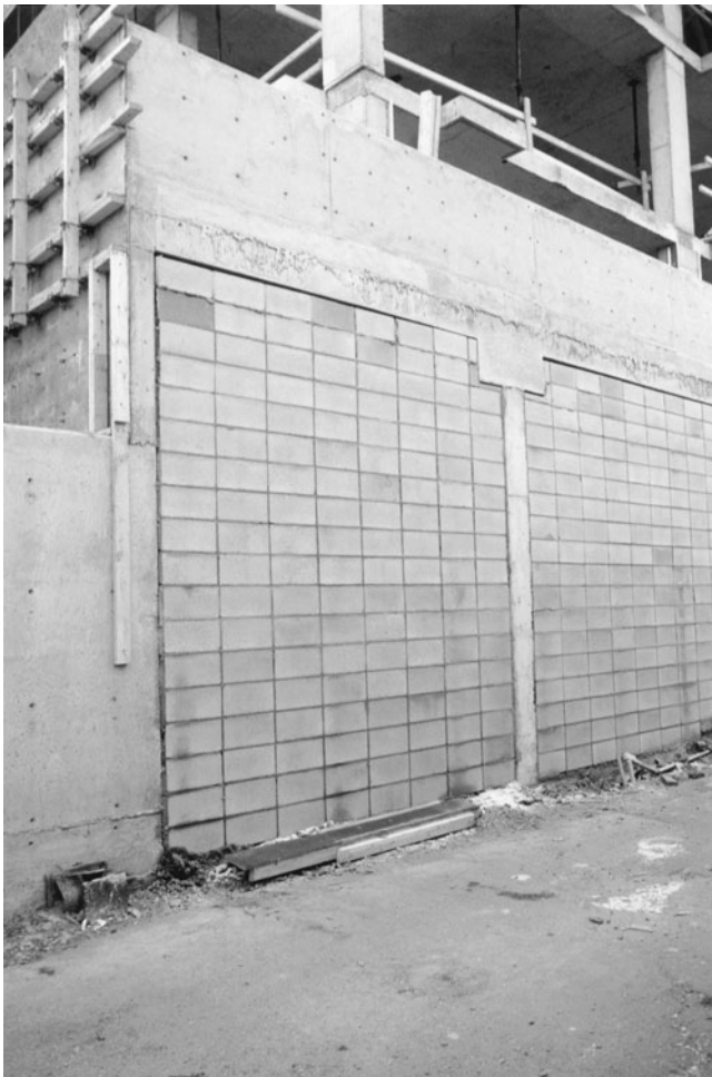
Figure 14-4 Non-Load-Bearing Lightweight Concrete Block Curtain Wall.
