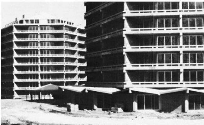
Figure 13-36 Brick Building with Interior Bearing Walls. (Reprinted by permission of International Masonry Institute.)
