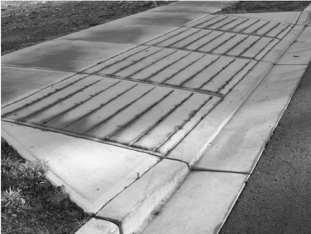
Figure 4-14 Driveway Ramp from Street.
