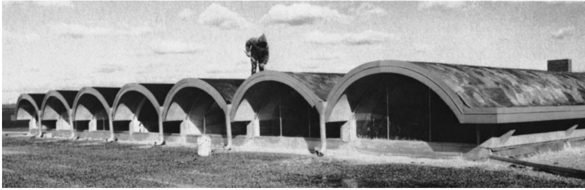
Figure 8-62 Plywood Vaulted Roof. (Reprinted with permission of Council of Forest Industries of British Columbia.)
