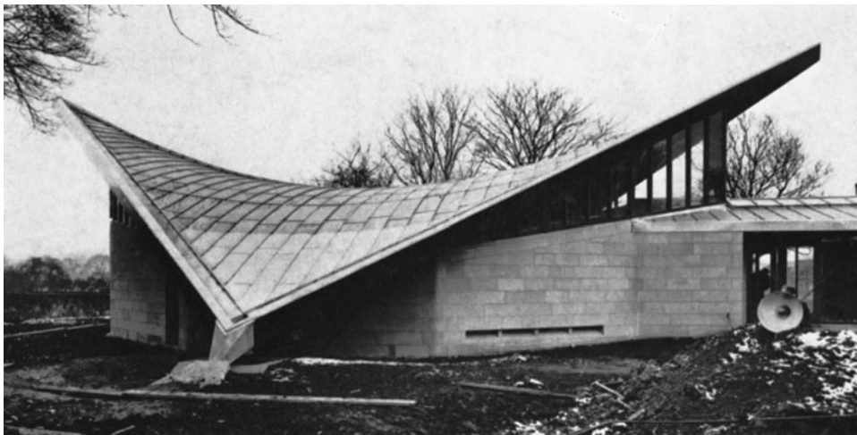
Figure 12-47 H/P Saddle-Shaped Roof.
