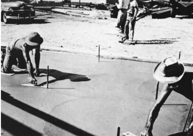
Figure 14-30 Finishing Tilt-Up Panel. (Reprinted with permission of Portland Cement Association.)
