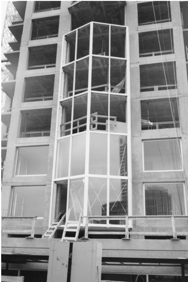
Figure 16-27 Aluminum-Frame Window Wall.
