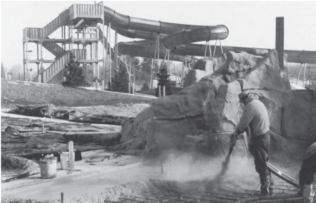
Figure 7-47 Shotcrete Application. The Rocks in the Background Were Also Formed Using Shotcrete. (Reprinted by permission of Allentown Equipment.)
