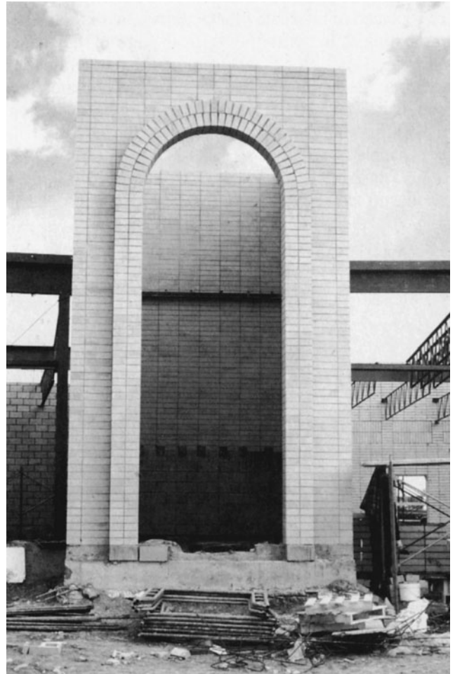
Figure 13-26 Main Entrance to Building of Load-Bearing Brick.
