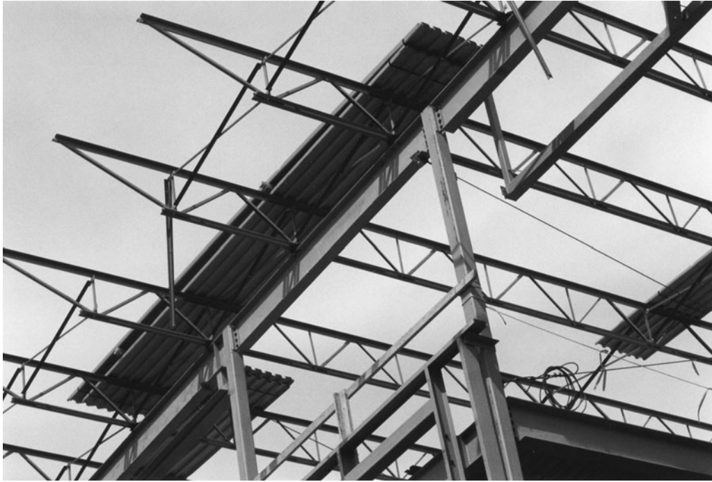
Figure 12-4 Columns Supporting Roof Beams, Roof Beams Supporting Joists, Joists Supporting Roof Decking.
