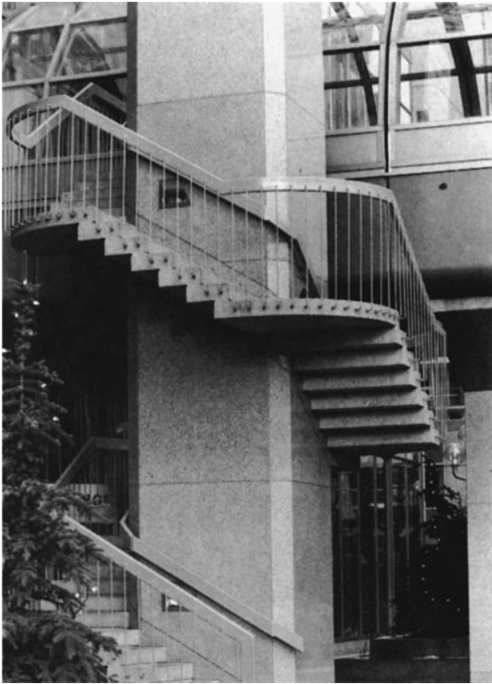
Figure 16-59 Cantilevered Concrete Stair.
