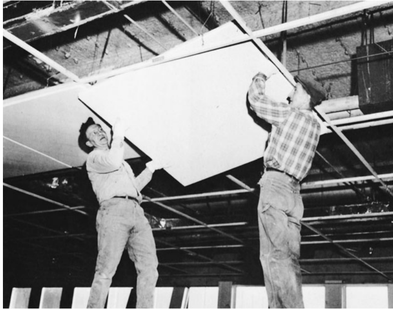
Figure 16-49 Suspended Ceiling System.
