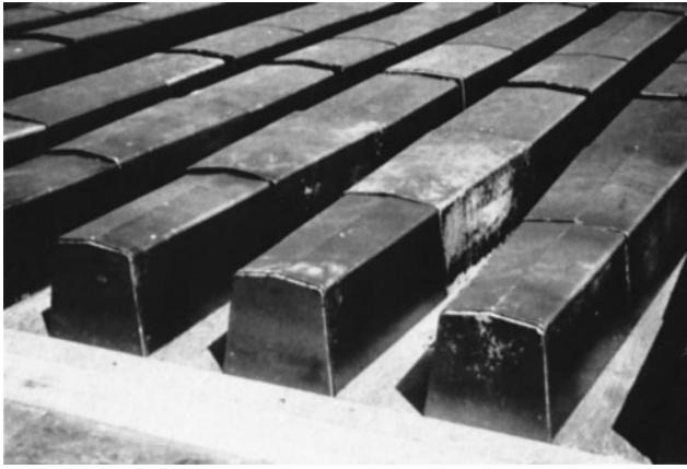
Figure 11-29 Pans for One-Way Joist System in Place.
