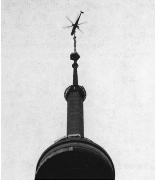
Figure 10-50 Sikorsky Sky-Crane Placing Steel Antenna Sections Atop a Tower. (Reprinted by permission of Canadian Institute of Steel Construction.)
