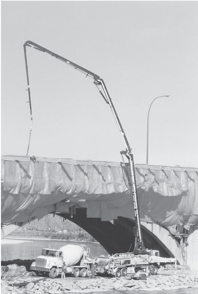
Figure 7-25 Hydraulic Boom Allows Concrete Placement on a Difficult Site.
