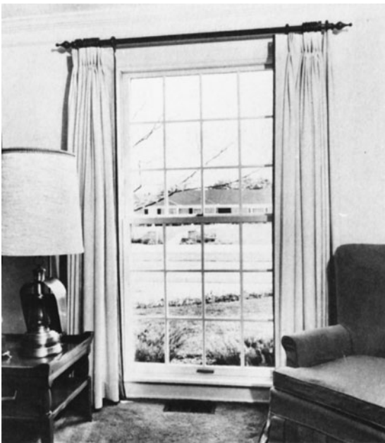
Figure 16-30 Typical Wood Sash Apartment Window.
