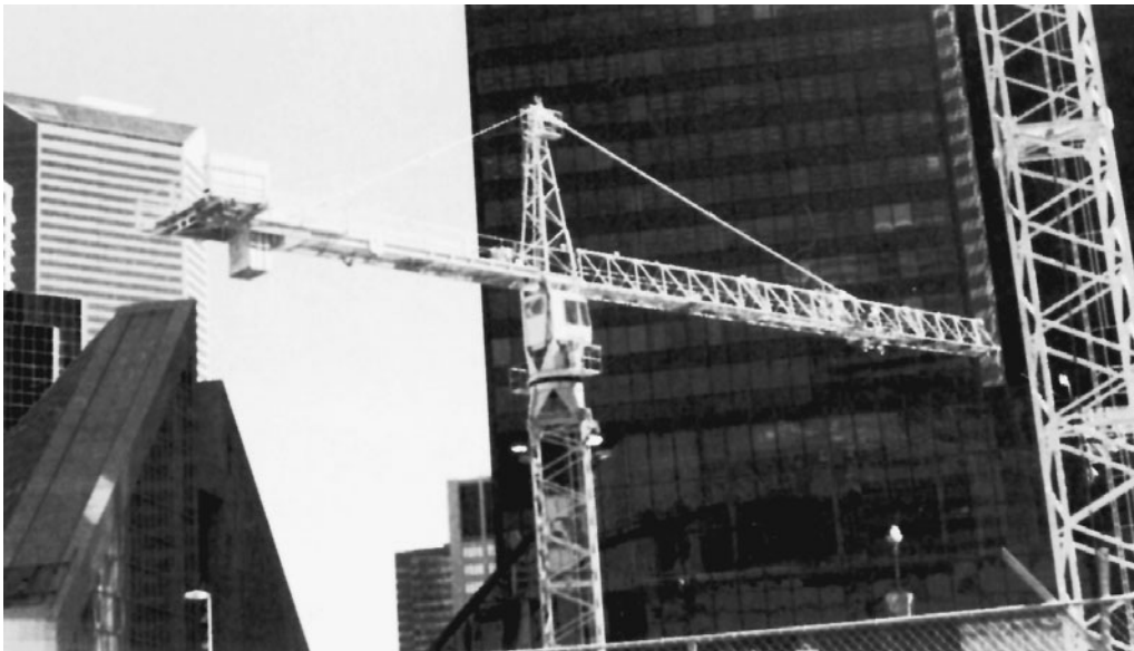
Figure 3-14 Tower Crane in a Downtown Construction Site.
