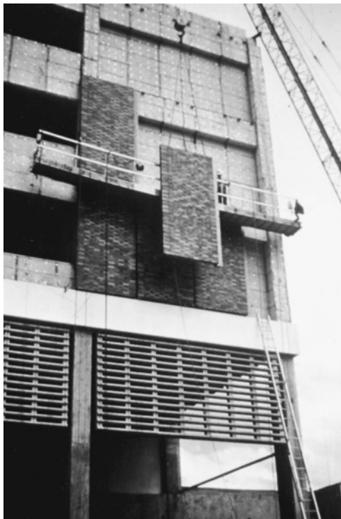
Figure 13-40 Precast Brick Facing Panels Being Set in Place.
