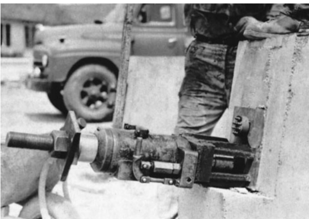
Figure 9-33 Hydraulic Tensioning Jack. (Reprinted with permission of Portland Cement Association.)
