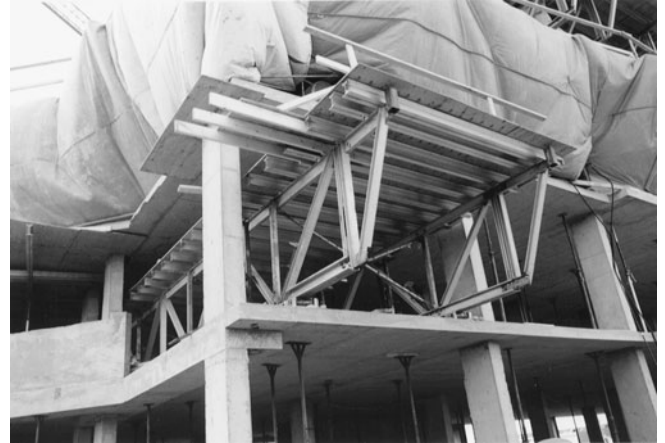
Figure 6-77 Section of Fly Form on Rollers, Ready to Be Moved.
