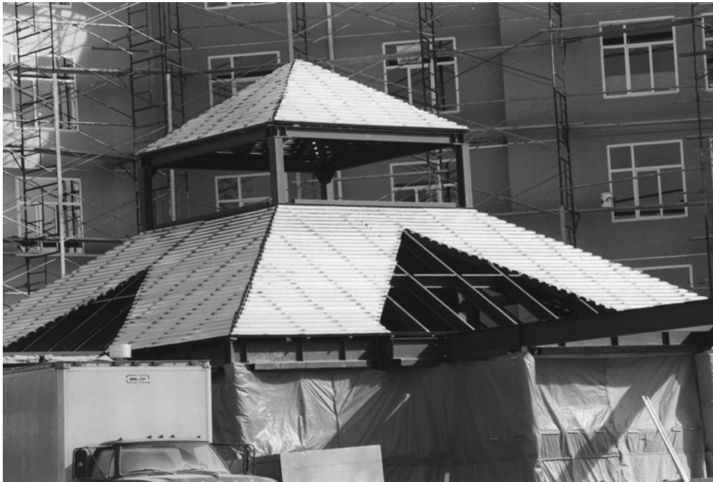
Figure 12-56 Steel Roof Decking.
