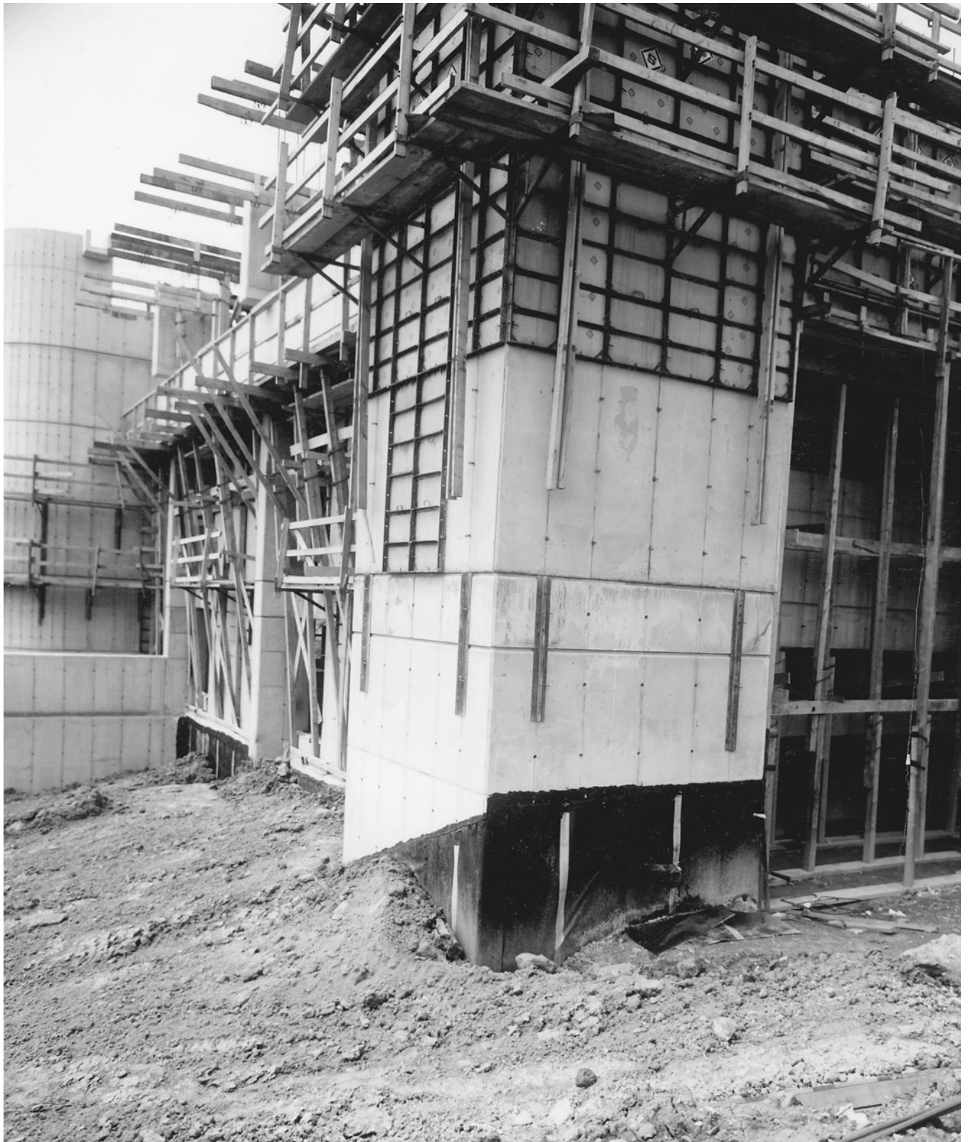
Figure 6-42 Formwork Panels Supported by Double 2" × 4" (38 × 89 mm) Wales.
