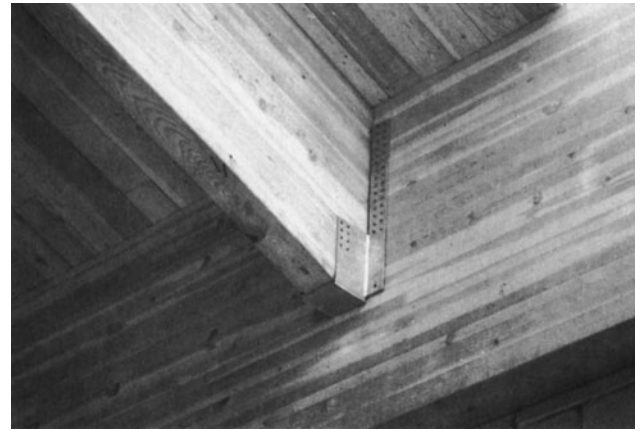
Figure 8-44 Intermediate Glulam Beam Supported on Metal Hanger Fastened to Main Girder with Glulam Rivets. (Reprinted by permission of Canadian Wood Council.)
