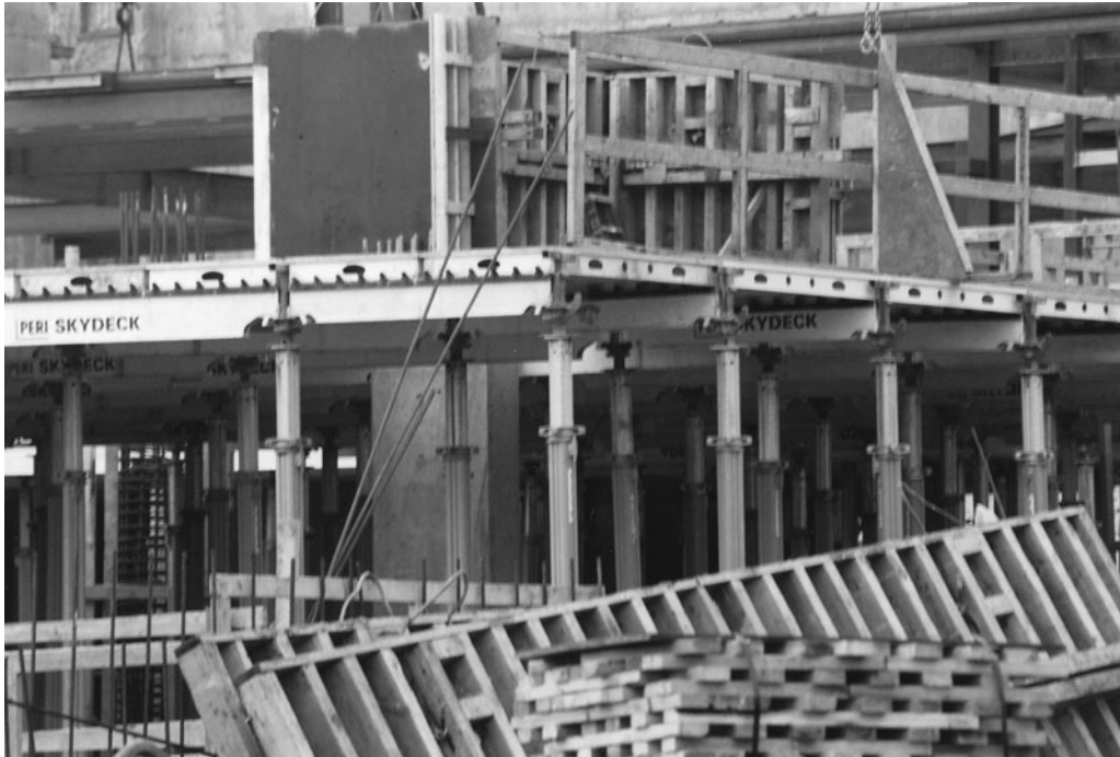
Figure 11-40 Metal Screw-Type Shore.
