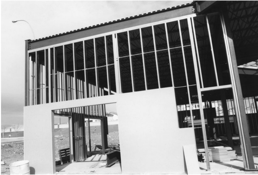
Figure 10-13 Cold-Formed Metal Studs Supporting Exterior-Grade Drywall Sheathing.
