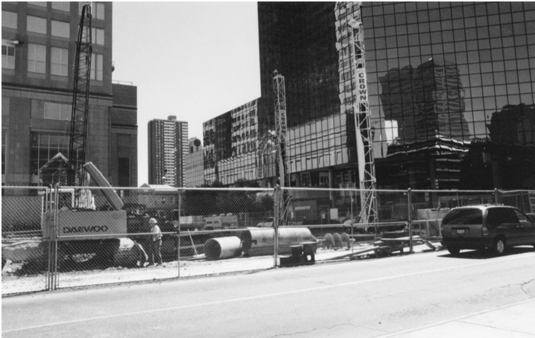
Figure 1-19 Proper Protection for the Public around a Building Site Is Paramount.
