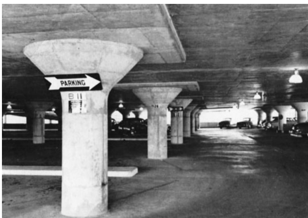
Figure 11-15 Column Capital. (Reprinted with permission of Portland Cement Association.)
