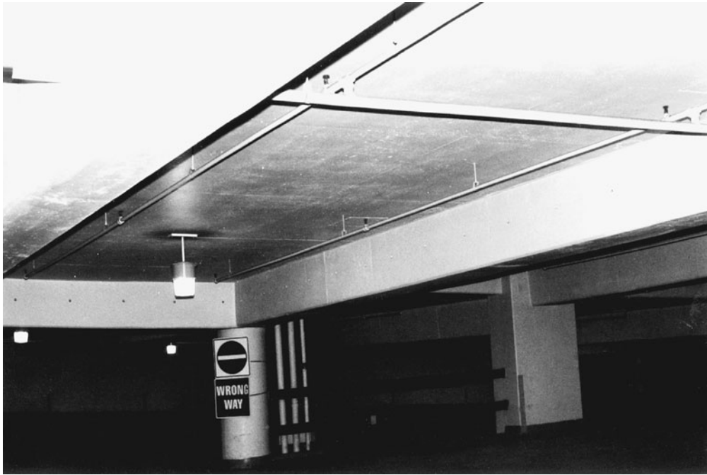
Figure 11-12 Beam-and-Slab Floor.
