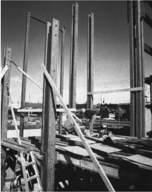
Figure 8-51 Parallel-Strand Sections Are Straight and Can Be Cut to Any Length. (Reprinted by permission of Trus Joist, a Weyerhaeuser business.)
