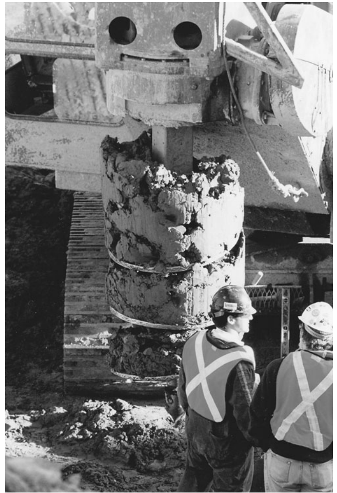
Figure 5-13 Drill Loaded with Earth.
