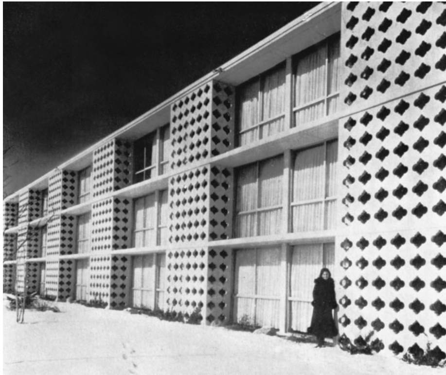
Figure 13-16 Screen Block Wall. (Courtesy of National Concrete Masonry Association.)
