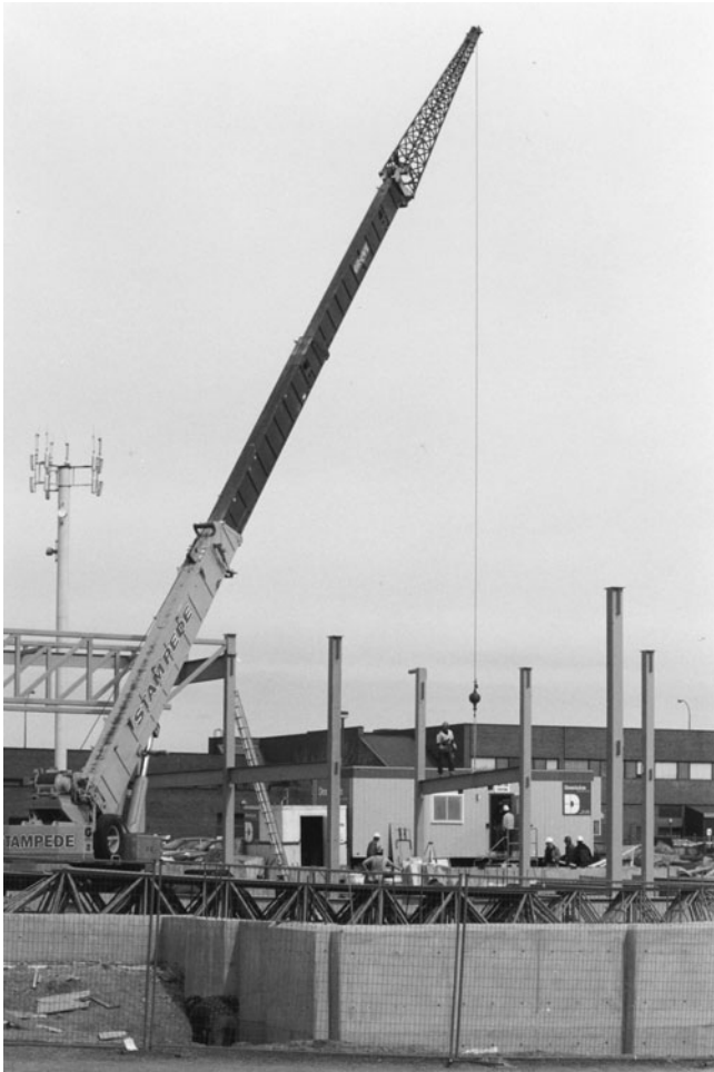
Figure 10-44 Erecting Structural Steel with Mobile Crane.
