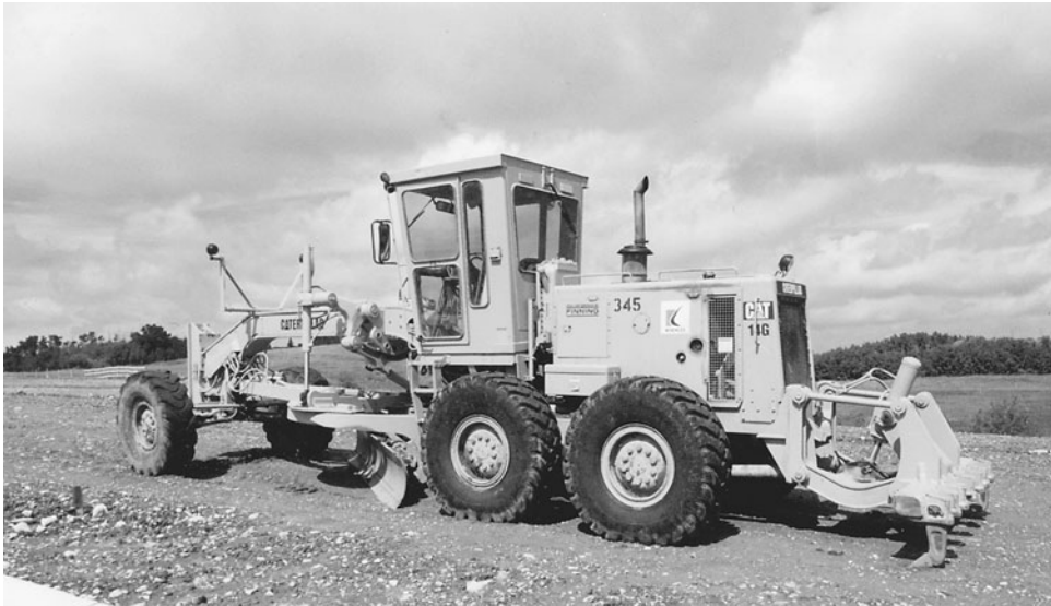
Figure 3-30 Grader Used for Leveling Granular Base Material in Parking Area.
