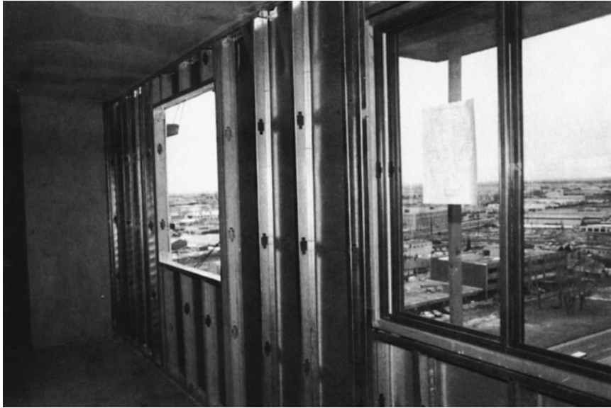
Figure 16-1 Curtain Wall Framing Ready for Insulation and Interior Finish.
