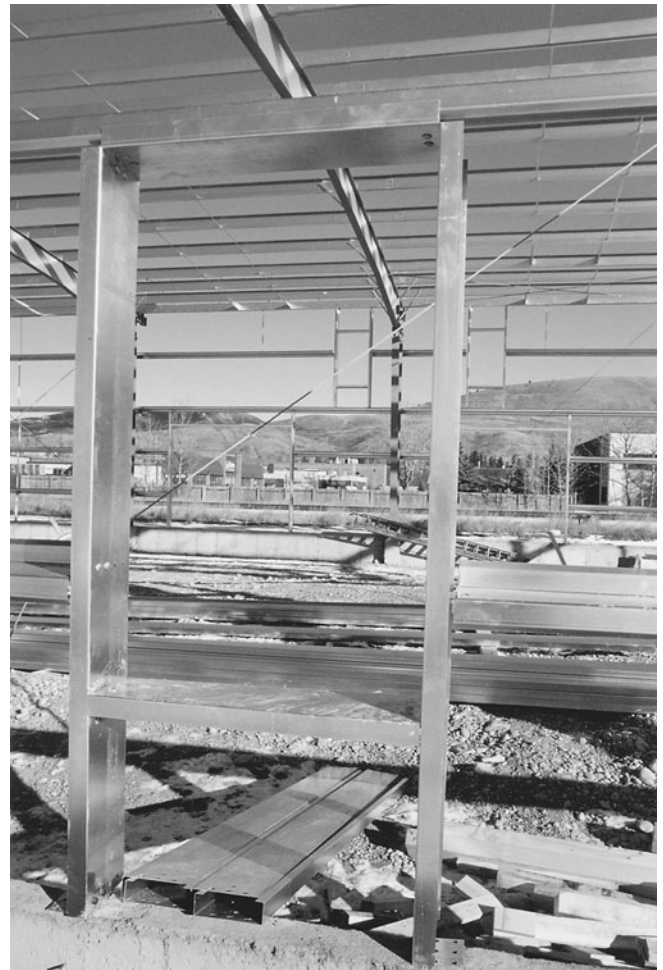
Figure 10-19 Cold-Formed Gauge Material C Shapes.
