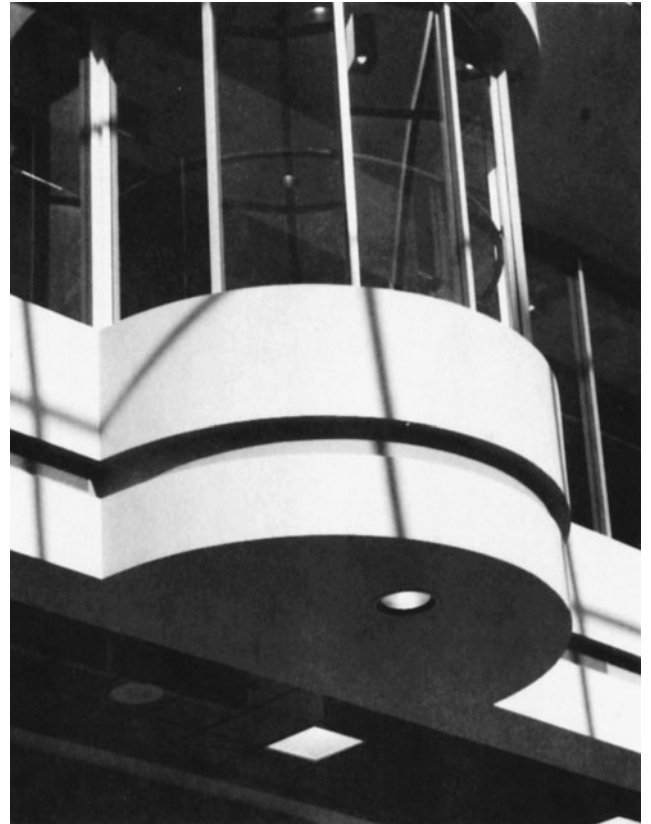
Figure 16-37 Gypsum Board Is an Easily Applied Material That Provides a Smooth Finish.
