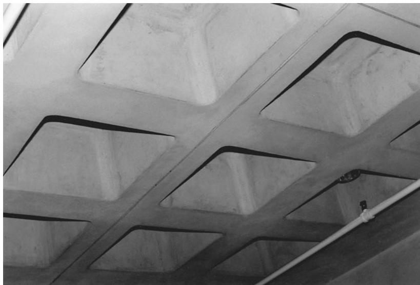
Figure 16-48 Underside of Waffle Slab as Finished Ceiling.
