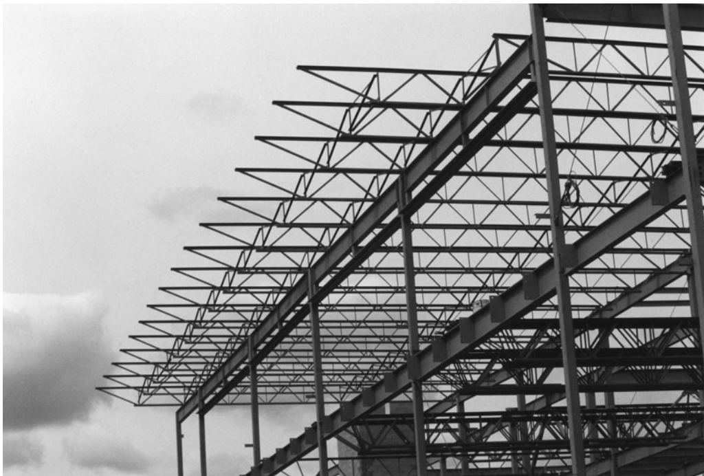
Figure 10-33 Preengineered Open-Web Steel Joists.
