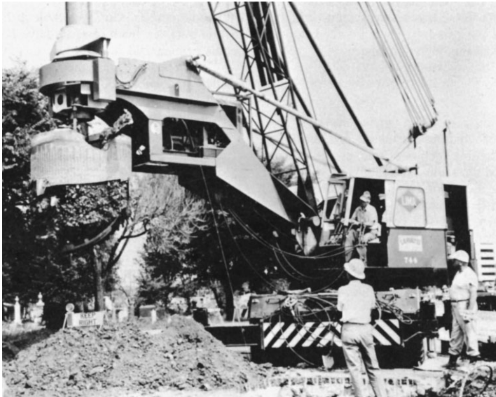
Figure 5-25 Six-Foot (1.8-Metre) Drilling Bucket with Reamers. (Reprinted by permission of Calweld, Inc.)
