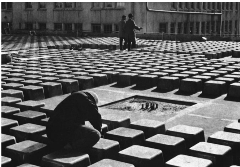
Figure 6-71 Waffle Slab Floor Forms.
