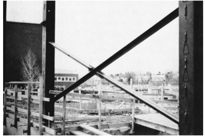
Figure 10-39 Double-Angle Cross-Bracing.
