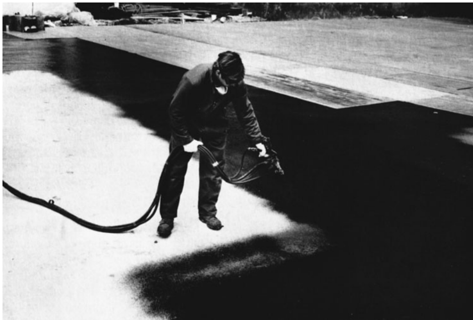
Figure 12-74 Polysulfide Polymer Waterproofing Being Applied by Spray. (Reprinted with permission of ATK Thiokol Propulsion.)
