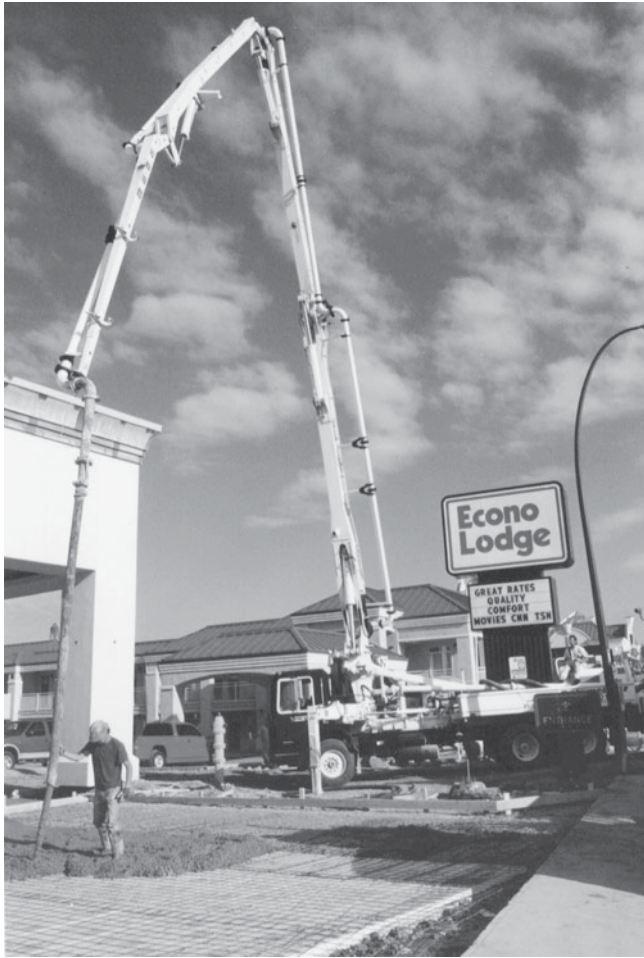
Figure 7-29 Using a Flexible Hose to Minimize the Free Fall of Concrete.
