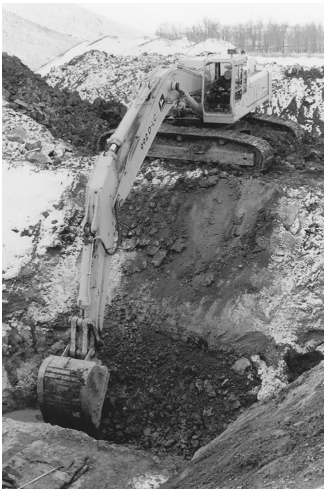
Figure 3-2 Excavator Clearing Out Excavation for Footing.
