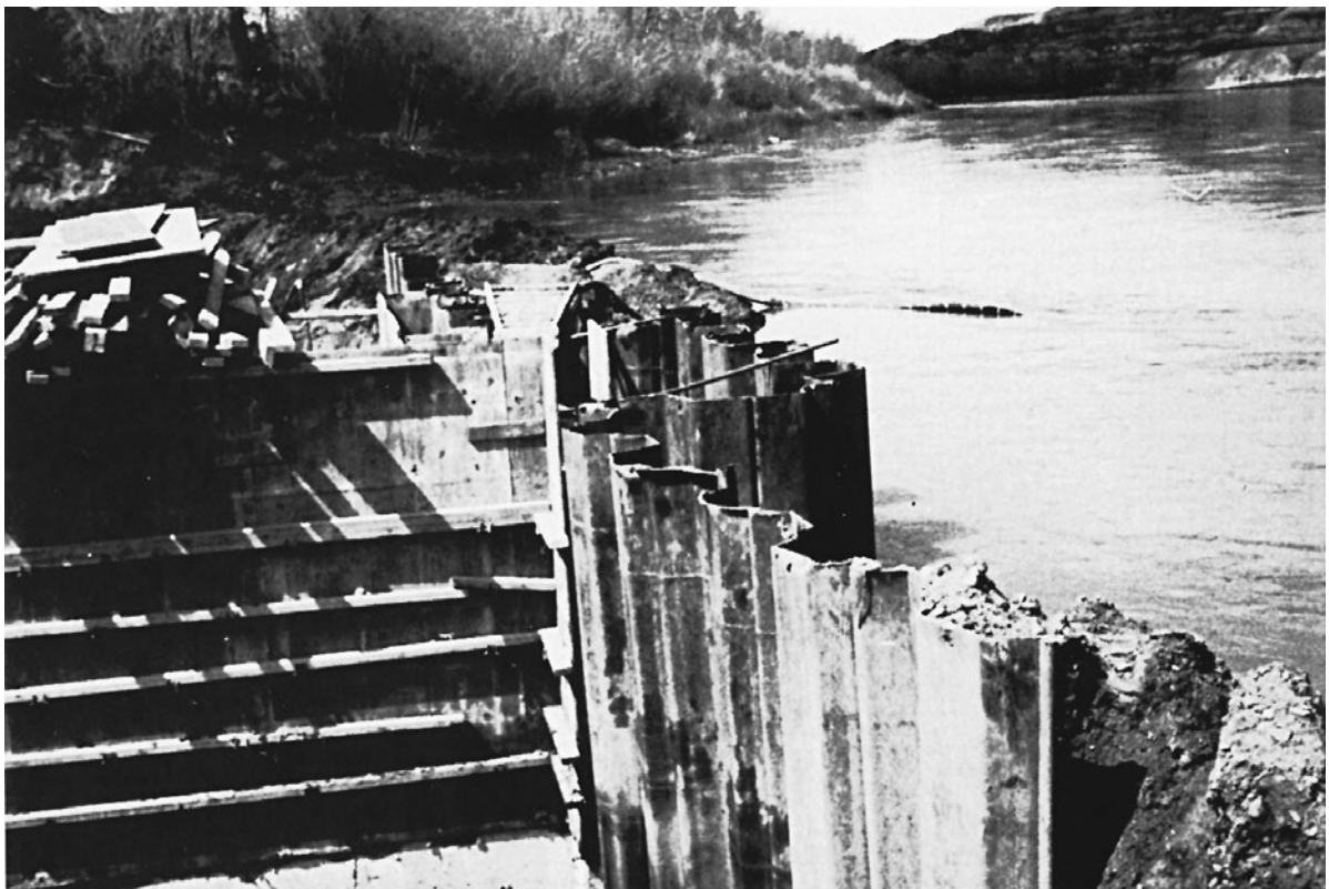
Figure 3-51 Steel Sheet Piling Providing Protection for Excavation Near Water's Edge.
