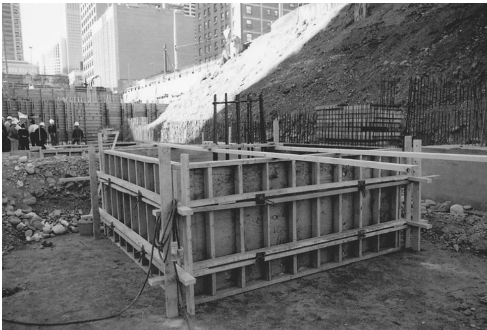
Figure 6-13 Double 2" × 4"s (38 × 89s) Used as Wales.
