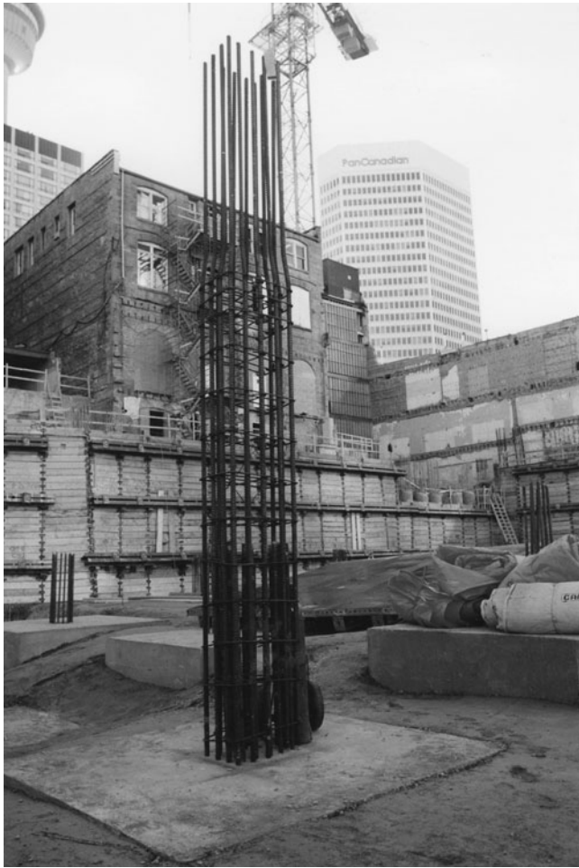
Figure 5-1 Building Site Surrounded by Existing Buildings.
