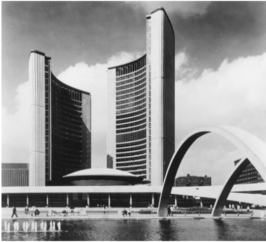
Figure 9-45 Toronto City Hall in Architectural Precast Concrete. (Reprinted by permission of Precast/Prestressed Concrete Institute.)
