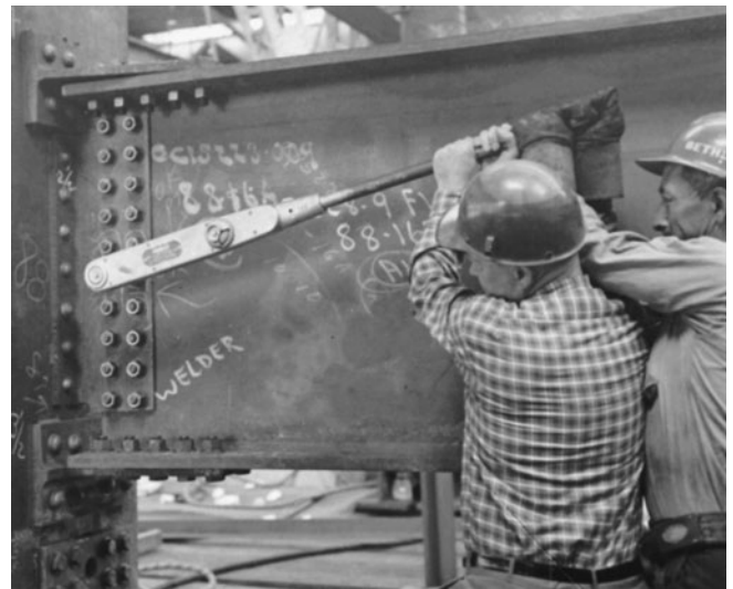
Figure 10-53 Checking Tension of High-Strength Bolts with Torque Wrench. (Reprinted by permission of Bethlehem Steel Co.)
