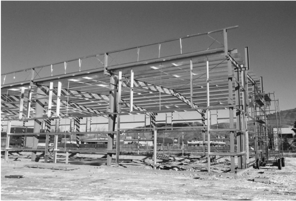
Figure 12-25 Rigid-Frame Building with Cold-Rolled Roof Purlins.
