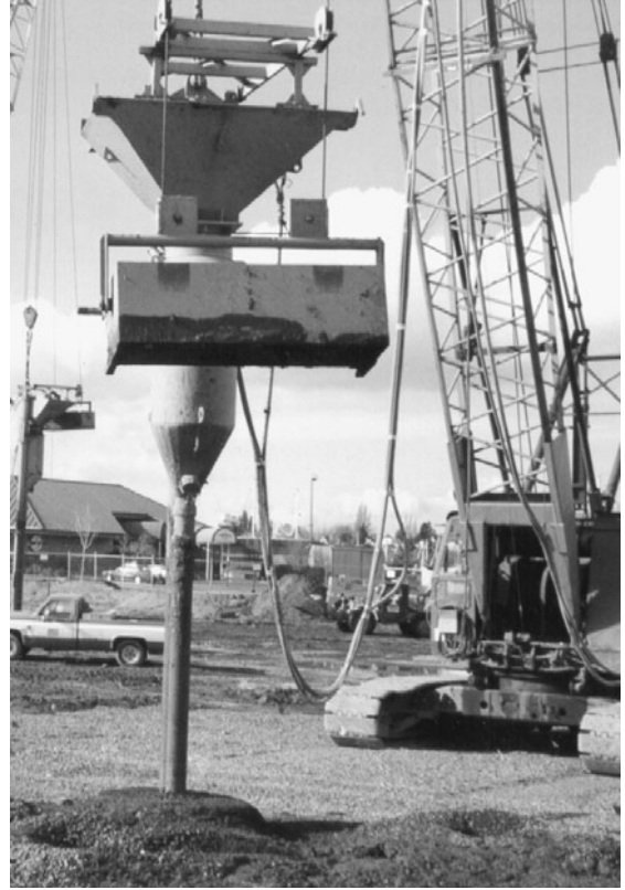
Figure 5-39 Fine Material Being Brought to the Surface. (Courtesy Hayward Baker Inc.)
