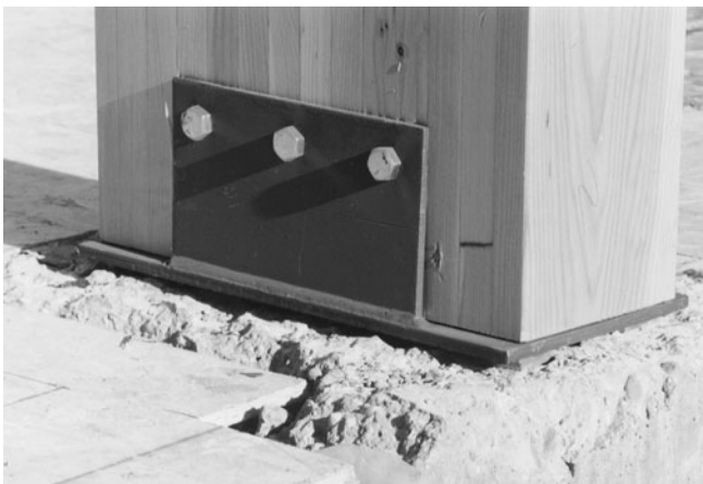
Figure 8-10 Column Base Plate Detail for Glulam Column.
