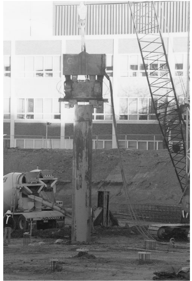
Figure 5-24 Vibro Driver Used in Driving Pile Shell.
