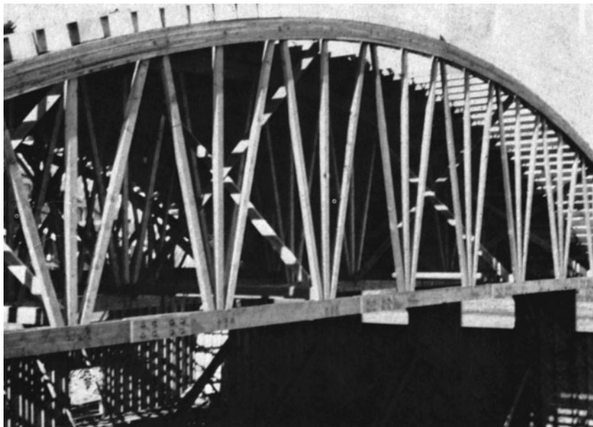
Figure 12-7 Bowstring Trusses with Curved, Glued-Laminated Top Chord.
