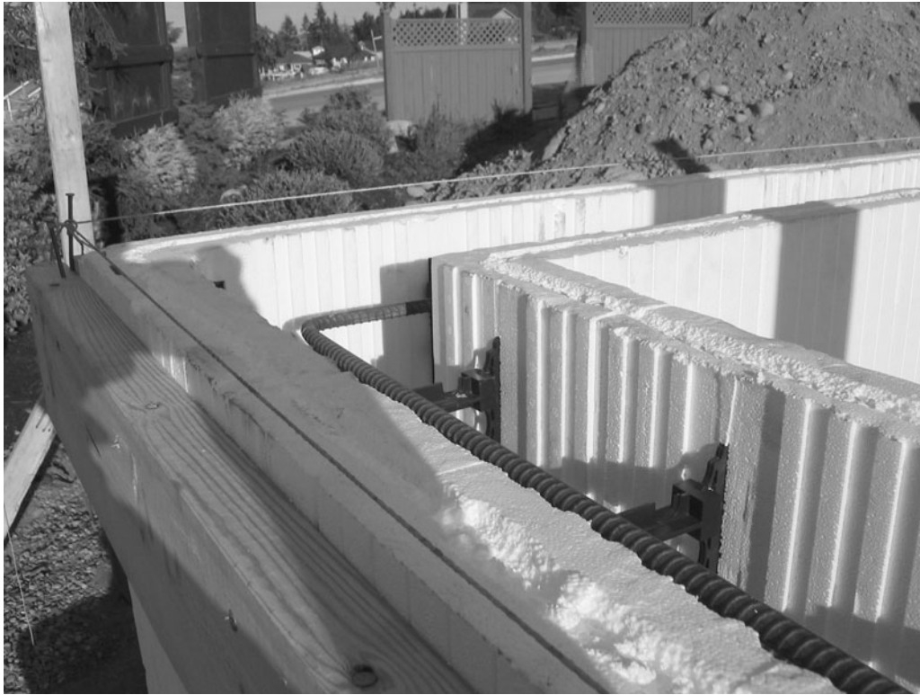
Figure 15-24 Expanded Polystyrene Block Units with Added Reinforcing Bars.
