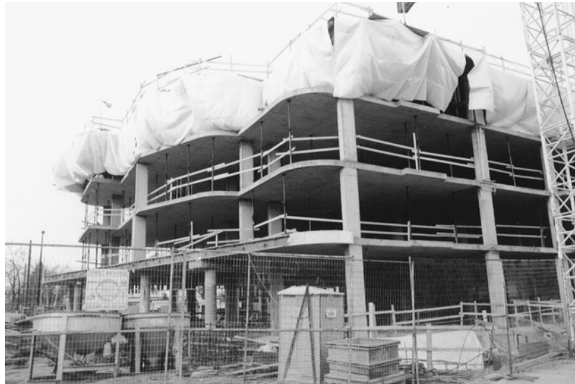
Figure 6-75 Series of Columns and Flat Plate Floors.
