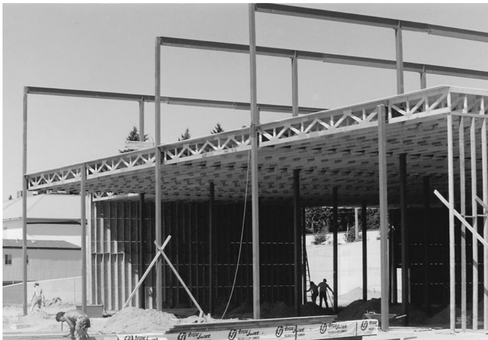
Figure 8-12 Stud Framing between Load-Bearing Columns.
