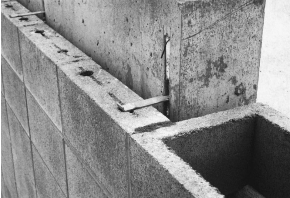
Figure 13-21 Dovetail Masonry Anchor.
