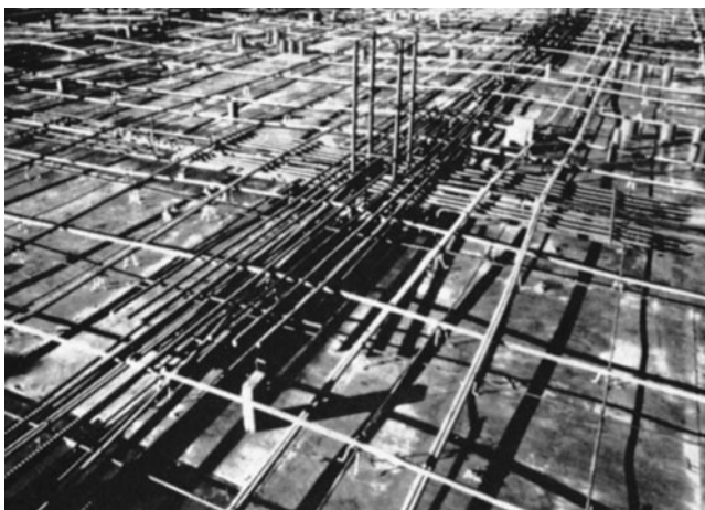
Figure 11-23 Two-Way Slab Ready for Concrete.
