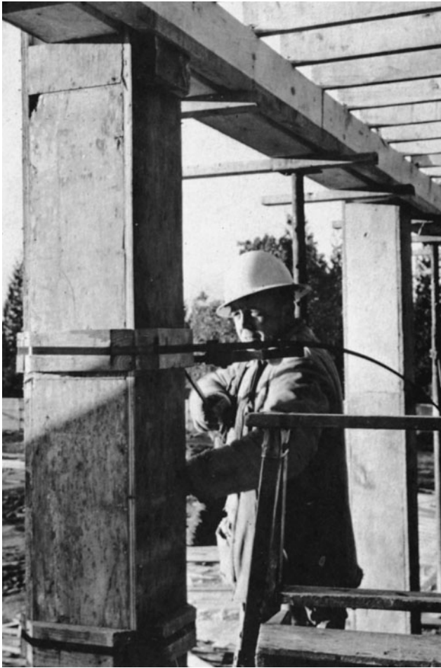
Figure 9-11 Banding a Plywood Column Form. (Reprinted with permission of Council of Forest Industries of British Columbia.)
