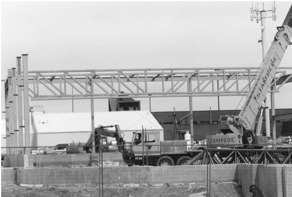
Figure 12-11 Trusses Supported on Columns and Roof-Framing Girders.
