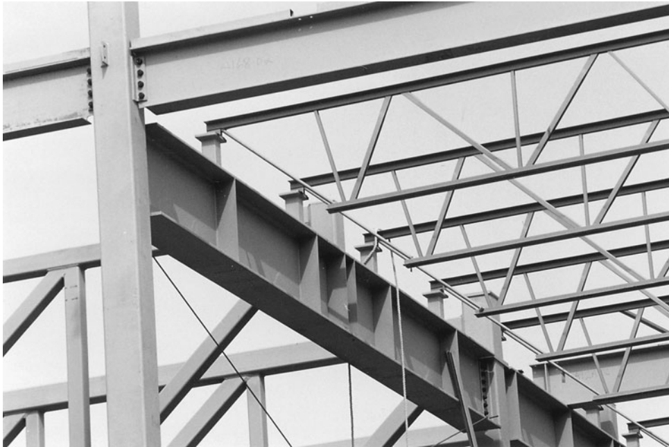
Figure 10-34 Open-Web Steel Joists with Double-Angle Chords.
