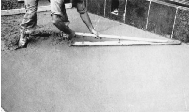
Figure 11-8 Darbying a Concrete Slab. (Reprinted with permission of Portland Cement Association.)
