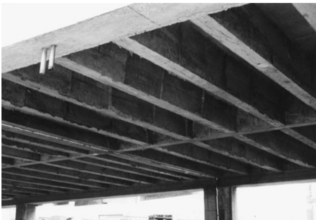
Figure 11-18 One-Way Joist Floor.
