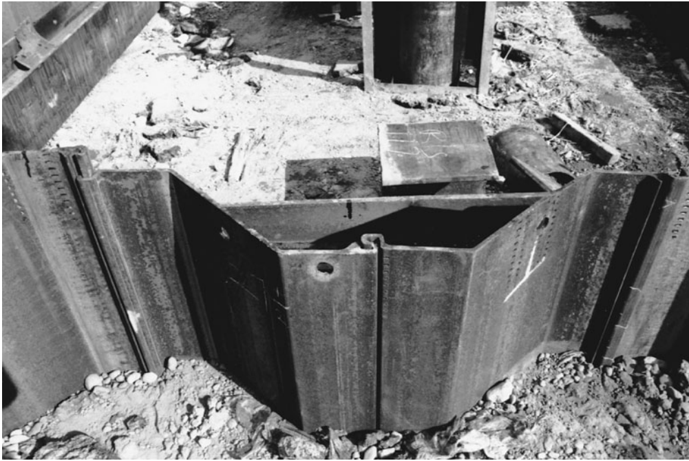
Figure 3-50 Interlocking Steel Sheet Piling.
