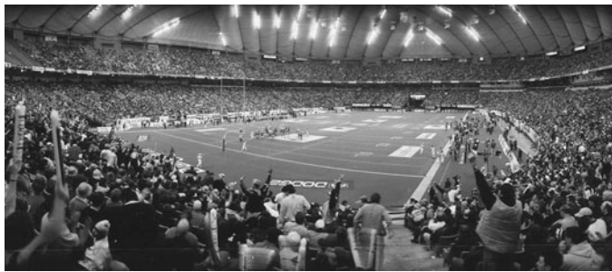
Figure 12-75 Inside One of the World's Largest Air-Supported Fabric Roof Stadiums. (Reprinted by permission of B.C. Place Stadium.)
