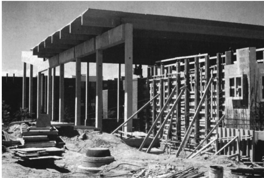
Figure 12-32 Single-Tee Roof Slab System.
