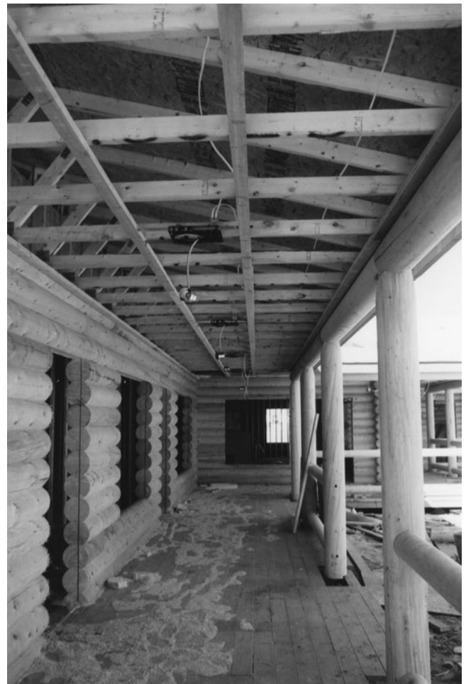
Figure 12-18 Light Frame Trusses Covered with Roof Sheeting.
