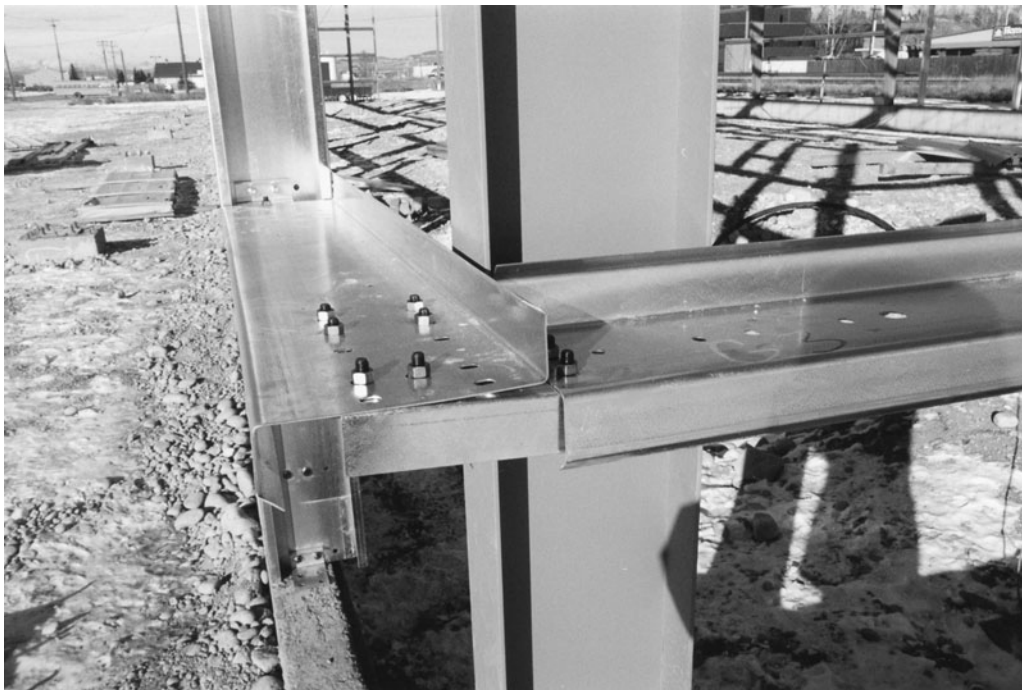
Figure 10-12 Cold-Formed Z Sections Used as Girts.
