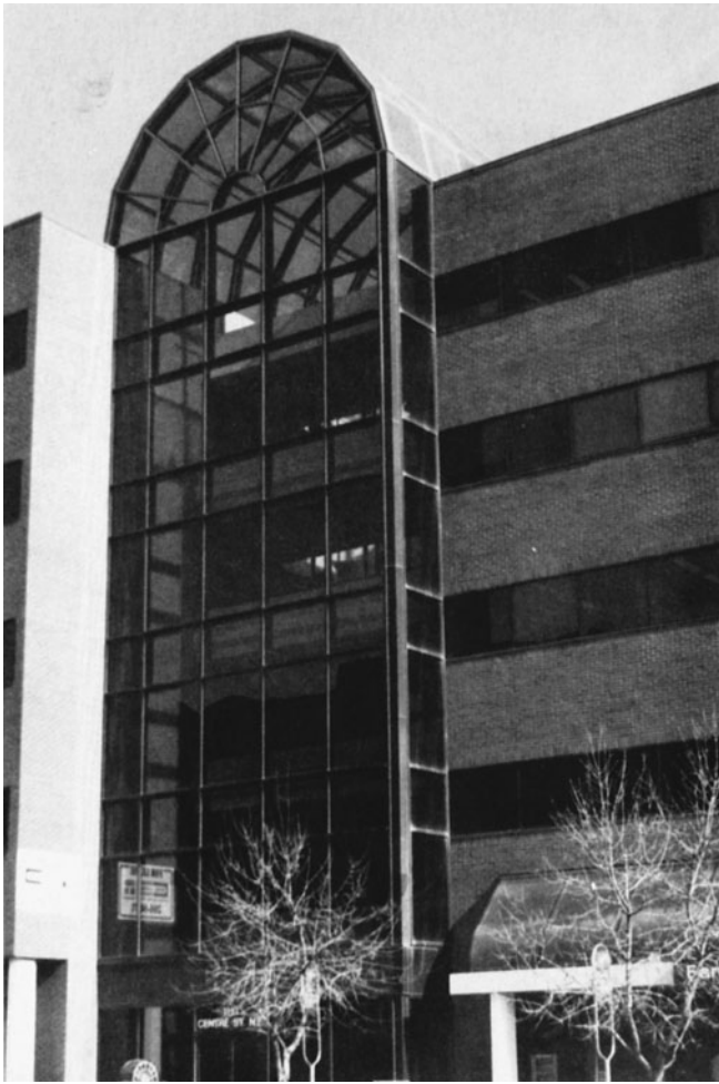
Figure 16-25 Atrium in Building Provides Excellent Light for the Entire Height of a Building.
