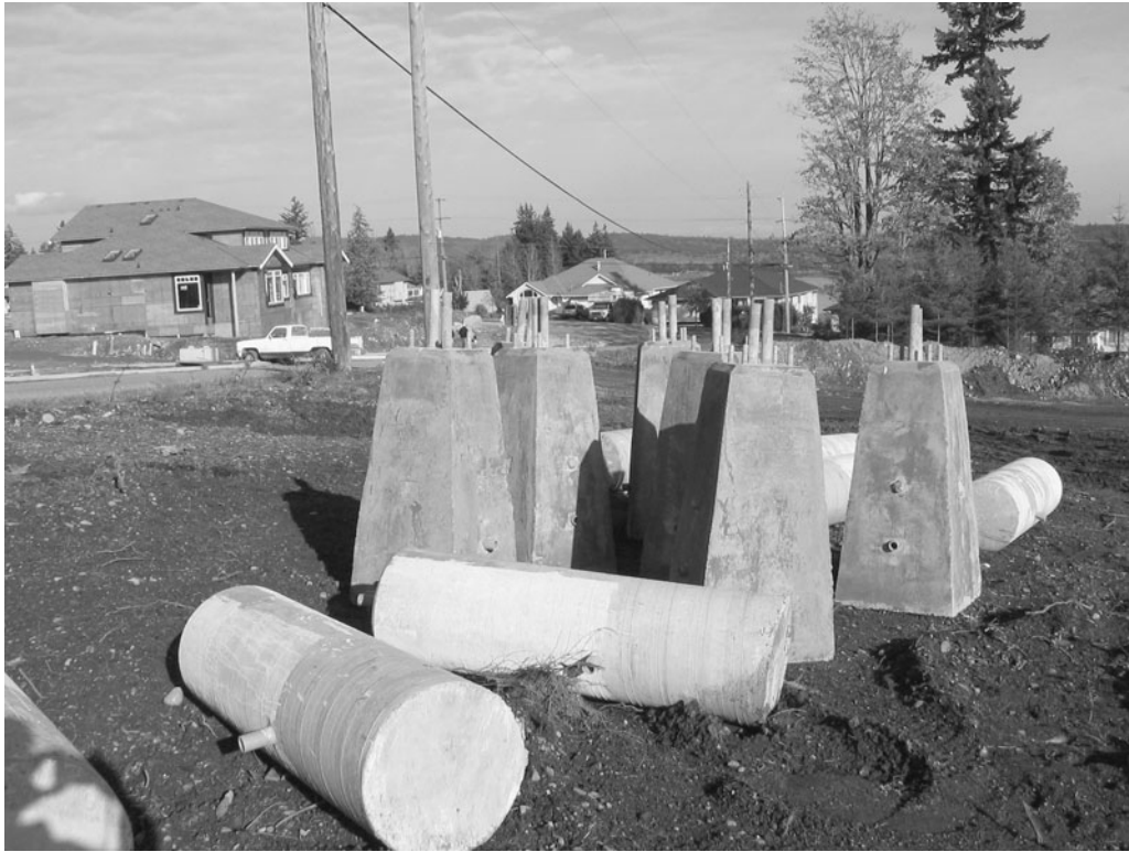
Figure 4-20 Precast Concrete Bases for Street Lighting Standards.
