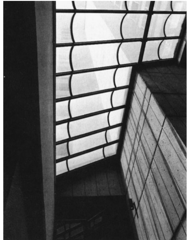
Figure 16-24 Skylights Consisting of Glass or Acrylic Panels Are an Excellent Source of Natural Light.
