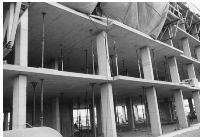
Figure 11-16 Flat-Plate Floors.
