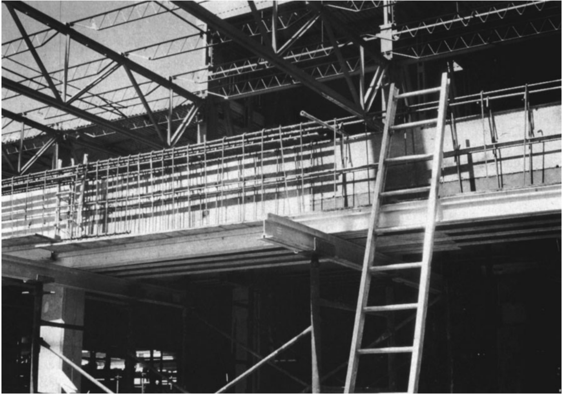
Figure 9-30 Beam Reinforcement for Continuous Beam.
