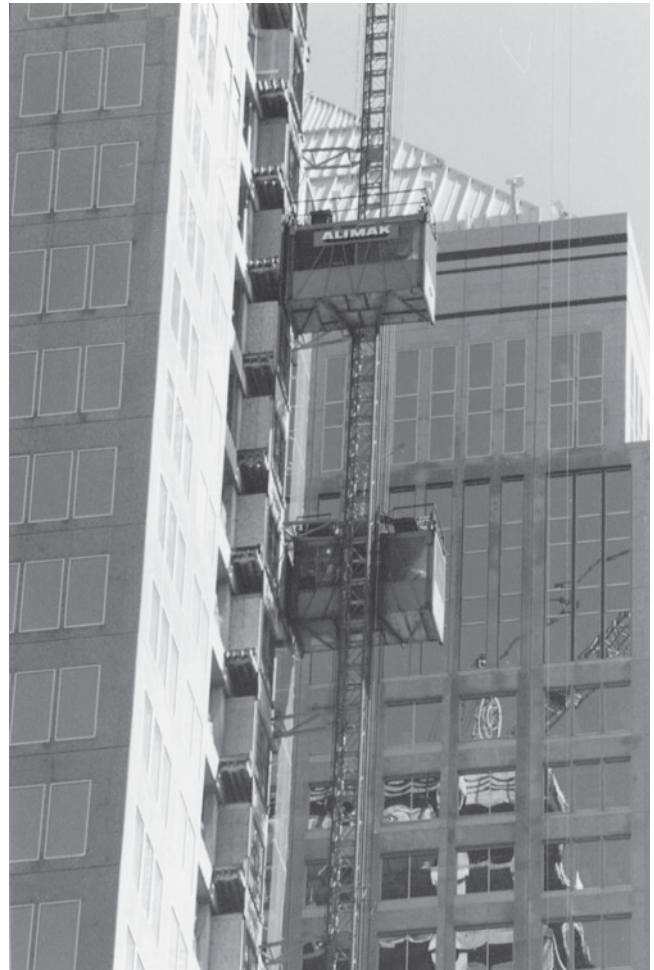
Figure 7-20 Materials Hoist for High-Rise Building.
