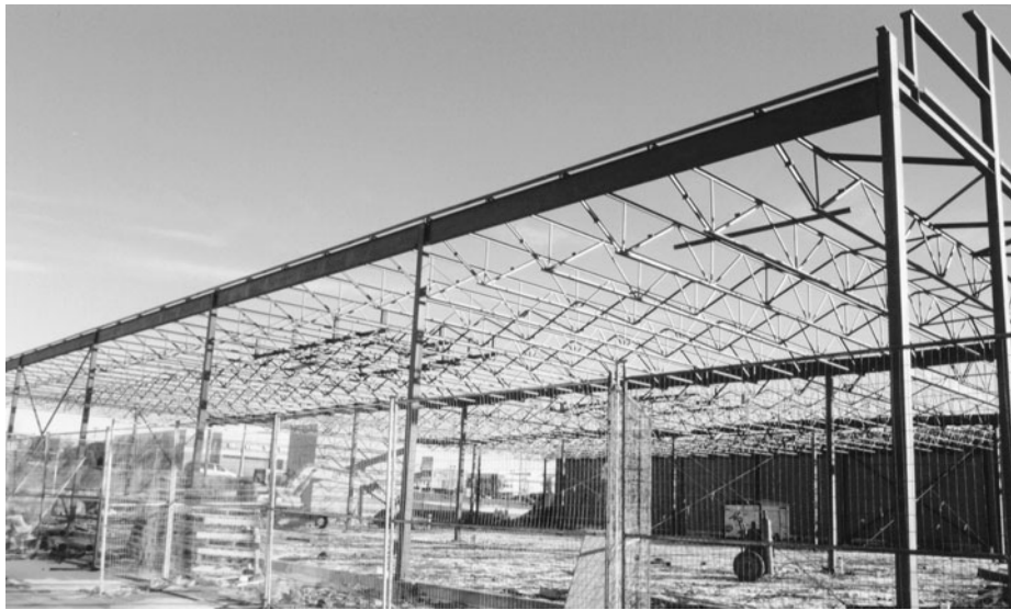
Figure 12-20 Open-Web Steel Joists.
