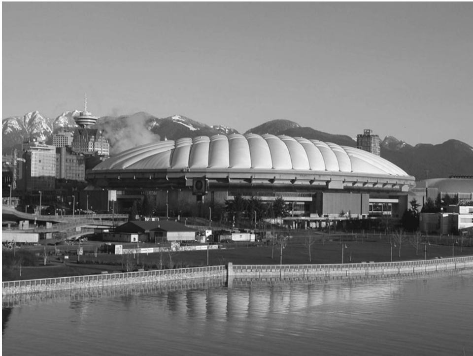
Figure 12-77 Air-Supported Fabric Roof on a Stadium. Note the Stabilizing Cables Anchored to the Compression Ring. (Reprinted by permission of B.C. Place Stadium.)
