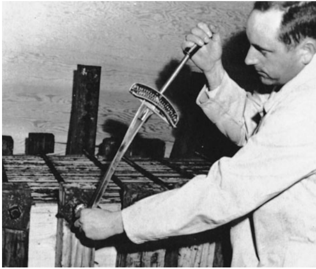
Figure 8-31 Checking Tension on Clamp Bolts with a Calibrated Torque Wrench. (Reprinted by permission of Canadian Wood Council.)
