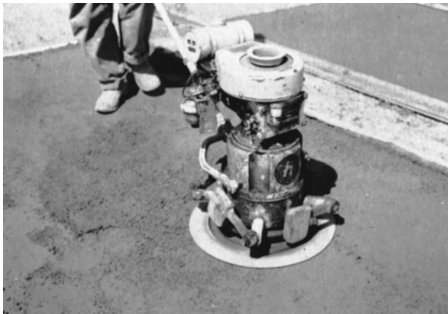
Figure 11-56 Power Tamper and Float. (Reprinted with permission of Portland Cement Association.)
