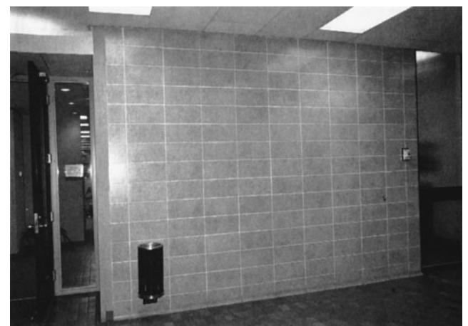
Figure 16-44 Wall of Block Units with Preglazed Finish.
