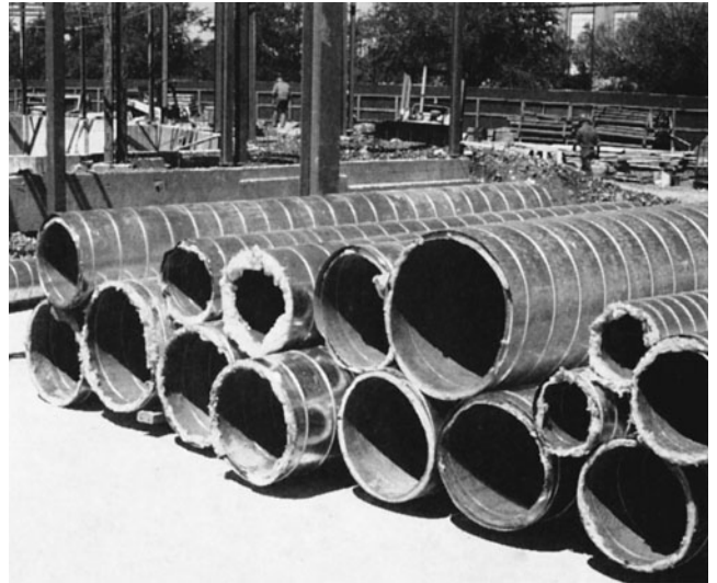
Figure 15-6 Air-Conditioning Ducts Lined with Glass Fiber Insulation.
