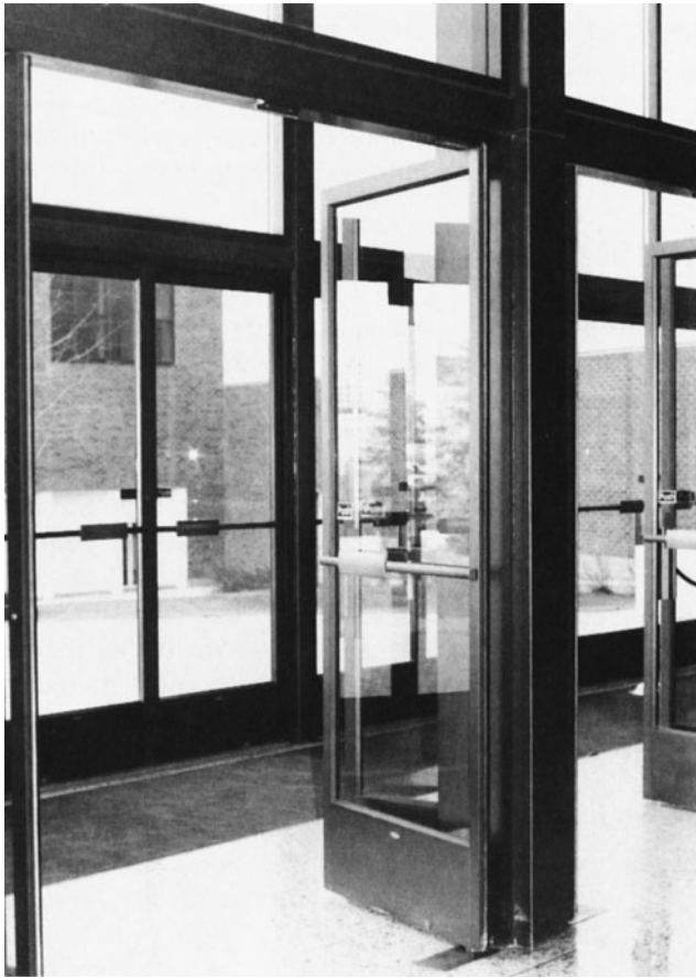
Figure 16-16 Double Sets of Doors Provide Good Access yet Control Air Movement.
