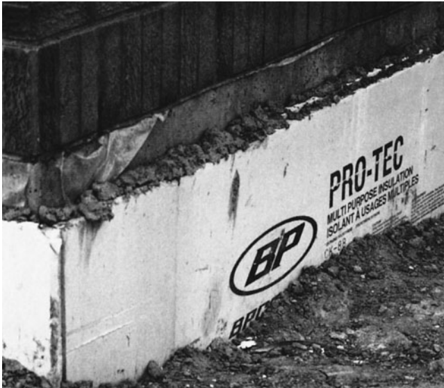
Figure 15-20 Foamed Plastic Rigid Insulation on Foundation Wall.
