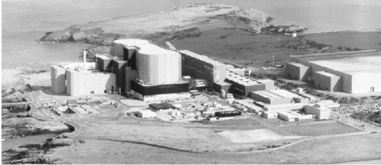
Figure 6.12 Power station project.
