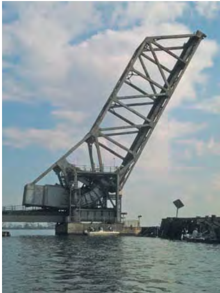
The counterweight on this bascule bridge does positive work as the bridge is lifted and thereby cancels the negative work done by the weight of the bridge. (© R.C. Hibbeler)
