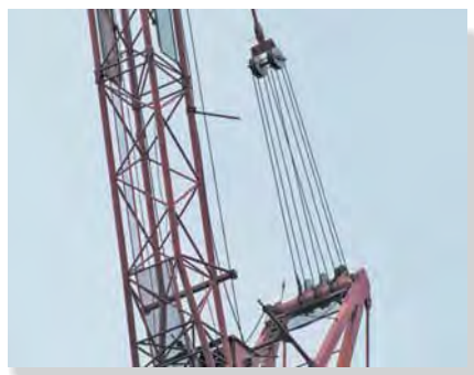
The cable is wrapped around the pulleys on this crane in order to reduce the required force needed to hoist a load. (© R.C. Hibbeler)
