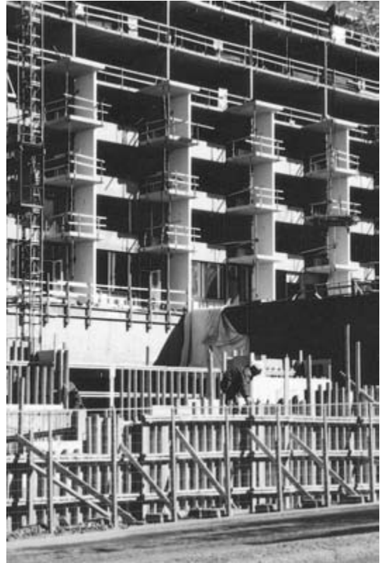
Figure 11.4 Concrete framed building under construction.
