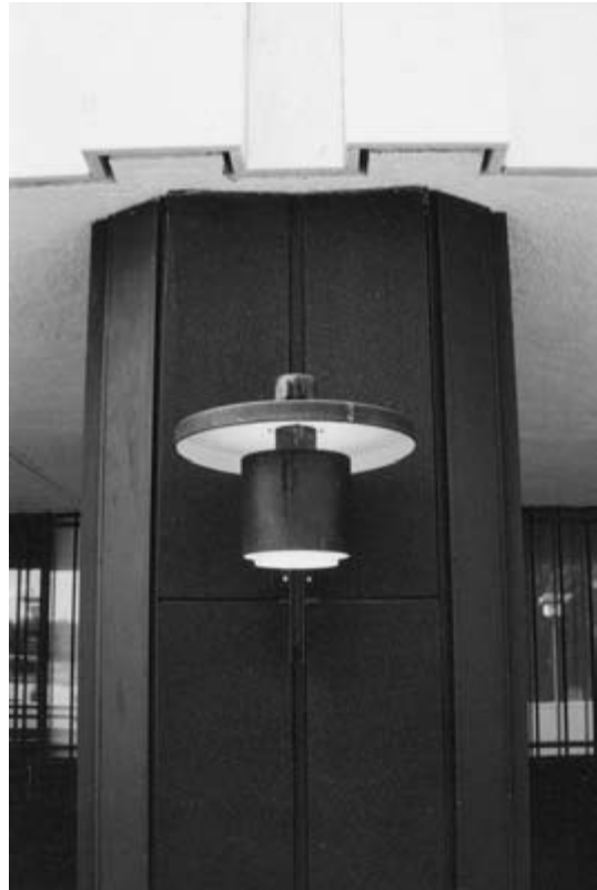
Figure 10.4 Finlandia Hall, Helsinki, column and light detail.
