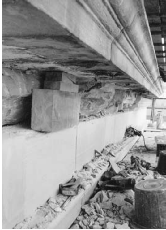
Figure 12.2 Stone replacement and restoration in progress, Harewood House, Yorkshire.
