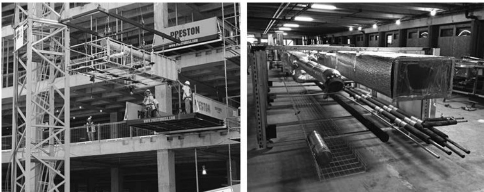
FIGURE 8.8 University Medical Center project, New Orleans, LA ( http://texas.construction.com/texas_construction_projects/2013/0617-prefab-gives-1-billion-hospital-job-a-big-schedule-boost.asp ).
