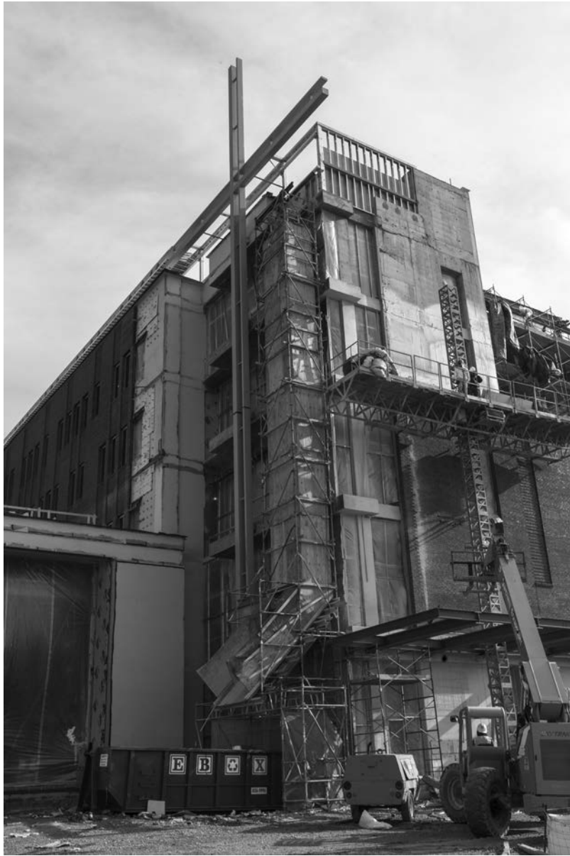
FIGURE 12.4 Trash chute. (Courtesy of aerial innovations of TN, Inc. and Turner Construction Company.)
