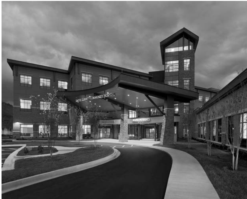
FIGURE 7.20 Smyth County Community Hospital (SCCH), Marion, Virginia. (Courtesy: Hal Jones, VDC Director, Skanska USA Building.)
