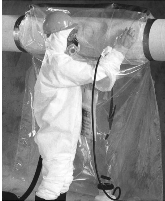
FIGURE 12.6 Glove-bag method. (Courtesy of Gobblell Hays Partners, Inc.)
