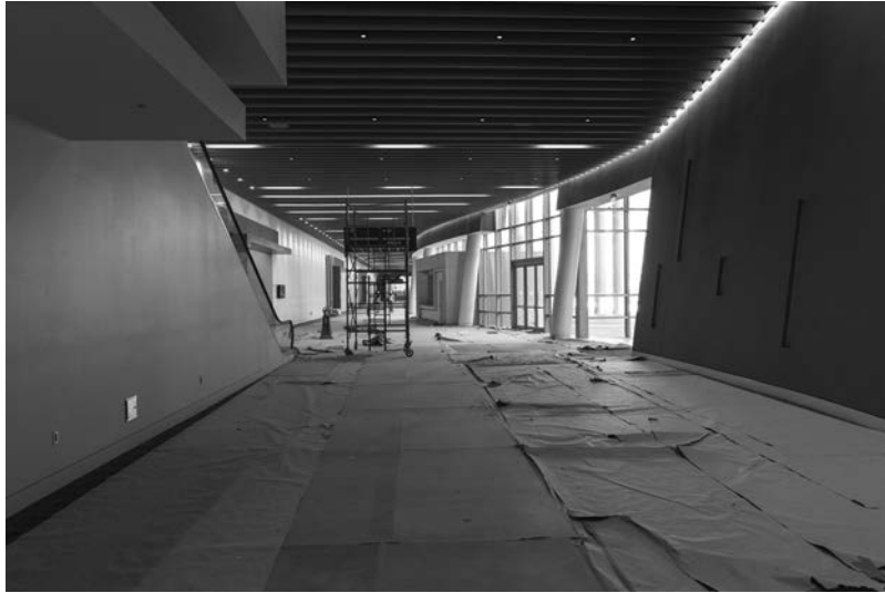
FIGURE 14.3 New flooring protected (FLEXBOARD) ( www.protectiveproducts.com/products/flexboard.html ).
