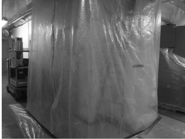
FIGURE 12.2 Temporary dust enclosure. (Courtesy of Gobblell Hays Partners, Inc.)
