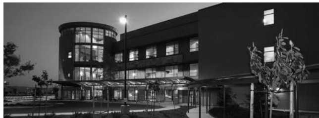
FIGURE 8.6 Sutter Health Fairfield Medical Office Building, Fairfield, California ( Integrated Project Delivery: Case Studies , AIA California Council, 2010).
