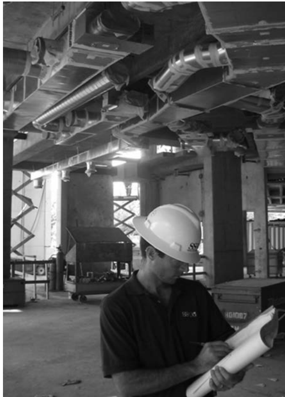
FIGURE 13.3 The HFCxA documents system installation, as systems are set in place.
