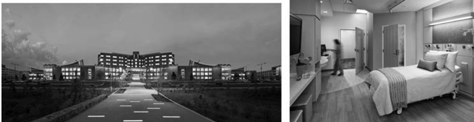
FIGURE 7.9 Fort Belvoir Community Hospital, VA, operated by Department of Defense—new hospital facade ( left ) and patient room ( right ).
