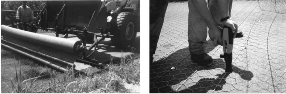
Figure 3. Details of the application of the geotextile and steel mesh.
