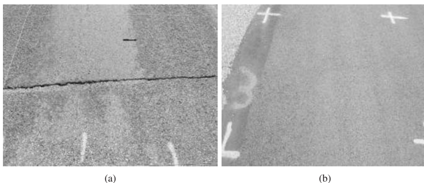
Figure 3. Sample of 1.8 by 1.8 meter parcel on SAMI section a) parcel 3A before treatment b) parcel 3A after treatment.
