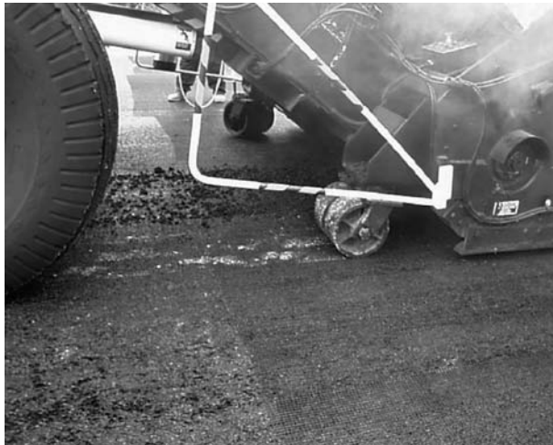
Figure 3. Material transfer device traveling on geogrid surface.
