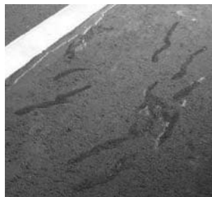
Figure 2. Parallel cracks and alligators.
