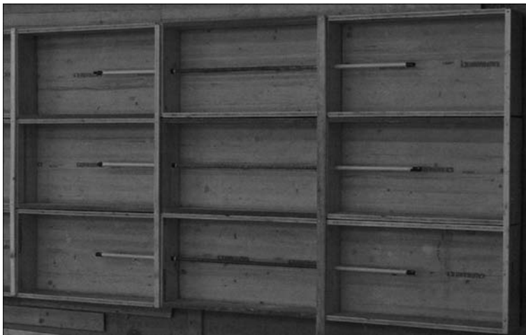
Figure 3. Wooden moulds with the reinforcing bars.
