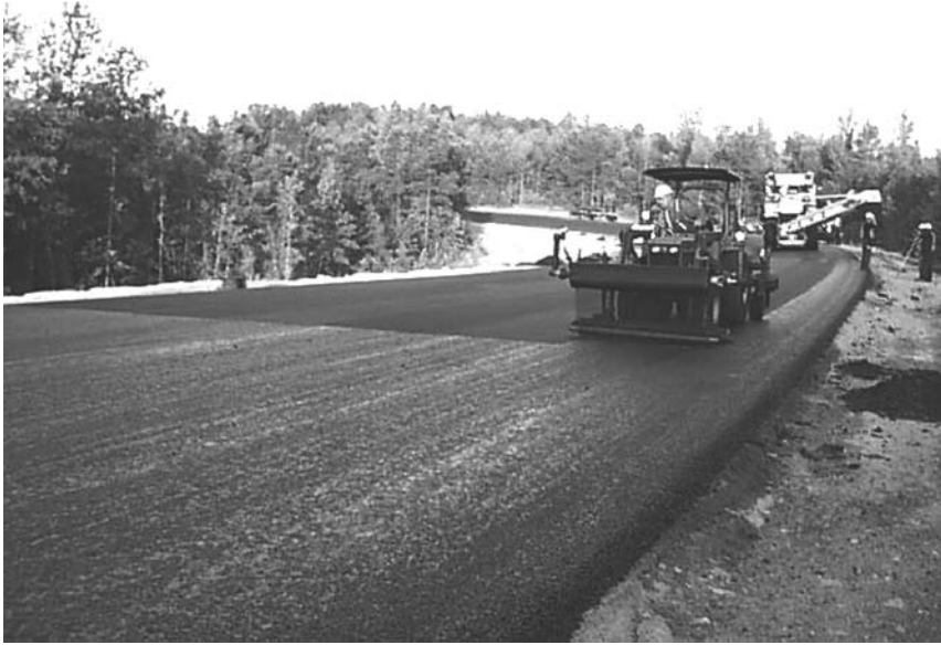
Figure 1. Application of fiberglass geogrid interlayer.
