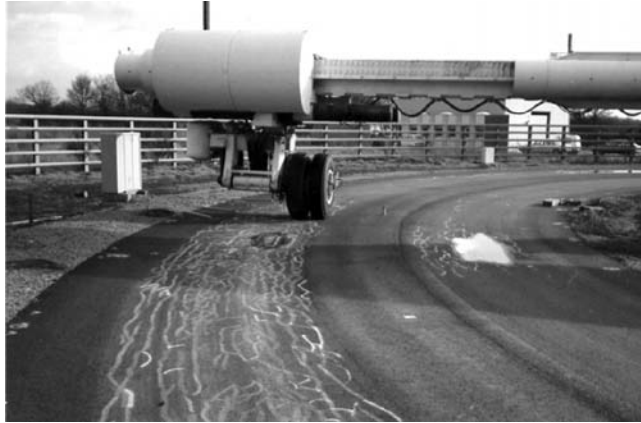
Figure 4. Illustration of cracks observed on structure S1 at the end of the experiment.
