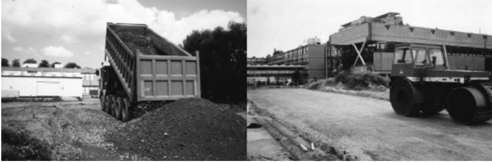
Figure 5. Construction of the base course.
