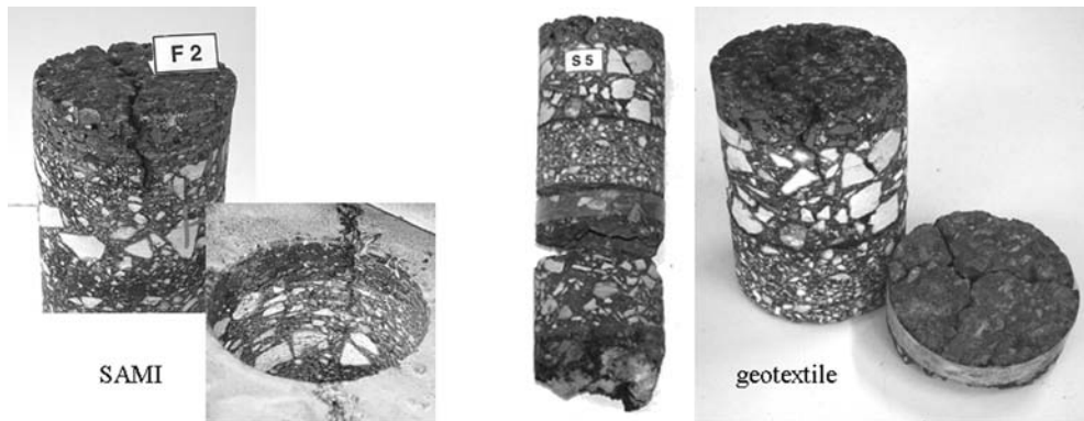
Figure 6. Cores showing crack initiation at the surface and above an existing crack.
