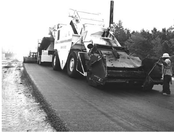
Figure 4. Paving train on geogrid surface.
