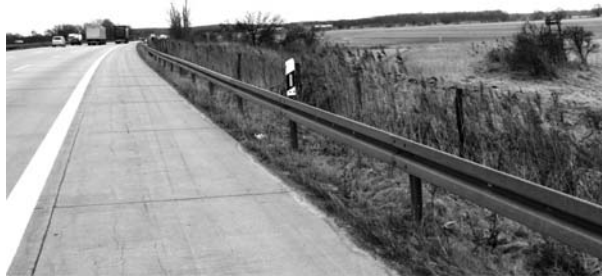
Figure 8. Reed beside the concrete pavement as consequence of ground-water-raising.
