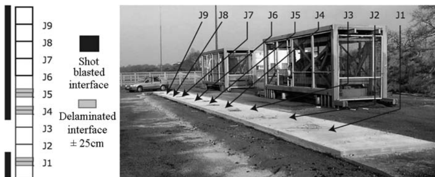
Figure 3. The composite pavement test section and the two FABAC machines (Pouteau, 2004a).
