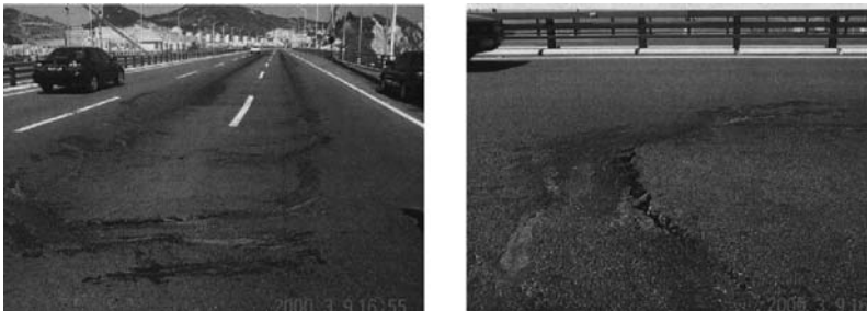
Figure 7. Slippage cracks.
