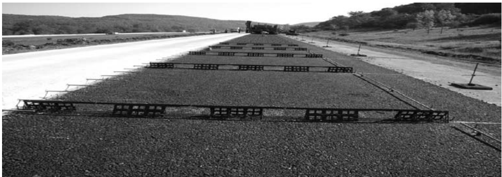
Figure 4. Setting devices prior to pouring concrete in Olean (NY).
