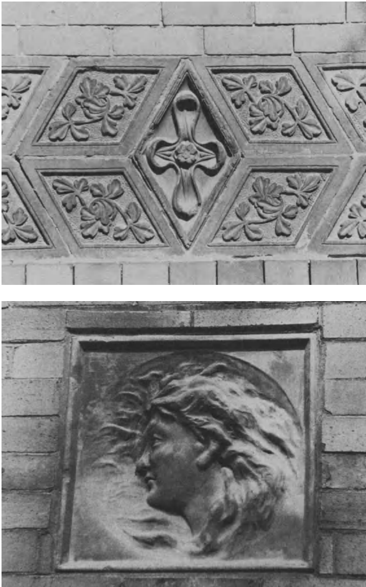
Fig. 6. Unglazed, red terra cotta manufactured at Alfred Center, N.Y., in the late 1890's. Courtesy of D. E. Rase
