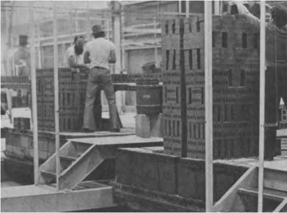
Fig. 52. Manual hacking of face bricks with kiln cars on elevators
