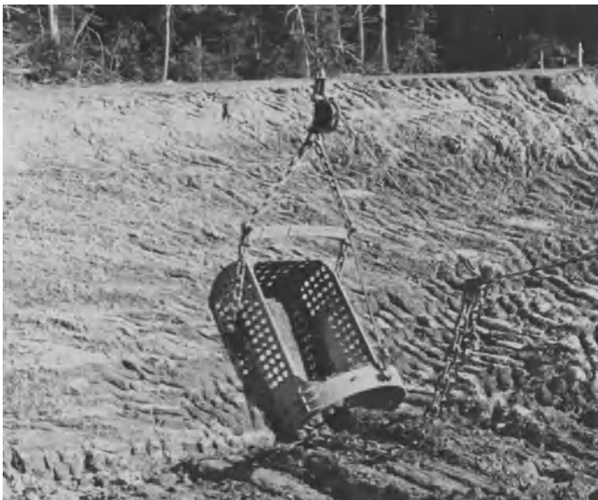
Fig. 18. Mining wet clay with a dragline
