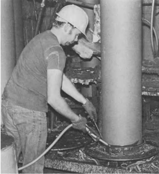
Fig. 110. Casting a polyester jointing unit on the spigot end of a sewer pipe
