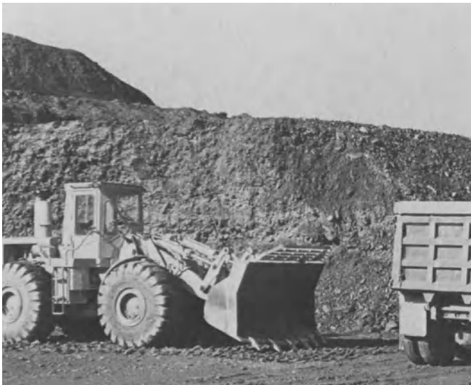
Fig. 21. Remining a stockpile with a front-end loader
