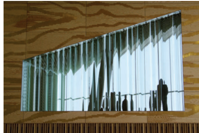
21.29. (upper right) An enlarged gold-leaf pattern of the plywood was applied on top of the plywood cladding in the main auditorium.
