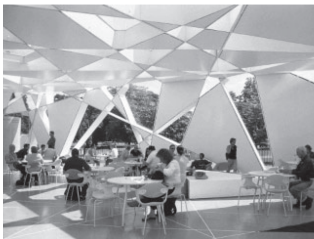
1.26. (far right) Serpentine Pavilion : the irregular-looking pattern is based on incremental scaling and rotation of a series of inscribed squares.
