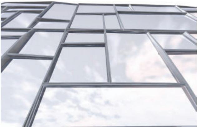
22.52a–b. 100 11th Avenue : the faceted façade is composed of tilted glass panes of varying shapes and materials.
