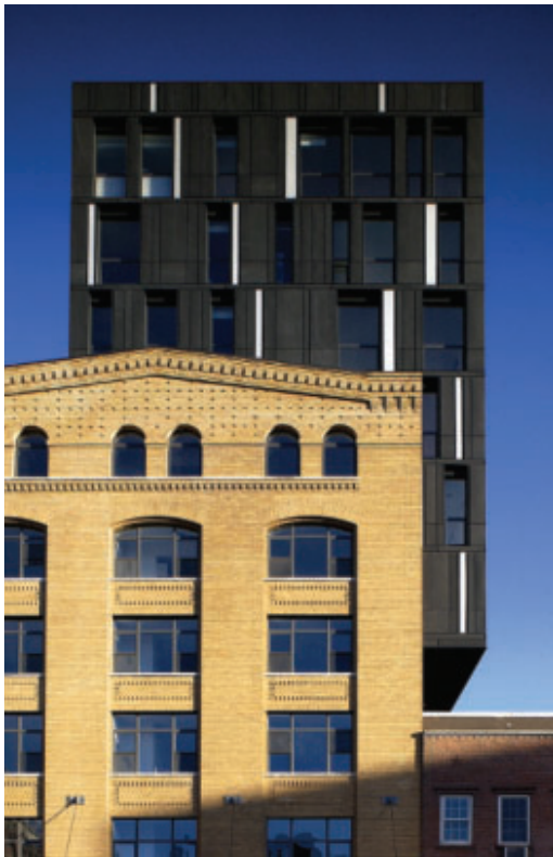
3.14. The Porter House : new zinc façade against existing brick façade.
