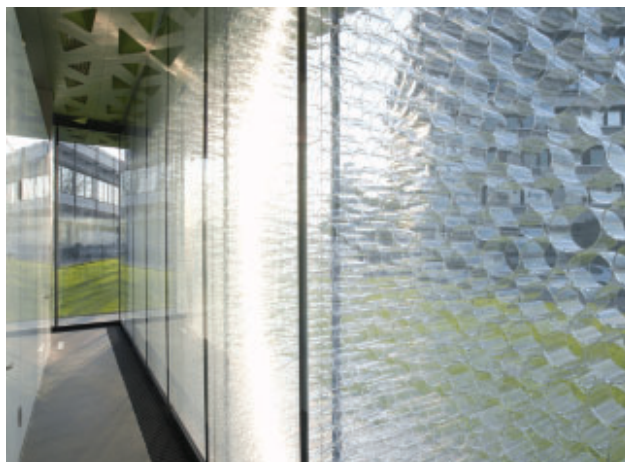
8.19. Trumpf Gatehouse : plexi-glass tube infill sunscreen material effect.
