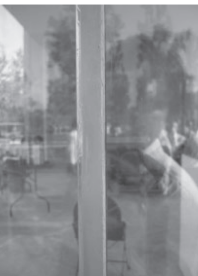
22.13. (left) Toledo Glass Pavilion: the translucent silicone joint between the panels.
