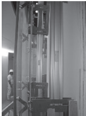
4.18a-d. Fidelity Center for Applied Technology: installation process, showing connection of the panels to the support structure.
