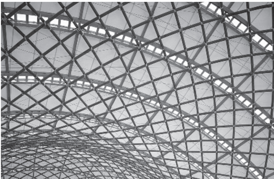
1.1. The structural enclosure of the Japan Pavilion at Expo 2000 , Hannover, Germany, designed by Shigeru Ban, is made from paper tubes.
