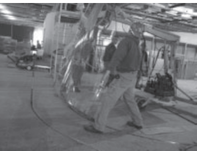
22.12a–c. Toledo Glass Pavilion: installing the glass panels into the recessed channels.
