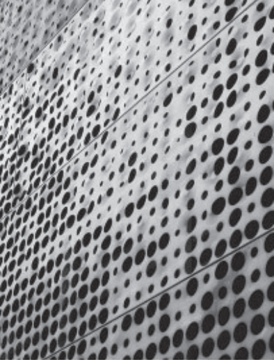
1.19. (above) The embossed and perforated rain screen panels in de Young Museum in San Francisco (2005), designed by Herzog & de Meuron .
