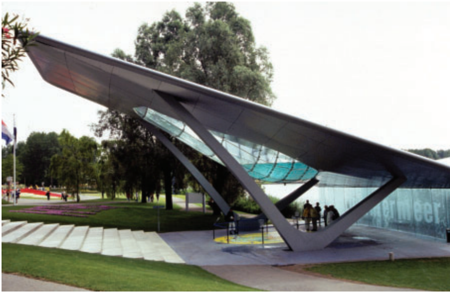
20.8a–b. (right) Hydra Pier: some of the aluminum roof panels have complex, double curved forms.
