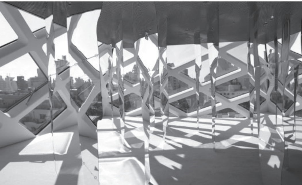
21.40. Waist Down : mirrors were applied to the backside of the two- dimensional cutouts.
