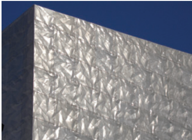
22.82a–b. Walker Art Center: the façade panels were made from stamped, expanded aluminum mesh.
