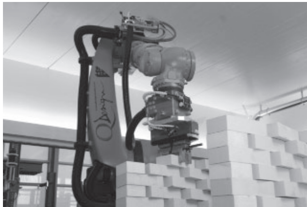
9.20a–b. Gantenbein Vinery : the bricks were laid in a layer-by-layer fashion by an industrial robot.
