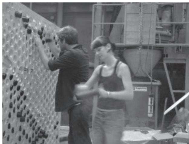
9.27a–b. Completing the formwork by inserting standard pipes into the holes.
