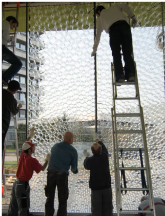
8.20. Trumpf Gatehouse : plexi-glass tube infill sunscreen installation.
