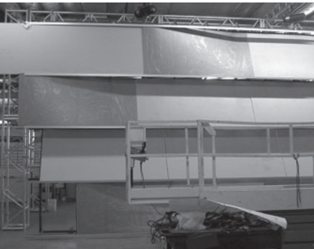
4.10a–c. Sunset Boutique Façade: the dry-fitting on the shop floor (off-site); the panels are shown with a protective cover.
