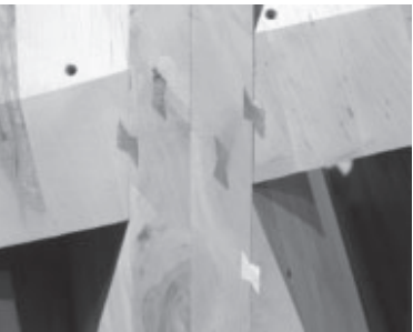
18.6. (below) Futuropolis : CNC-cut boards connected with aluminum dovetails.
