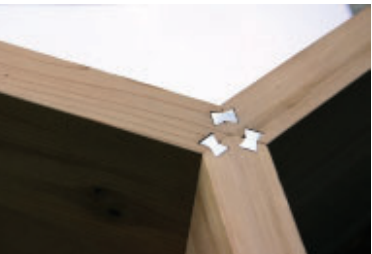
18.22. Futuropolis : aluminum dovetail connectors.
