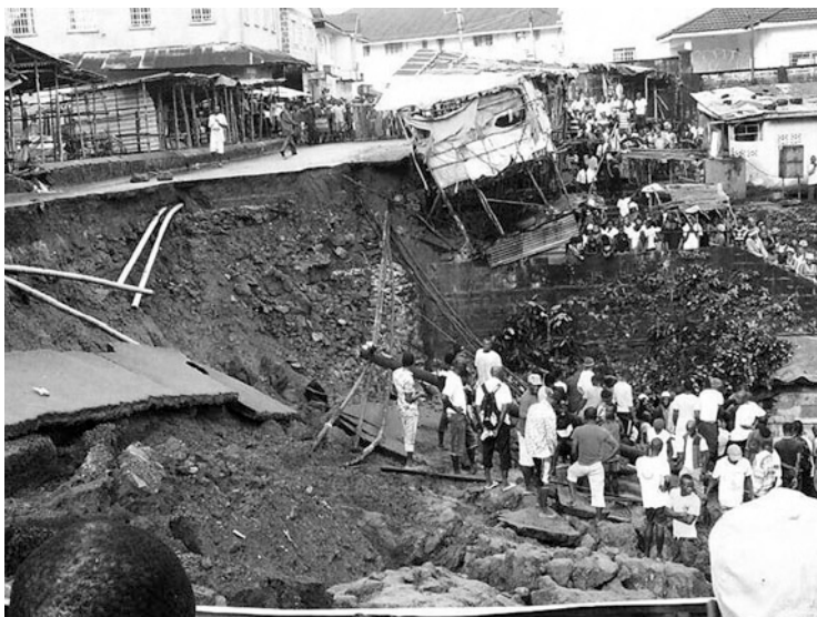
Fig. 10.1 Sierra Leone's King Jimmy bridge collapsed after torrential rains in August, 2013, killing six people
