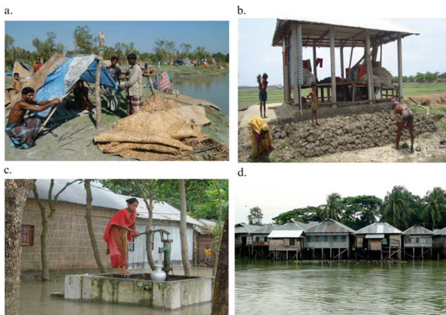
Fig. 21.2 (a) Making temporary shelter after cyclone, (b) raising the homestead land to combat flood, (c) tubewell base is raised high for protection from floodwater, (d) houses erected to make flood proof
