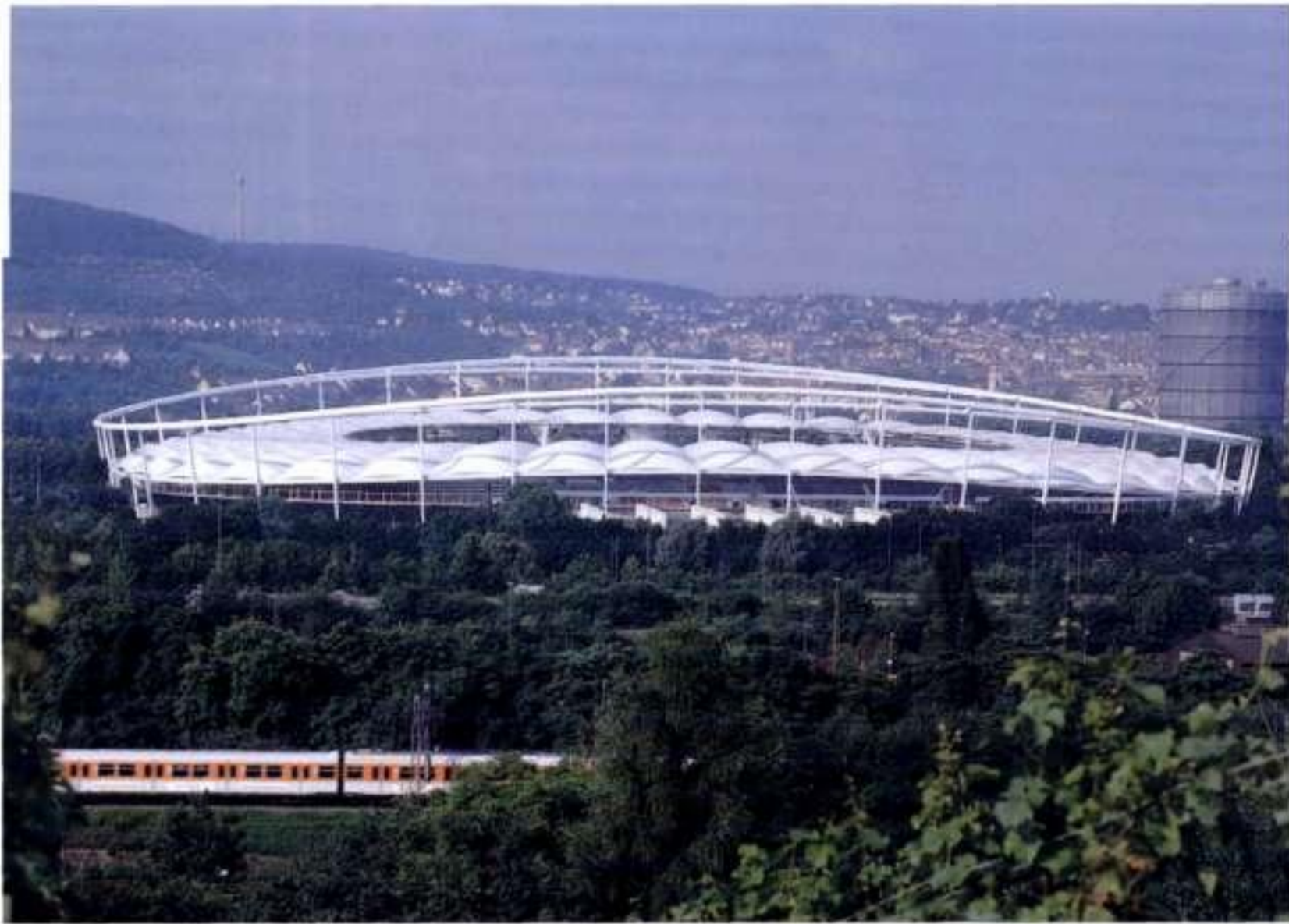
7.55 The Gottlieb-Daimler Stadium roof at Stuttgart
