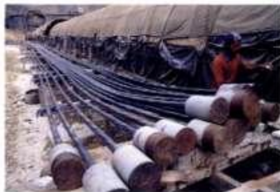
B.44-B.47 Manufacture of the parallel-wire cables on site
