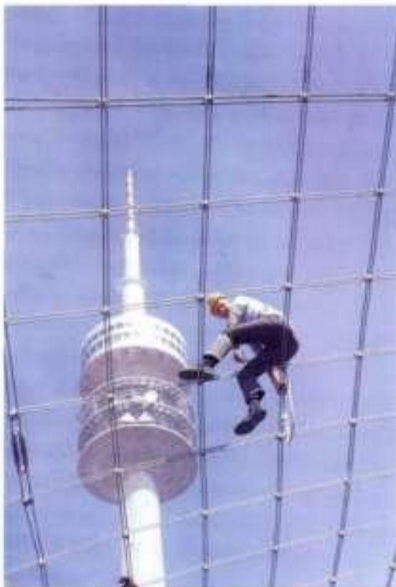
5.13 The Munich cable net with its 75 cm mesh width
