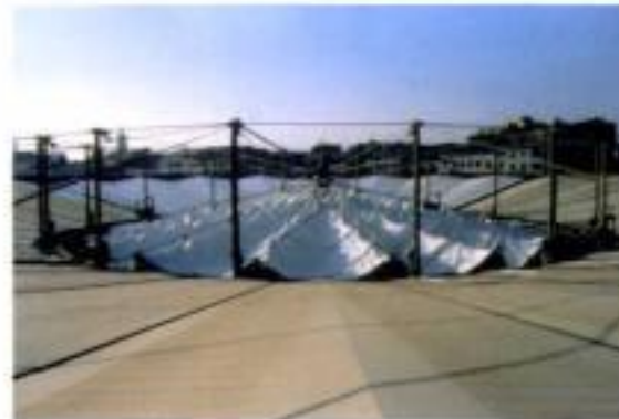
7.46 The retractable roof from above
