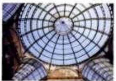
12.10 The glass dome of the Galleria Vittorio Emanuele II in Milan, 1867
