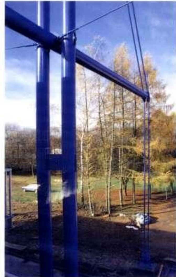
Details of the masts, booms and cables
