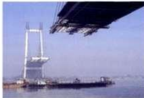
Barges deliver segments of the grid to be lifted into position
