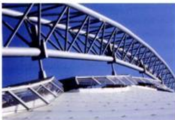
5.74 The skylights in position
