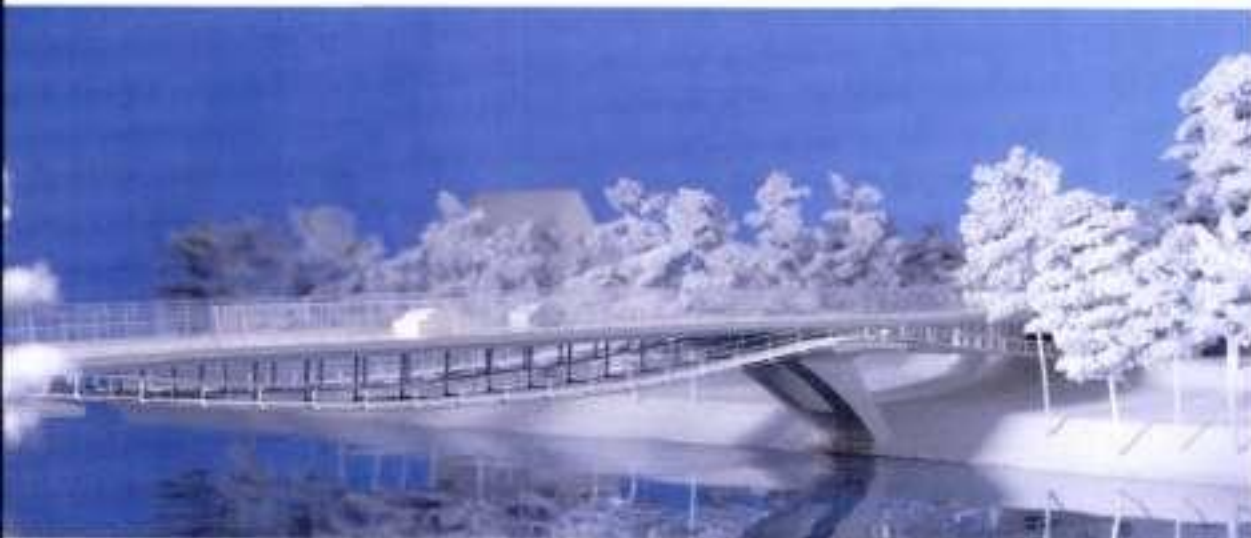
8.103 + 8.104 The road and pedestrian bridge over the Danube at Ingolstadt (under construction). The concrete deck of the roadway is supported by underslung cables and the footpaths follow the vertical curve of the cables.
