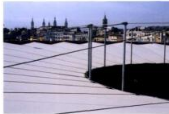
7.45 The outer roof seen from above with its cables and vertical struts
