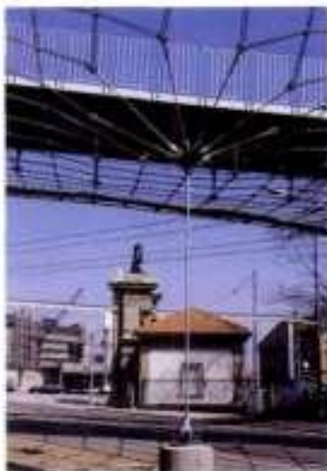
9.91+9.92 A low-point in the net where it is pulled down by a tensioned anchor rod. A row of deck props may be seen
