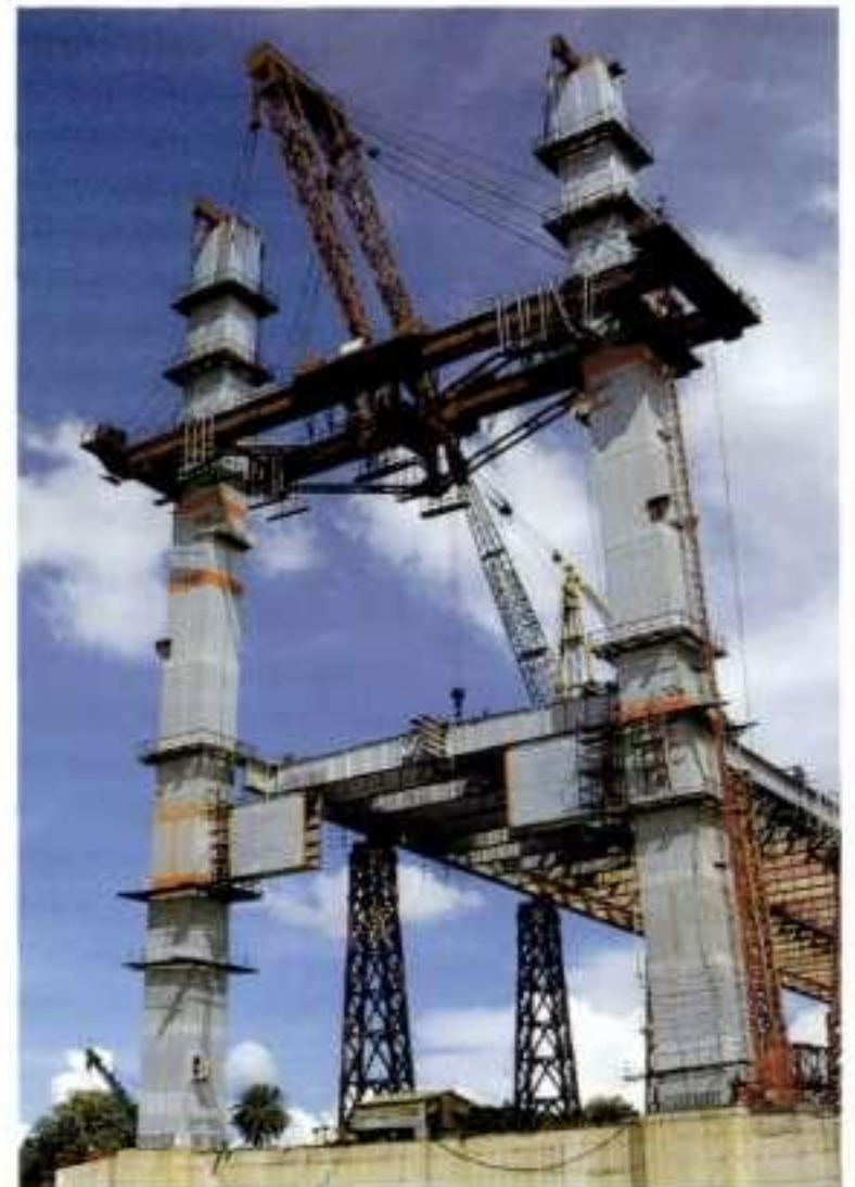
Pylon assembly using a specially built derrick
