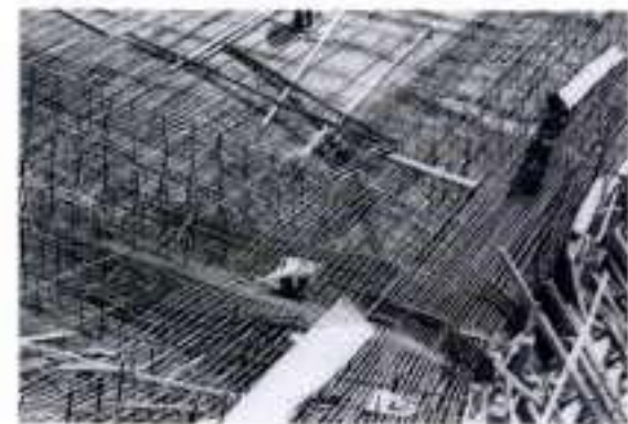
Reinforcement of the valley
