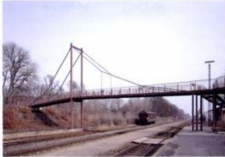
9.128 The Bad Windsheim footbridge
