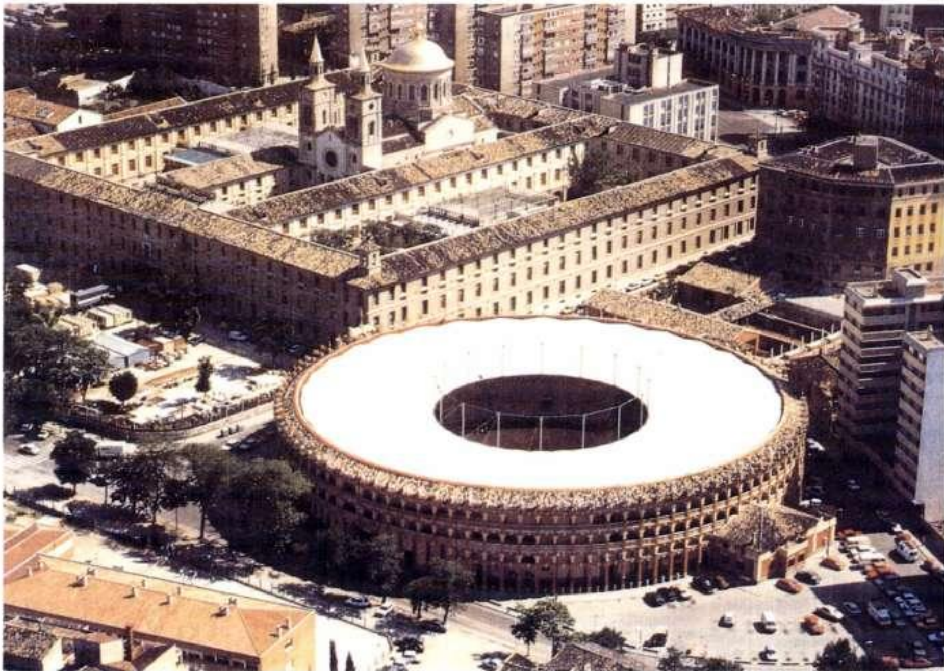
7.42 The roof over the bull-ring at Zaragoza showing only the outer permanent part of the roof
