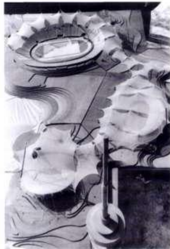
5.9 The final tulle model of the entire roof
