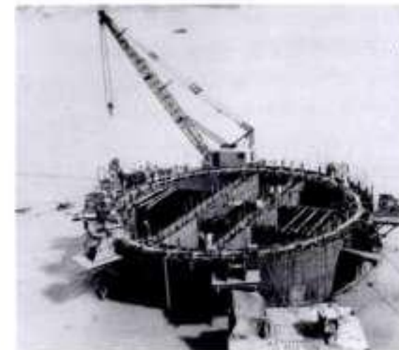
Concreting and sinking a pylon caisson
