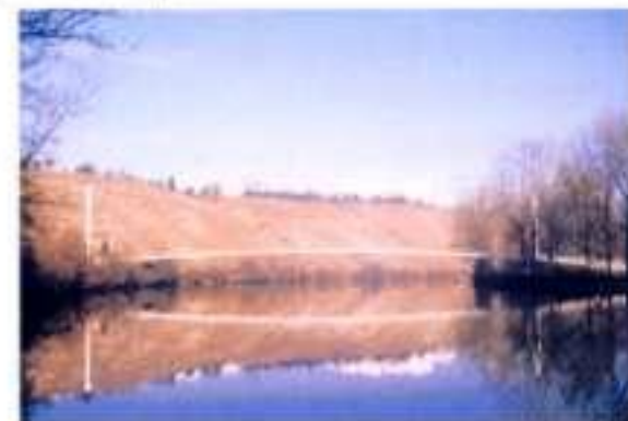
9.33+9.34 Competitive photomontages of: - a box girder bridge of only 75 m span - a suspension bridge of 114 m span
