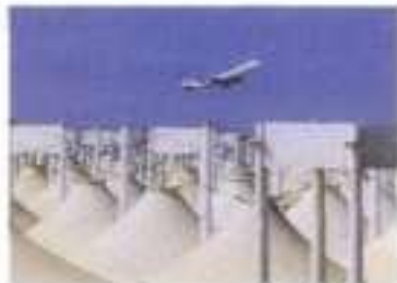
7.2 + 7.3 Jeddah Airport Haj Terminal Building - the tent roofs
