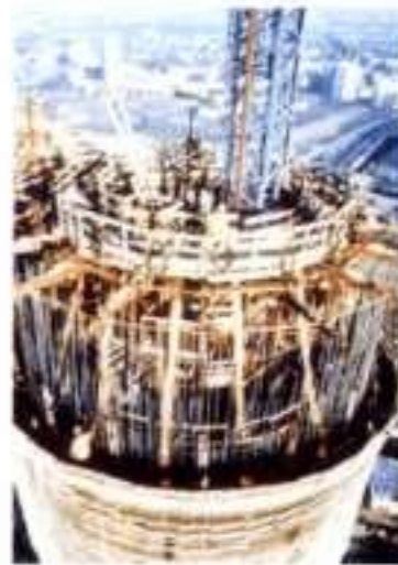
3.6 Climbing formwork for a tower shaft
