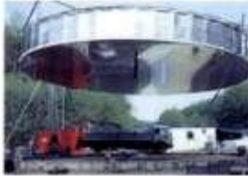
11.19-11.22 Fabrication of 17 m diameter dish concentrators
