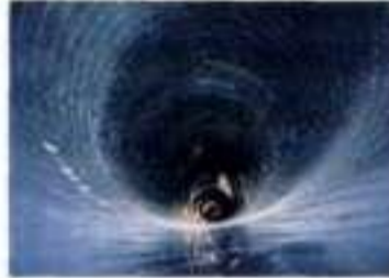
11.52 Looking from the top down into the chimney
