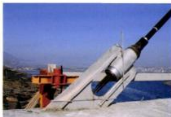
8.52+8.53 The cable anchorage at the deck
