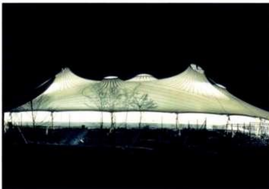
7.68 From outside, at night
