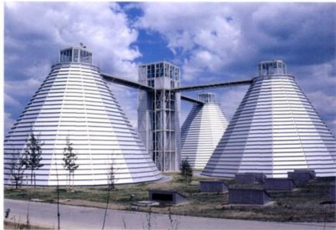
Three of the tanks with central access tower and linking walkways
