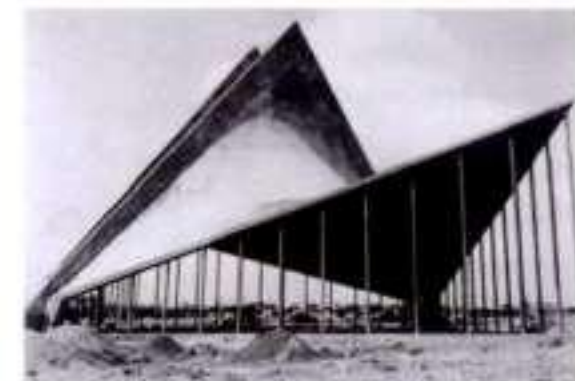
4.7 A beautiful hypar shell designed by Felix Candela with edge beams propped by mullions
