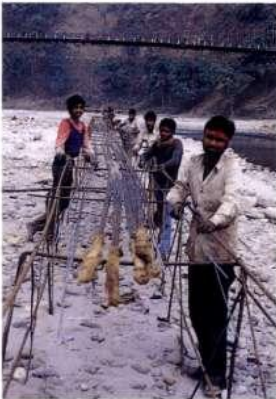
B.44-B.47 Manufacture of the parallel-wire cables on site
