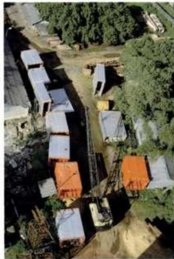
Pylon segments on site as seen from deck level
