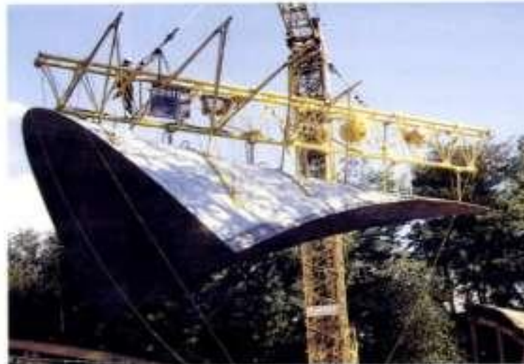
Lifting the hardened segment with the aid of suction strips
