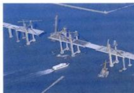
8.108–8.111 The second Macau-Taipa connection (completed in 1994)
