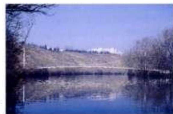
9.35+9.36 The bridge as built with its main cable not yet painted white and after painting it white.
