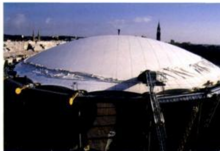
7.37–7.40 Hoisting and inflating the roof
