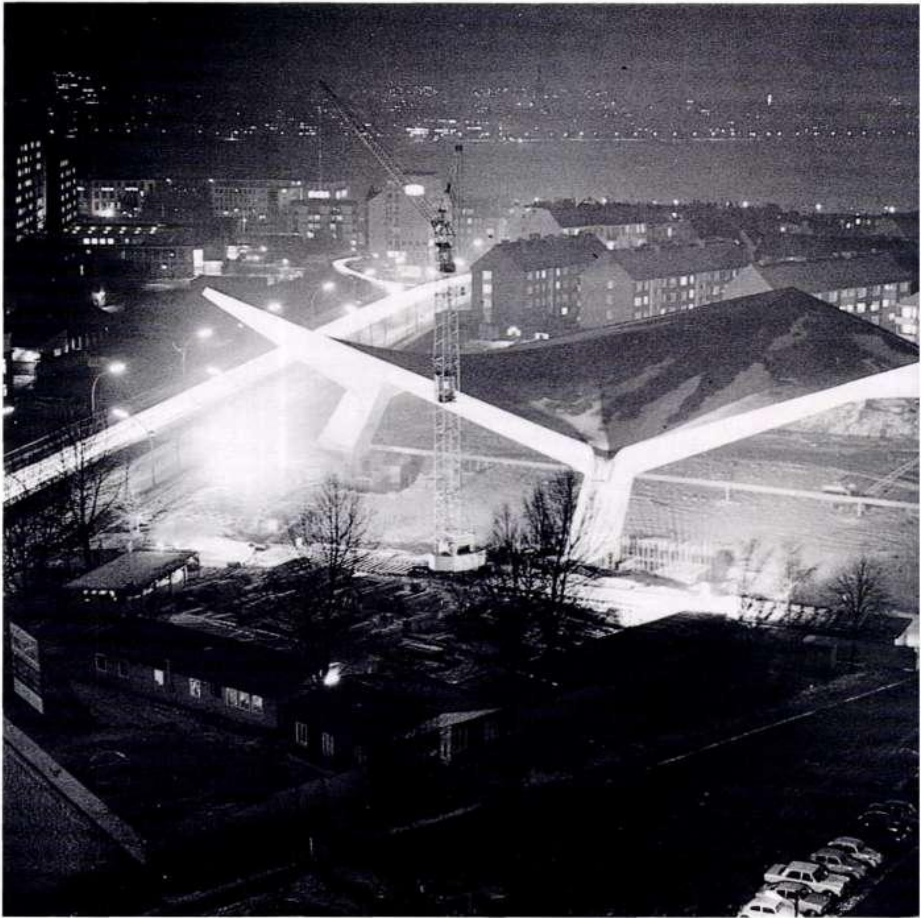
4.16 The completed shell
