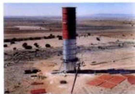
11.48 + 11.49 Erecting the 195 metre high 10 metre diameter guyed tube from corrugated sheet using an incremental lifting method
