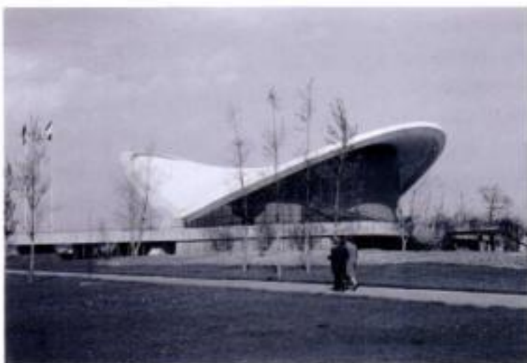
4.41 Berlin Congress Hall: exterior view before collapse
