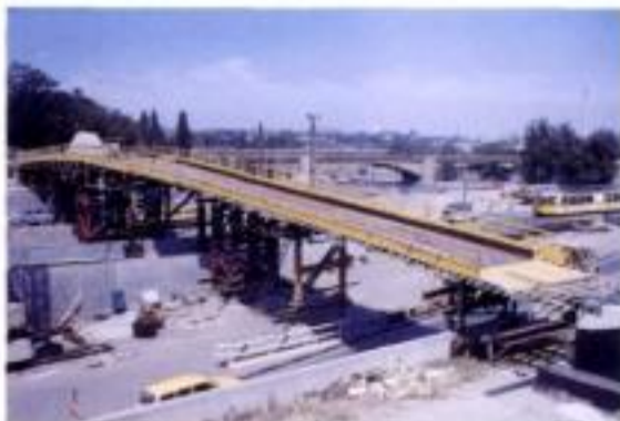
Concreting the deck on formwork
