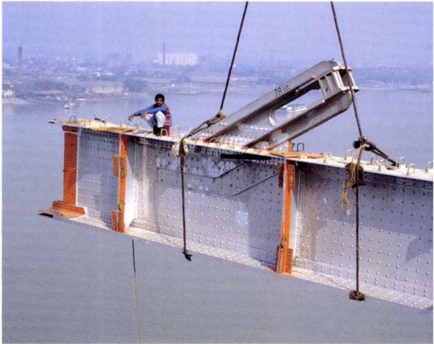
8.22-8.30 Scenes of the construction of the main span composite deck
