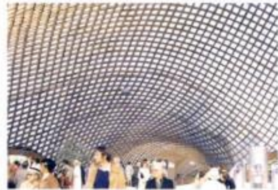
6.5 + 6.6 Frei Otto's timber grid roof at Mannheim (with C. Mutschler and E. Happold), 1974
