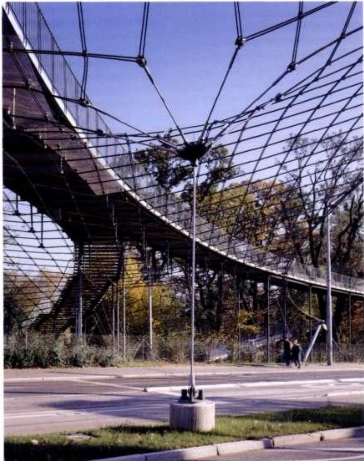
9.91+9.92 A low-point in the net where it is pulled down by a tensioned anchor rod. A row of deck props may be seen
