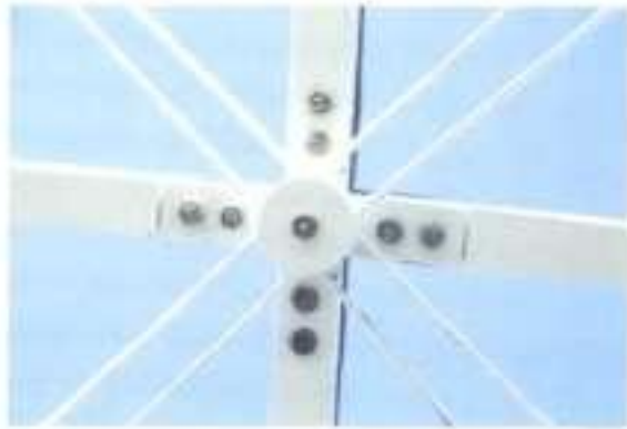
6.17 Close-up of the joint assembly with diagonal cables installed
