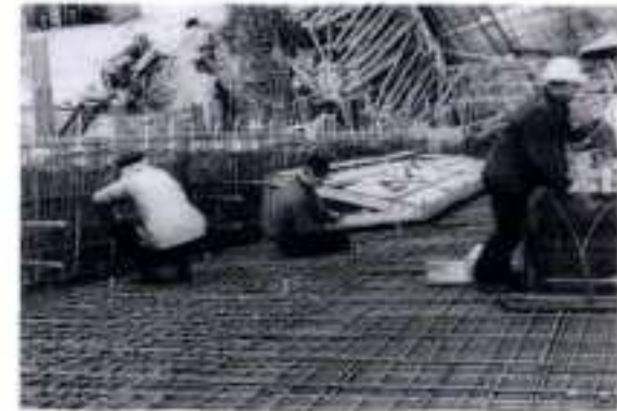
A form for a hollow portion of an edge beam
