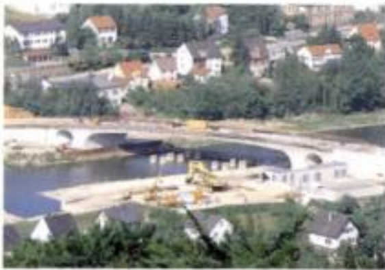
8.70 The Kelheim Westtangente bridge during construction – general view
