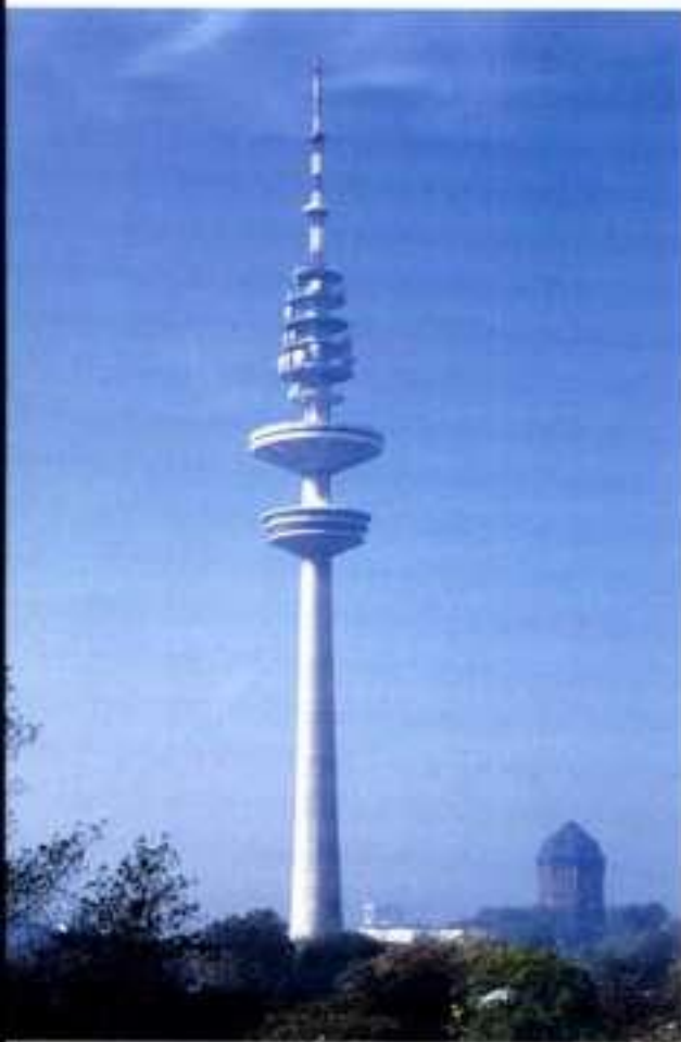
3.5 The Hamburg telecommunications tower, completed 1967
