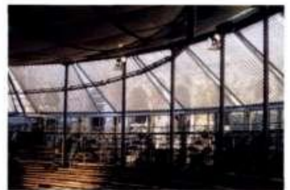
7.35 The inclined translucent facade from inside
