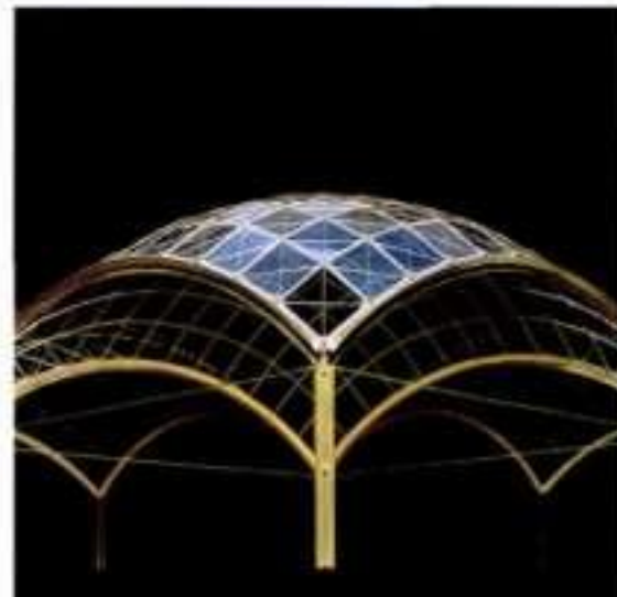
6.46 Two examples of double-curved surfaces of translational origin permitting cladding with plane (glass) panels
