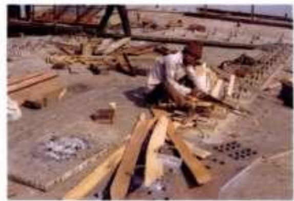
A carpenter preparing the formwork for the concrete slab
