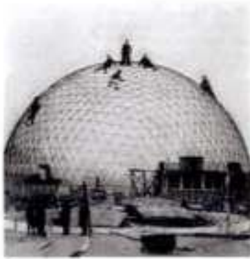
6.1 Framework for the Planetarium on the roof of the Zeiss company building, with a span of 16 m the first icosahedron-grid or geodesic dome, 1925
