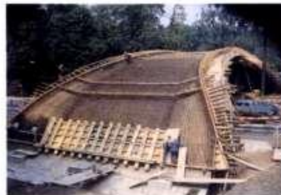
The formwork
