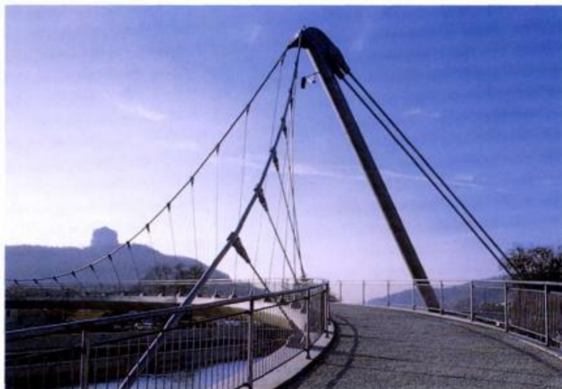
9.57-9.59 Kelheim footbridge (with Kurt Ackermann, architect)
