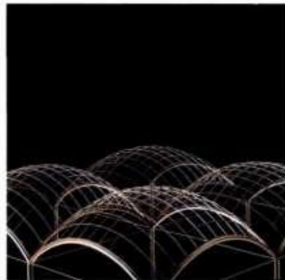
6.48 - 6.50 Helsinki station competition entry. The roof modules 16/16 m have synclastic translational surfaces
