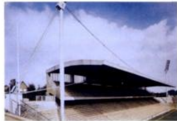
10.19 The grandstand roof at Mönchengladbach, 1977
