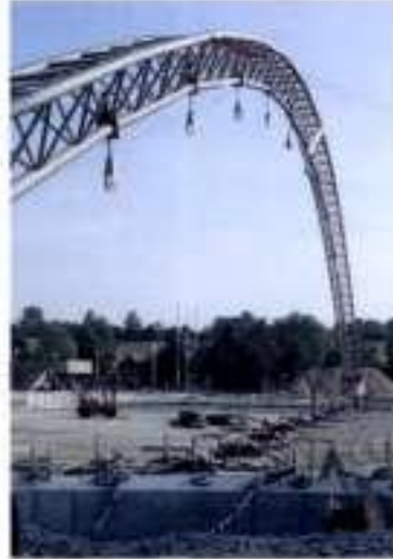
5.68 The arch erected: the cable net assembled on the ground
