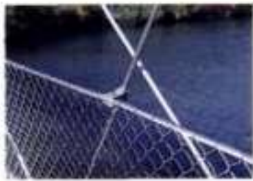
9.37-9.39 Details: cable clamps and handrail
