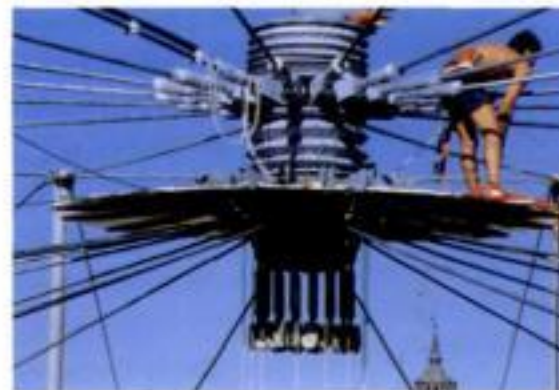
7.47 View of the prestressing system
