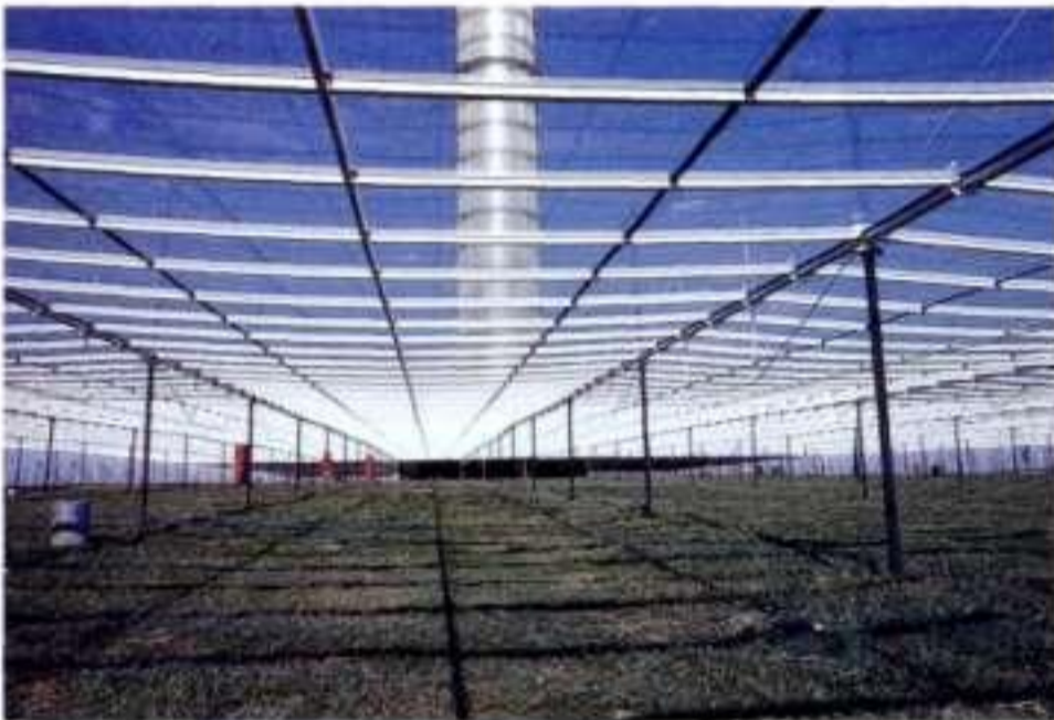
11.51 The glass collector roof from underneath
