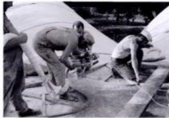
4.20 + 4.21 Glass fibre reinforced concrete: spraying on the form and rolling
