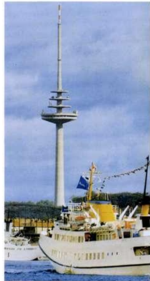
3.25 The telecommunication tower at Kiel (completed 1976)
