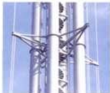
3.40+3.41 The model of the Leipzig Fair tower. Parallel guy wires acting through outriggers prestress and stiffen a core consisting of four tubes which are surrounded by four non-load bearing chimney tubes and with a central access shaft. The tower will support the symbol of the Leipzig Fair
