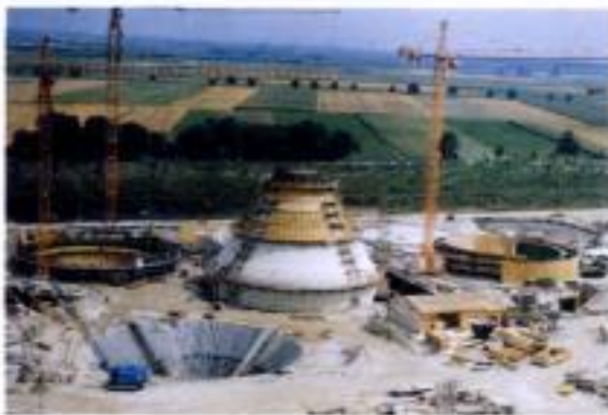
The project under construction
