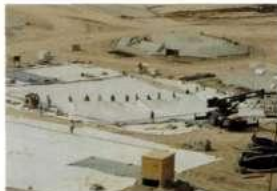
7.5 + 7.6 Riyadh Stadium - Lifting of the membrane
