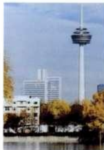
3.32+3.33 The Köln (Cologne) tower (completed 1980)
