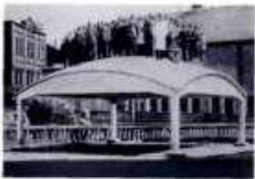
12.2 One of the first concrete shells, a spherical dome only 1.5 cm thick set on a square with sides 7.3 m long. Designed by Dischinger of Dyckerhoff and Widmann, 1932. Ulrich Finsterwalder and Anton Tedesko are part of the load
