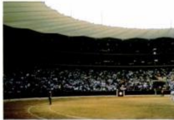
7.44 Close-up of the outer roof viewed from inside the stadium
