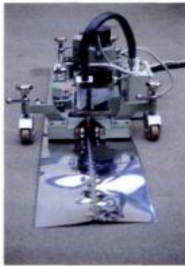
Welding 0.2 to 0.5 mm stainless steel sheet
