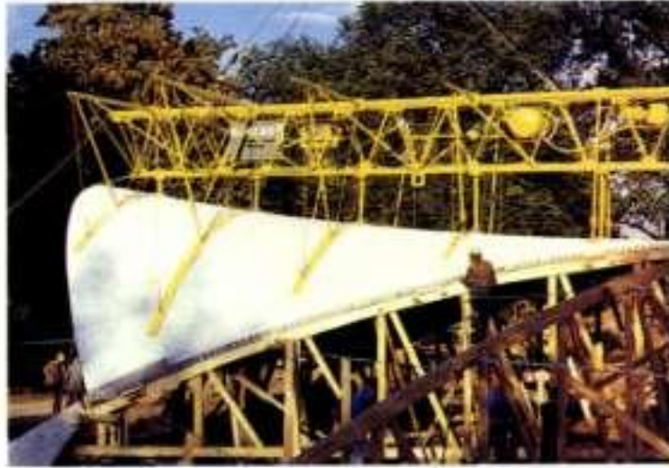
A completed segment still resting on its form
