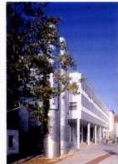
The front of the building
