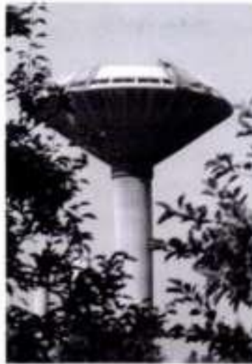
3.37+3.38 The water tower at Leverkusen
