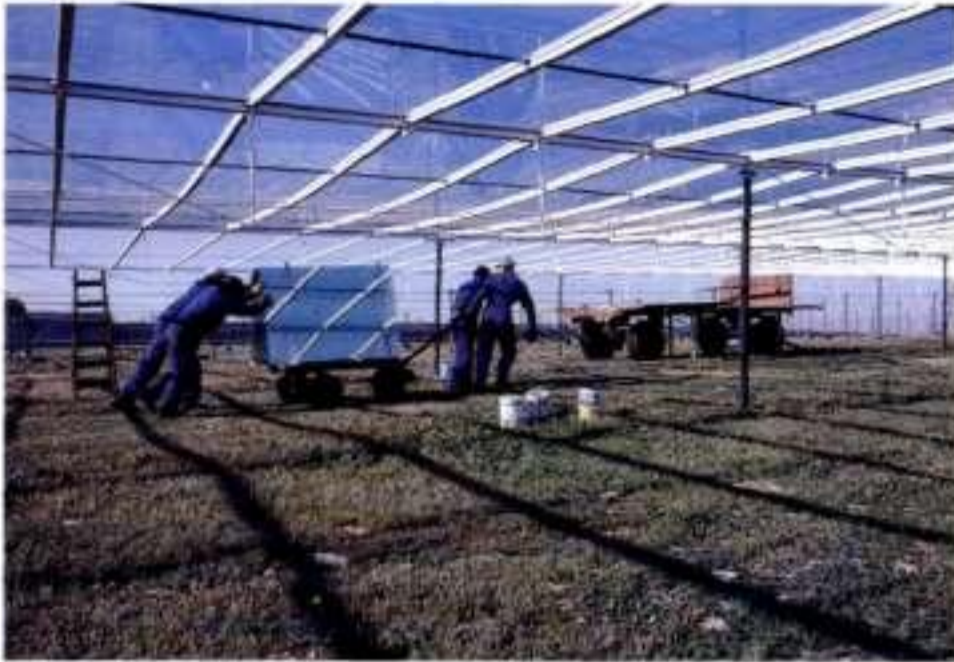
11.50 Fabrication of the later glass collector roof
