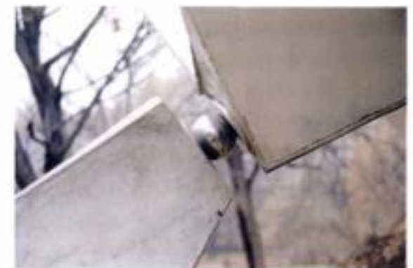
4.23 One of the eight steel balls which support the shell
