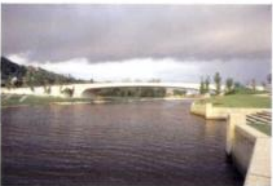
8.72 Kelheim Westtangente: views of the completed bridge
