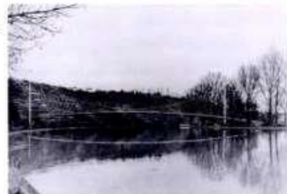
9.33+9.34 Competitive photomontages of: - a box girder bridge of only 75 m span - a suspension bridge of 114 m span
