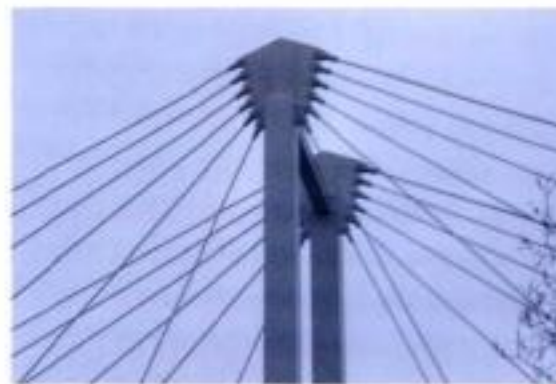
The mast tops before being painted white
