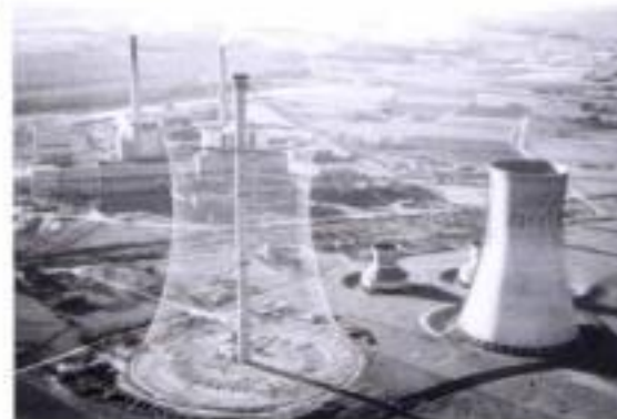
5.107 The completed cable net
