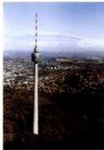
3.2 The Stuttgart television tower of Fritz Leonhardt and Erwin Heinle (completed 1955)
