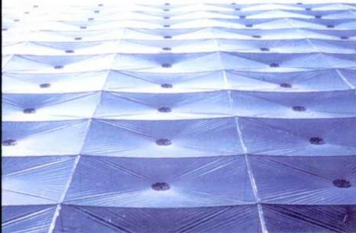
11.44 + 11.45 The plastic collector. The soil underneath is sprayed black
