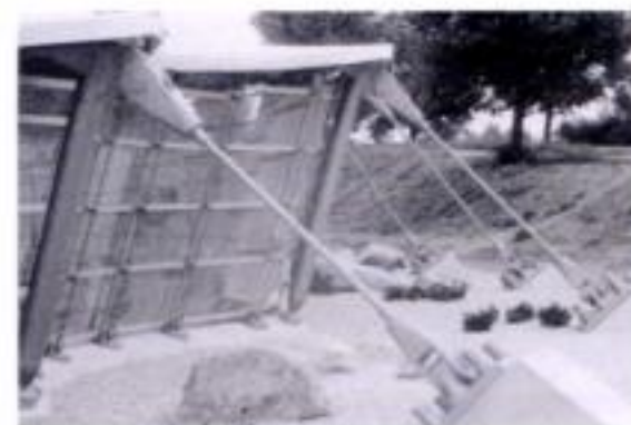
5.79 An exterior view showing the cable-net façade
