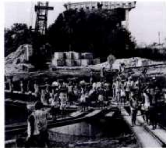
Concreting an end pier well
