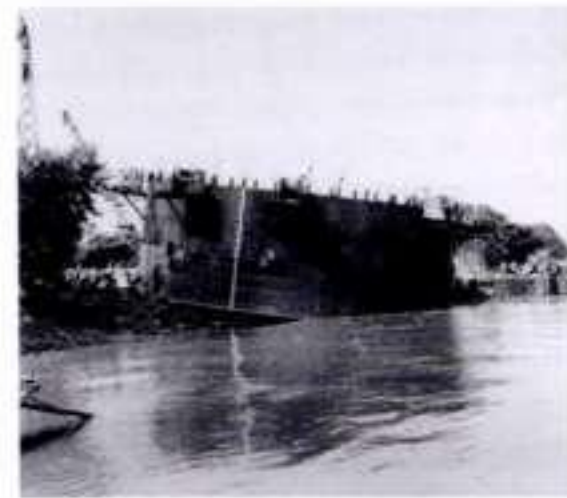
Launching the steel caisson of a pylon foundation
