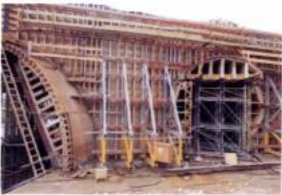
8.71 Falsework and formwork for the pedestrian tunnels through the abutments
