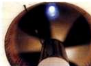
11.54 A view into the chimney from the base looking up (showing also the turbine with the four adjustable blades)
