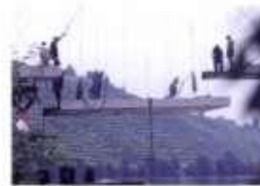
The last unit is lifted
