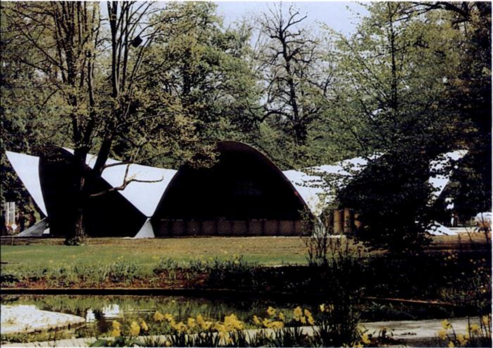
4-27 The completed shell with a temporary façade for the Stuttgart Federal Garden Fair 1977
