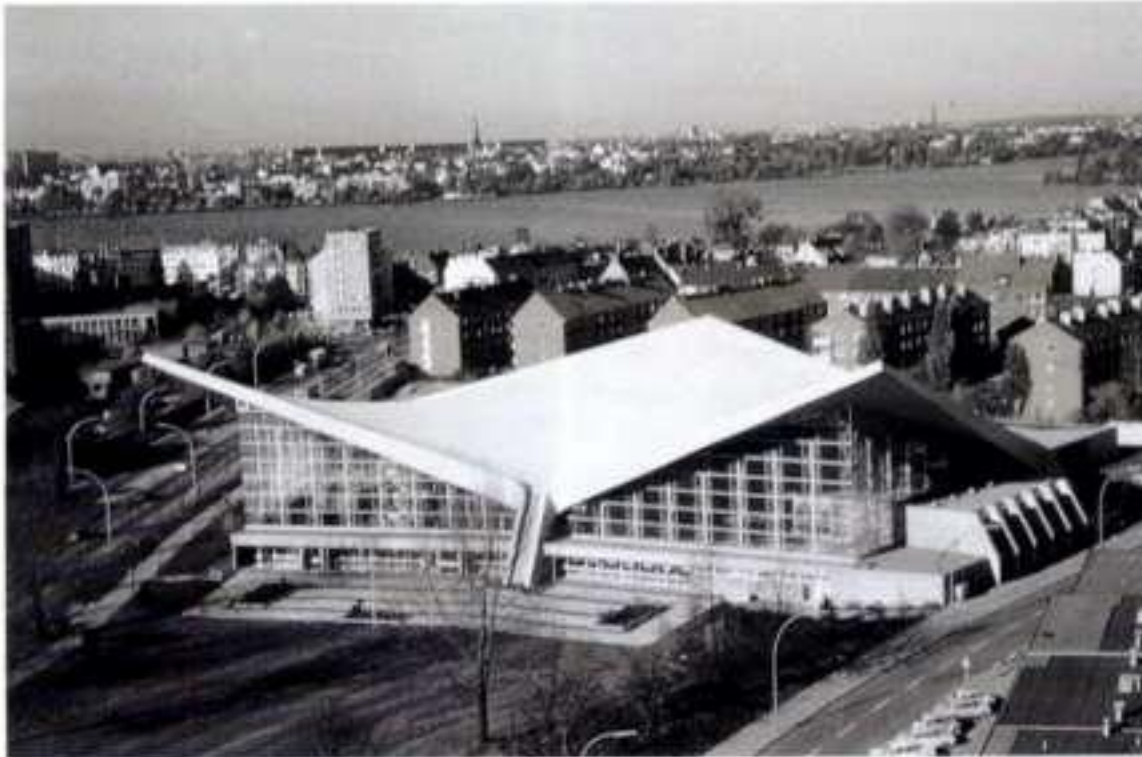
4.2+4.3 The Hamburg-Sechslingspforte swimming centre hypar shell roof (completed 1967)
