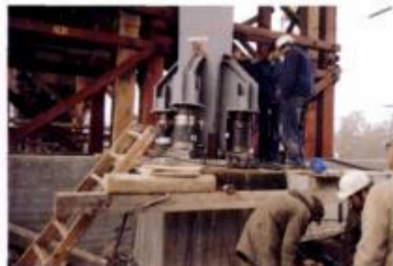
Jacking the mast base ...
