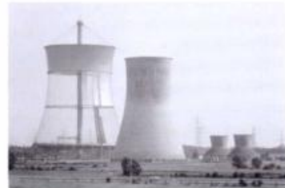
5.108 Installation of cladding
