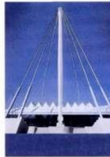
10.13–10.15 Details of mast and cables
