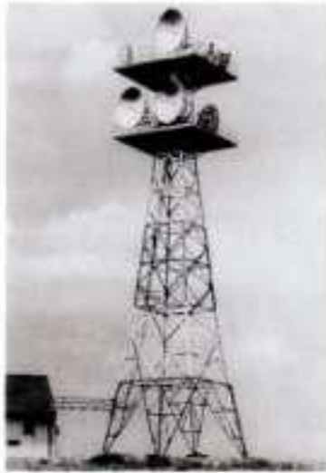
3.1 An example of the once-standard steel lattice transmission towers
