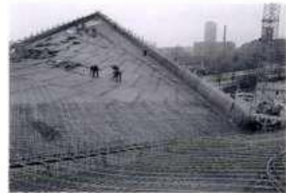
Laying the reinforcement
