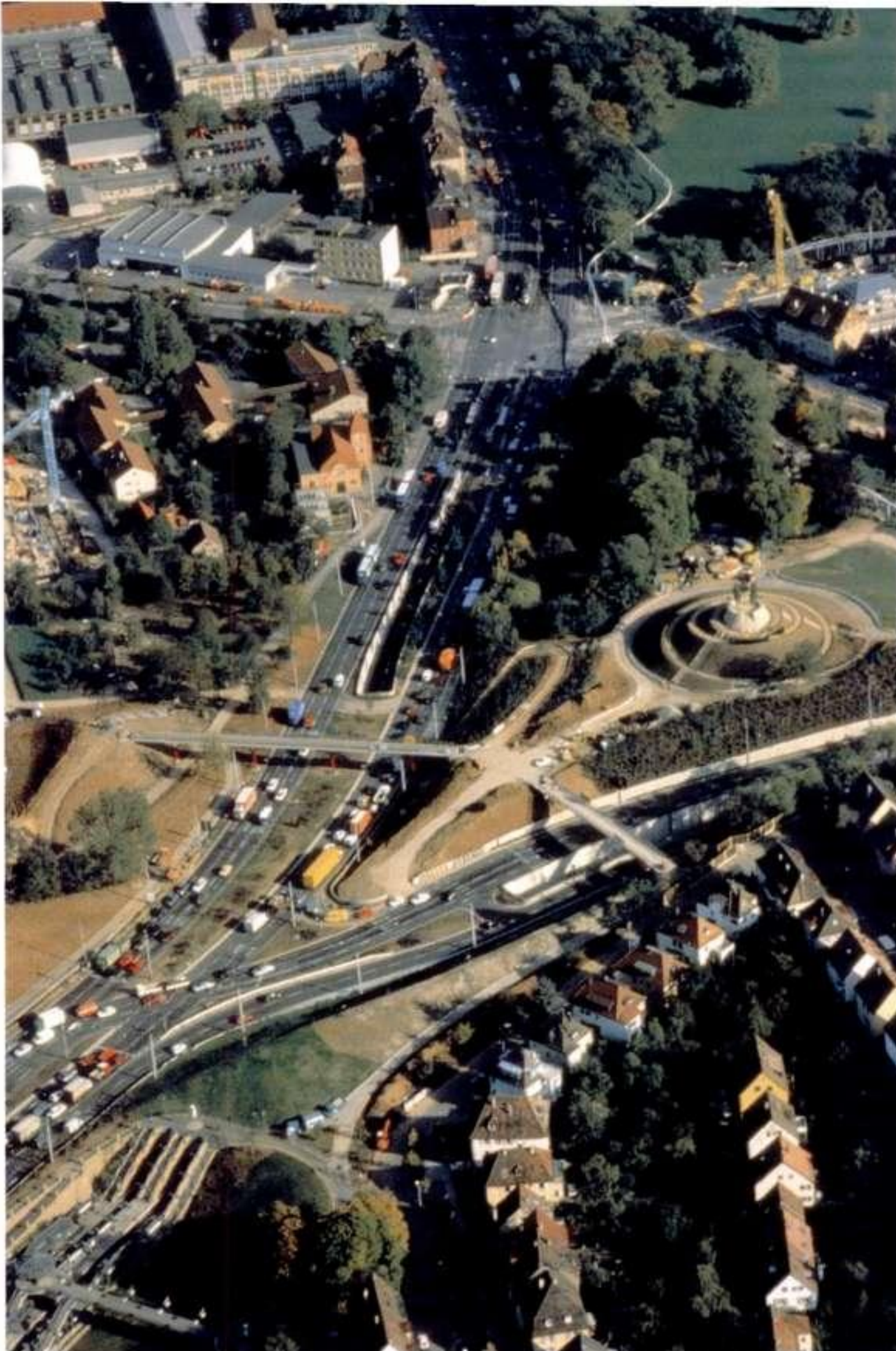
9.116 An aerial view of the Pragsattel (see also 9.74) with its two bridges (9.117 - 9.124) at the centre and the Löwentor cable-net bridge (9.87 to 9.92) - with the yellow crane - in the background
