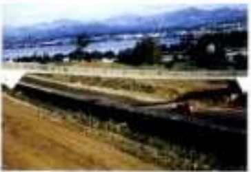
2.15 René Walther's stress ribbon overpass near Zürichsee, 1965
