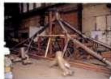
Pre-assembly of a tree-column from tubes with cast steel joints
