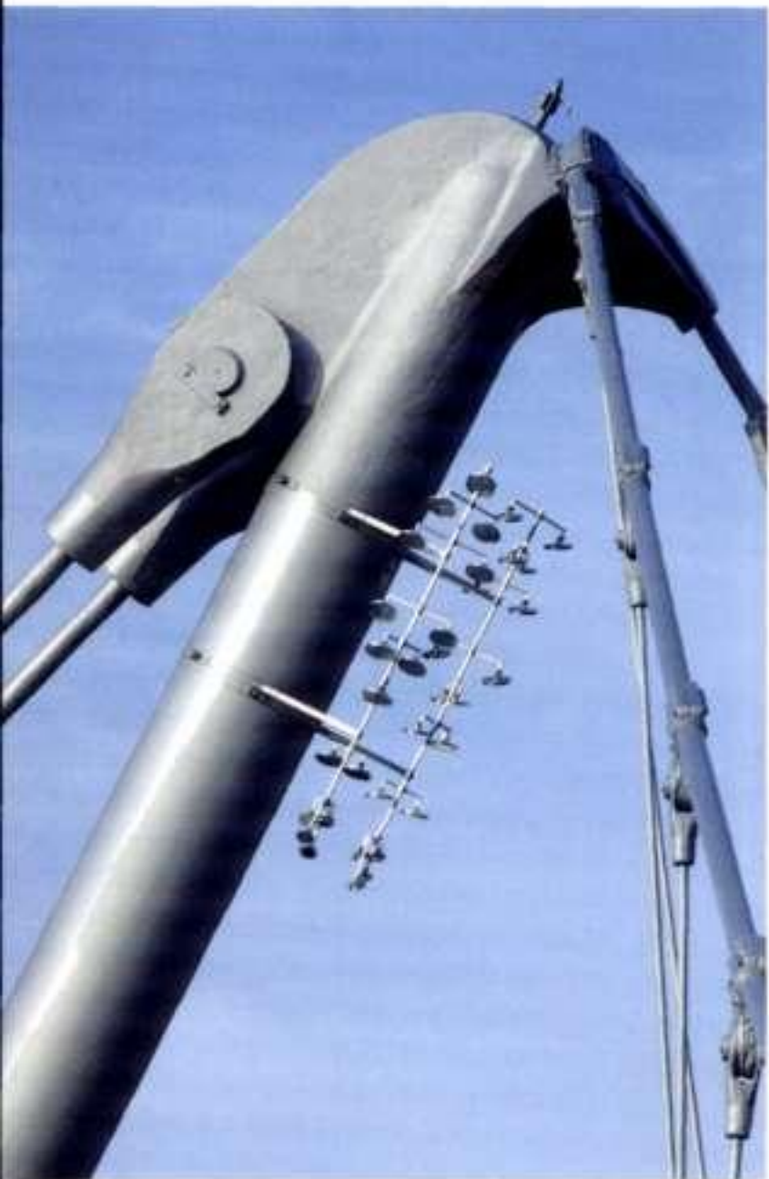
9.55+9.56 Details of the mast and cables
