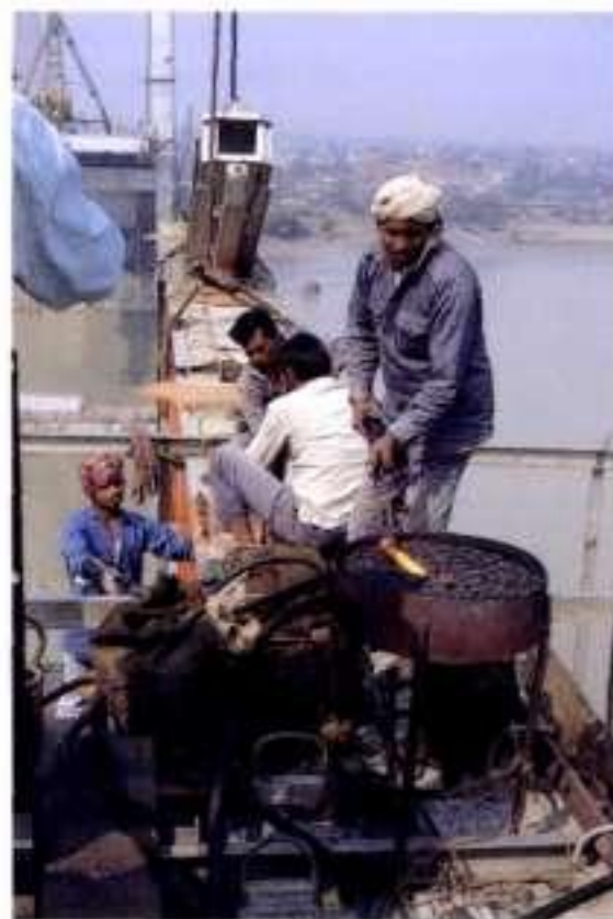
Rivetting of a connection in the freely cantilevering main longitudinal girder
