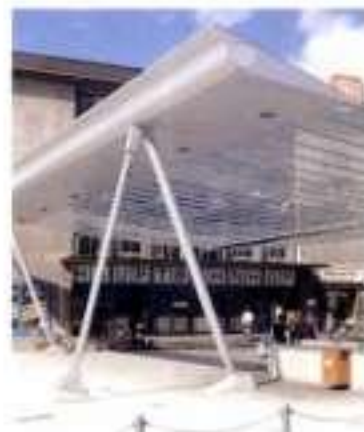
10.29 - 10.32 The suspended glass canopy in front of the Ulm railway station, 1992
