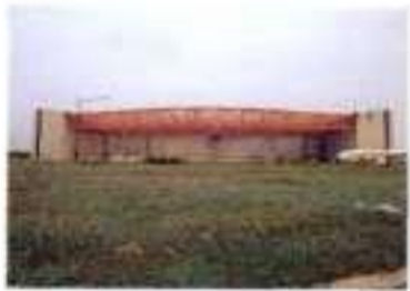
12.8 Changi Airport, Singapore, 1981. Hangar roof designed by Y. S. Law
