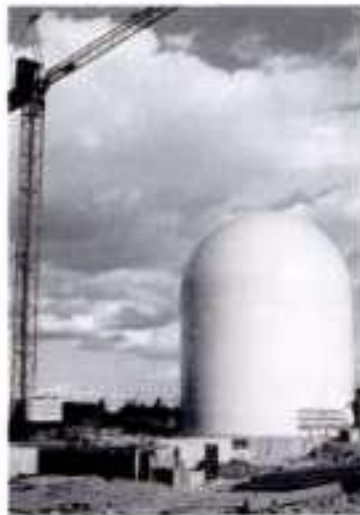
4.30 Inflated shell formwork using the van Eeden system
