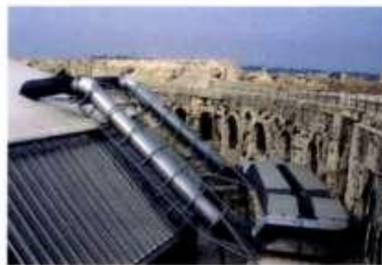
7.34 View of the facade from outside including the blowers and inflation tubes
