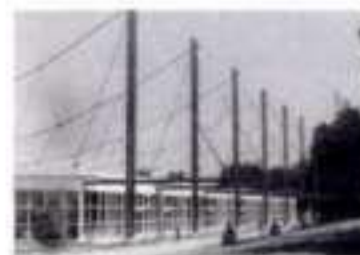
10.16–10.18 The suspended roof of the ice-rink in Memmingen, 1988
