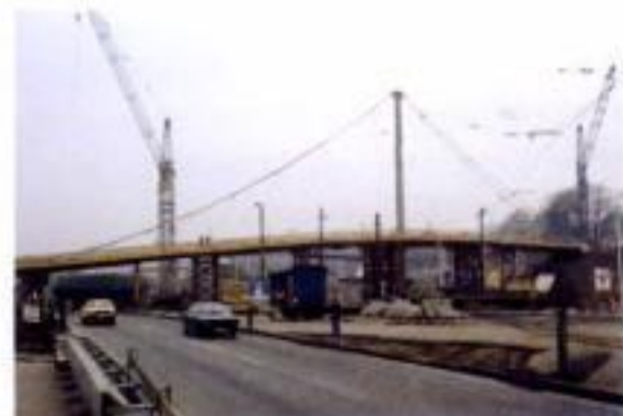
to lift the deck from the formwork
