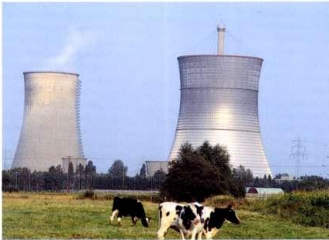
5.88 The cable-net dry cooling tower at Schmehausen. (In the background, a conventional concrete-shell wet cooling tower), photo taken in June 1991
