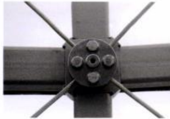
6.43 Joint of slats and cables
