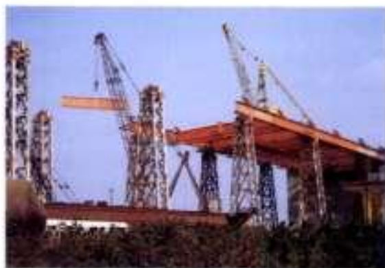
8.14+8.15 The steel grid of the side spans advances over temporary supports
