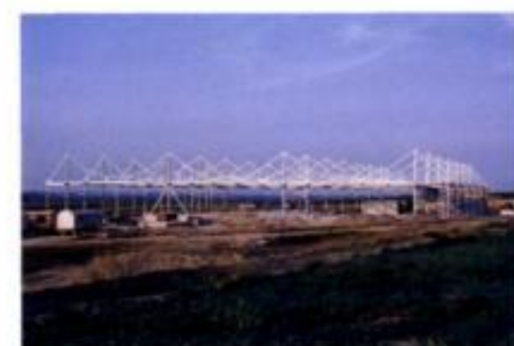
10.20 + 10.21 The Dachwig factory roof during erection, 1993
