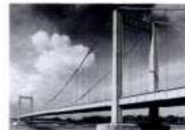
2.7 Fritz Leonhardt's bridge over the Rhine at Rhodenkirchen (1941)
