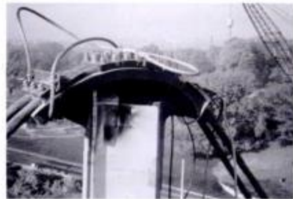
The mast top during construction
