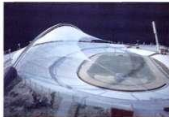
Fig. 5.64 The design model for the cable net roof of the soccer stadium, Hannover (1973)
