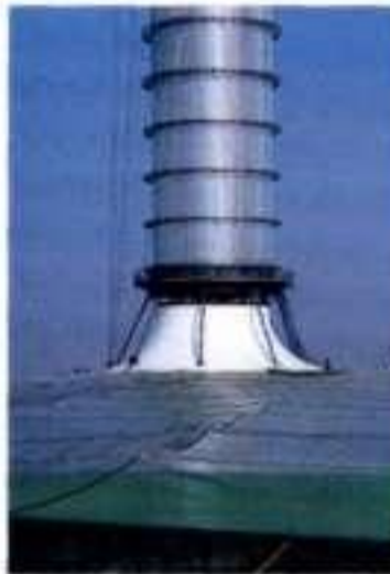
11.53 The transition between collector roof and chimney
