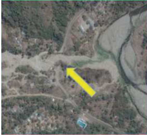
Fig. 5.19 Bridge destroyed from a landslide/debris flow N’ of Aemuta, Flores (Google Earth, City of Ende, access: March 2014)
