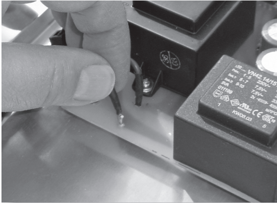
FIGURE 6.31 Using insulating sleeving over a mains circuit soldered joint. Here the joint has been made, and the sleeving is being pushed into position to cover the joint.
