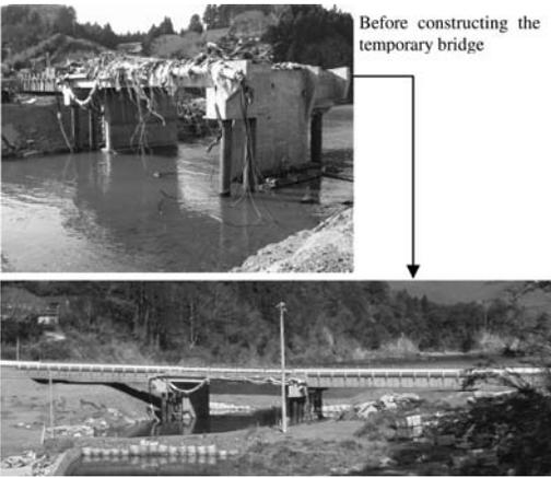
Figure 8. Temporary bridge using the original components
