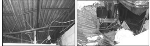
Figure 1. Failure due to increased snow loads.
