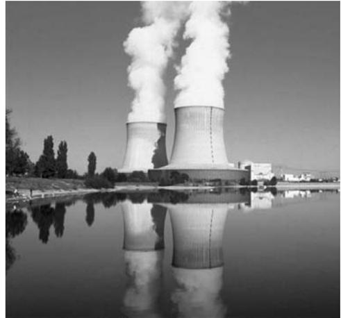
Figure 1. Natural draft cooling towers.
