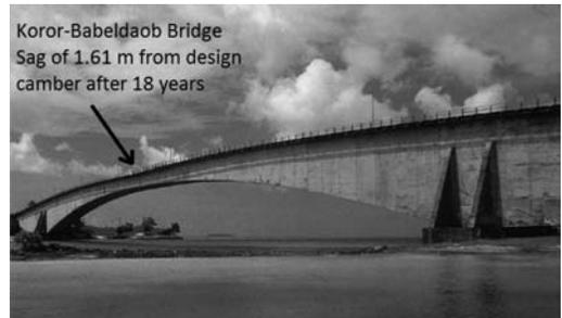
Figure 1. Image of the Palau Bridge shortly before collapse.
