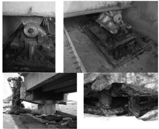
Figure 9. Corrosion of reinforcing bars and bearings attacked by chloride.
