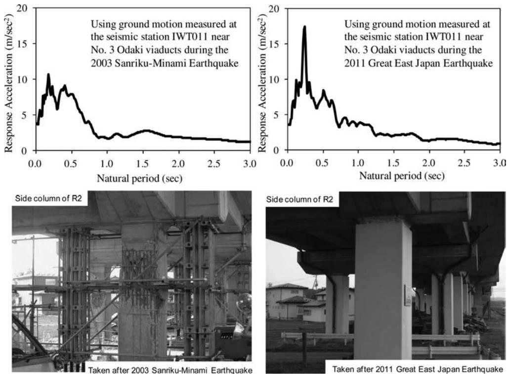
Figure 2. No. 3 Odaki viaduct taken after the 2003 Sanriku-Minami earthquake and the 2011 Great East Japan earthquake (Note: The viaducts were retrofitted before the 2011 Great East Japan earthquake).
