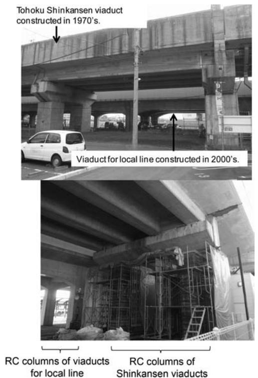
Figure 3. Comparison of damage states of RC columns constructed by 1970's and 2000's.
