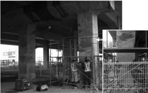
Figure 4. Damage to RC columns repaired after the 2011 Great East Japan earthquake on March 11 due to the large aftershock on April 7.
