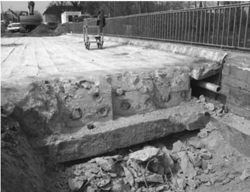
Figure 1. View on the 80 cm thick superstructure.
