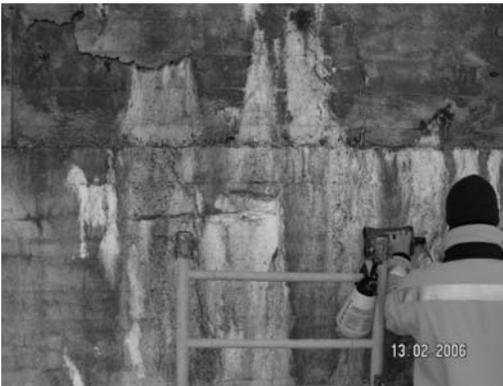
Figure 1. Corrosion case or mainly visual effect? A corrosion survey helps to understand and to decide correctly.
