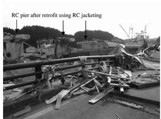
Figure 6. RC bridge pier with retrofit using RC jacketing which had no damage during the 2011 Great East Japan earthquake.
