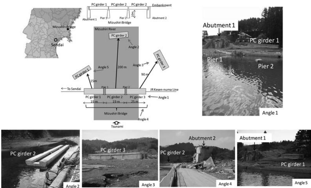
Figure 5. Damage to Mizushiri bridge by the tsunami due to the 2011 Great East Japan earthquake.
