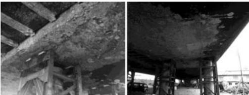
Figure 1. Visual impression of fire damaged bridge sections.
