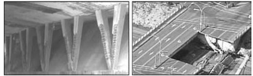
Figure 2. Failure due to the use of deicing salts.
