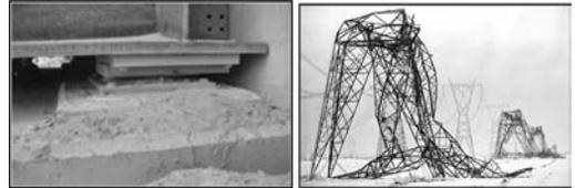
Figure 3. Failure due to temperature loads (left) and failure due to freezing rain (right).
