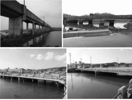
Figure 7. Bridges which were not washed away by tsunami
