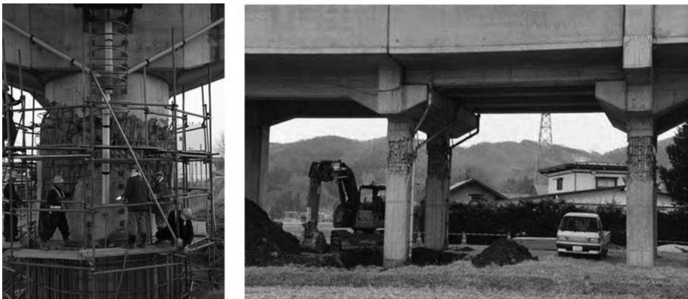
Figure 1. Example of damages to Tohoku Shinkansen viaducts before retrofit during the 2011 Great East Japan earthquake (Left and right photos were provided by East Japan Railway Company and Dr. Takahashi, Kyoto University, respectively).
