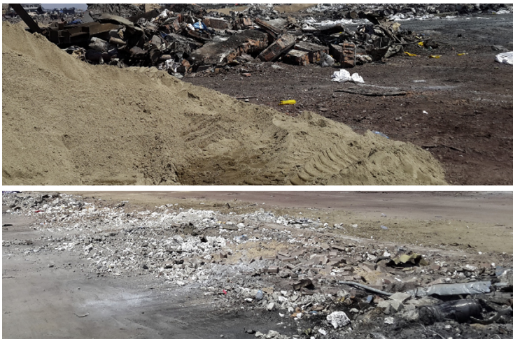
Figure 4.14 Pictures of construction and demolition waste generated in a great fire/explosion accident.
