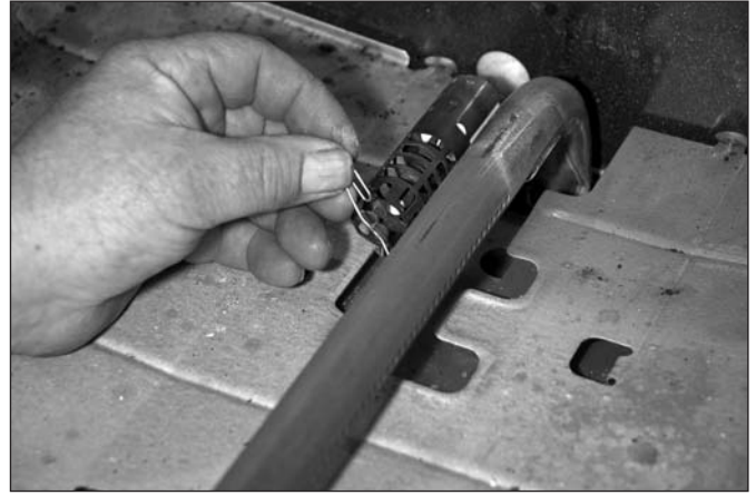
Figure 11-6: Cleaning burner flame openings
