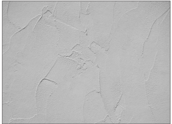
Figure 8-61: Spanish texture on drywall (Image copyright Cousin_Avi, 2009. Used under license from Shutterstock.com)
