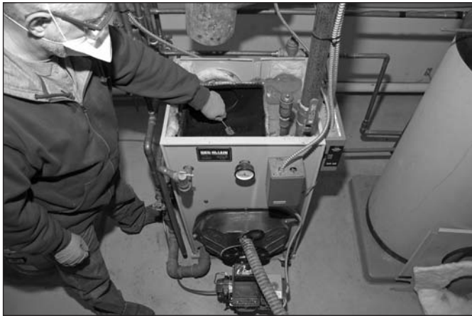
Figure 10-25: Boiler being cleaned
