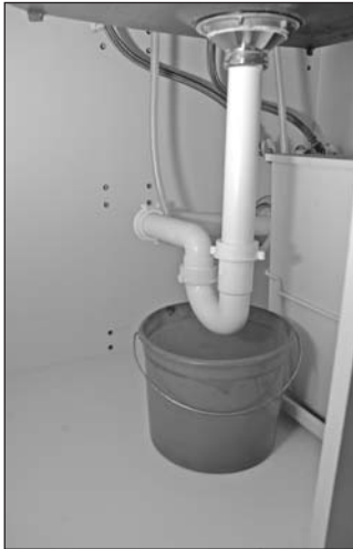
Figure 9-40: Place a bucket under a sink
