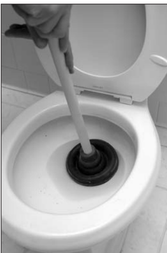
Figure 9-37: Plunger covering drain opening
