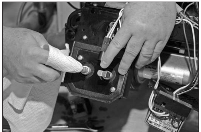
Figure 10-36: Cleaning the springs
