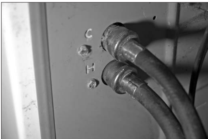
Figure 11-48: Inlet valve
