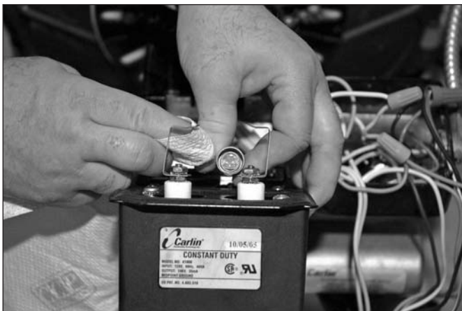
Figure 10-35: Cleaning the cad cell
