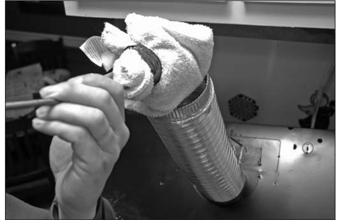
Figure 11-43: Clean exhaust ductwork
