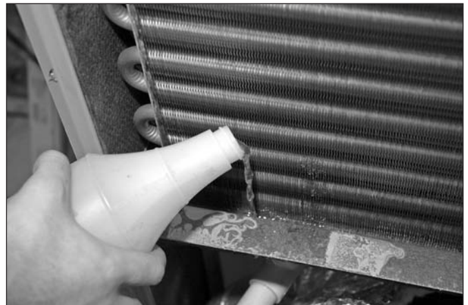
Figure 10-53: Pour water into condensate drain pan
