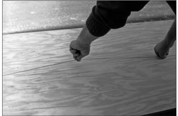
Figure 4-16: Snapping a chalk line
