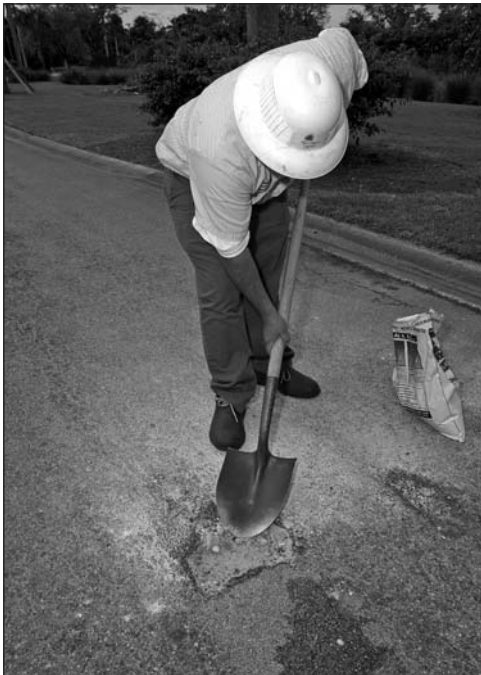
Figure 15-44: Clear loose debris
