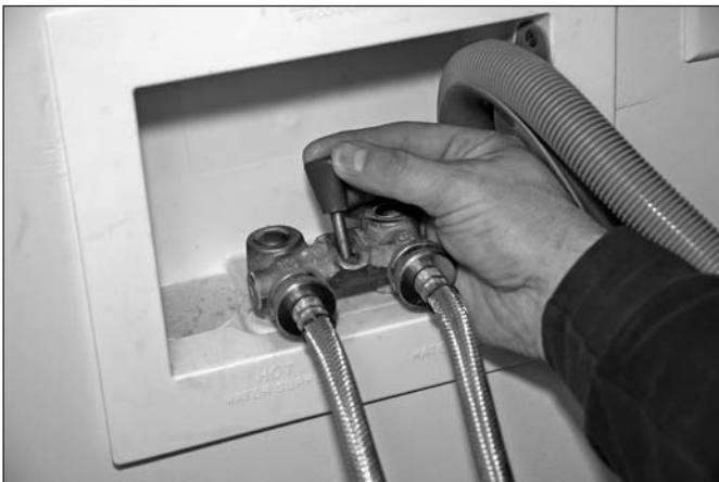
Figure 11-51: Inlet valve
