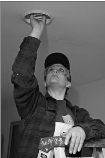
Figure 6-49: Removing light bulb
