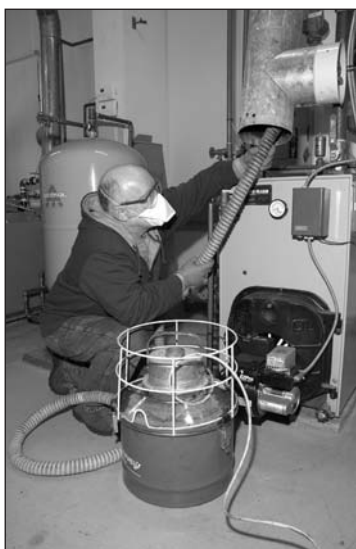
Figure 10-28: Cleaning the flue
