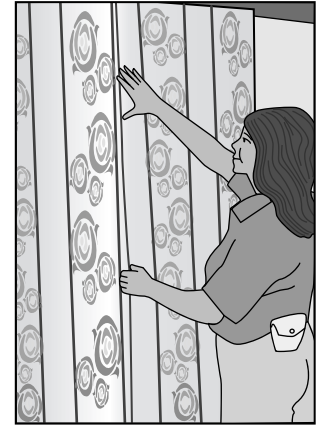
Figure 8-45: Aligning the pattern and butting the seams together
