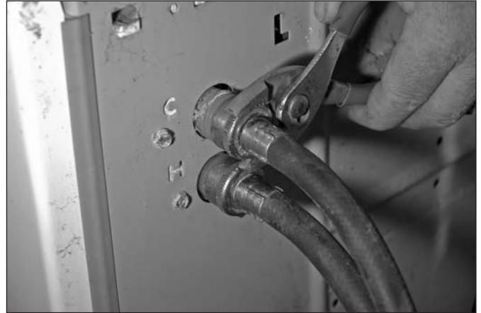
Figure 11-50: Disconnect hoses
