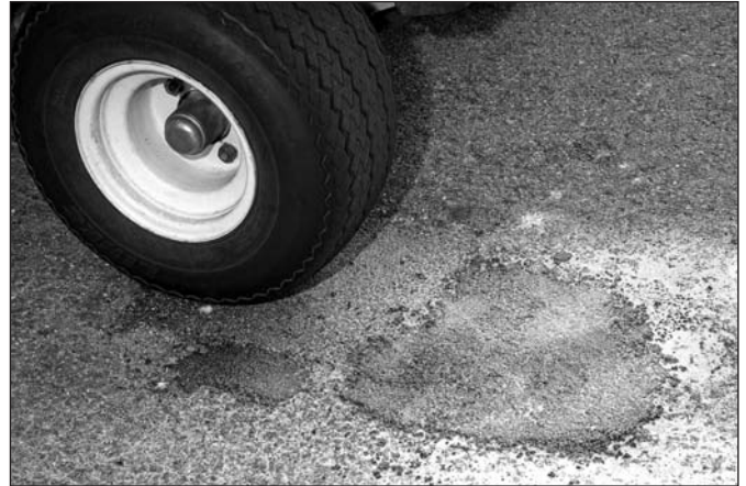
Figure 15-47: Drive a car over the cold patch to spread it
