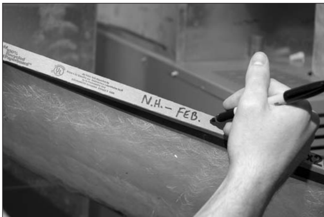
Figure 10-20: Mark or initial the filter
