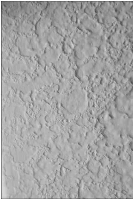
Figure 8-58: Knockdown texture on drywall (Image copyright Kanwarjit Singh Boparai, 2009. Used under license from Shutterstock.com)
