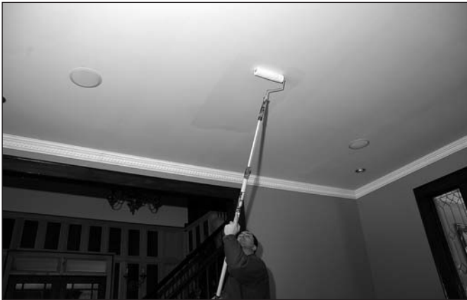
Figure 8-20: Paint ceiling in small sections
