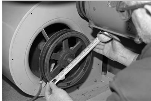
Figure 10-11: Measure pulley diameters
