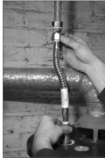
Figure 9-58: Install water lines
