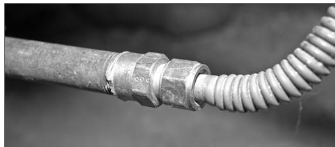
Figure 11-12: Connector line connecting gas lines
