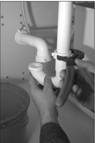
Figure 9-43: Replacing a sink trap using angled jaw pliers
