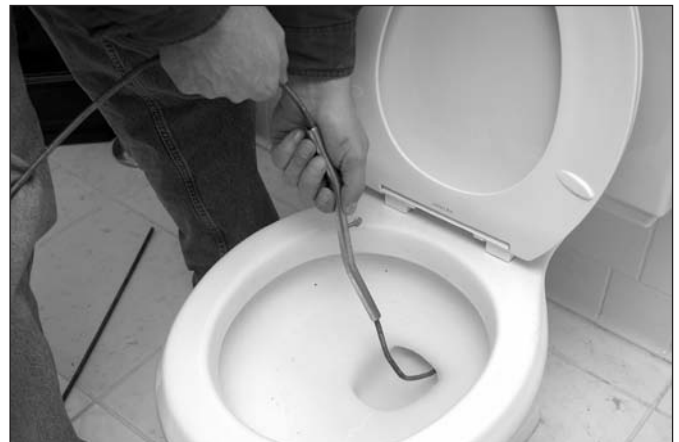
Figure 9-46: Pushing auger cable into drain opening
