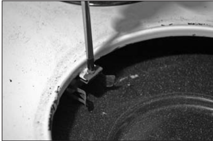
Figure 11-21: Disconnecting old receptacle
