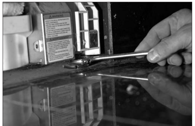
Figure 11-40: Leveling legs of dishwasher
