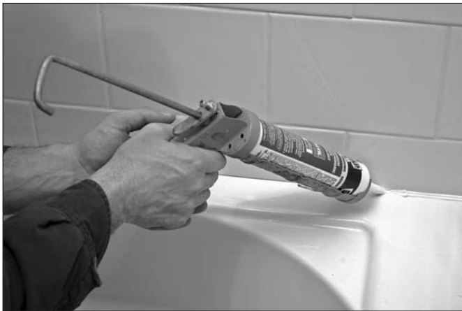
Figure 9-49: Applying caulking
