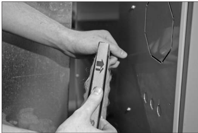
Figure 10-19: Directional arrow on the filter
