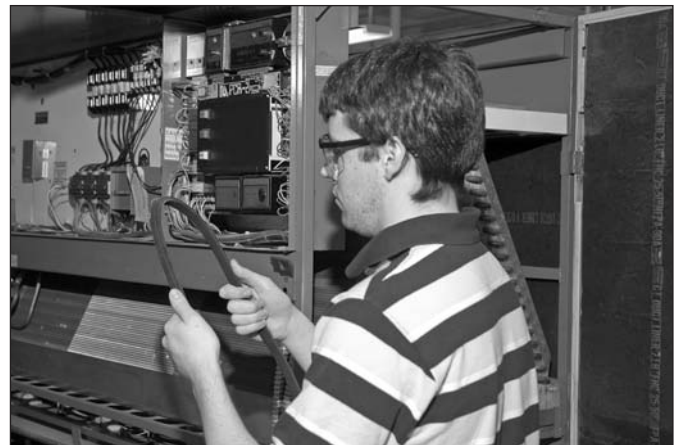
Figure 10-4: Technician inspecting the belt
