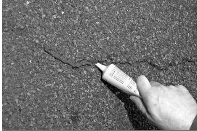
Figure 15-43: Apply crackfiller to the crack
