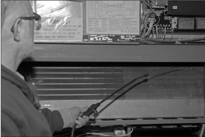
Figure 10-47: Spray the coil cleaner on the coil
