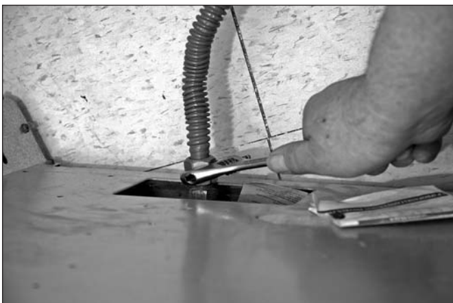
Figure 11-9: Disconnect gas lines
