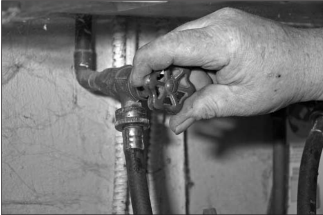
Figure 11-49: Shutting off water supply
