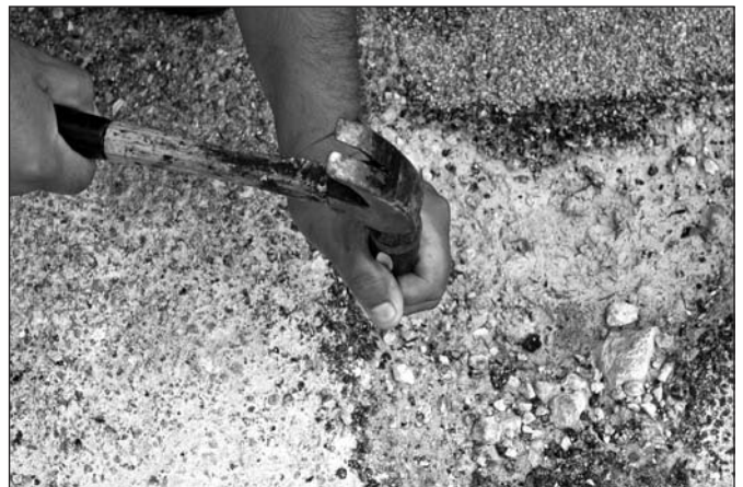
Figure 15-45: Use hammer or cold chisel to remove jagged edges around a hole
