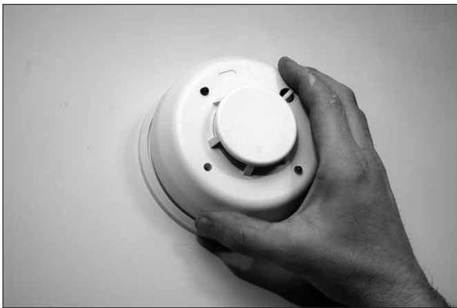
Figure 6-40: Removing faulty detector
