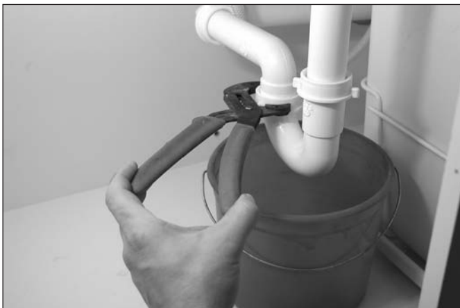
Figure 9-38: Removing a sink trap using angled jaw pliers
