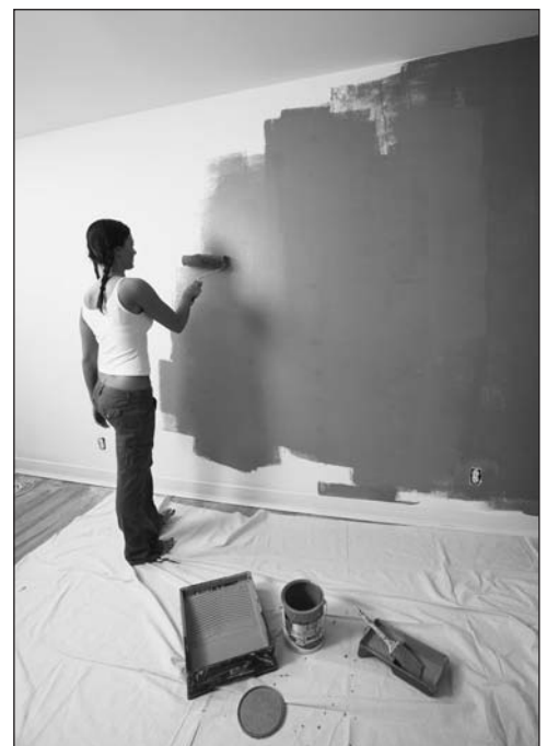
Figure 8-21: Painting a wall with a roller
