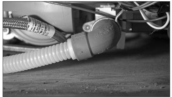
Figure 11-39: Drain line connection
