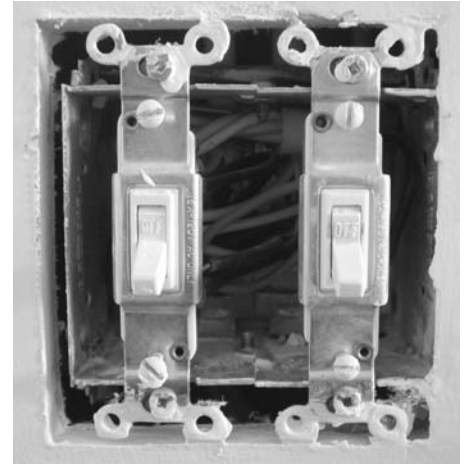
Figure 6-44: Cover plate removed (Image copyright Tootles, 2009. Used under license from Shutterstock.com)
