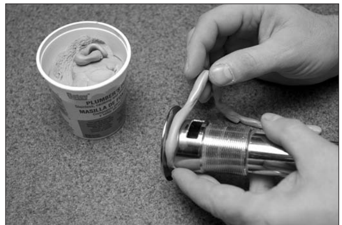
Figure 9-52: Applying caulk on drain outlet
