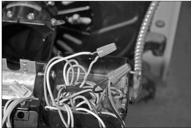
Figure 10-40: Side-by-side nut connections done correctly and incorrectly
