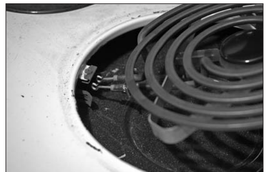
Figure 11-20: Installing new heating elements
