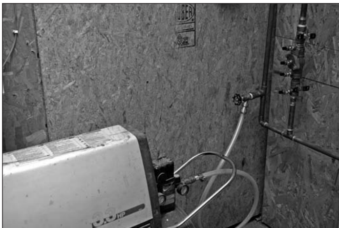
Figure 15-24: Compressor attached to the mainline
