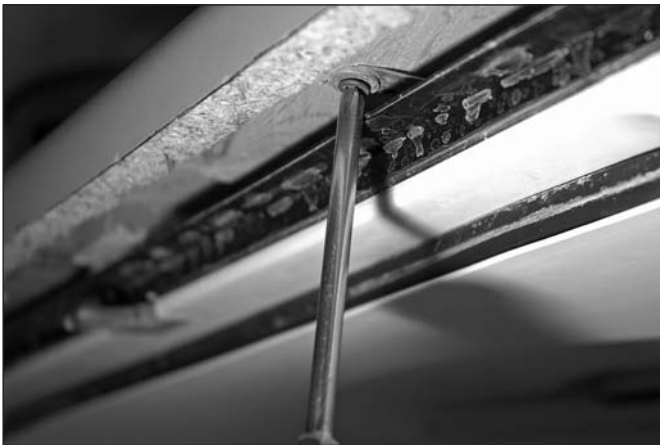
Figure 11-38: Removing screws in counter
