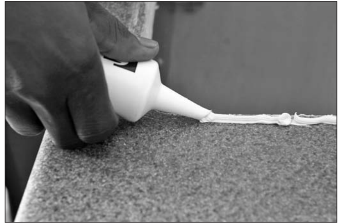
Figure 4-9: Person applying caulk
