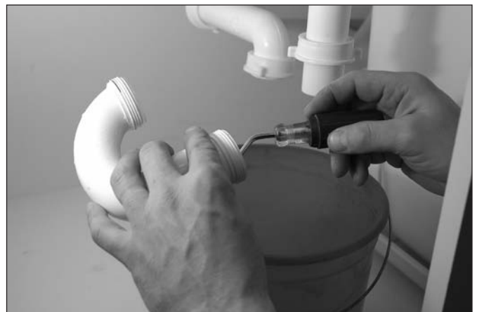
Figure 9-39: Probing with a screwdriver
