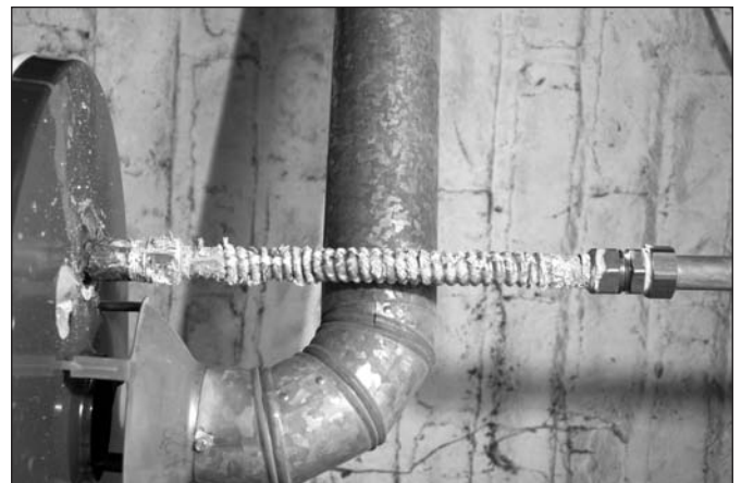
Figure 9-56: Disconnect water lines
