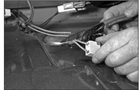
Figure 11-23: Wires being cut
