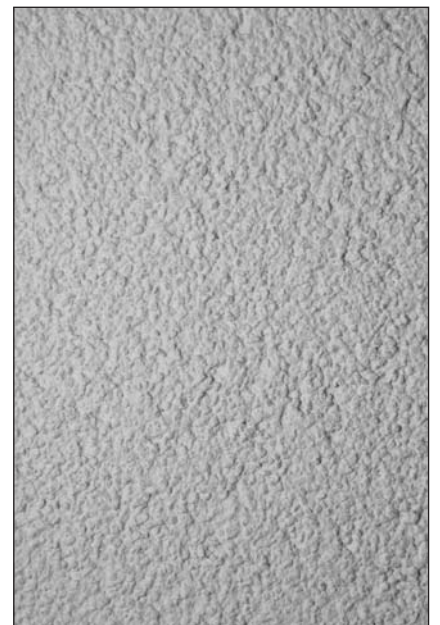
Figure 8-57: Orange peel texture on drywall (Image copyright Simon Krzic, 2009. Used under license from Shutterstock.com)
