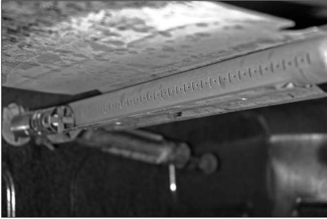
Figure 11-5: Upper burner in the oven of a gas stove
