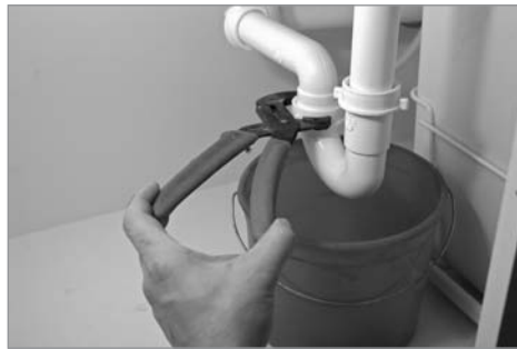
Figure 9-41: Removing a sink trap using angled jaw pliers to unclog a drain using a sink snake
