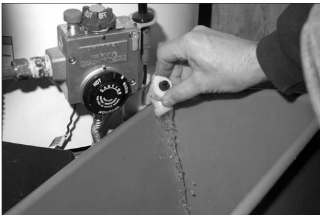
Figure 9-55: Drain the water heater
