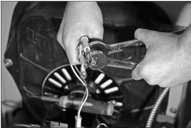
Figure 10-33: Replacing the nozzle on the oil heating system
