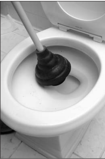
Figure 9-36: Positioning plunger over drain opening
