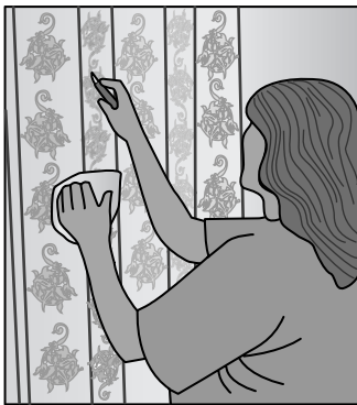
Figure 8-46: Rolling the edges with a seam roller
