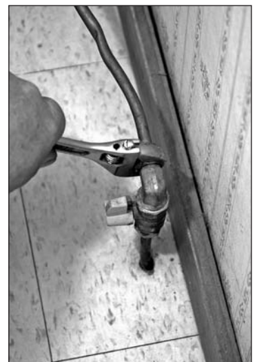
Figure 11-8: Disconnect copper tubing
