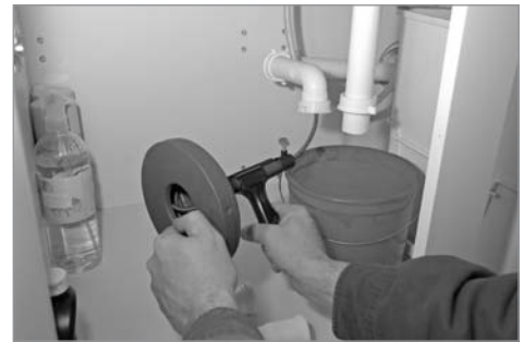
Figure 9-42: Using a sink snake
