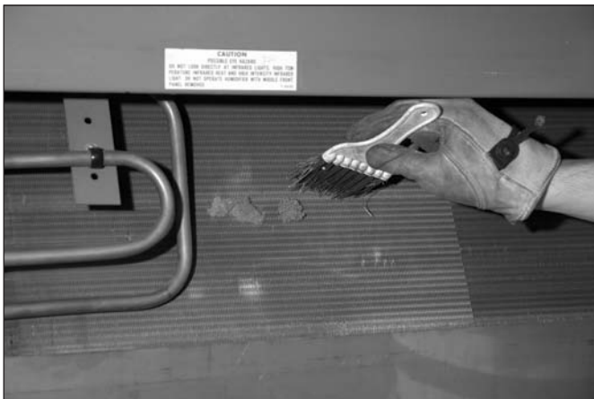
Figure 10-45: Brush the evaporator coil
