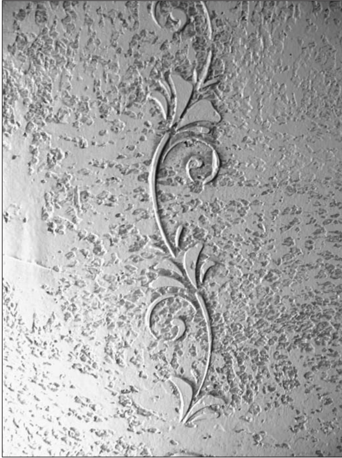
Figure 8-64: Drag texture on drywall (Image copyright Thoma, 2009. Used under license from Shutterstock.com)
