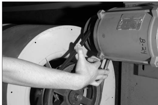
Figure 10-7: Check the belt tension
