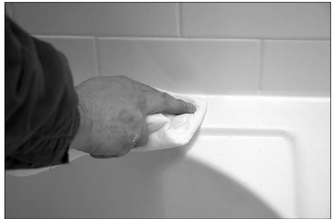
Figure 9-50: Smoothing caulking with your finger
