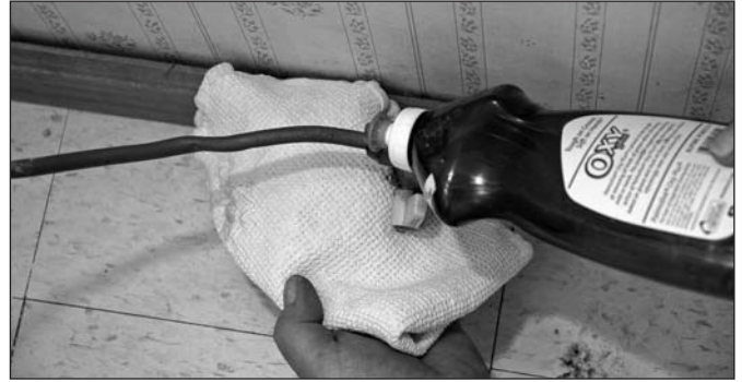
Figure 11-13: Testing gas line
