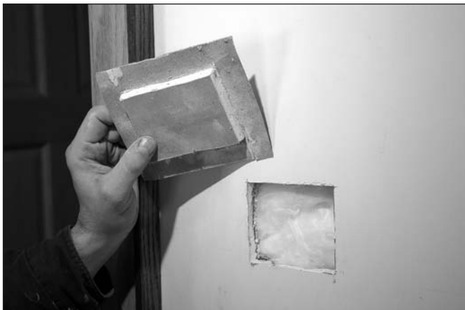
Figure 8-8: Cut drywall patch
