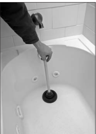
Figure 9-44: Using a plunger in bathtub to unclog drain
