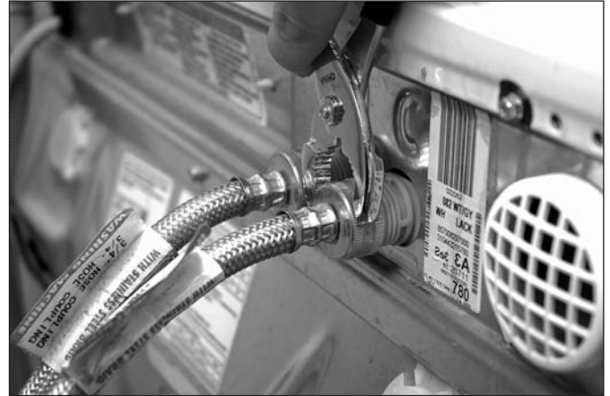
Figure 11-57: Attach hose to the washer
