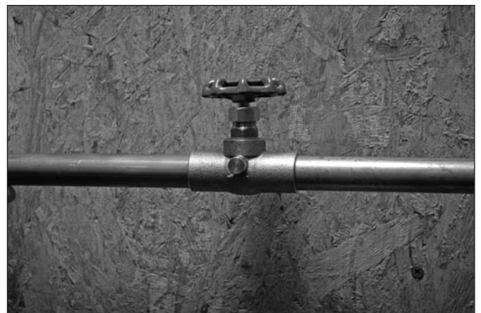
Figure 15-18: Stop/waste valve
