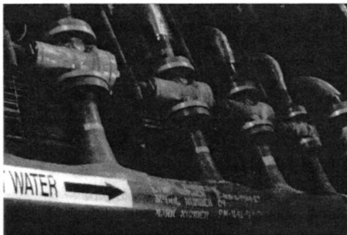
Figure 5.6 FRP piping in a water flood plant.
