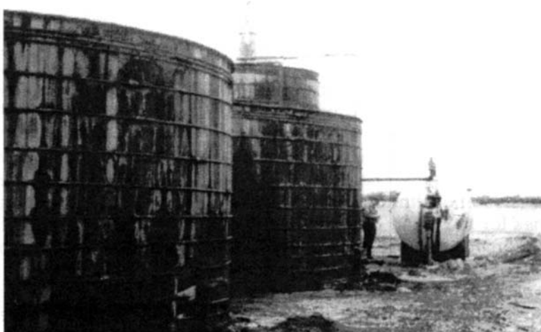
Figure 5.1 Wooden tank battery in a western Kansas oil field producing sour gas, crude, and water. The taller vessel—called a “gun barrel”—serves as a free-water knockout. (Photo circa 1970.)
