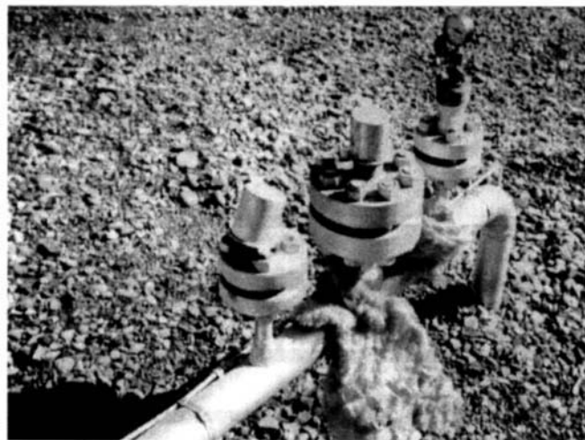
Figure 10.1 Monitoring installation on a sour gas gathering line in western Canada. Three monitoring techniques are in use on this line. All three are installed through access fitting that allows servicing the equipment while the line is in operation at normal producing pressure. They are, left to right, an electrical resistance probe, corrosion coupons, and a hydrogen probe.
