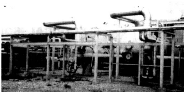
Figure 9.1 Typical plant piping. Note the control valve piping forming water traps.
