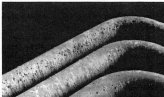
Figure 11.1 Transfer lines between storage tanks and a tanker berth. These overwater lines were coated to withstand the marine atmospheric environment.
