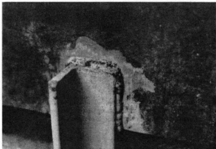
Figure 6.7 Poor weld not properly ground.
