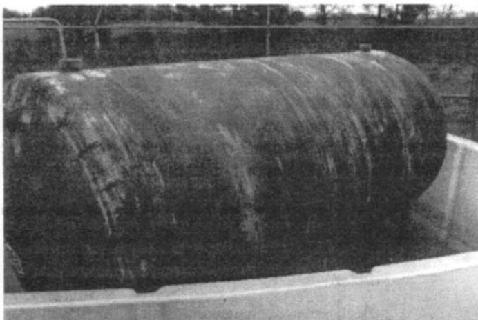
Figure 5.11 A FRP tank used for chemical storage. Note the secondary containment walls.
