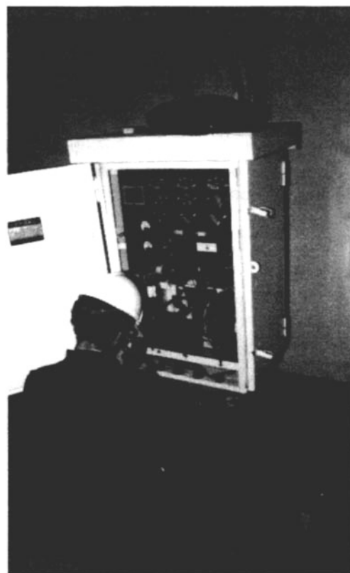
Figure 7.17 A CP rectifier on an offshore facility.
