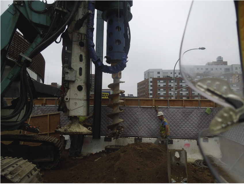
Plate 2.1 Auger drill rig.
