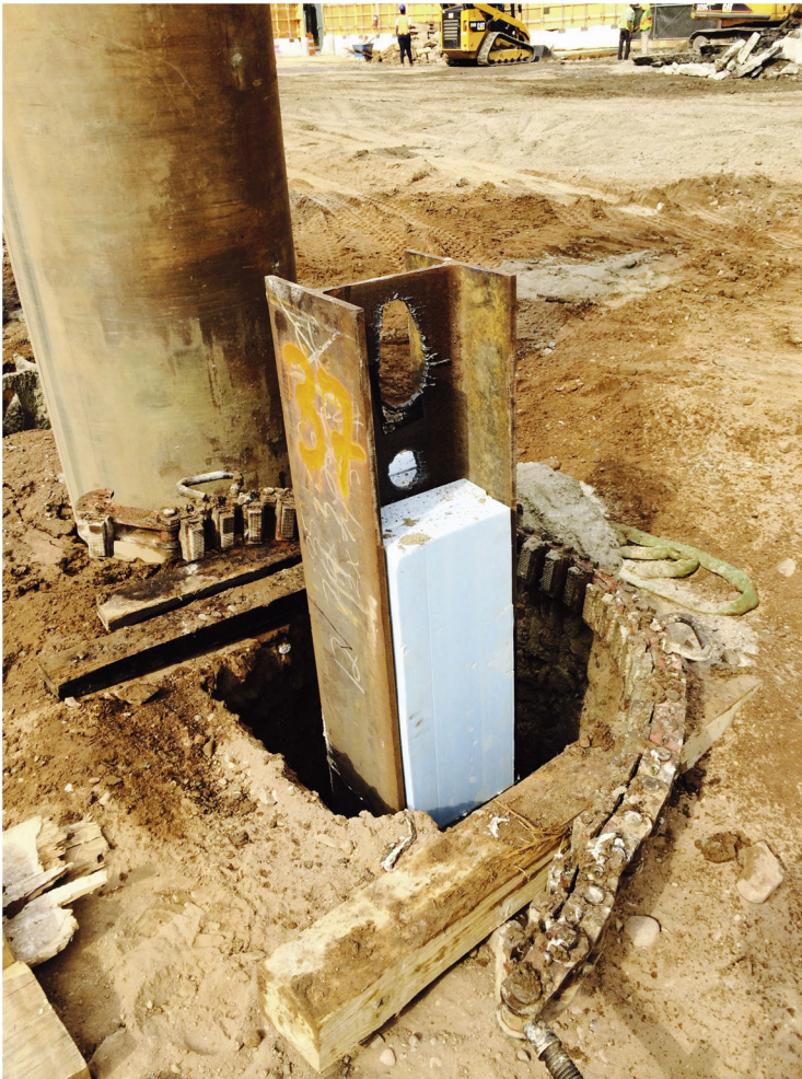
Plate 40.2 Steel H-pile.
