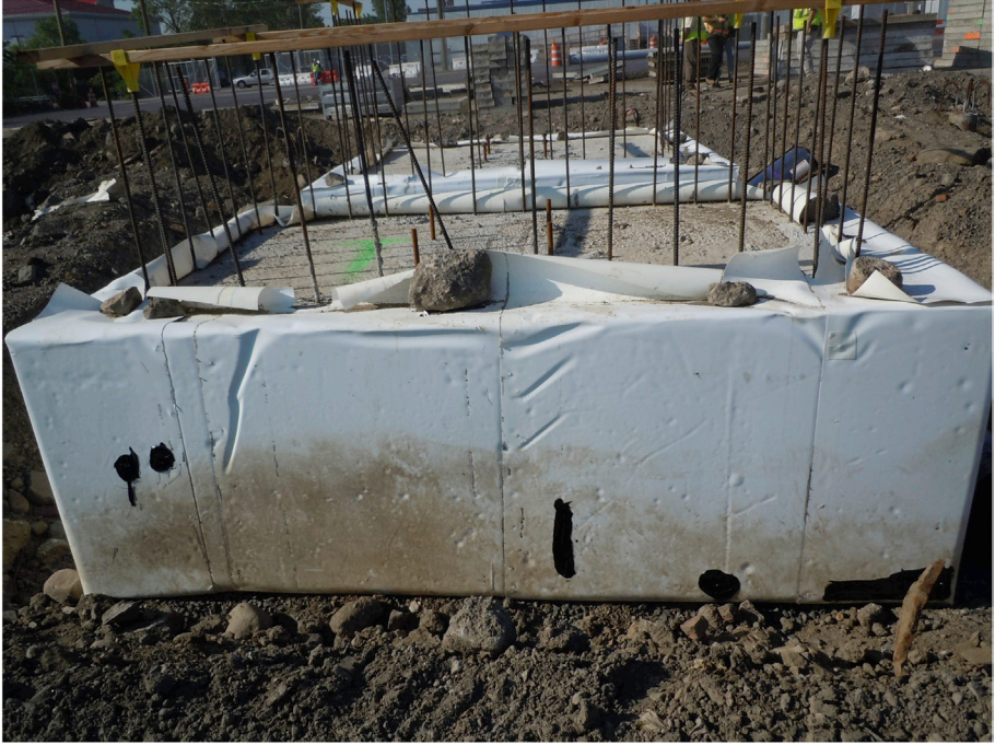
Plate 14.2 Pile cap after concreting.
