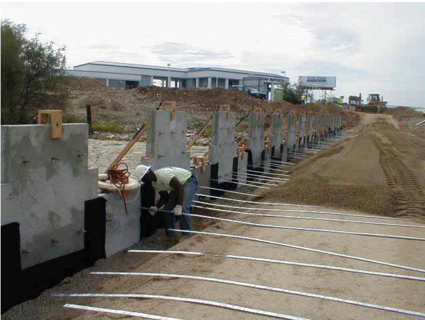
Plate 24.1 Construction of metal strips.
