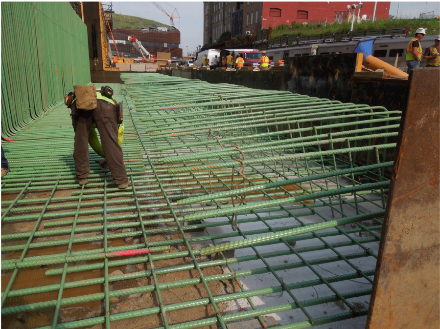
Plate 30.1 Rebars for a raft.
