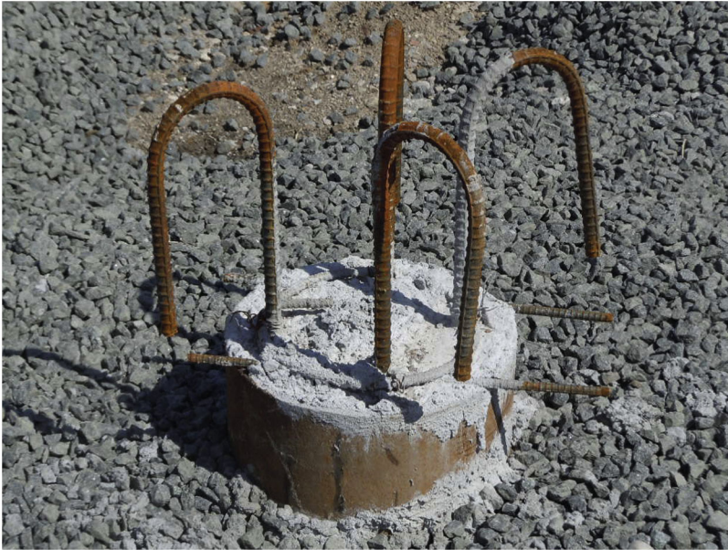
Plate 40.8 Concrete pipe pile.
