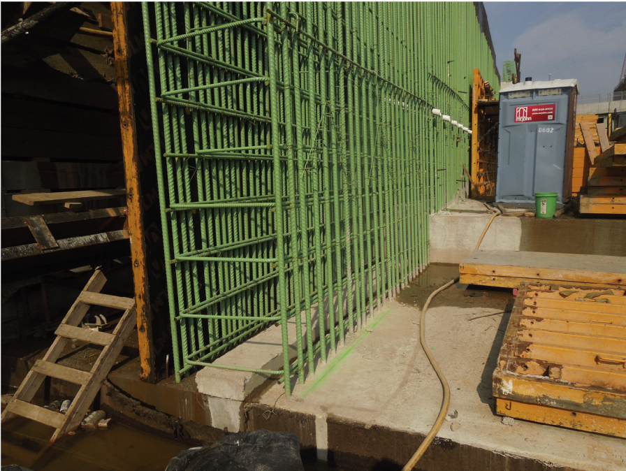
Plate 25.1 Rebars for a cantilever retaining wall.
