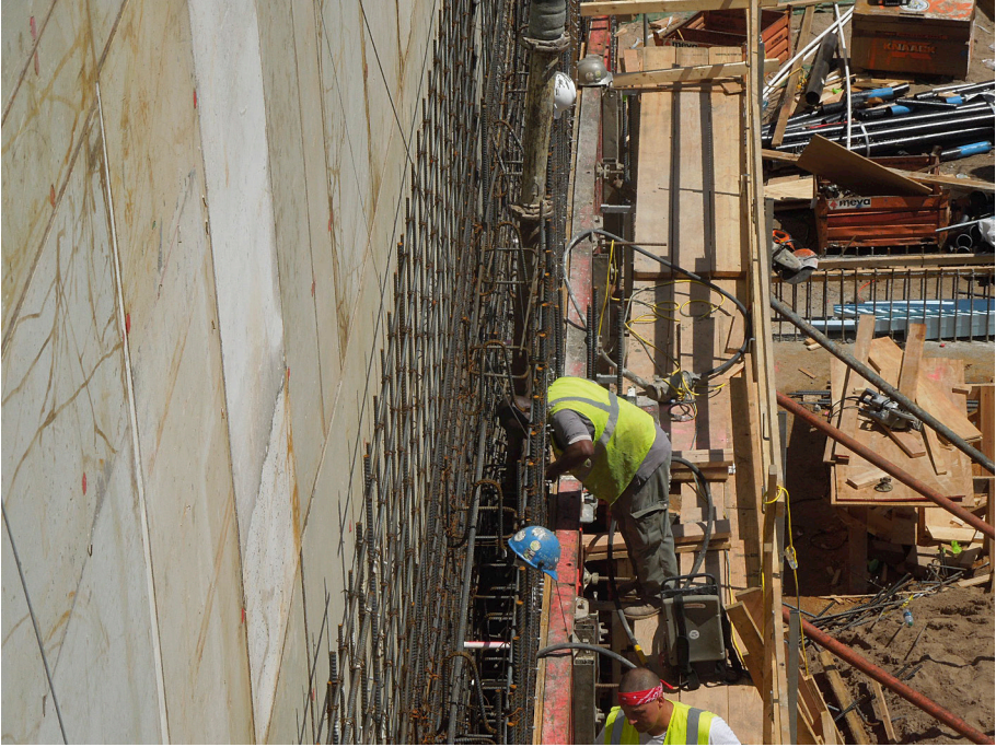
Plate 20.2 Concreting the stem of a cantilever wall.
