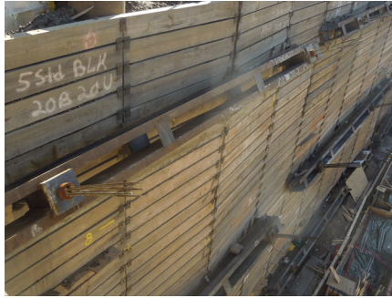
Plate 34.2 Soil anchors and wales.
