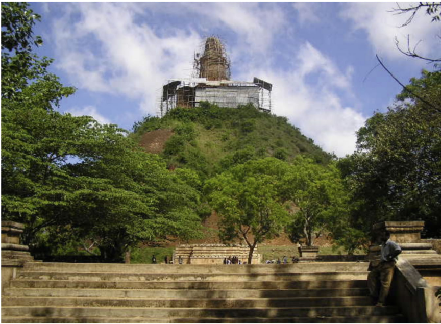
Plate 40.1 Jethavana structure with a 252 ft. deep shallow foundation.
