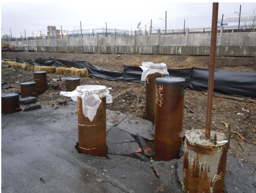
Plate 40.7 Installed pipe piles.
