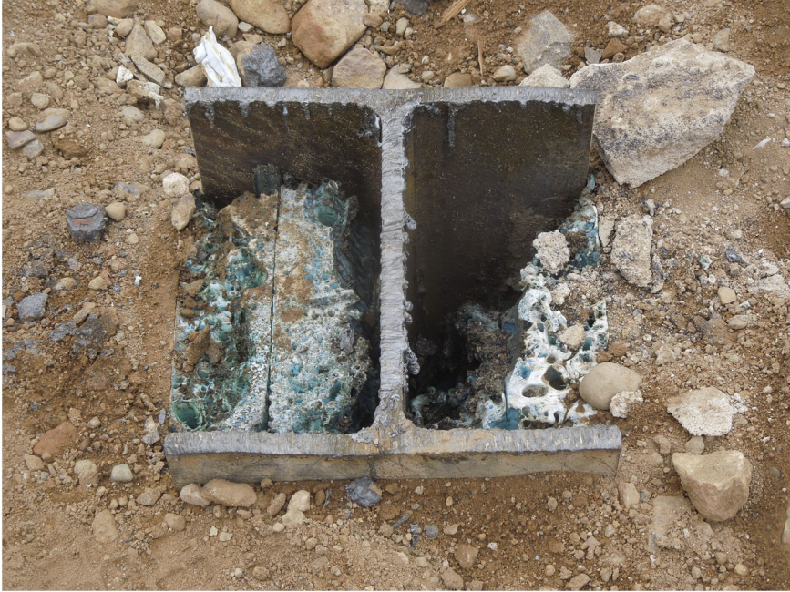
Plate 40.3 Steel H-pile installed.
