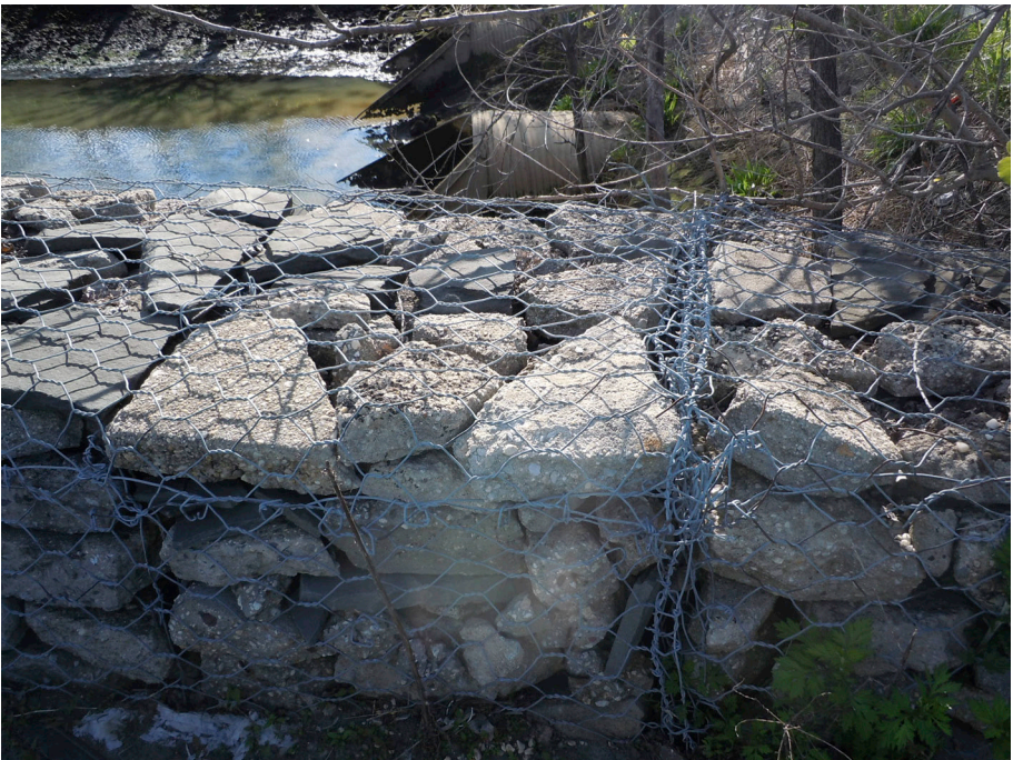
Plate 23.2 Gabion wall completed.
