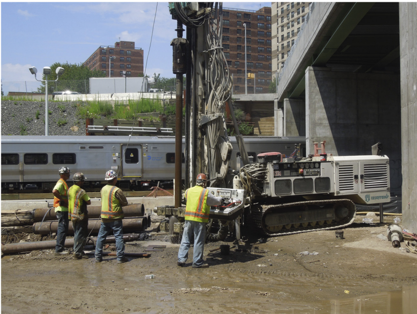
Plate 2.2 Mud rotary drill rig.
