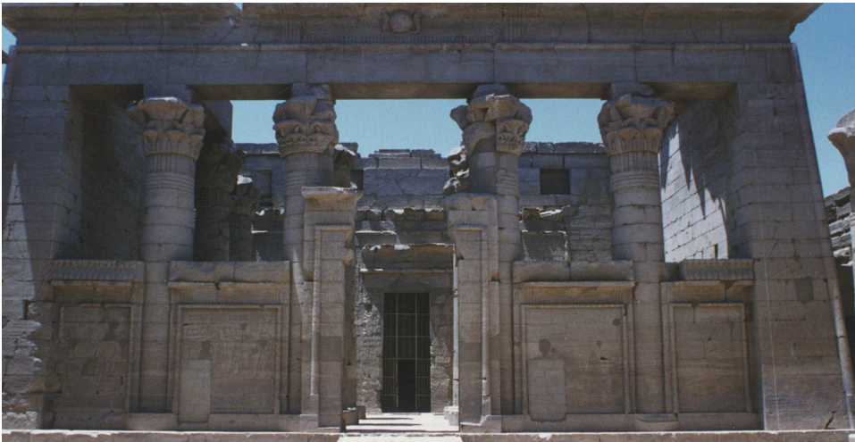
The pronaos , or anteroom, of the Temple of Kalabsha. The roof has collapsed, making it look light and airy. (John A. Shoup)
