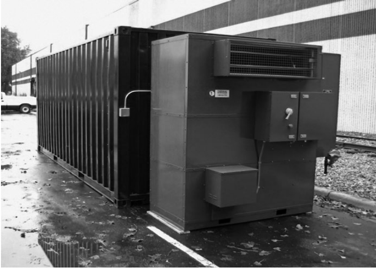
Figure 28.3 Shipping container fitted with a heater for larger containerized heat treatments. (Courtesy of J. Bruesch, Plunkett's Pest Control, Fridley, MN, USA).
