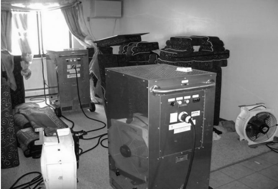
Figure 28.5 Whole-room heat treatment with electric furnaces. (Courtesy of Raj Hulasare, Temp-Air, Inc., Burnsville, MN, USA).
