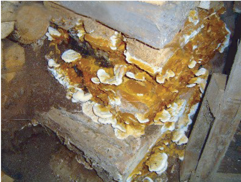
Figure 9.4 Serpula lacrymans – Dry rot spores © Lutz Weidner. Reproduced under the terms of the GNU Free Documentation License
