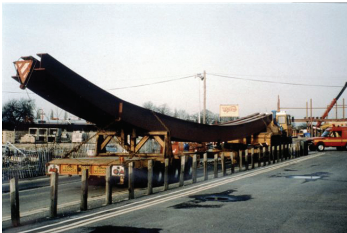
Figure 18.19 21+ m long roof beams
