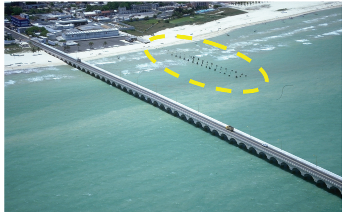
Figure 5.5(a) Aerial view of Progreso piers Original 1940s Progreso pier still in service, with the remnants of the 'modern' 1970s neighbouring pier shown ringed
