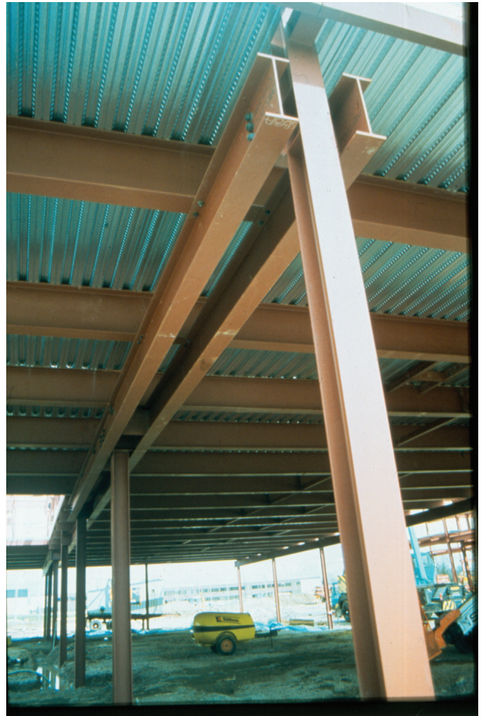
Figure 18.23 Sometimes the main framing members need only three serial sizes to be ordered in bulk by the steelwork contractor, assuming a ‘minimum weight/high complexity’ frame has been avoided
