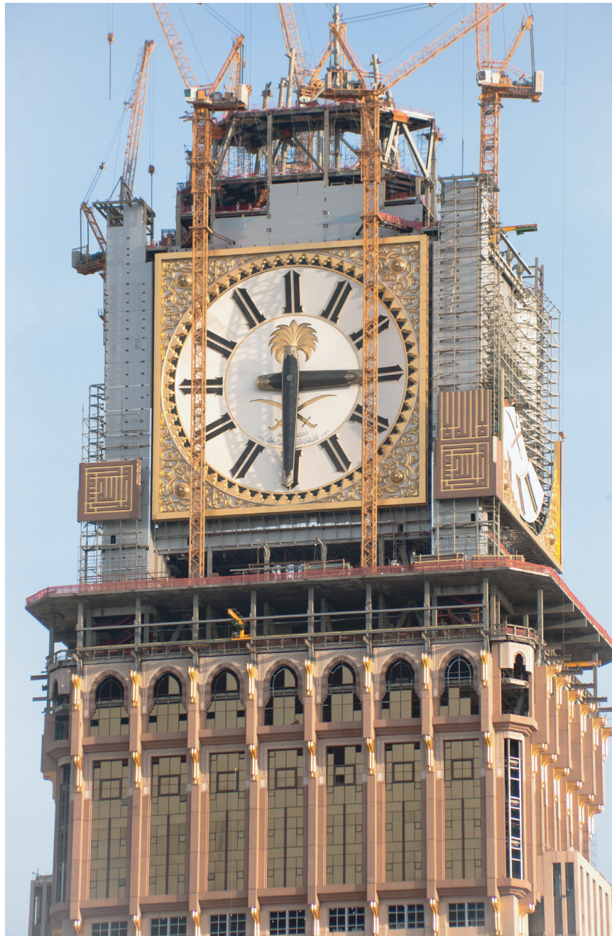
Figure 16.2 Dokaee Clock Tower, Mecca, KSA: carbon fibre clock faces under construction (Courtesy of Premier Composite Technologies)
