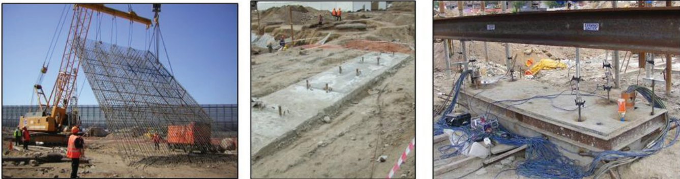
Figure 13.11 Full-scale load testing of barrette foundations
