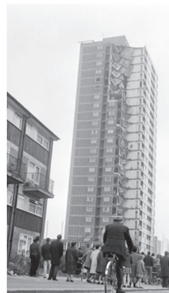
Figure 9.1 Progressive collapse, Ronan Point, 1968. All rights reserved
