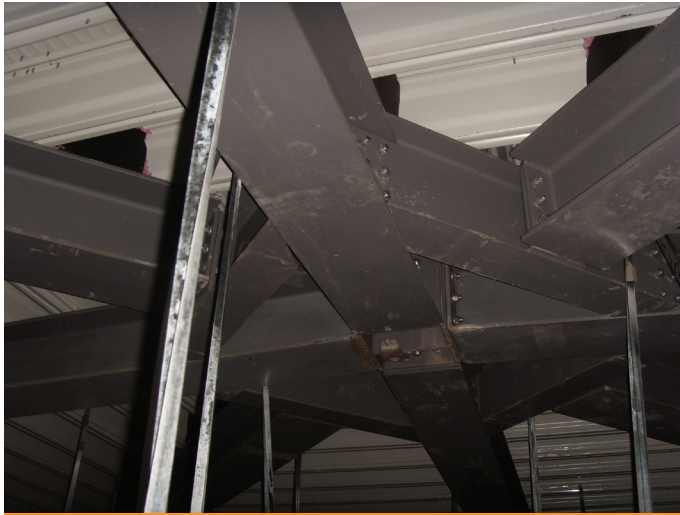
Figure 18.3 At concept stage, avoid multiple member junctions
