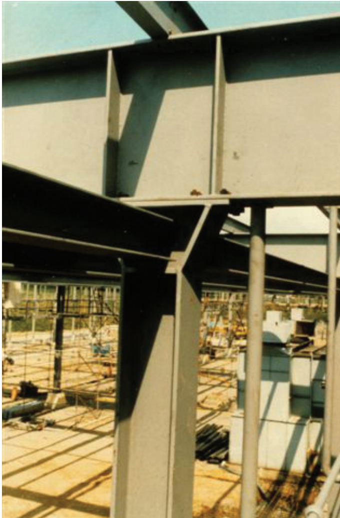
Figure 18.30 Aesthetic detailing, stiffeners set back, column head detail accommodates restraint tie in an industrial building
