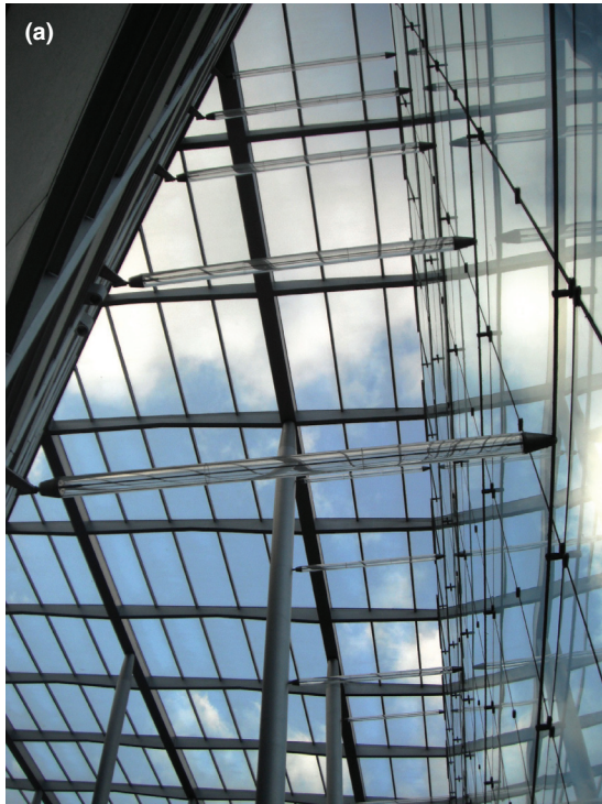
Figure 21.1 Glass struts: (a) glass circular hollow struts providing horizontal restraints to the facade at Tower Place, London; (b) vertical structural glass walls bearing the weight of the steel roof at the Rhenbach Pavilion, Germany
