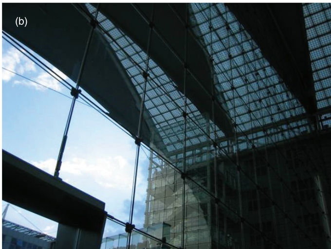
Figure 21.3 Glass plates: (a) frameless glass facade at the at Parc La Villette, Paris; (b) post-tensioned glass facade at Kempinski Hotel, Munich
