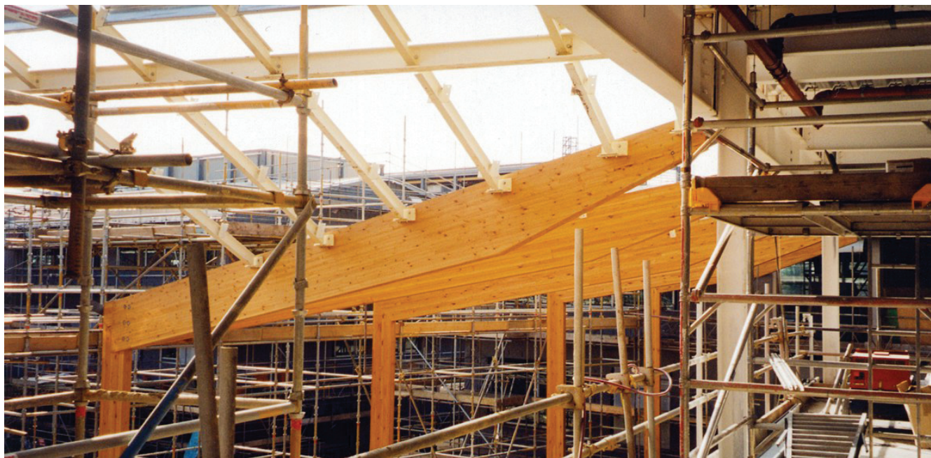
Figure 18.45 Hybrid structure in steel and timber
