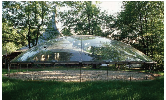
Figure 21.4 Prototype glass shell at the University of Stuttgart, Germany (image courtesy of Werner Sobek Engineers)
