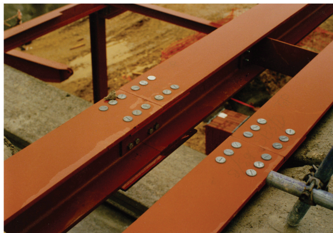
Figure 18.36 Slimfloor twin continuous beam and precast
