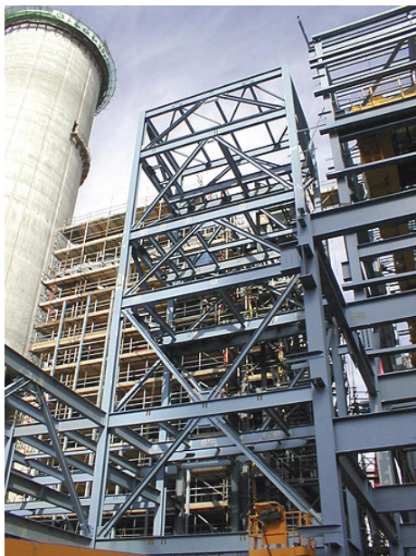
Figure 15.33 Power station steelwork, braced tower. Courtesy of Bourne Steel
