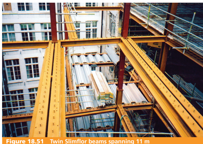
Figure 18.51 Twin Slimflor beams spanning 11 m
