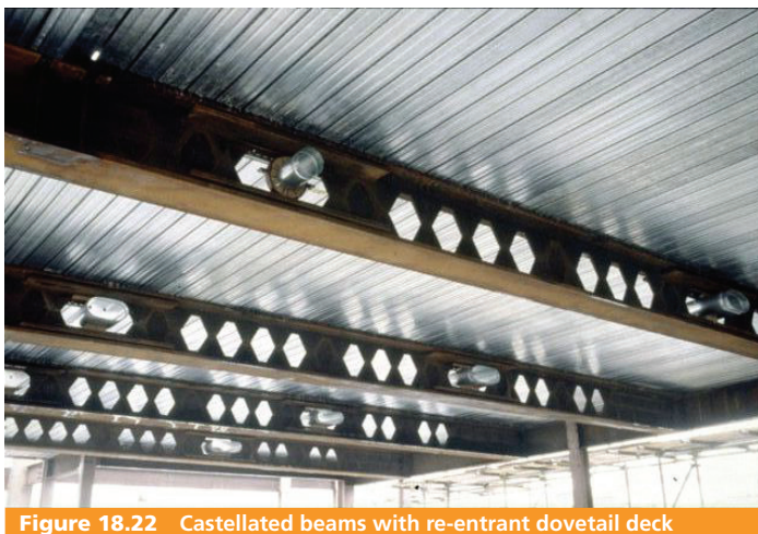
Figure 18.22 Castellated beams with re-entrant dovetail deck
