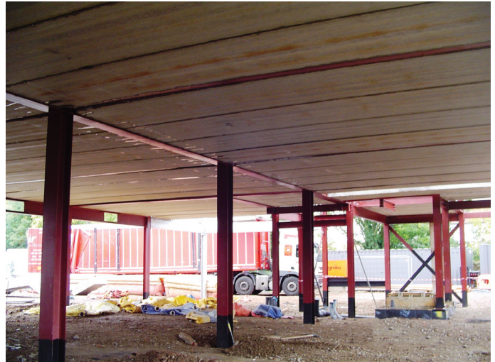
Figure 18.11 UC sections used with precast planks
