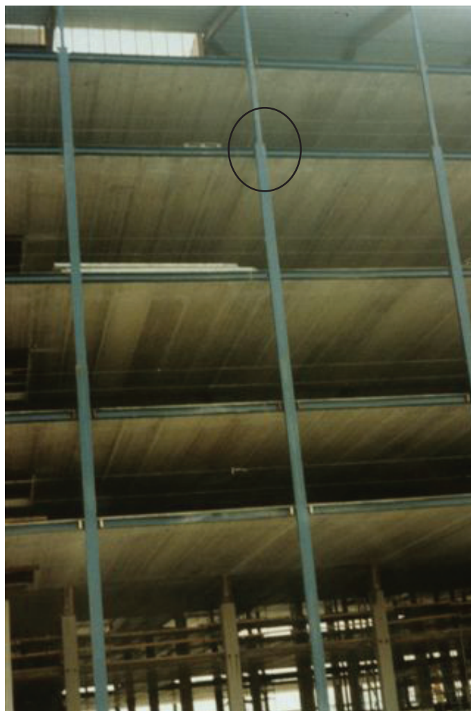
Figure 18.9 Elevation on perimeter column splice
