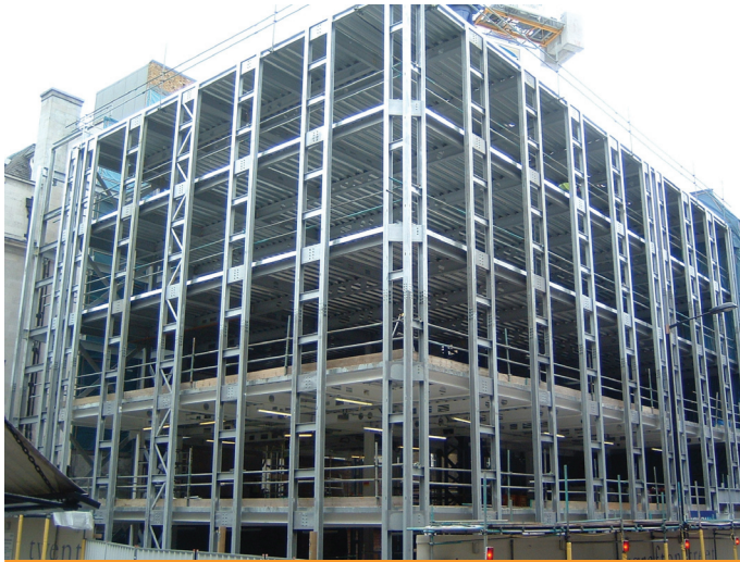
Figure 18.5 Elevation of twin perimeter columns set into the wall construction
