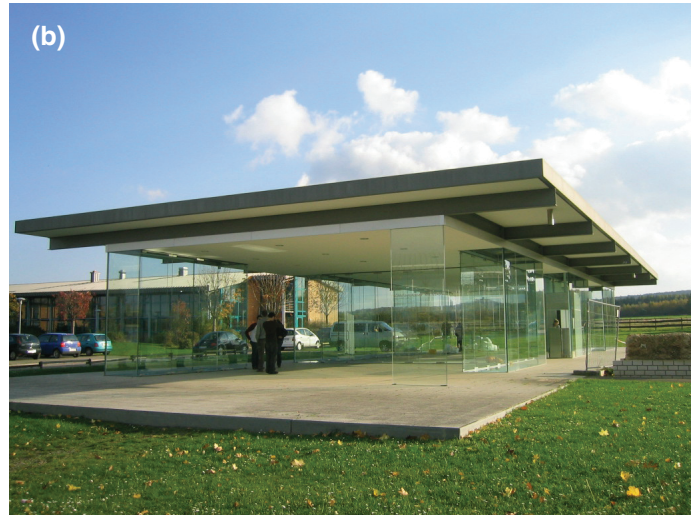
Figure 21.1 Glass struts: (a) glass circular hollow struts providing horizontal restraints to the facade at Tower Place, London; (b) vertical structural glass walls bearing the weight of the steel roof at the Rhenbach Pavilion, Germany
