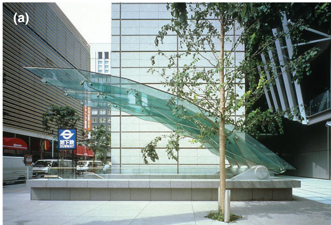
Figure 21.2 Glass beams: (a) cantilevered glass segmented beams in the Yurakucho canopy, Tokyo (image courtesy of Dewhurst Macfarlane Engineers); (b) simply supported glass threads in Apple Store spiral staircase, New York (image courtesy of Eckersley O'Callaghan Engineers)
