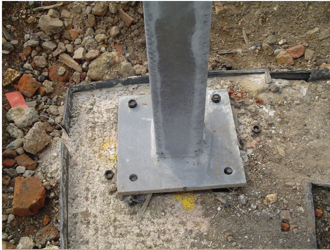
Figure 18.25 Substructure/steel interaction detailing without generous tolerance allowance leads to costly remedial work; avoid 'economising' on HD bolt length
