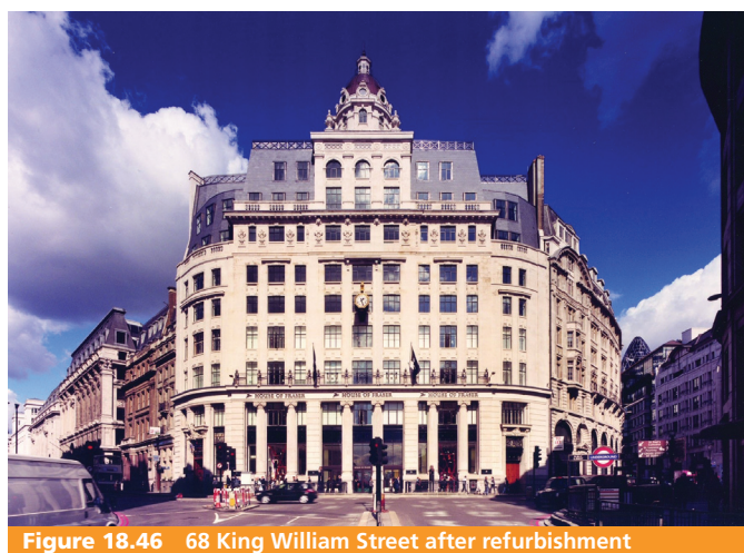
Figure 18.46 68 King William Street after refurbishment
