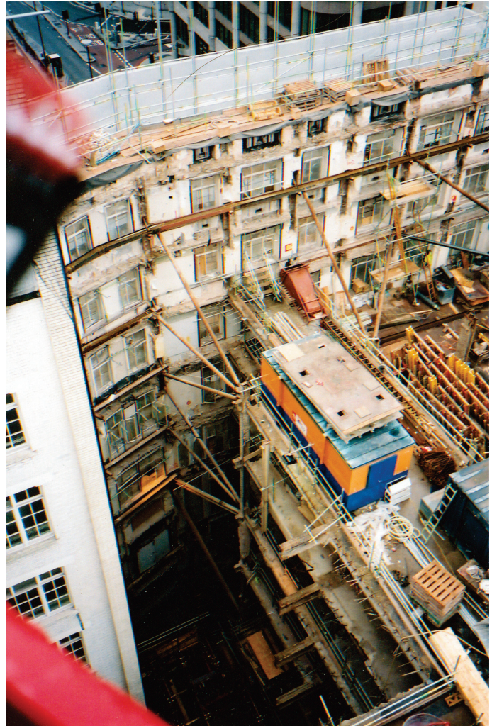
Figure 18.48 Temporary works for the retained facade
