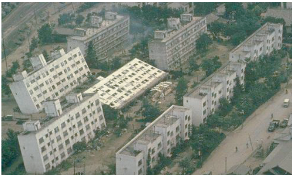
Figure 9.3 Liquefaction failure – Niigata earthquake, Japan 1964. Photograph in the public domain
