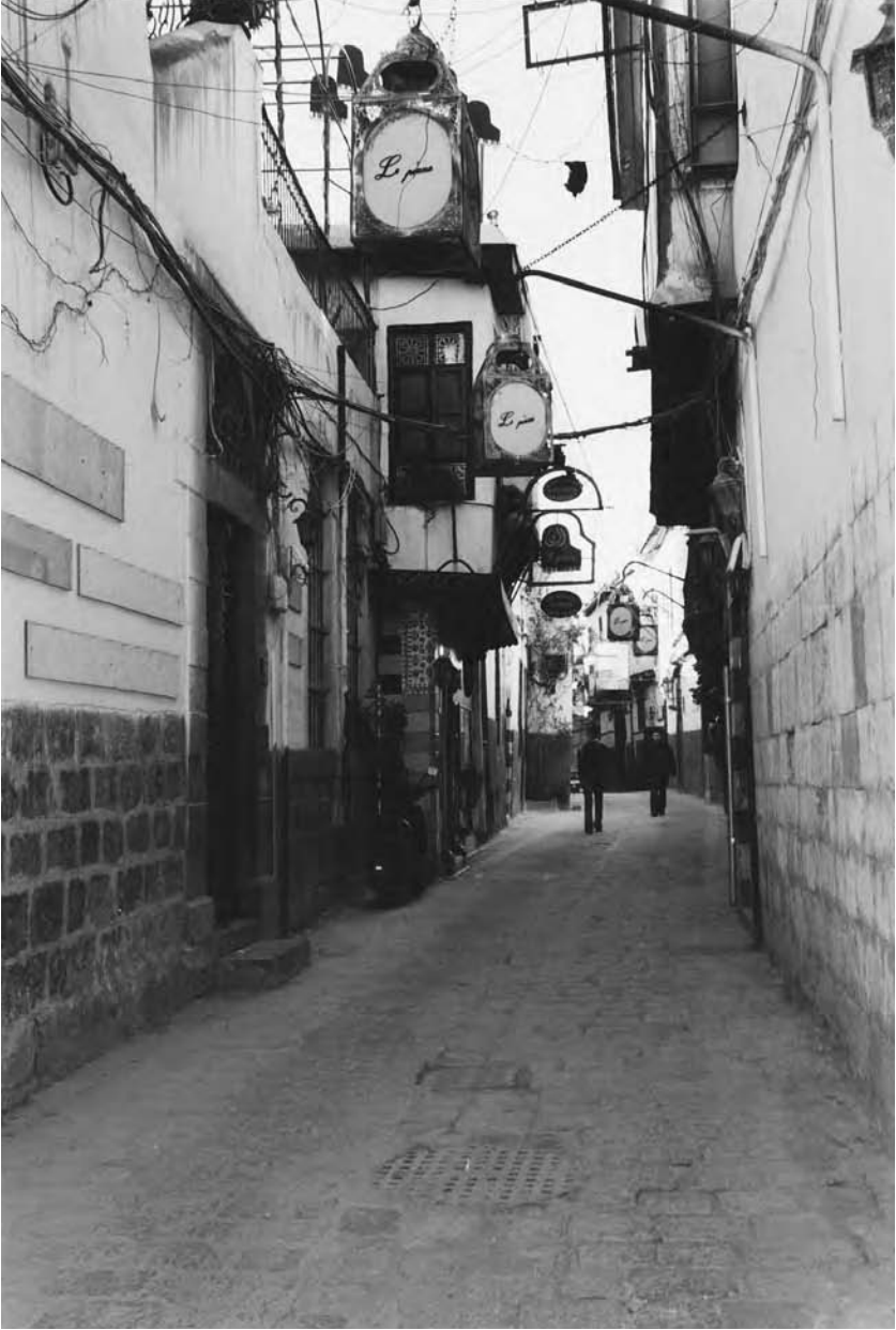
Le Piano Bar, exterior
