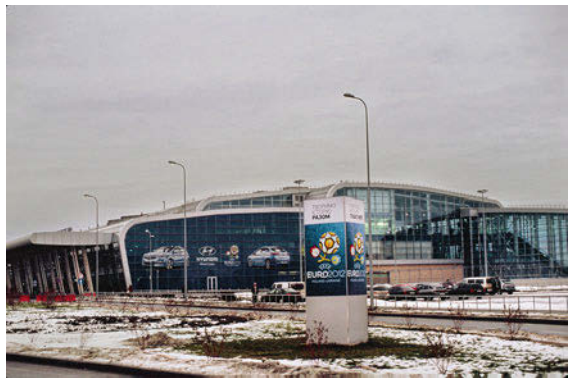
Photo 6.9 The national government makes decisions concerning Lviv’s airport. Thus, the municipality cannot decide on measures to attract, e.g., airline companies that could bring more tourists to the city
