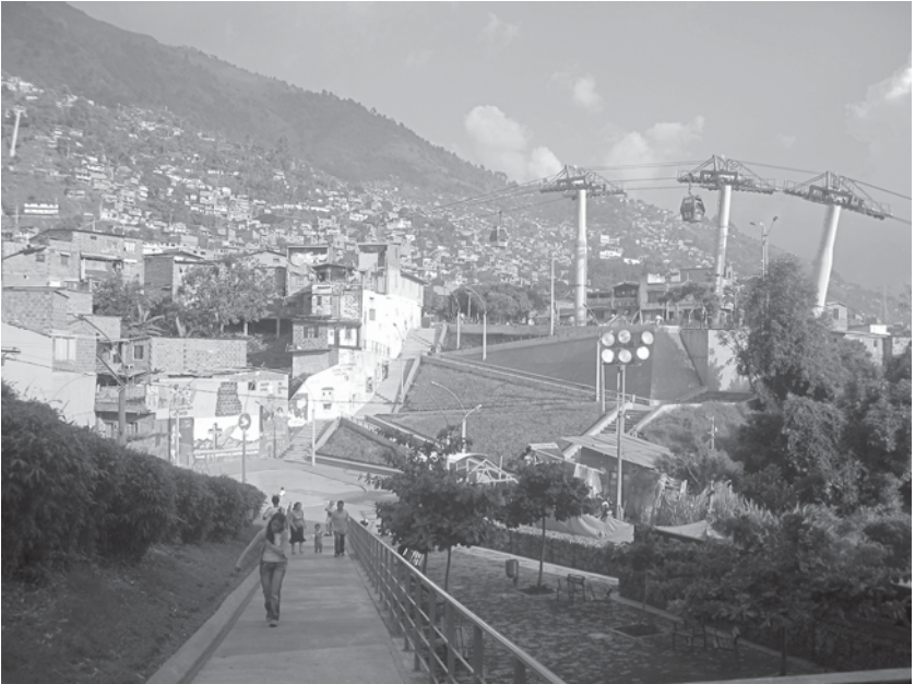
Figure 10.4. Zigzagging terraces and Metro-cable pillars, Barrio Santo Domingo, Medellín, Colombia. (Photo courtesy of David Gouverneur.)
