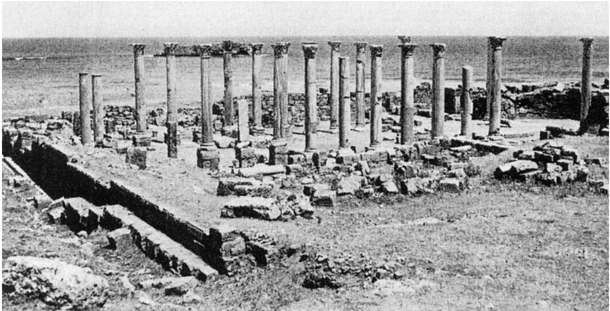
245. Apollonia East Church. View after anastylosis during the Italian Regime showing Monolithic Columns. Marsa Sousa. Cyrenaica. ca 450 AD. This church complex was constructed of (roughly) squared rubble masonry from local sandstone together with reused columns of Greek Island (Cipollino) Marble. The columns are all monoliths and demonstrate how monolithic marble columns ousted columns constructed of drums of local stone. This practice of importing pre-fabricated marble columns is particularly apparent in Cyrenaica, since most of the sites are on or near the coast, thus facilitating shipment and transport on site. Also the walling of rubble etc is abstracted for reuse over the ages, leaving broken column shafts as the residue of the building. After Christian Monuments of Cyrenaica , p.39, Ill 5.
