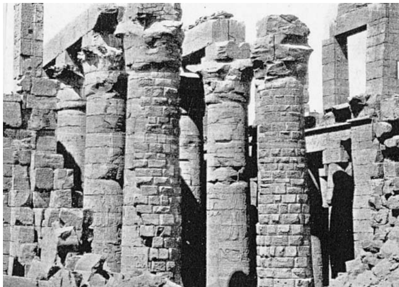
231. Karnak. Great Hall. Ancient Repairs to Columns effected in normal small block Masonry. Thebes New Kingdom or later. After Clarke and Engelbach, figs 166, 167.
