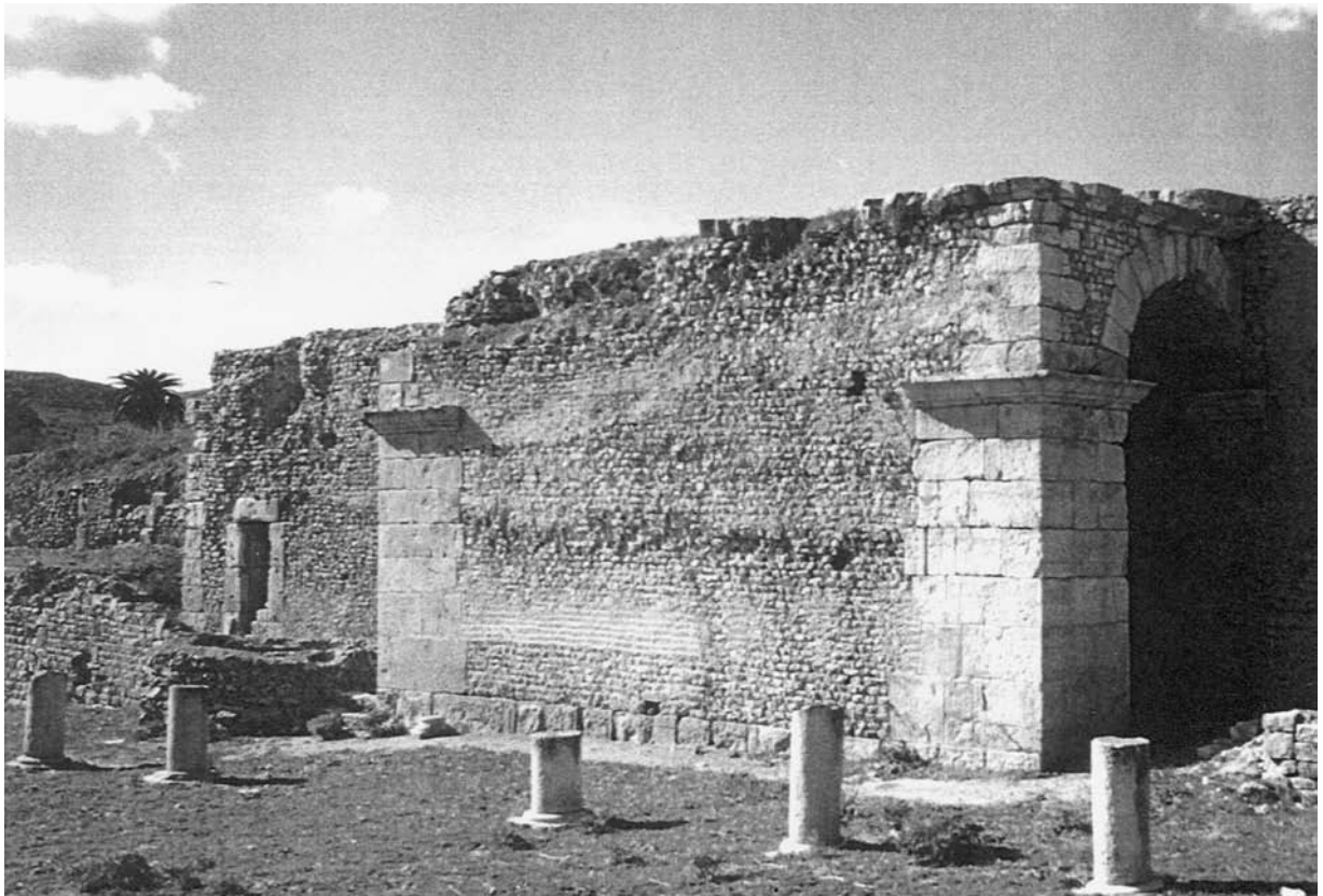
210. Bulla Regia. Temple of Isis. Mixed Ashlar and Rubble Construction. Tunisia, Roman ca 200 AD. Masonry of coursed rubble stiffened by ashlar coigning and framing. This is a more solid and substantial expression of the mode than the previous example.
