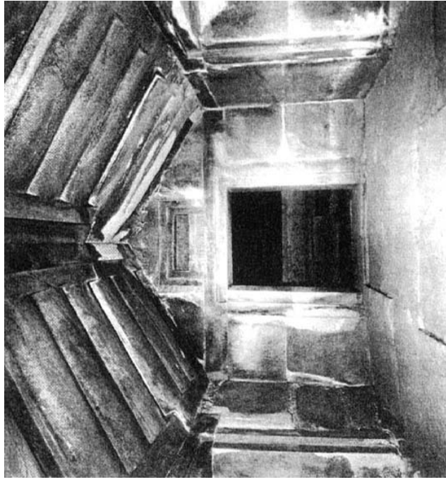
265. Tamassos Royal Tomb. View from Antechamber into Burial Chamber. Cyprus 650 BC – 600 BC. This view shows the triangular vaulted stone roof with soffite carved to represent timber construction.
