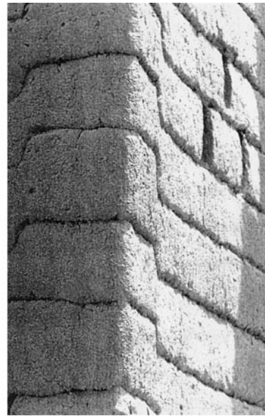
327. Typical Puddled Mud (Zubur) Construction. North Yemen. 20th Century AD. These traditional tower houses (left) in the desert region of North Yemen are massive and strongly built for reasons both of security and of heat insulation. The average height is ca 10-12 m fashioned in horizontal registers of plastic earth of ca 50 cms height. These horizontal layers are built up at the angles in the semblance of decorative horns (right). This is a functional device to put the layers of earth in compression so as to counteract the tendency of such material to fissure and collapse at the angles. The entire construction is carried out by hand with lumps of plastic earth and requires no installations or tradesman's tools. After G.R.H. Wright ABADY 4 1988 pl. 42.
