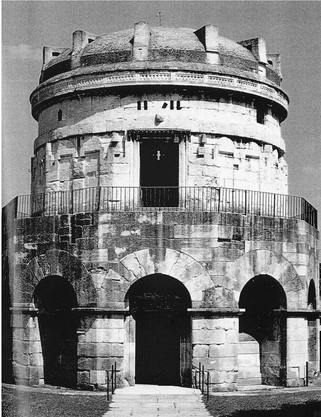
301. The Mausoleum of Theodoric the Ostrogoth with a Monolithic Capstone Roofing. Ravenna ca 520 AD. The domed roof is a monolith ca 11m in diameter, with a rise of ca 3m, weighing 300 tons and more, fashioned to simulate the form of a (saucer) dome. It was perhaps levered up to the required height and propped in position so that the underlying masonry structure could be built up beneath it.
