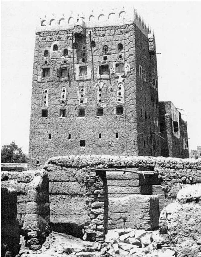
326. Saada. Traditional Modern Puddled Mud (tauf) Construction. North Yemen. 20th Century AD. This typical building in the desert regions of Northern Yemen shows a strong tower house of 4-5 floors entirely of plastic mud construction identical with that of garden walls and sheds in the lower foreground. The building procedure requires no installations or equipment of any description. After G.R.H. Wright ABADY 4 1988 pl. 44a.
