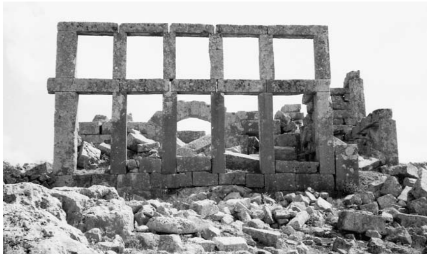
216. Dehès. Ashlar Stone Framed Wall Construction. North Syria. ca 500 AD. After 1500 years the massive blocks of the frame (ca 2m in length and of 1 ton burden) remain standing in situ on their rocky outcrop foundations, while the panelling of the ashlar blocks and slabs has collapsed and/or been robbed out. The surviving disposition of some buildings gave investigators the impression that these constructions were originally open porticos with at most a low balustrade between the piers. However, from examples like this, it is visually evident that the construction is the surviving skeleton of a stone framed wall – which is demonstrated by the traces remaining on the stone framing of the engagement of the panelling. Photo J-L Biscop.
