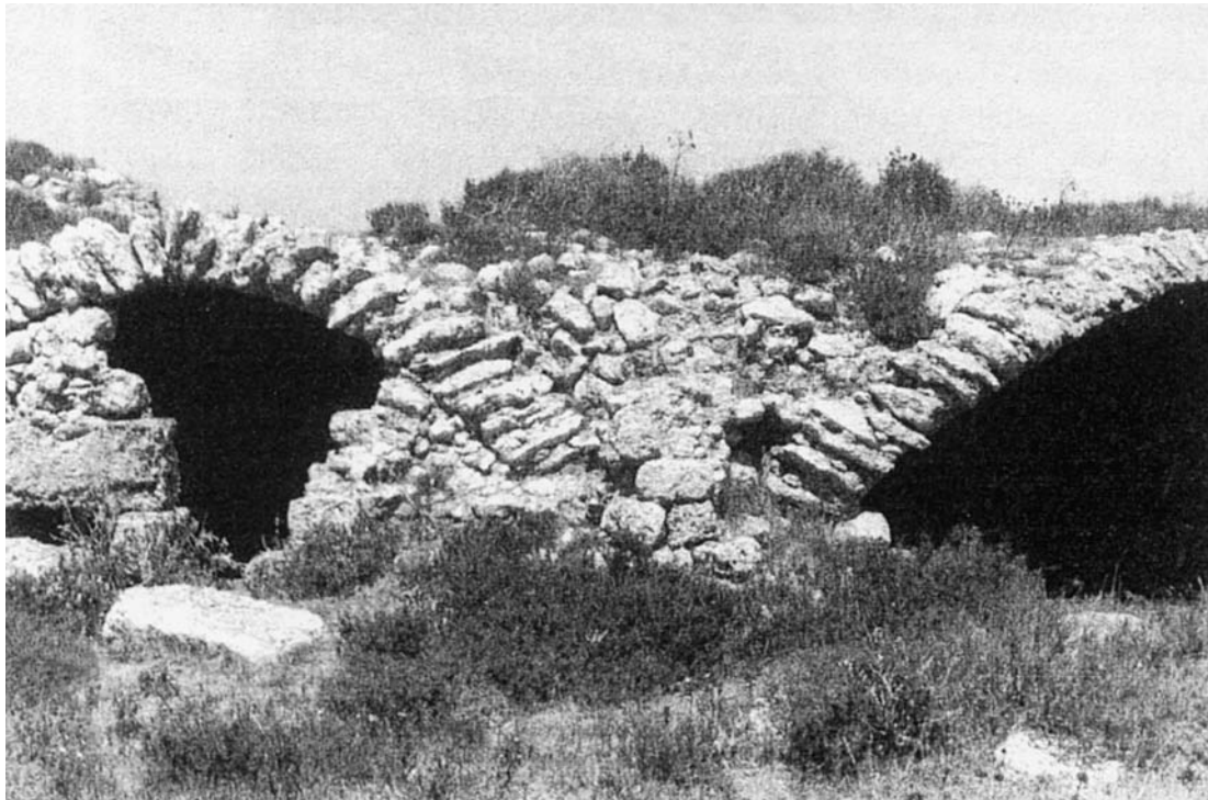
276. Siret el Reheim. Barrel Vaulted Cisterns of Rubble Masonry Construction. Cyrenaica. ca Early 6th Century AD. A pair of vaulted cisterns set against the enclosure wall of a church, probably from the time of Justinian are of utilitarian construction. The barrel vaulting of depressed parabolic contour is constructed of long flat field stones set radially in strong mortar. Cisterns of similar construction occur elsewhere in the region. After Christian Monuments of Cyrenaica, p. 359, ill 303.
