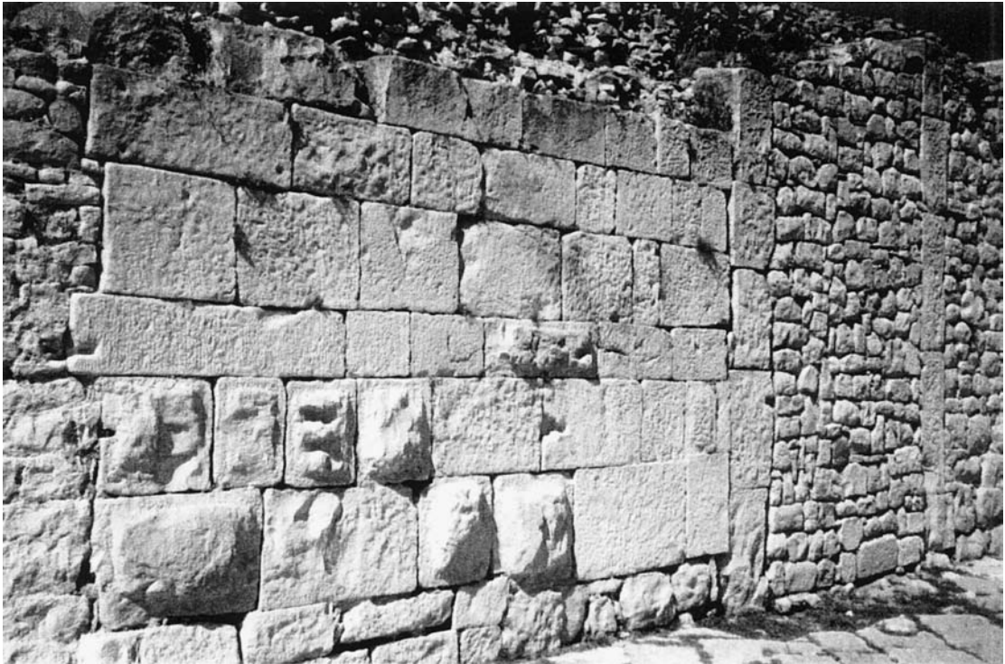
211. Ain Doura Baths. Mixed Ashlar and Rubble Masonry ( opus africanum ). Tunisia, Roman. Opus Africanum , rubble stiffened by pillars of dressed stone was the masonry heritage of Punic North Africa from original Phoenecian antecedents. It survived in the North African provinces throughout Roman rule and into Byzantine times. Not infrequently it was used together with opus quadratum .
