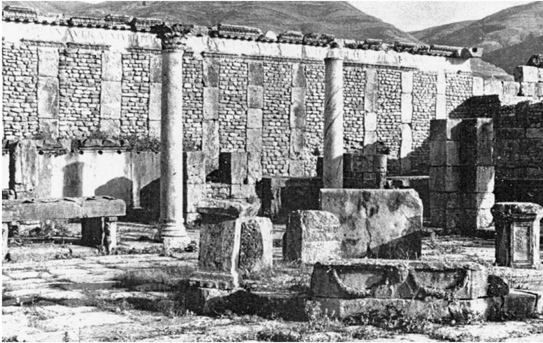
213. Cuicul. Market of Cosinius. Opus Africanum . Fully Framed Construction. Jemila, Algeria, ca 150 AD. This type of masonry appears the logical fulfilment of opus africanum and bestrides it and stone baulk framed construction familiar from Les Villes Mortes of Northern Syria. After Ward Perkins. Pl 241.
