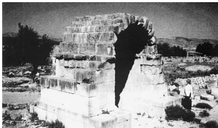
270. Ain Thunga. Ruins of Small Triumphal Arch exposing Ashlar Vaulting of Passageway. Tunisia. ca 2nd Century AD. The construction of ashlar barrel vaulting in the classical world remained unchanged from its first appearance during the later 4th Century BC in the Macedonian Vaulted Tombs. It was highly functional for roofing passageways, corridors, etc; but it was virtually never exposed to external view – cf the unusual appearance of the ruins of this small Triumphal Arch where the structure of the ashlar vaulting is now exposed.
