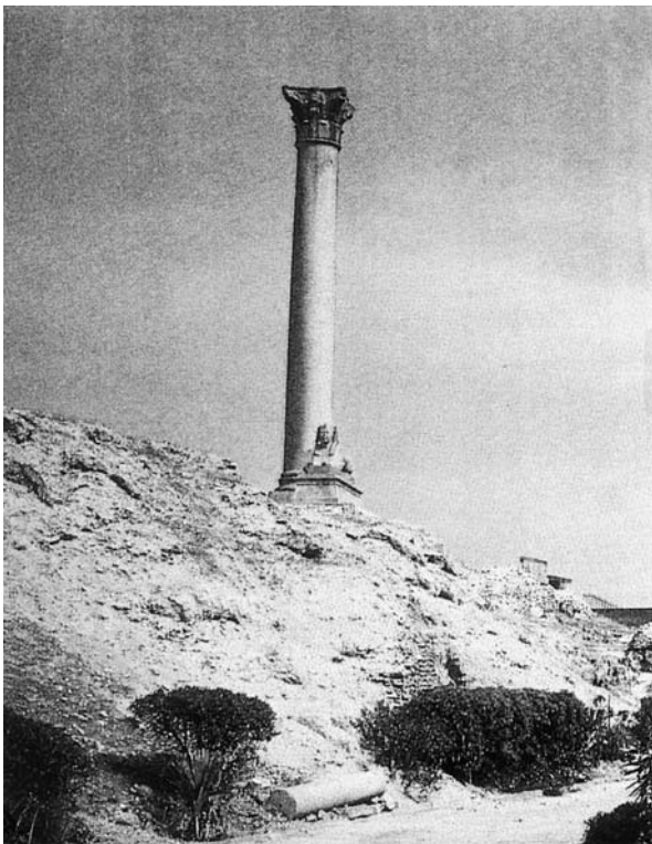
244. Alexandria. The Monolithic Victory Column of Diocletion alias Pompey's Pillar. Egypt 298 AD. It is interesting to note that once more after 2000 years massive monumental columns in Egypt were monoliths not built up in drums. This perhaps bespeaks the fact that the absolute rule of the Roman Emperor as Egyptian Pharaoh was comparable to the absolute status of the Old Kingdom Pharaohs. After G. Hölbl I, p. 39, abb 32.
