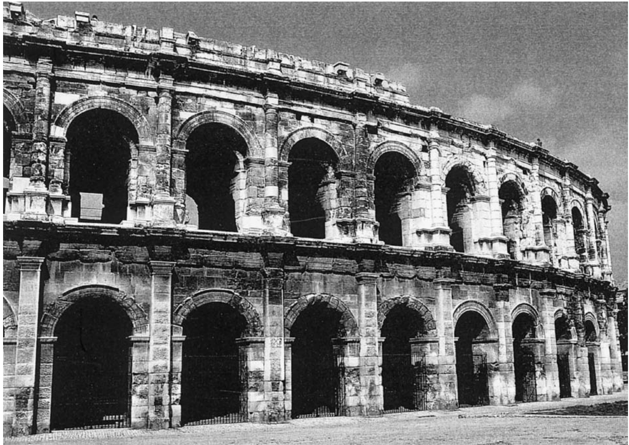
206. Nîmes. The Amphitheatre (Les Arènes). Opus quadratum Façade. Provence. Later 1st Century AD. The masonry is entirely of large ashlar blocks set dry stone.
