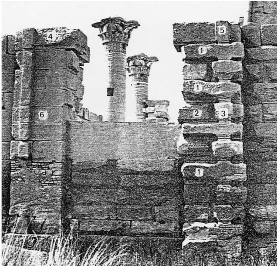
169. Medinet Habu. The Small Temple. View of Screen Wall featuring an Entrance with ornamental mouldings. Thebes. Roman Period. The unfinished state of the dressing indicates that the fine dressing of the masonry including the working of the mouldings was carried out in situ and proceeded directionally from left to right. The left jamb of the portal was finely dressed while the blocks comprising the right jamb were largely in bossed form, with only the initial stages of in situ dressing under way to work the vertical strip (torus) moulding. Key: (1) Blocks as set in bossed form with only marginal draughts worked prior to setting; (2) Face of blocks partly dressed back to delimit roughly the vertical strip moulding (torus / Rundstab ); (3) Preparatory draught of vertical moulding; (4) Fine dressing of face of jamb in progress; (5) Finely dressed grounds for vertical strip moulding to be later worked into a torus ( Rundstab ); (6) Fair faced masonry of jambs. After Golvin & Laronde ASAE 68 1982 pp 165-194, Pl VII.
