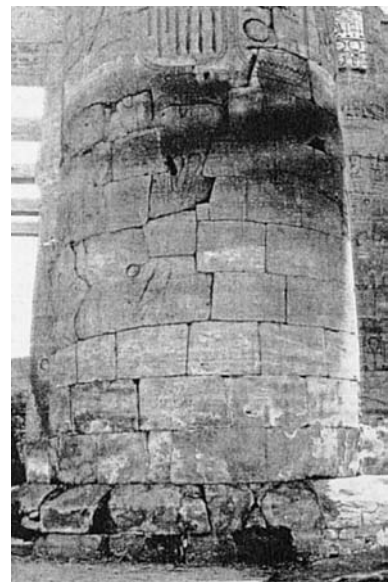
231. Karnak. Great Hall. Ancient Repairs to Columns effected in normal small block Masonry. Thebes New Kingdom or later. After Clarke and Engelbach, figs 166, 167.
