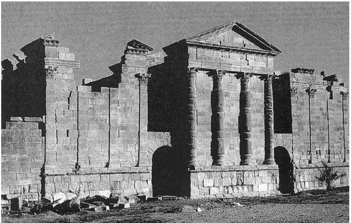
204. Sufetula. Temples of Capitoline Triad. Typical Roman opus quadratum masonry. Sbeitla, Southern Tunisia. 2nd Century AD. It is a characteristic of the aspect of Roman ashlar masonry ( opus quadratum ) that the blocks are of compact, squarish form rather than the elongated format of Greek ashlar blocks.
