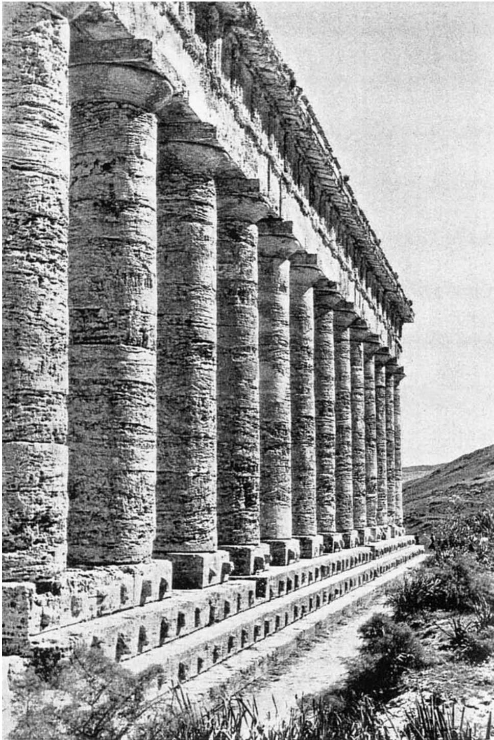
234. Temple of Segesta. Unfinished Column Construction showing unfluted Drums. Sicily. Late 5th Century BC. Work on this large temple was abandoned after the erection of the peristasis. This clearly demonstrates that the normal procedure for fluting columns was to carry out the work in situ after erection. These sizeable columns are each built up out of ca 12 drums, and narrow registers at the base of the lower drum and at the crown of the uppermost drum have been dressed back to the final dimension as a guide to the work of fluting. After Lawrence, pl 84.
