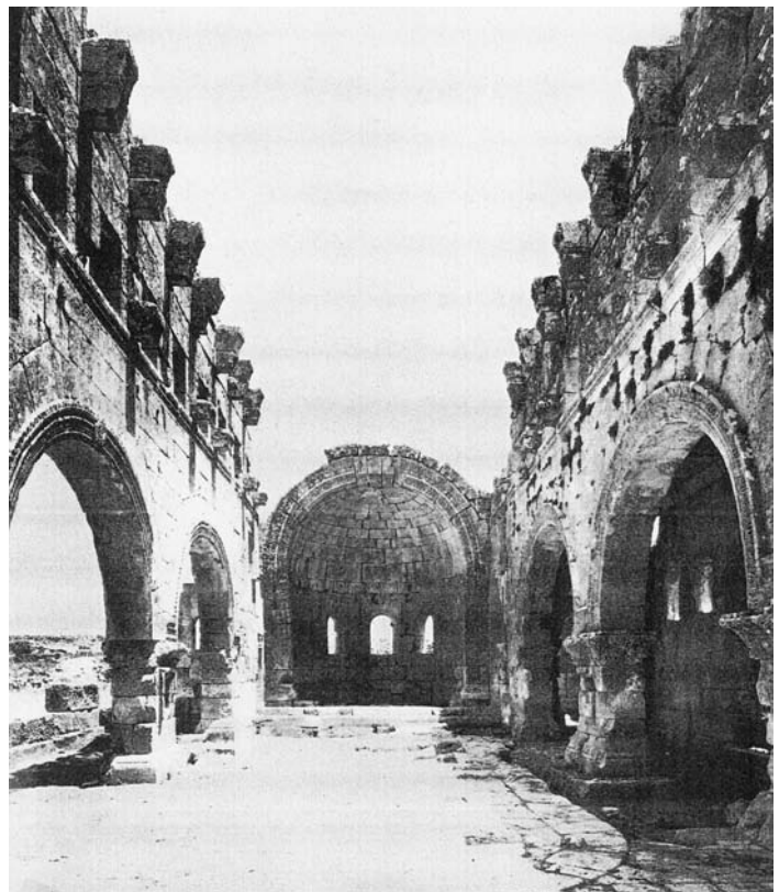
245. Apollonia East Church. View after anastylosis during the Italian Regime showing Monolithic Columns. Marsa Sousa. Cyrenaica. ca 450 AD. This church complex was constructed of (roughly) squared rubble masonry from local sandstone together with reused columns of Greek Island (Cipollino) Marble. The columns are all monoliths and demonstrate how monolithic marble columns ousted columns constructed of drums of local stone. This practice of importing pre-fabricated marble columns is particularly apparent in Cyrenaica, since most of the sites are on or near the coast, thus facilitating shipment and transport on site. Also the walling of rubble etc is abstracted for reuse over the ages, leaving broken column shafts as the residue of the building. After Christian Monuments of Cyrenaica , p.39, Ill 5.
