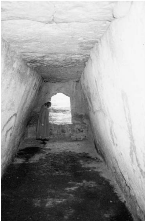
303. Grotte de la Source. Rock Cut Gallery Grave. Interior view looking out and in. Near Arles, ca 3000 BC. The gallery is cut down into bed rock with smoothly dressed walls splaying apart below. The roofing is constructed of deep and massive slabs spanning the excavation.
