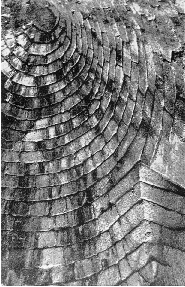
286. Mycenae. Treasury of Atreus. Tholos Tomb. Interior View showing finely dressed masonry of Bastard Ashlar type. Greece. ca 1300 BC. This masonry is interior facing to earth matrix, and the jointing is less exact behind the exposed face. The development in finely dressed monumental masonry over ca 150 years from the tholos tombs at Epano and Kato Phournos is striking. After Lawrence, pl 11.
