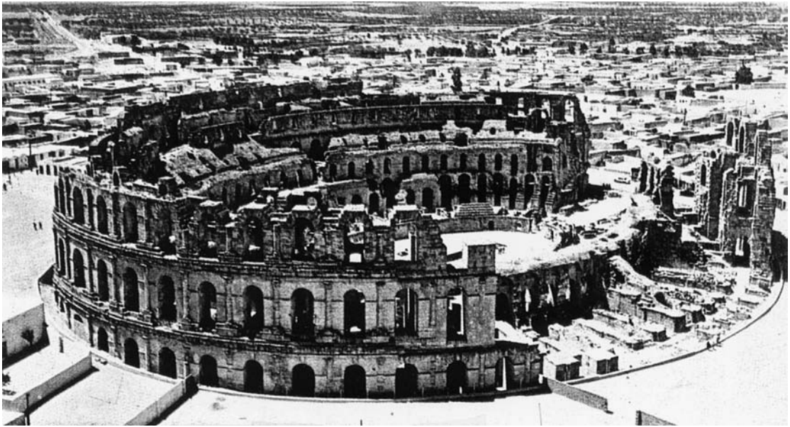
272. Thysdrus. Amphitheâtre. Aerial Photograph of large scale Vaulted Construction. El Jem, Tunisia. ca 240 AD. This large amphitheatre modelled on the Colosseum was unfinished, which together with its present state of ruin exposes to view the pervasive incidence of barrel vaulting in its structure. The circulation both horizontal and vertical was effected by barrel vaulted passages. This vaulting could be constructed in ashlar masonry, rubble masonry or Roman Concrete.
