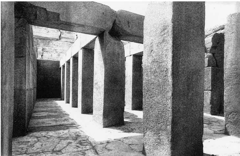
160. Gizeh. The Valley Temple of Khafra (Khephren). Lower Egypt. ca 2500 BC. Aerial view and masonry detail of pillared hall. The simplicity and majesty of this massive stone masonry produced an awesome effect. The pillars are ca 5 m high. The stone is Rose Red Granite and the Temple is sometimes known as the Granite Temple. The pillars and beams were dressed true with hand stone tools (dolerite pounders) and their faces polished. As opposed to coursed masonry blocks, the finished dressing of these items was carried out prior to setting – perhaps at the quarry. After Stadelman Pl 51.
