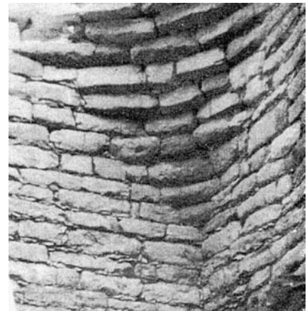
289. Mycenae. Treasury of Atreus. Santillo's Analysis of Mycenaean Tholos Construction. The heavy arrowing indicates the proposed static analysis of the structure. The gist of it is to avoid the stigma of a corbelled dome construction being any less a true dome than one with voussoirs set radially in the vertical sense. The limiting case is taken that each course of dome masonry, because of the lateral compression, behaves as a rigid unit resisting all tensile stresses, and transmitting all compressive stress from the superincumbent masonry vertically downwards – i.e. the construction is to be imagined as a succession of annular elements (e.g. metal rings) of decreasing radius placed one above the other (obviously a stable assemblage). Key: 1. Excavated Terrain; 2. Earth debris and fill; 3. Finely dressed closely jointed ashlar masonry; 4. Bastard ashlar facing to earth fill with splayed rising joints; 5. Masonry at crown of tholos set as radial voussoirs; 6. Megalithic lintel; 7. Relieving triangle; 8. Relieving arch; (a) Wooden strutting. Flying shoring across entrance gap to maintain tholos masonry in lateral compression. (Further secured against displacement by dead weight of Megalithic lintel.); (b) Wooden Scaffold device to give centre of 'Beehive' tholos masonry; (c) Nail for attaching cord to give radii of successive courses; (d) Cords to control positioning of masonry. After Op Ath XV 1984, p. 47, fig 1.
