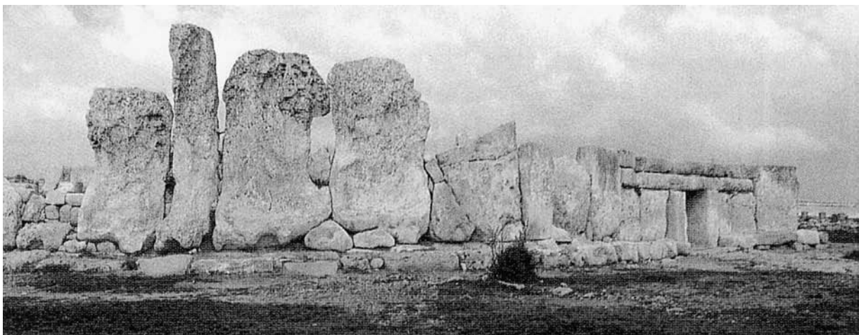
155. Mnajdra. Flank View of Neolithic Temple. Malta ca 3500 BC. This view demonstrates that the Maltese Temples belong to the Megalithic Tradition (v the rude slabs in the foreground), yet incorporate considerable dressed masonry (v façade blocks to right).
