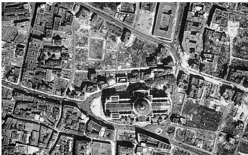
Figure 9.3 War damage around St Paul's, London
