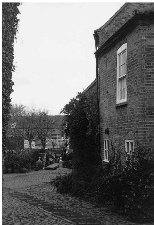
Figure 9.53 Access to the canal, Millgate
