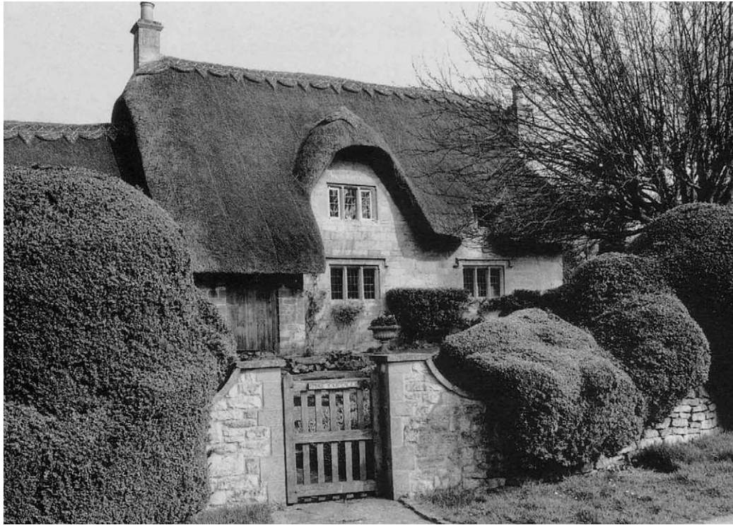
Figure 3.7 Cottage, Chipping Campden
