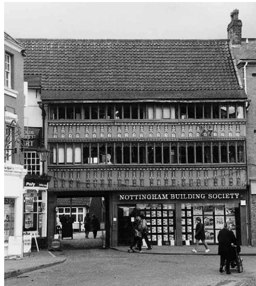
Figure 9.49 Rehabilitation, Market Square, Newark
