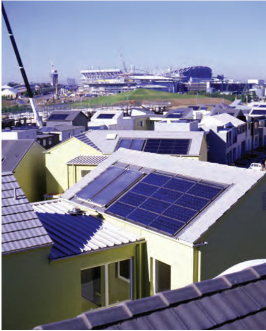
Typical PV roof system with the Sydney Olympic Stadium in the background
