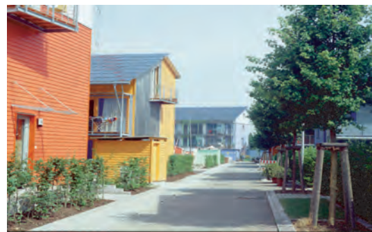
View of the Schlierberg Solar Estate from south
