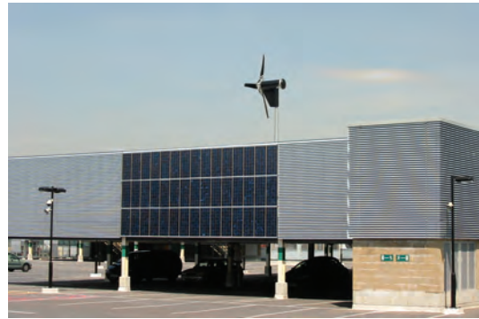
View of the Croydon Centrale shopping centre with newly installed solar cladding
