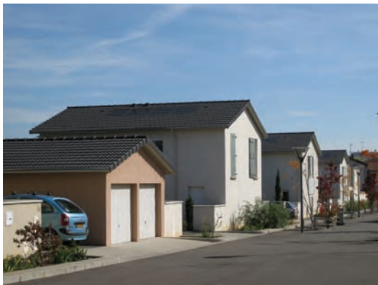
France-Terre detached houses each equipped with 1kWp integrated PV system
