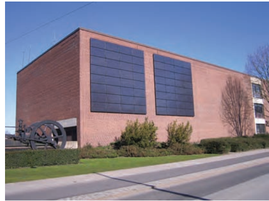
PV façade of the Museum of Science and Technology
