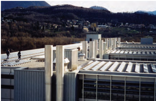
Roof outline of the UBS bank in Suglio (Switzerland). The detachable PV console modules form a total concept with the 'high-tech' image of the roof outline
