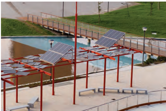
PV shelter used to provide shade in public spaces
