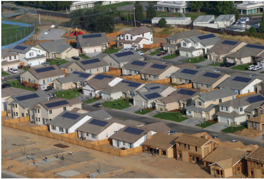
Group of PV systems installed in a new urban development
