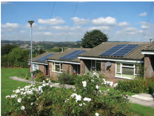
Fernside solar village housing
