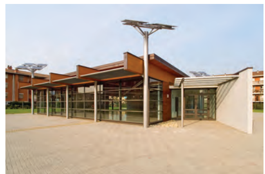
The social centre equipped with PV
