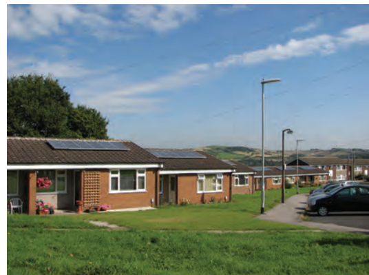
PV on housing association properties in Fernside
