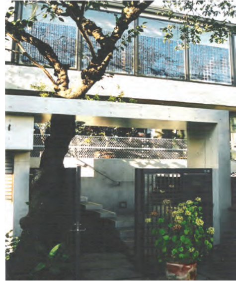
J-House, Tokyo, Japan. Natural integration of the PV system in the building. Architect: Jiro Ohno, Tokyo, Japan
