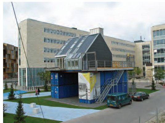
CO 2 neutral rooftop apartment with PV developed for the city of Copenhagen
