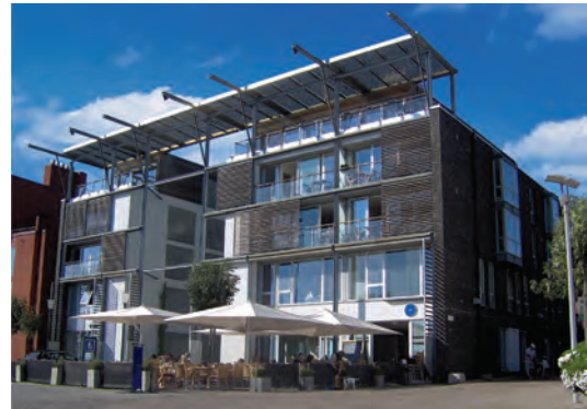
PV shading device integrated into the building design
