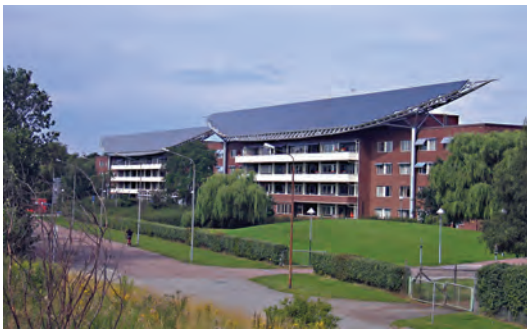
The Sege Park PV system
