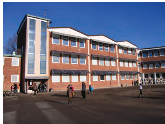
PV shading devices on the façade of the Mellanhed School in Malmö
