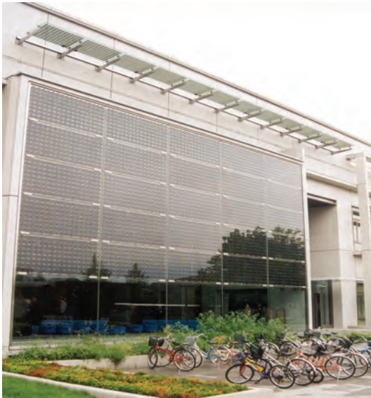
Tsukuba Open Space Laboratory, Tokyo, Japan. PV has replaced the conventional glass façade. Architect: Jiro Ohno, Tokyo, Japan
