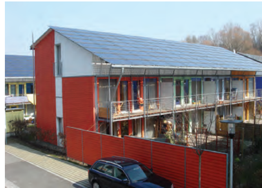
Single-family houses in Freiburg, Germany. PV adds to the architectural image of these ‘Plus-Energie’ Passive Houses
