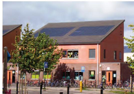
School houses with PV modules each replacing four standard roofing tiles
