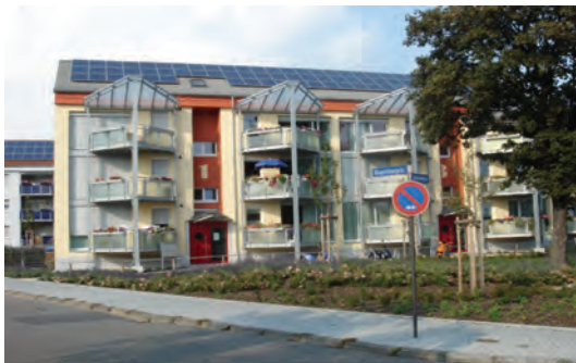
Renovated apartment buildings, Ludwigshafen, Germany. PV is added to the design, thus strengthening the architectural appearance
