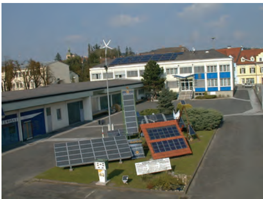
10.4kW p PV power plant on the roof of the utility Feistritzwerke-Steweag GmbH
