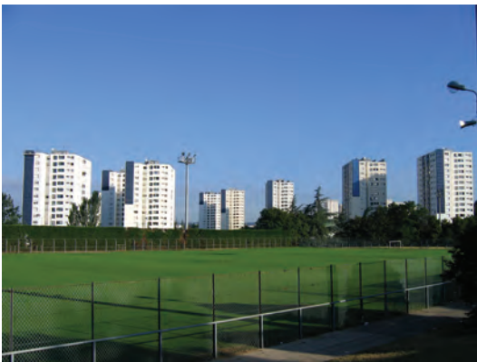
View of the southern façades of La Darnaise district early in the morning
