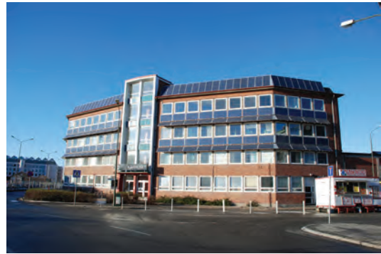
PV shading devices on the façade of the Student Union House in Malmö
