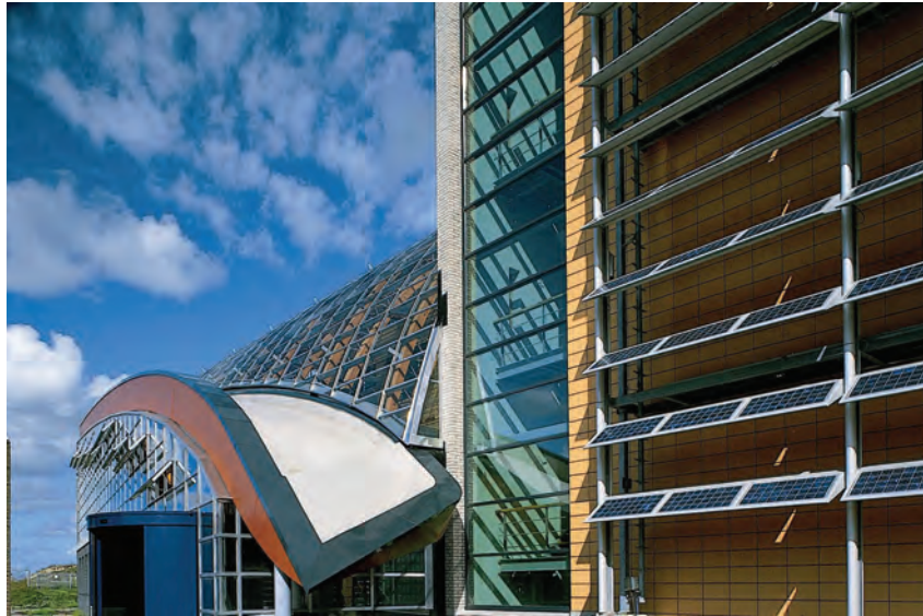
ECN building 42 and 31, The Netherlands. PV has led to an innovative building design. Architect T. H. Reijenga, BEAR Architecten
