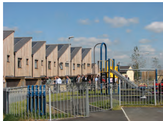
PV on new housing at Primrose Hill
