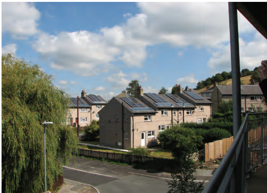
PV and solar thermal retrofit to houses in Primrose Hill
