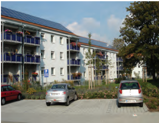
Renovated apartment buildings, with roof-integrated PV, Ludwigshafen, Germany
