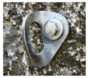
*<sup>3</sup>/<sub>8</sub>-inch stainless steel Powers bolt with stainless steel Petzl hanger, painted to match the rock color.*
