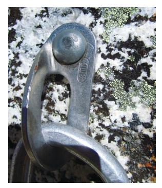
5/16-inch buttonhead Rawl contraction bolt with "good" SMC hanger. In a good placement in solid granite, these bolts are rated at over 4,000 pounds shear strength.
