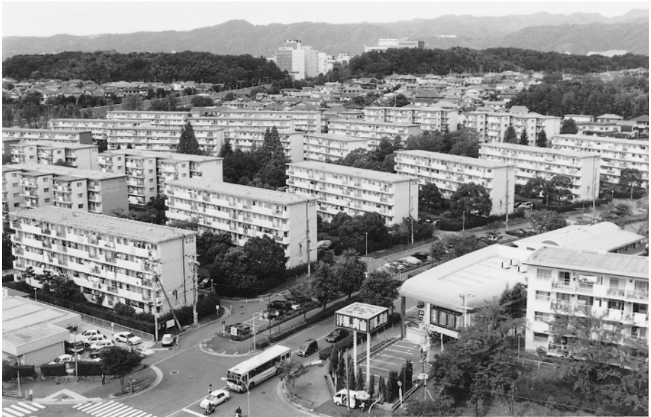
Figure 5.10 Senri New Town housing. These five-storey walk-up apartment blocks in Senri New Town north of Osaka are typical of the economical public housing of the 1960s and 70s. This area in Senri is adjacent to the main rail station, allowing easy access to central Osaka. Single-family houses are located further from the station on the hills in the background.
