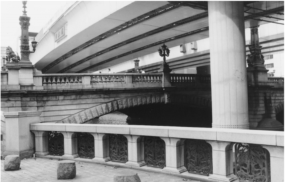
Figure 5.14 Nihonbashi and the metropolitan expressway. Tokyo's noble Nihonbashi, a beautiful historic structure and the symbolic heart of Japan from which all distances throughout the archipelago are measured, buried beneath the elevated metropolitan expressway is expressive of the values of the rapid growth period (see Figure 3.2, page 97).
