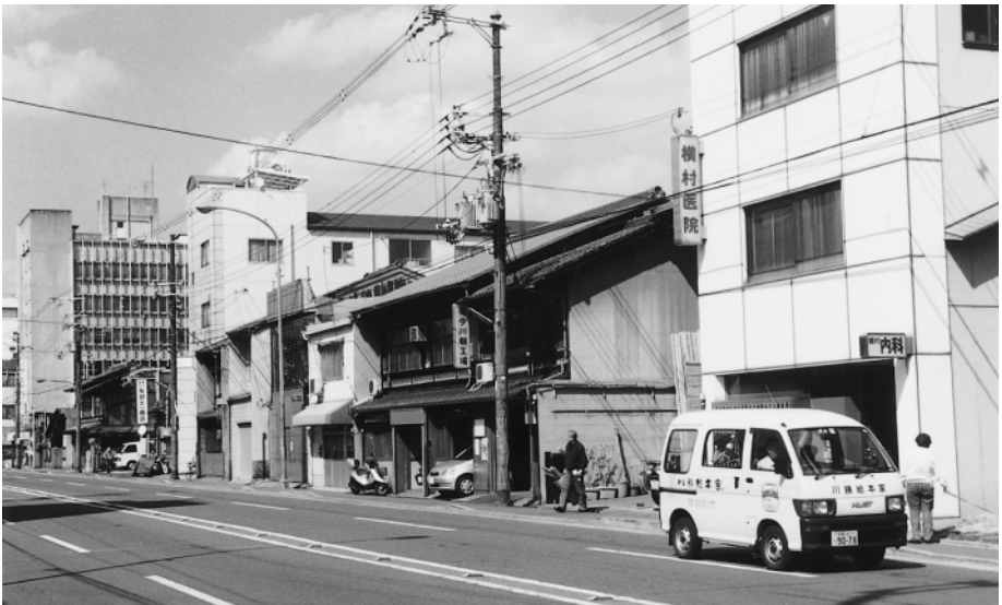
Figure 10.1 The loss of historic townscapes. One of the biggest surprises for many foreign visitors to Japan is the scarcity of old buildings. Kyoto, shown above, is an excellent example of the rapid loss of traditional townscapes, even though, having escaped wartime bombing, it still retains probably a larger proportion of traditional buildings than any other major city in the country.
