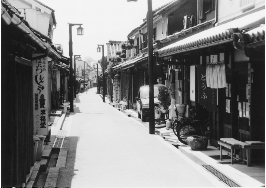
Figure 1.4 Imaichō near Nara in central Japan is an almost perfectly preserved town dating from early in the Tokugawa period.
