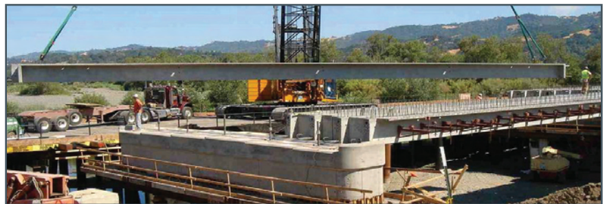
Figure 2.9 Installation of double-tee precast girders
