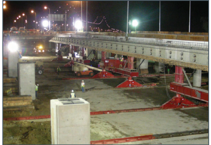
Figure 3.4 Roll-in of the new YBI viaduct
