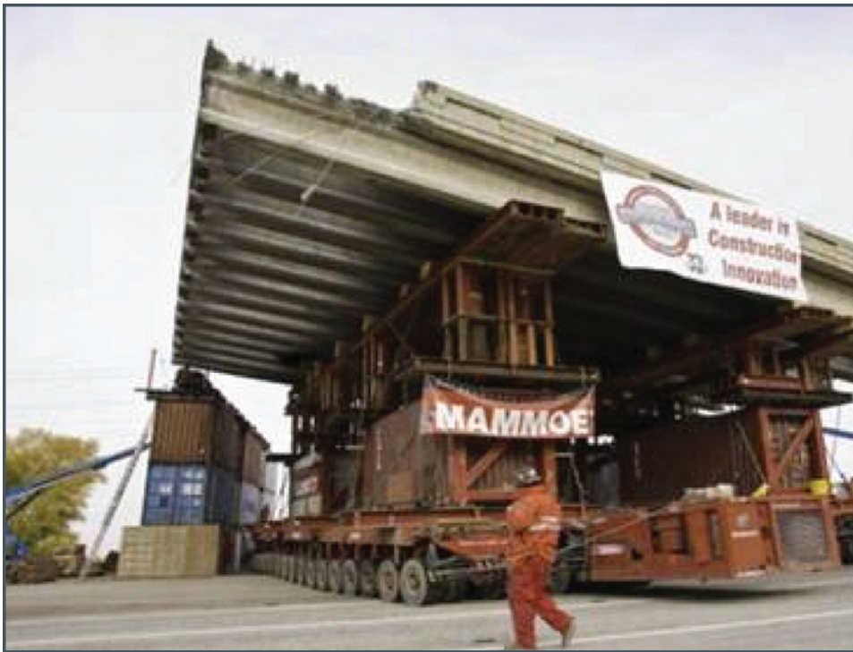
Figure 4.10 Moving existing superstructure to demolition area
