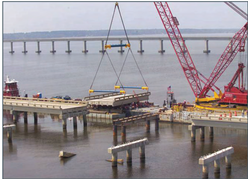
Figure 2.17 Lifting an Escambia Bay Bridge deck section with a ringer crane
