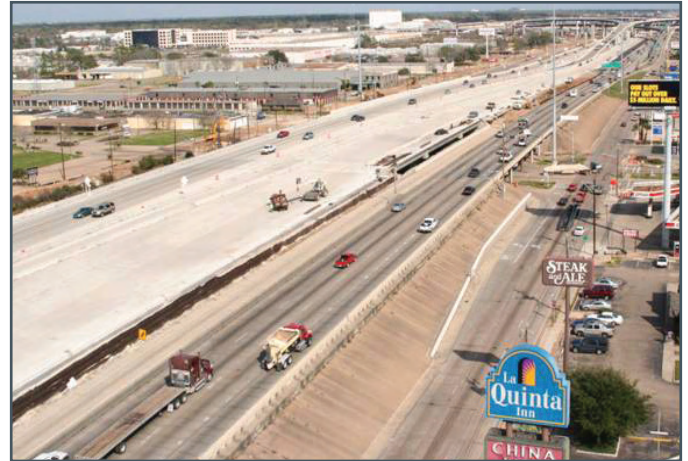
Figure 3.13 Mainline I-10 construction
