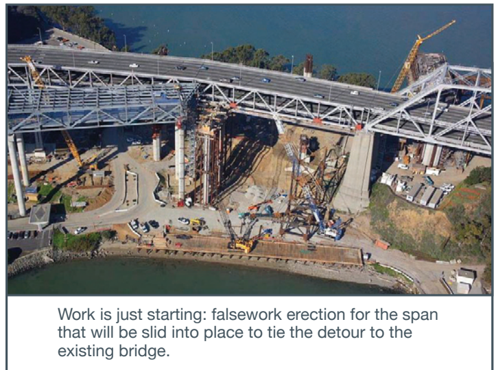
Figure 3.6 YBI detour construction
