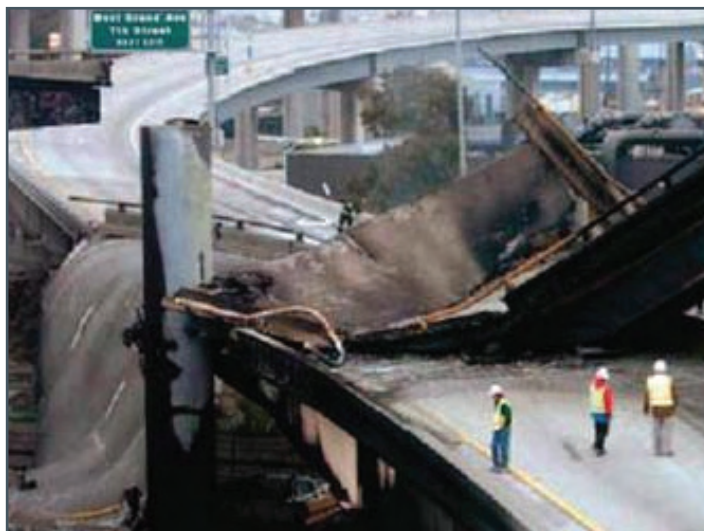
Figure 2.5 MacArthur Maze bridge damage
