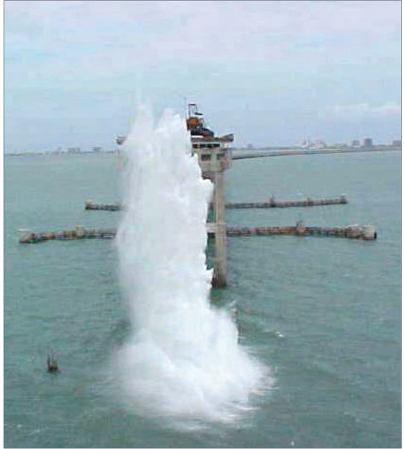
Figure 2.21 Demolition with blasting
