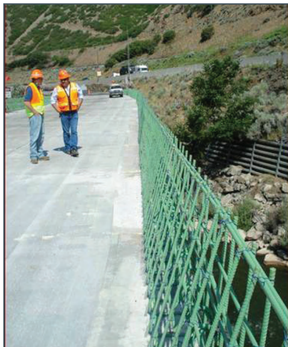
Figure 4.7 Weber Canyon precast deck panel project parapet
