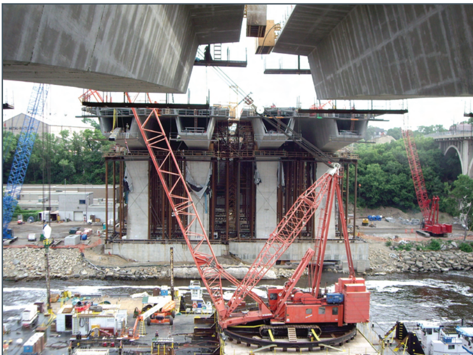
Figure 2.1 Construction of the I-35W Bridge in Minneapolis
