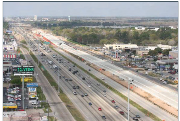
Figure 3.14 Frontage road construction
