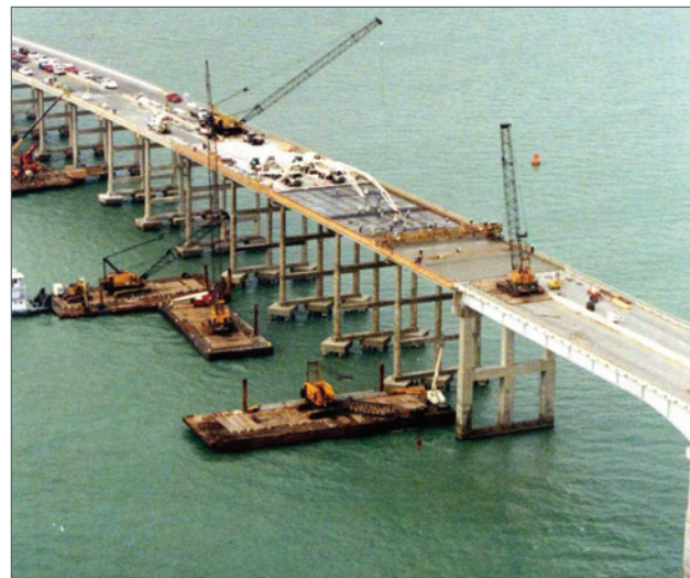
Figure 2.23 Last three spans poured on November 15
