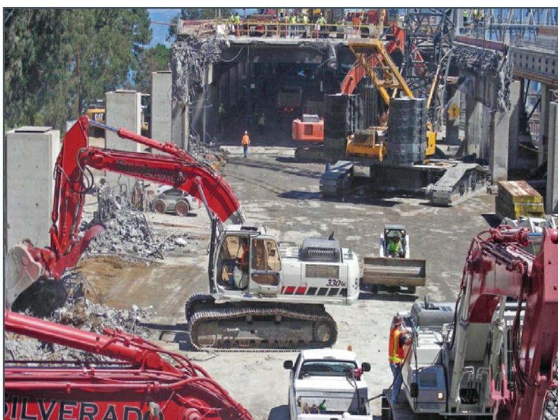
Figure 3.3 Demolition of the old YBI viaduct
