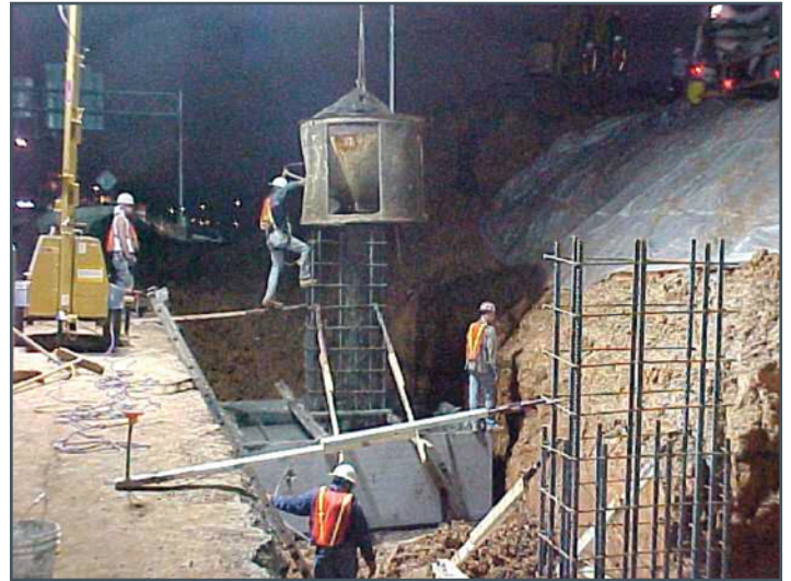
Figure 2.4 Using precast box culvert as forms
