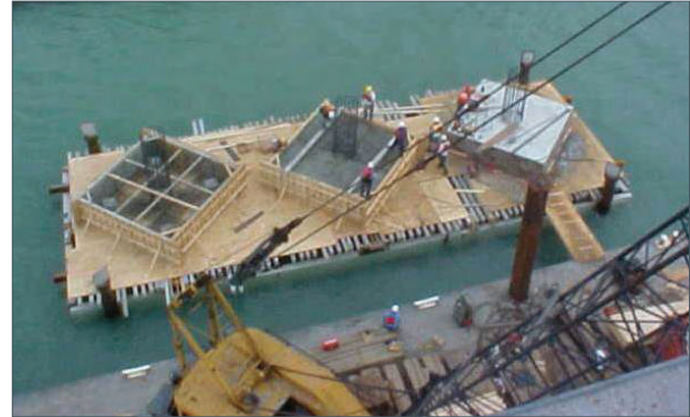
Figure 2.22 New footing construction at bent 30
