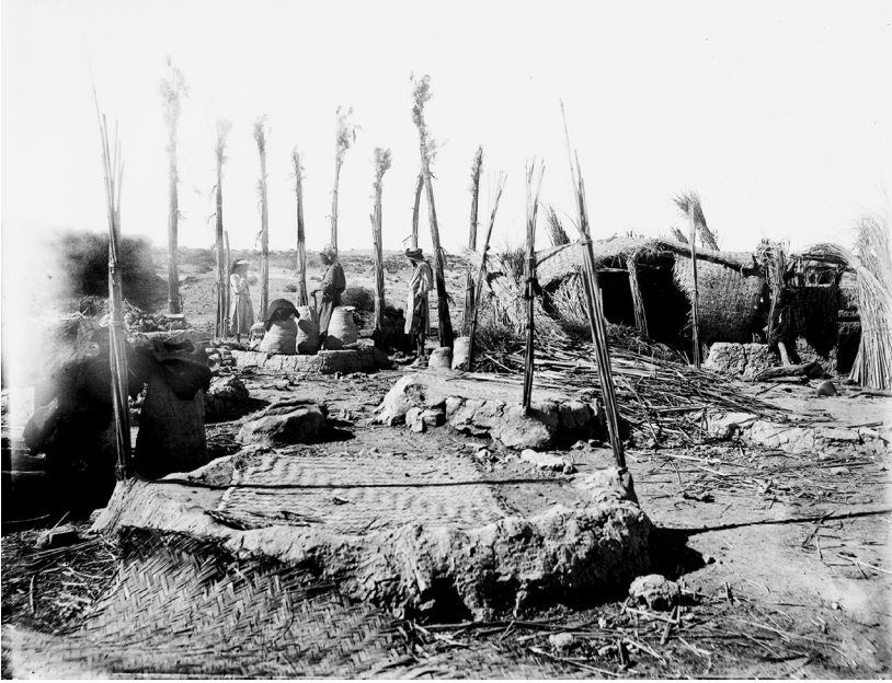
FIGURE 6.23 Nippur, construction of a hut, preparation of bundles of reeds to form the frame. (UPMAAA, Nippur 5751)
