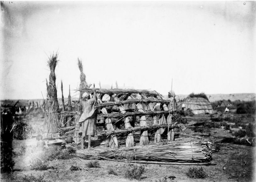
FIGURE 6.24 Nippur, construction of a hut, assembling the frame. (UPMAAA, Nippur 7003)
