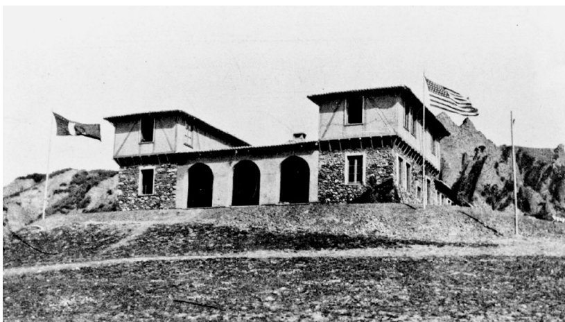
FIGURE 6.9 Sardis, front view of the field house. (PUAA, Sardis, C.7.7.f)
