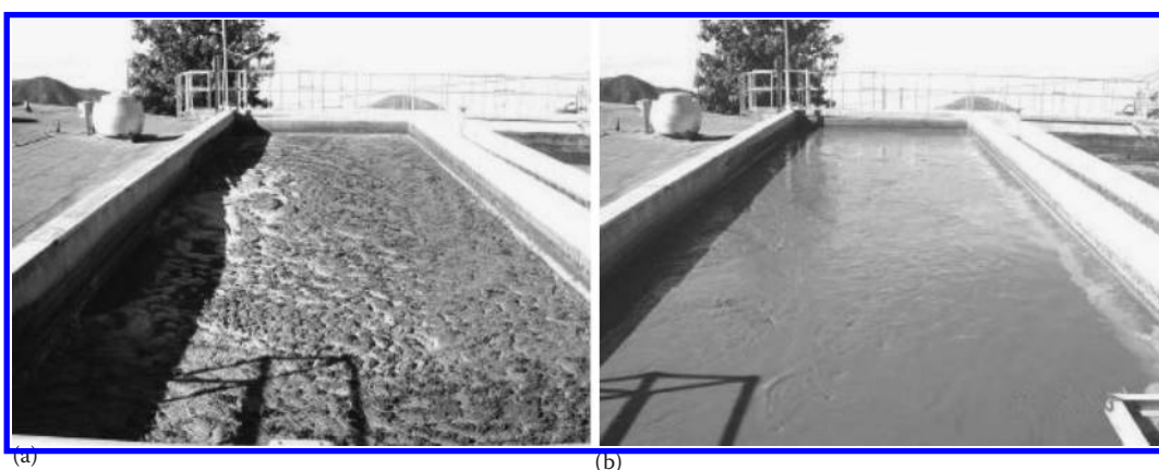
FIGURE 5.31 Effect of MPE50 on biological foam. Thick brown foam layer disappeared from anoxic tank in a municipal MBR. (a) Before MPE50 addition. (b) After MPE50 addition (400 mg/L). (From Yoon, S.-H. et al., Application of membrane performance enhancer MPE for full scale membrane bioreactors. IWA's Water Environment Membrane Technology (WEMT) Conference , Seoul, Korea, 2004a.)
