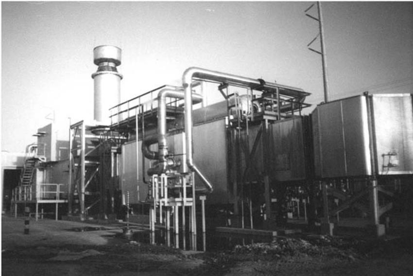
**FIGURE 1.14b** Photograph of a furnace-fired ABCO HRSG in a cogeneration plant.
