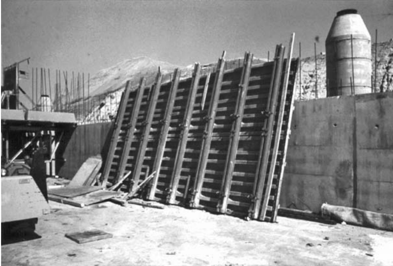
FIGURE 7.15 Ganged forms allow movement by crane and reduce re-erection costs.
