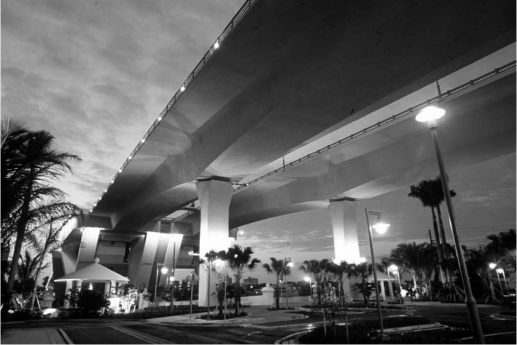
FIGURE 29.21 Clean lines and smooth undersides of the box girder superstructure enhance Fort Lauderdale's 17th Street Bridge approaches, which largely cross over land.
