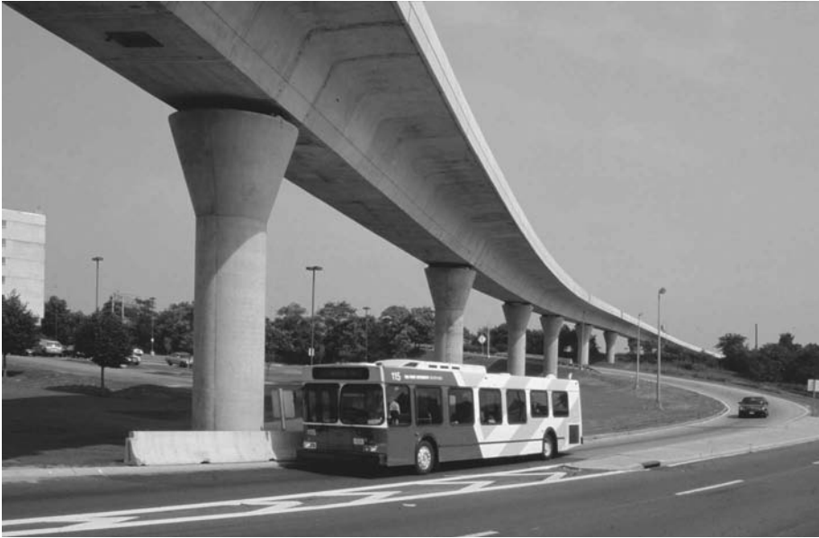
FIGURE 29.28 Consistent concrete color was achieved on New York's AirTrain JFK, despite three mixing locations.
