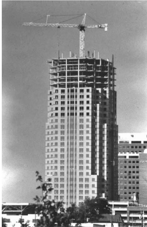
FIGURE 7.4 Planning is required to achieve maximum overall construction efficiency.
