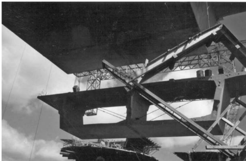
FIGURE 11.37 Erecting precast match-cast segment in cantilever construction.
