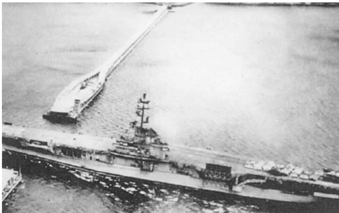
FIGURE 13.15 Hood Canal floating concrete bridge.
