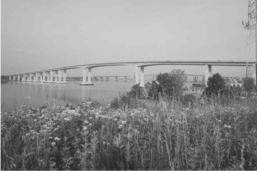
FIGURE 29.9 A high span-to-depth ratio results in structures that have elegant proportions. The Victory Bridge (440-ft main span) over the Raritan River in New Jersey serves as an excellent example.
