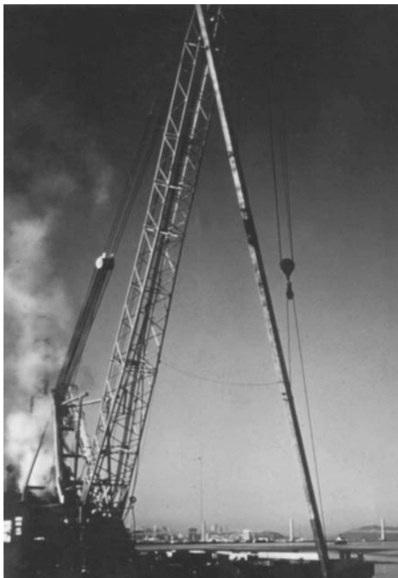
FIGURE 11.50 Lifting prestressed concrete pile into position for driving.
