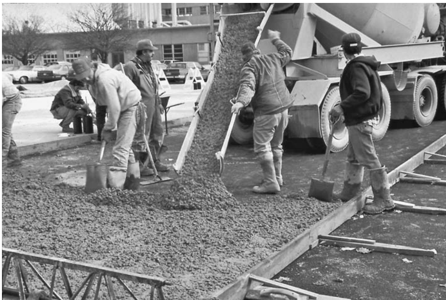
FIGURE 5.4 Workable concrete should flow sluggishly into place without segregation. (Figure courtesy of the Portland Cement Association, Skokie, IL.)
