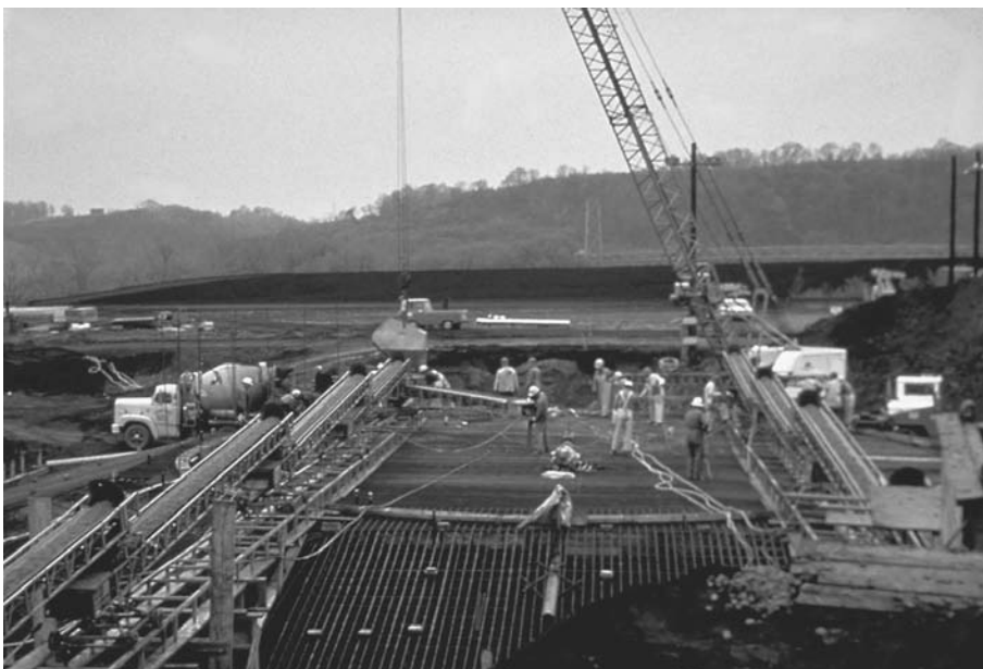
FIGURE 30.30 Conveyors in use at construction site.
