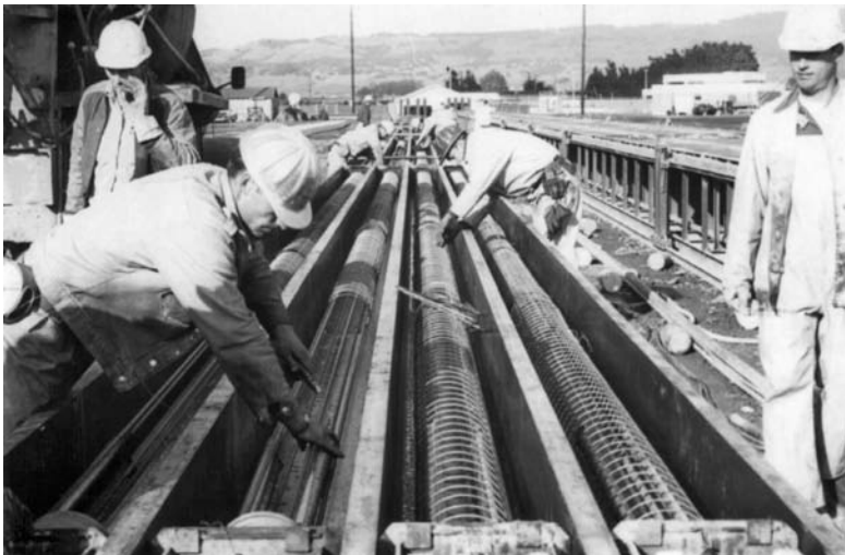
FIGURE 11.43 Spreading spirals along tensioned strands of prestressed concrete piling.
