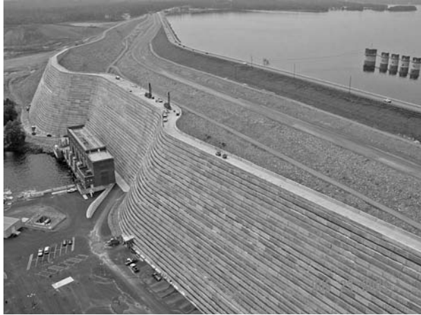
FIGURE 20.8 Saluda Dam in South Carolina, which was built downstream of an existing unstable embankment dam using 150 lb of cement and 150 lb of dumped waste ash per cubic yard. (Photograph courtesy Paul C. Rizzo Associates; Monroeville, PA.)
