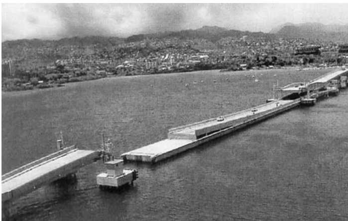
FIGURE 13.16 Ford Island (Admiral Clarey) Bridge, with the precast prestressed floating drawspan being retracted under fixed bridge spans.
