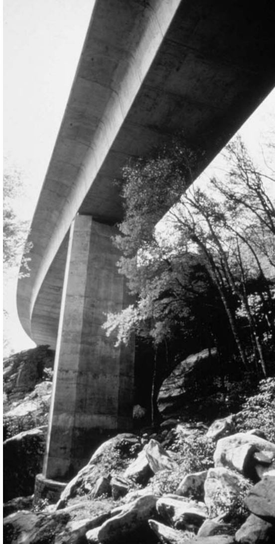
FIGURE 29.27 Octagonal-shaped piers with concave surfaces help the piers of the Blue Ridge Parkway Viaduct blend with the mountain.
