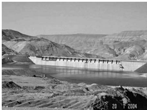
FIGURE 20.7 Mujib Dam in Jordan, which primarily used 143 lb of cement per cubic yard (no ash). (Photograph courtesy of Lahmeyer International, Bad Vilbel, Germany.)
