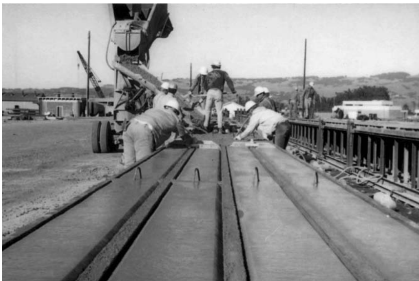
FIGURE 11.22 Concreting and finishing operations.
