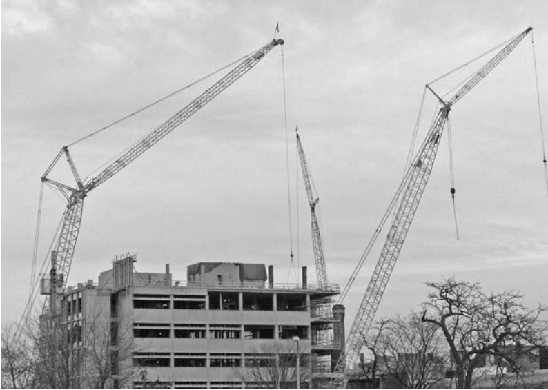
FIGURE 19.19 Mobile cranes on a mid-rise concrete building construction project.
