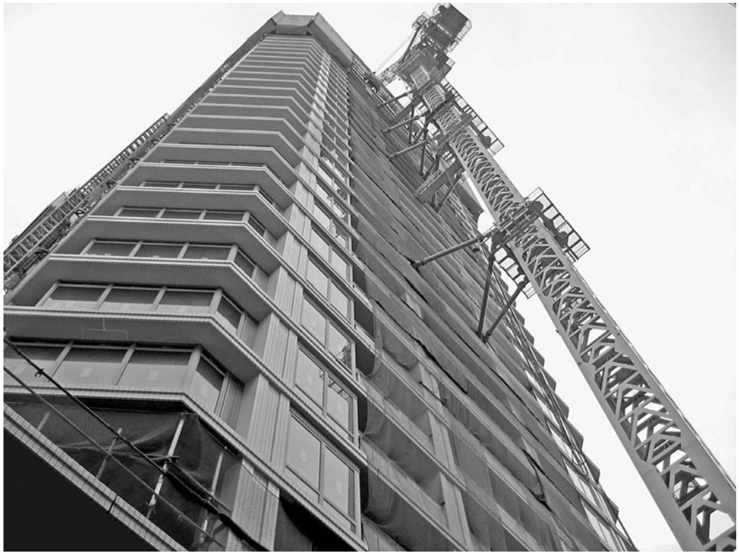
Nabeaura Tower in Yokohama, Japan, with precast ECC coupling beams in the building core for seismic resistance; the 41-story building was completed in 2007.
