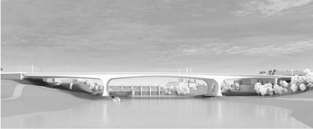
FIGURE 29.37 A functional sculptural bridge (I-35W, St. Anthony Falls Bridge in Minnesota) reflects a series of modern arch forms softly set in the context of the site to maximize openness, light, green space, and a focus on the river.
