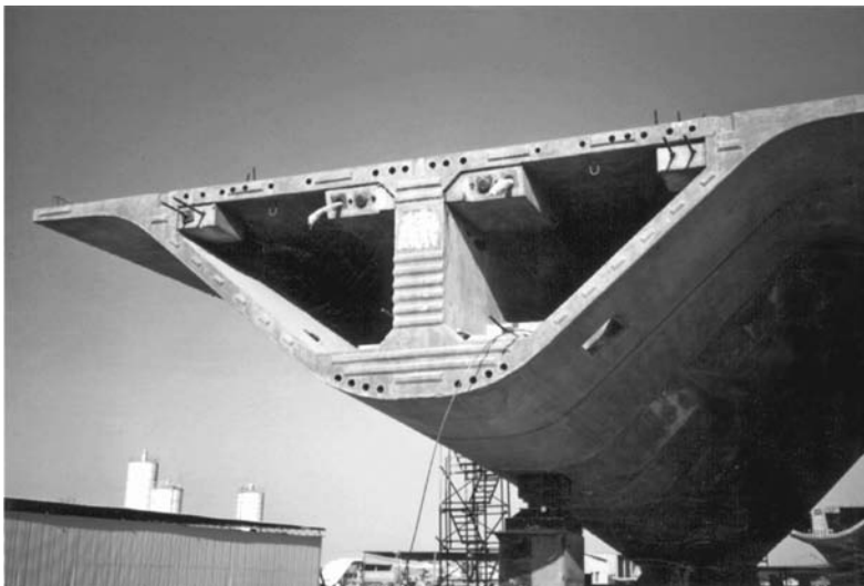
FIGURE 11.35 Precast match-cast segment for viaduct in Riyadh, Saudi Arabia. Note shear keys and anchor blocks (blisters). (Photograph courtesy of CCC Group, Athens, Greece.)
