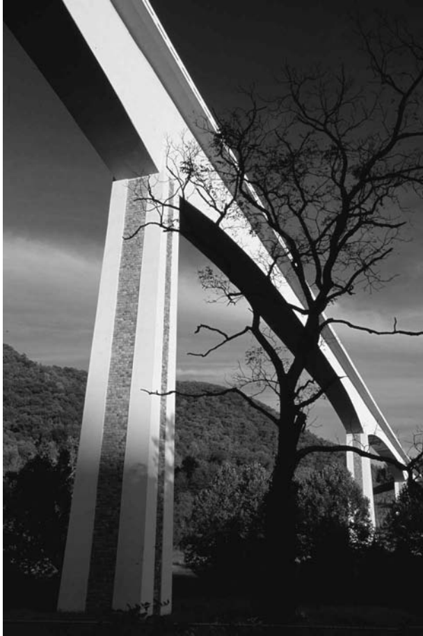
FIGURE 29.33 The pier recesses of the Smart Road Bridge are faced with Hokie Stone.
