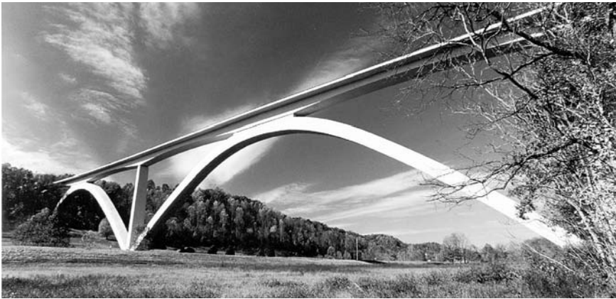
FIGURE 29.2 Natchez Trace Parkway Arches has a 582-ft main span and is located outside of Nashville near Franklin, Tennessee; the bridge was awarded the 1995 Presidential Design Award.
