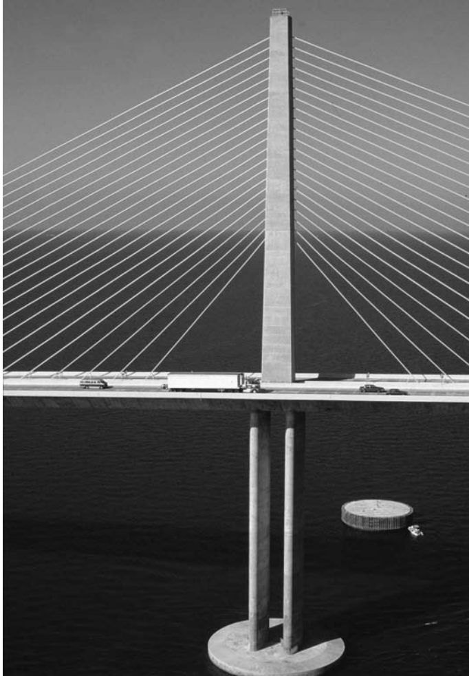
FIGURE 29.24 Elliptical pier shapes add aesthetics while reducing wind drag, an important consideration in hurricane-prone areas (I-275 Bob Graham Sunshine Skyway Bridge).
