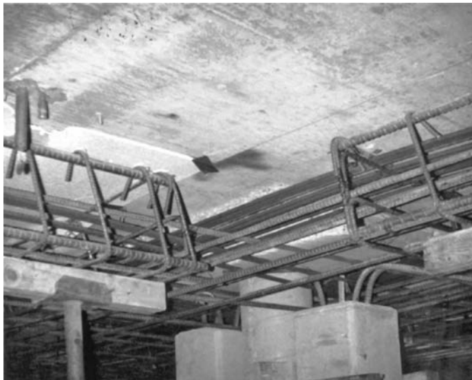
FIGURE 12.34 Tendons installed within a reinforcing cage.
