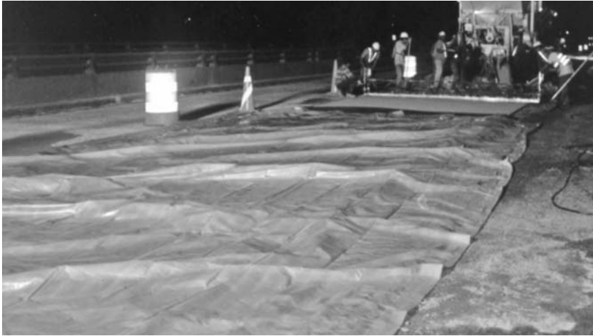
FIGURE 23.11 Polyethylene sheeting covers wet burlap for the curing period.
