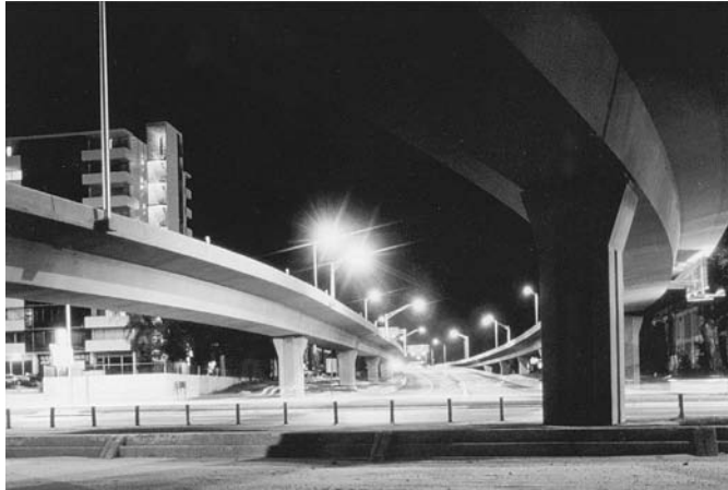
FIGURE 29.20 Interstate 110 runs through downtown Biloxi, Mississippi, on an elevated structure.
