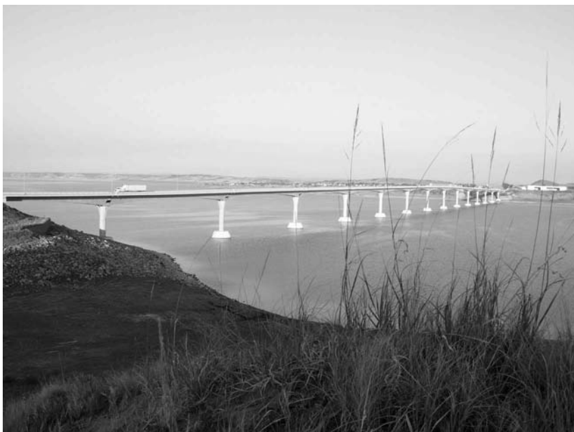
FIGURE 29.8 Four Bears Bridge in rural North Dakota has a variable depth superstructure for 316-ft spans following a uniform pattern for construction efficiency.
