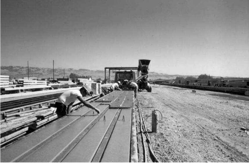
FIGURE 11.44 Placing inserts for lifting piles in pretensioned concrete piles.
