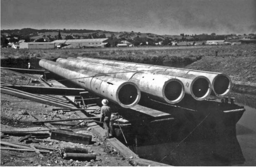
FIGURE 11.48 Loading heavy prestressed cylinder piles on barge by rolling.
