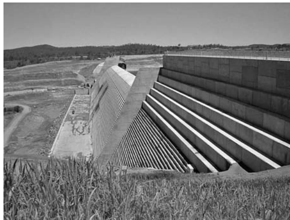
FIGURE 20.6 Burnett River (Paradise) Dam in Australia, which used 106 lb of cement per cubic yard (no ash). (Photograph courtesy of Ernest K. Schrader.)
