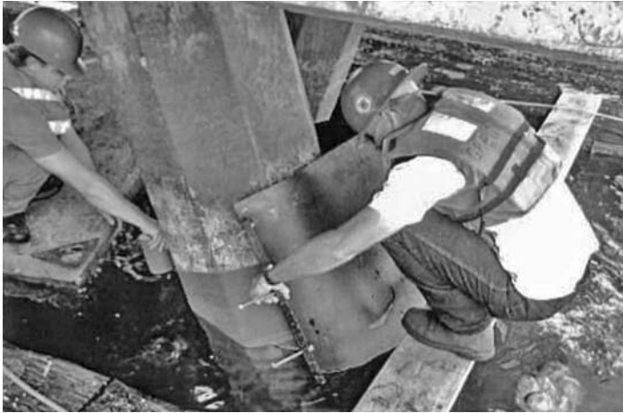
FIGURE 11.56 Attaching plastic sleeve to repair damaged prestressed concrete pile.
