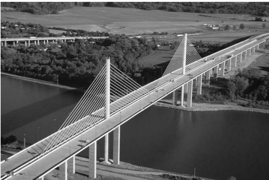
FIGURE 29.6 The Chesapeake and Delaware Canal Bridge in Delaware uses repetition of form and construction.
