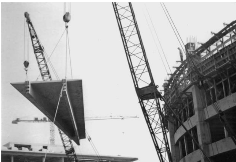
FIGURE 11.27 Erecting a tapered double-tee floor slab in circular parking garage.
