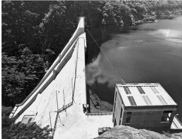
FIGURE 20.5 Miel I Dam in Colombia, which is 620 ft high and used low to medium cement content mixes and no ash. (Photograph courtesy of Ingetec S.A., Colombia.)
