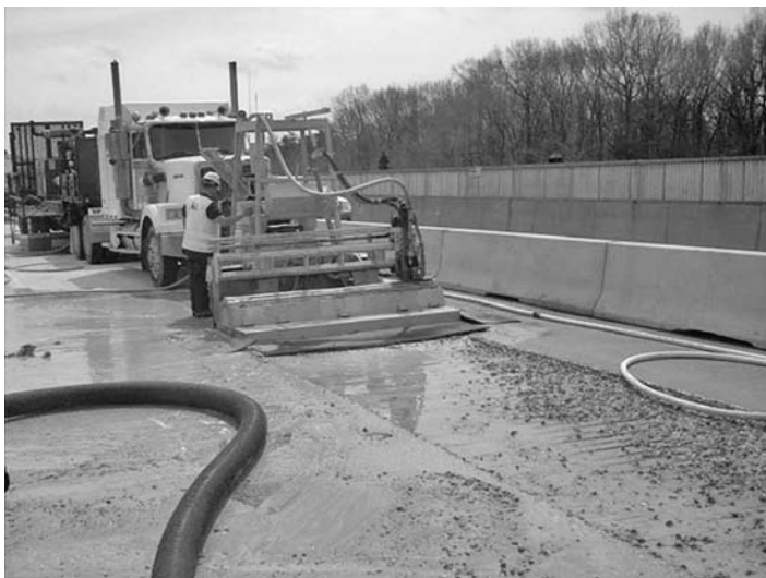
FIGURE 23.4 Hydro demolition can be used to remove concrete around reinforcing steel.
