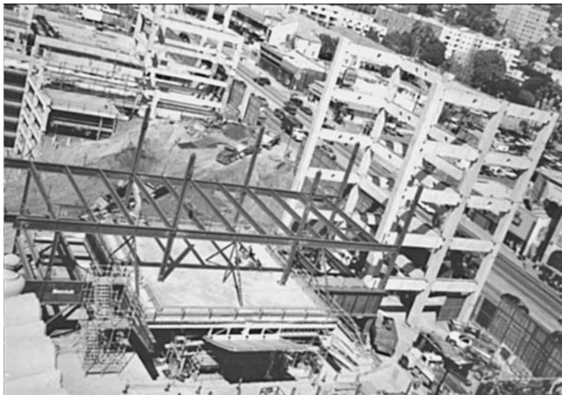
FIGURE 34.13 Precast concrete bracing tower. (Photograph courtesy of Englekirk Partners, Los Angeles, CA.)
