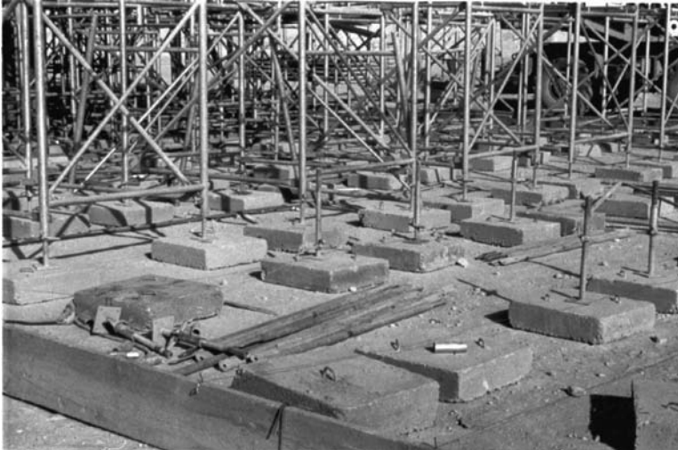
FIGURE 7.19 Precast concrete mudsills distribute bridge falsework load to soil.
