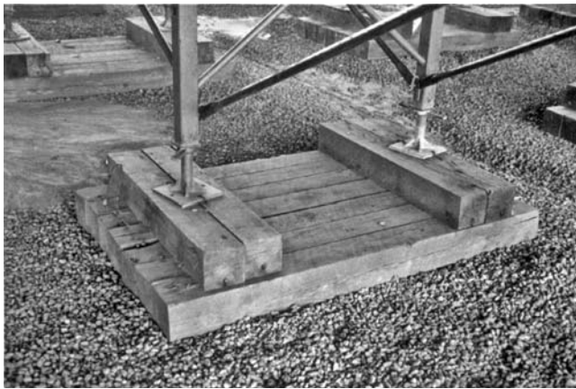
FIGURE 7.36 Wood timber grillage mudsill.
