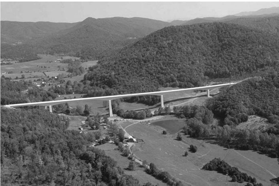
FIGURE 29.7 The long spans of Virginia's Smart Road Bridge provide for open views of the valley; the bridge was built via balanced cantilever construction.
