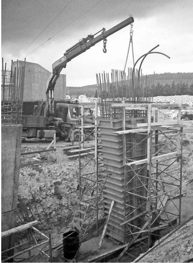
FIGURE 19.25 Knuckle-boom truck loader in form-assembly work.
