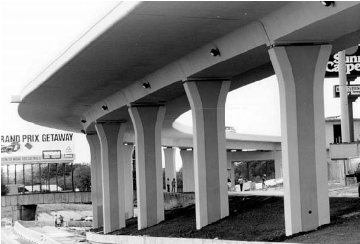
FIGURE 29.23 Subtly shaped piers carry Interstates 10 and 35 in San Antonio, Texas.
