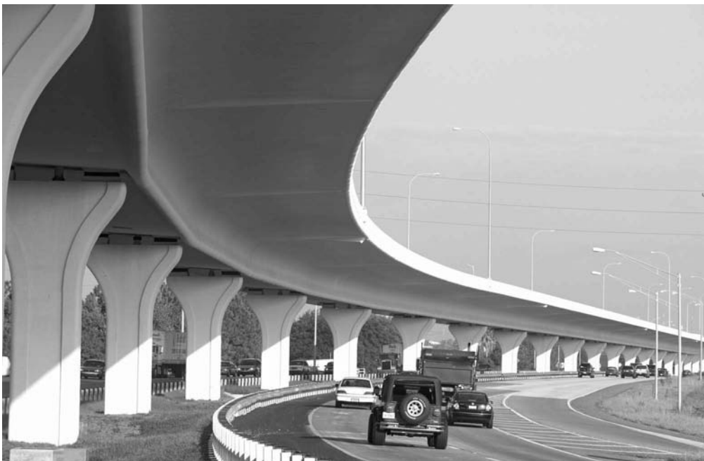
FIGURE 29.18 Utilizing the existing median for an elevated structure solved commuter congestion in Tampa, Florida. Piers use 6 ft of space in the median to carry three lanes of traffic above.
