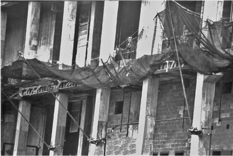
FIGURE 7.23 Fall-protection nets.
