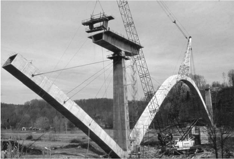
FIGURE 29.5 During construction, proven construction techniques combine to create a unique design.
