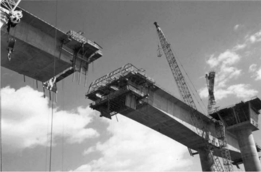
FIGURE 11.36 Cast-in-place cantilever segmental construction for the I-205 Columbia River Bridge.
