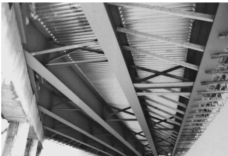
FIGURE 7.8 Stay-in-place corrugated galvanized metal deck for bridge-slab form.
