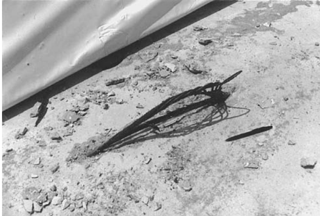
FIGURE 12.17 Vertical loop resulting from exit of seven-wire strand.
