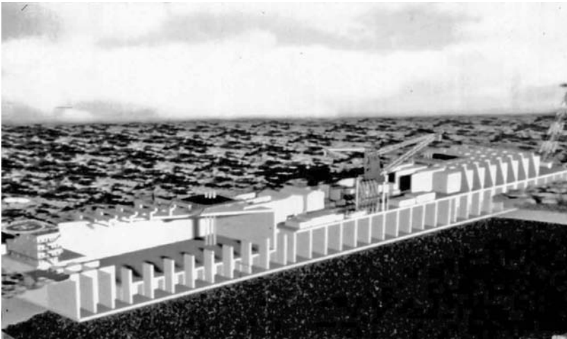
FIGURE 11.53 Offshore LNG Import Terminal under construction; it will be towed to the Adriatic and be seated as a gravity-based structure (GBS). (Photograph courtesy of Exxon-Mobil, Irving, TX.)
