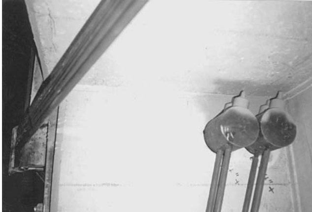
FIGURE 12.26 Alternative connection of external unbonded tendons.
