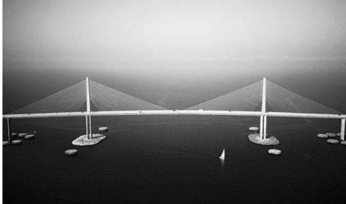
FIGURE 29.1 Bob Graham Sunshine Skyway Bridge has a 1200-ft main span and carries I-275 across Tampa Bay, Florida; the bridge was the recipient of the 1988 Presidential Design Award.
