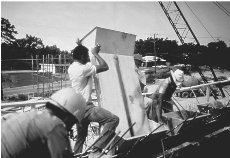
FIGURE 30.32 Tremie being placed in position for use.
