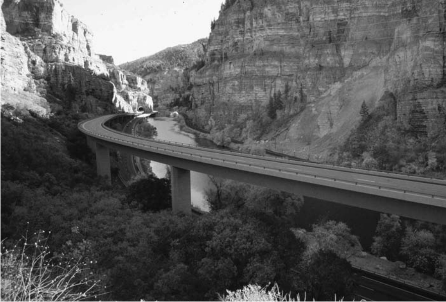
FIGURE 29.31 A stain was used to blend the Hanging Lake Viaduct into Glenwood Canyon, Colorado.
