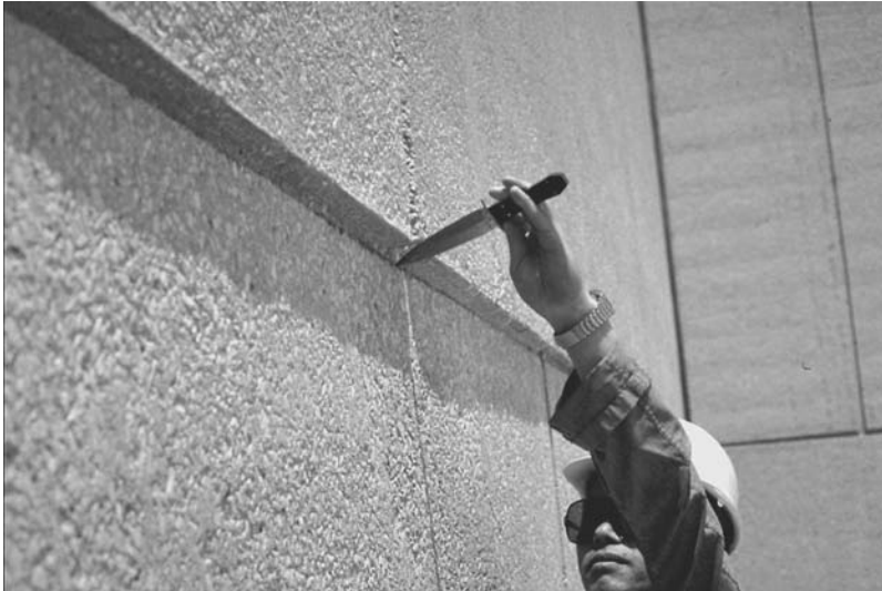
FIGURE 30.12 Movement of upper form from the plane of the form below during placement and consolidation of the concrete.
