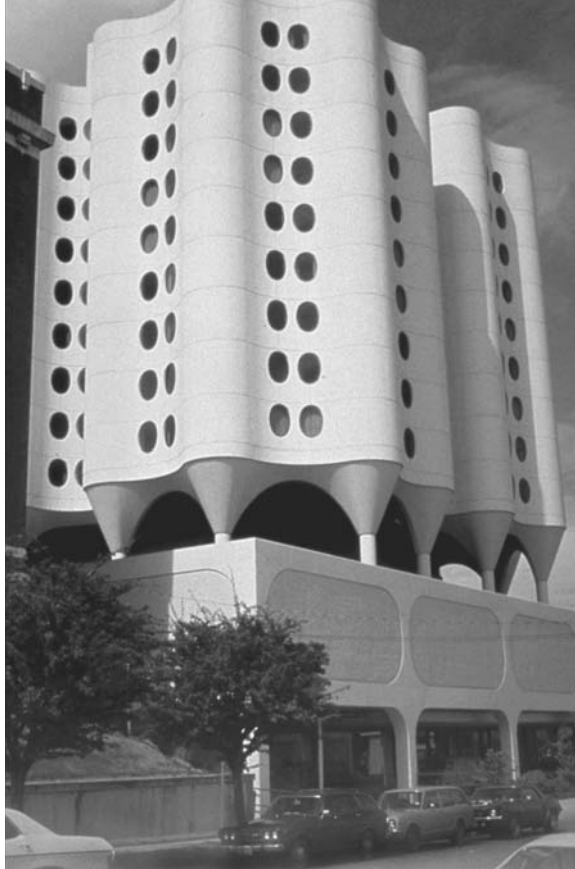
FIGURE 30.33 Concrete pumped from the bottom up to minimize consolidation problems and bug holes. This hospital building was designed by Bertram Goldberg of Chicago.
