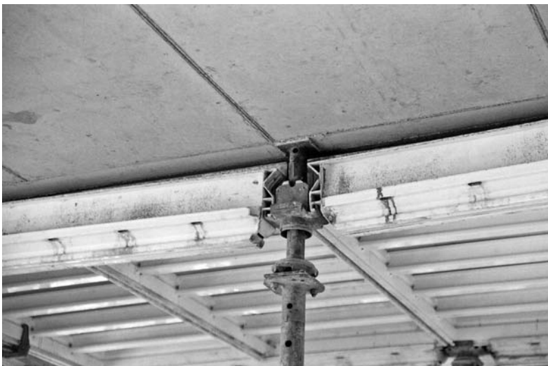
FIGURE 7.18 Drop-head shore allowing removal of panels and beams. (Figure courtesy of MEVA Formwork Systems, Haiterbach, Germany.)
