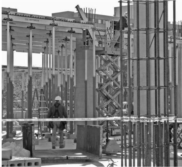
FIGURE 19.28 Scissor lift in slab deck formwork.
