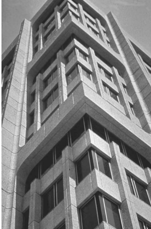
FIGURE 30.9 Heavy abrasive, blasted, cast-in-place, gap-graded concrete texture on the Tennessee State Office Building in Memphis, Tennessee; architect, Roy Harover.
