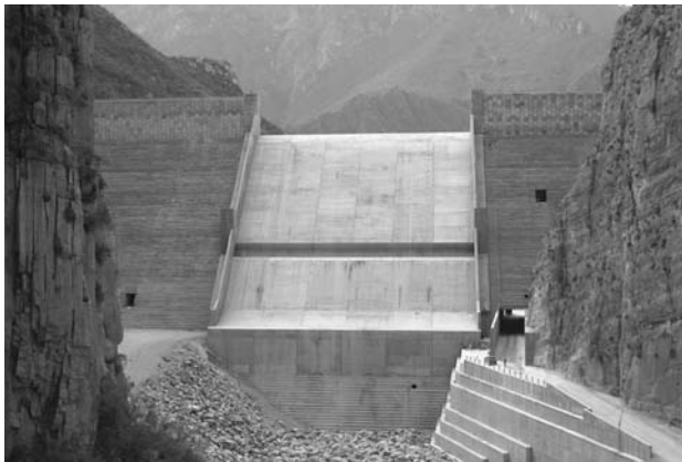
FIGURE 20.9 Rompepicos Dam in Mexico, which is 350 feet high; mostly used 73 lb of cement and 54 lb of waste ash per cubic yard. (Photograph courtesy of Ernest K. Schrader.)
