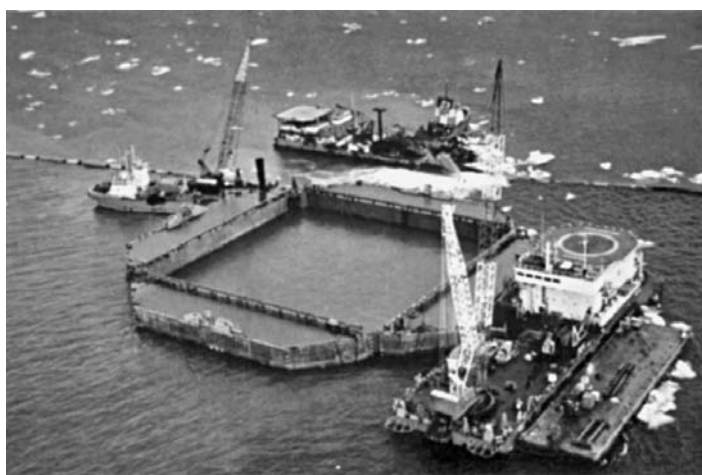
FIGURE 13.21 Concrete retaining-wall caissons. (From Anon., Ocean Industry , 21(8), 32, 1986.)
