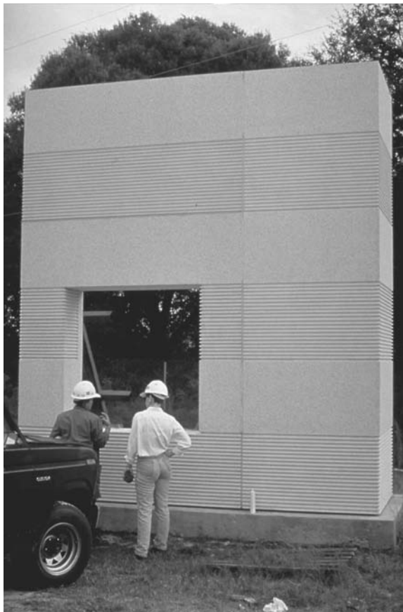
FIGURE 30.5 Mock-up panels for USAA regional office in Tampa, Florida; architect, Spillis Candela & Partners, Inc., Coral Gables, Florida.
