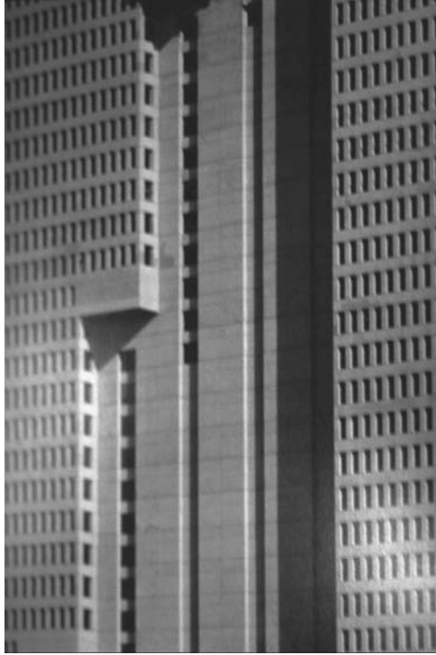
FIGURE 30.1 First United Tower, Fort Worth, Texas; architect, Sikes, Jennings & Kelly, Houston; medium, sandblast texture.
