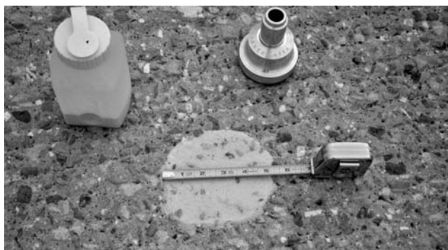
FIGURE 23.7 Macrotexture depth measurement to ensure surface preparation (ASTM E 965).
