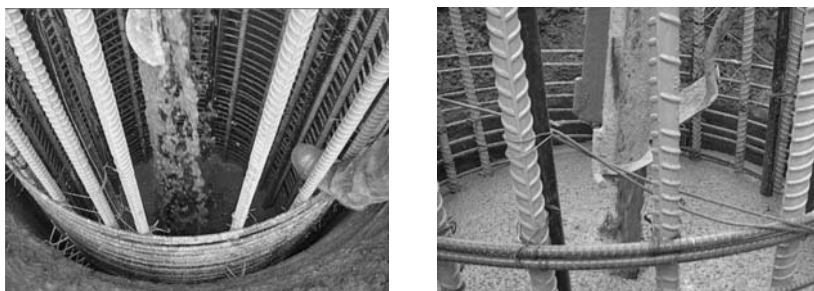
FIGURE 15.10 SCC in drilled shafts.
