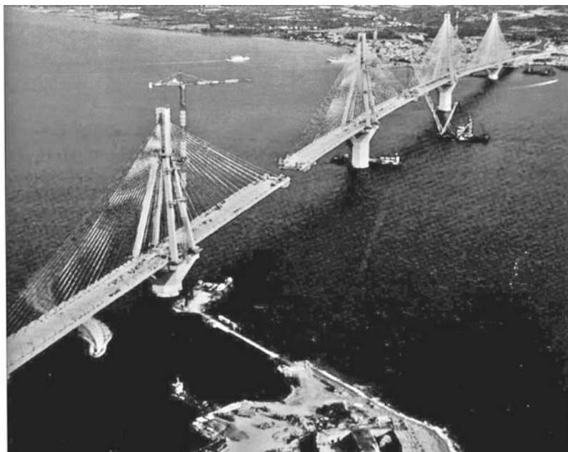
FIGURE 11.58 Rion-Antirion cable-stayed bridge across Gulf of Corinth, Greece.
