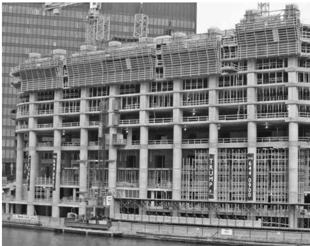
FIGURE 19.30 Crane-independent self-climbing forming system (Trump Tower, Chicago).
