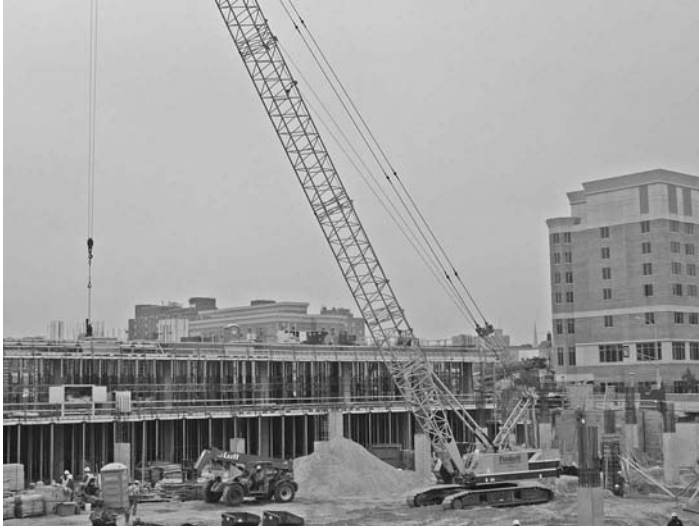
FIGURE 19.20 Crawler crane.
