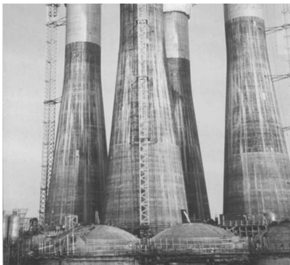
FIGURE 11.2 Statford B offshore platform with prestressed concrete shafts. (From Gerwick, B.C., Jr., Construction of Prestressed Concrete Structures , John Wiley & Sons, New York, 1996. With permission.)
