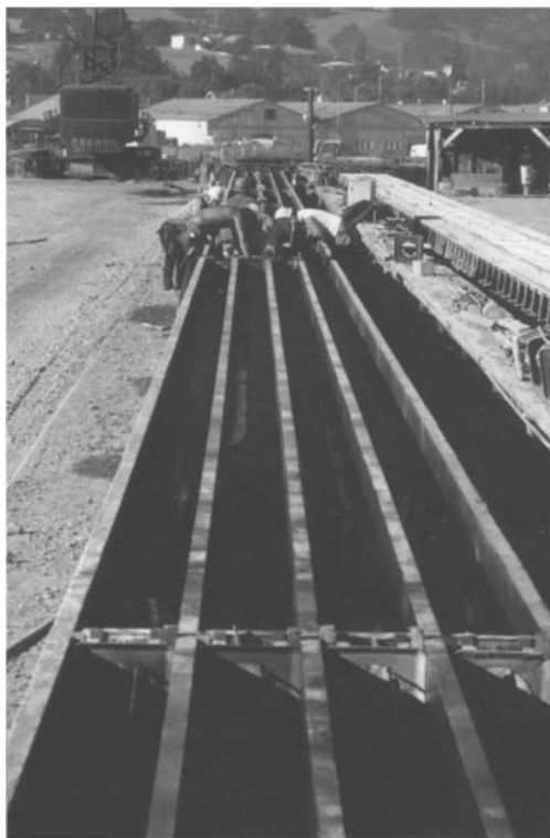
FIGURE 11.20 Stretching strands down pretensioning bed.
