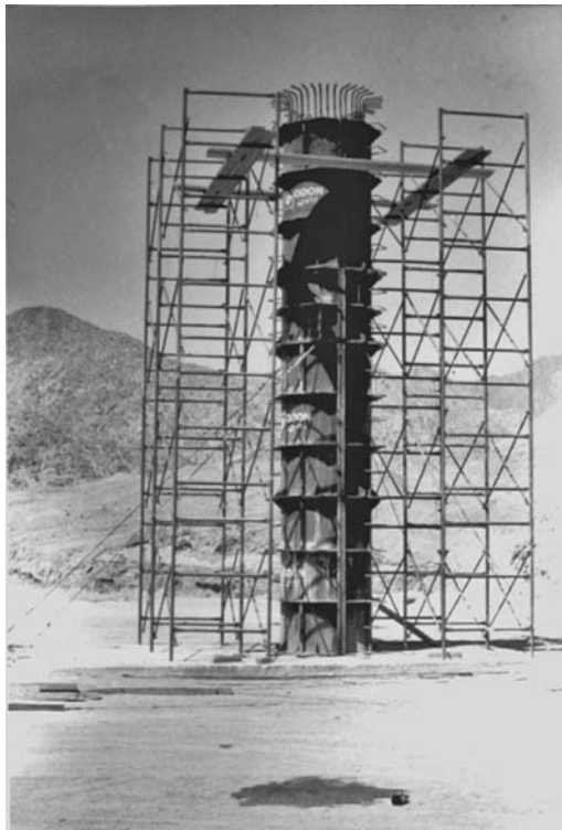
FIGURE 7.12 Steel round-column form with access scaffolding in preparation.
