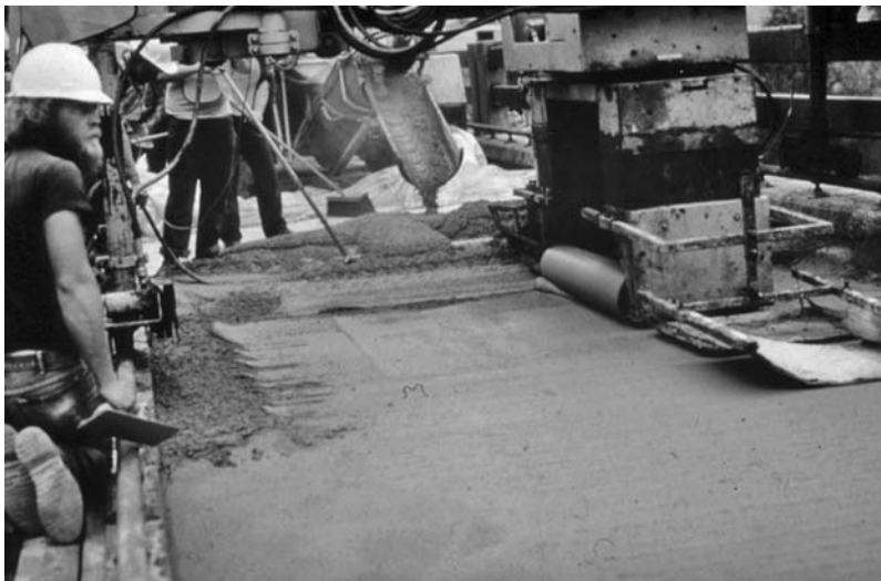
FIGURE 23.9 Screed strikes off and consolidates the overlay concrete.
