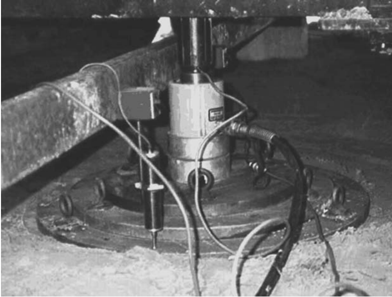
FIGURE 14.36 Plate load test.
