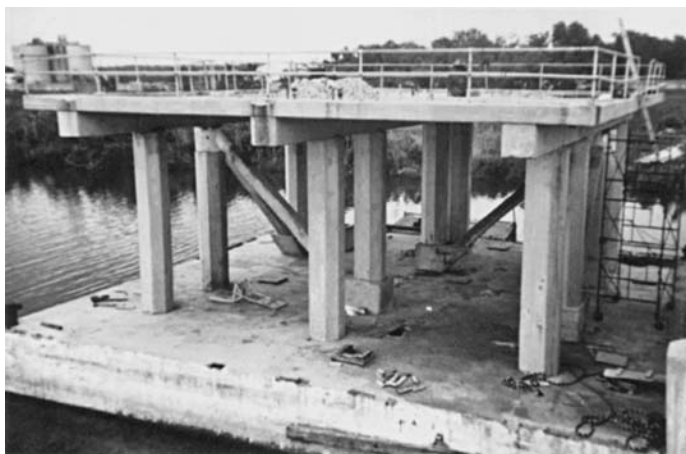
FIGURE 13.5 Eighteen-year-old floatable/bottom-founded platform after refloating and relocation to wet dock for equipment modifications.
