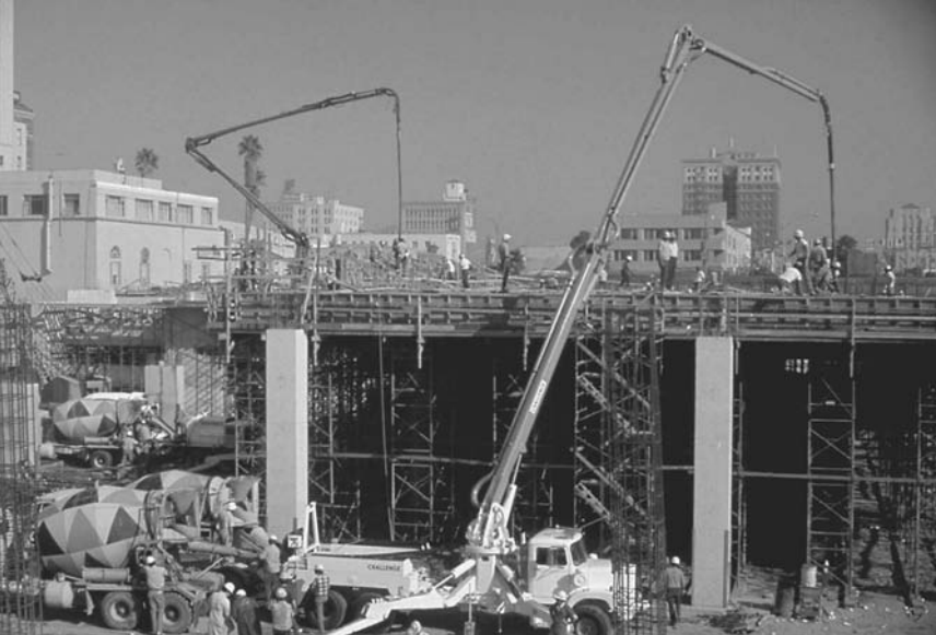
FIGURE 30.31 Several concrete pumps in use at construction site.
