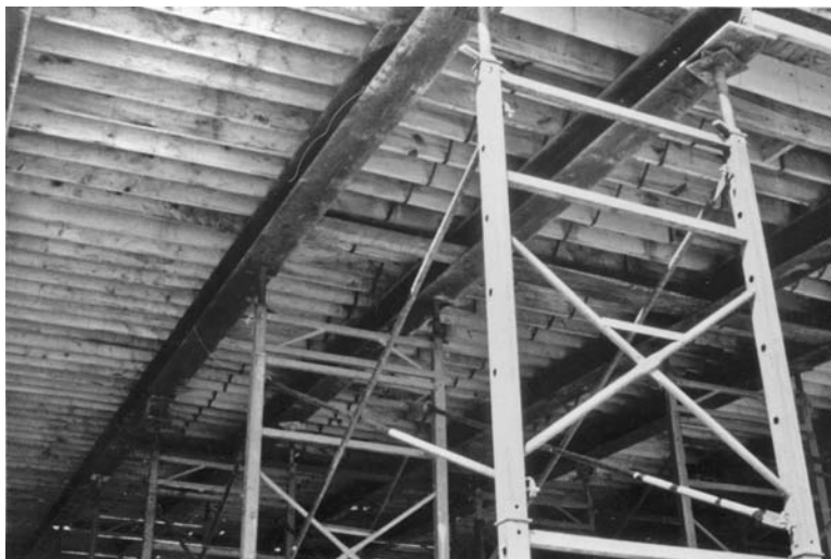
FIGURE 7.31 Wood joists supported on steel beams and steel scaffolding towers.
