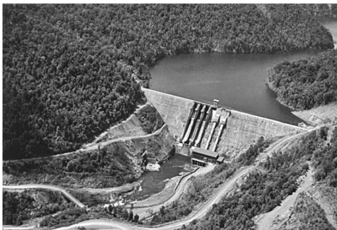
FIGURE 20.4 Balambano Dam in Indonesia, which used 121 lb of cement and 81 lb of fly ash per cubic yard. (Photograph courtesy of Ernest K. Schrader.)
