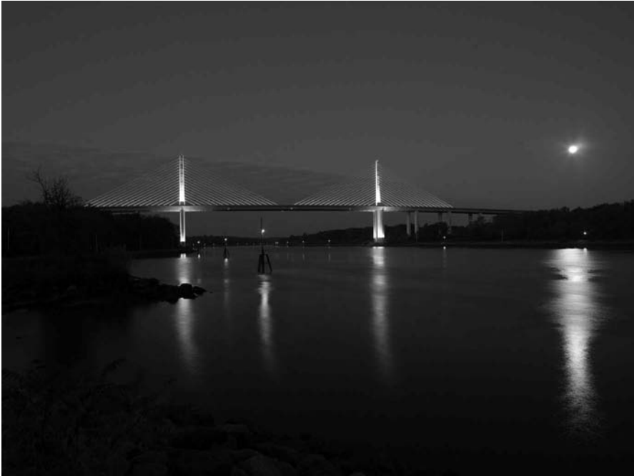
FIGURE 29.34 The Chesapeake and Delaware Canal Bridge has aesthetic lighting suitable to its less populated location.
