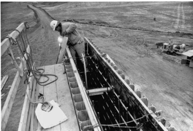
FIGURE 7.24 Work platform being installed on tall wall form.
