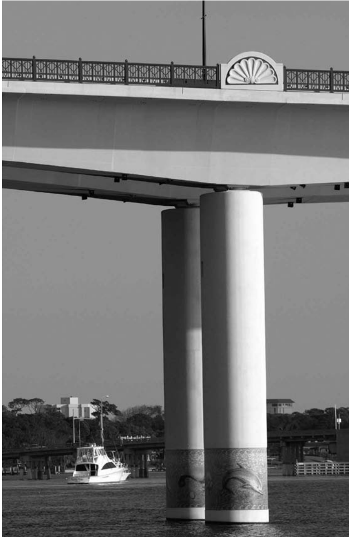
FIGURE 29.26 Mosaic tile patterns on the piers provide visual interest for boaters under Florida's Broadway Bridge.
