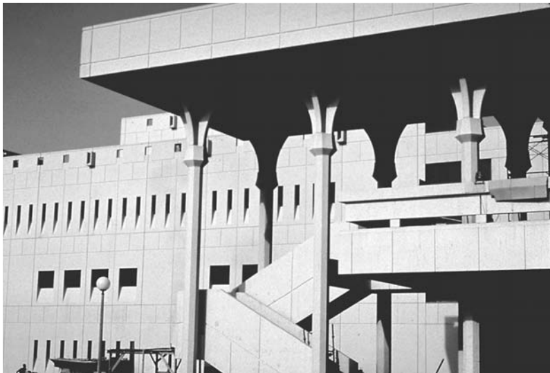
FIGURE 30.4 Matching architectural cast-in-place and precast concrete at King Saud University in Riyadh, Saudi Arabia; architects, HOK, St. Louis, MO.
