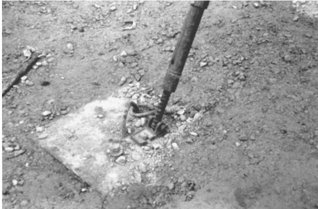
FIGURE 7.20 Formwork brace anchored to buried concrete mass.
