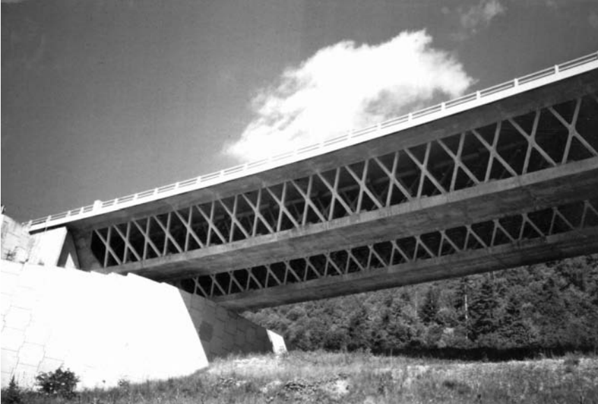
FIGURE 11.12 Sylhan Viaduct in the French Alps combines high performance, high-strength concrete truss members with external tendons inside trussed extension. (Photograph courtesy of Bouygues, Paris, France.)
