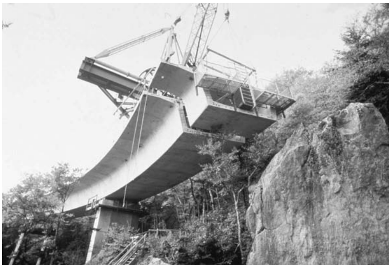
FIGURE 29.12 A progressive unidirectional cantilever, from above, protected the mountain during construction.
