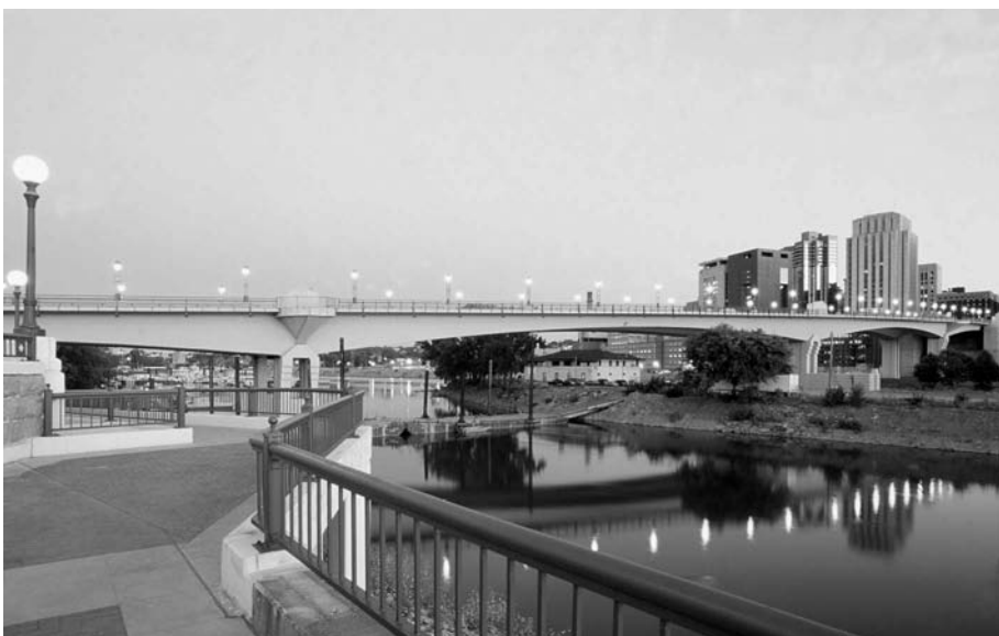
FIGURE 29.10 The Wabasha Freedom Bridge in St. Paul, Minnesota, achieves a span-to-depth ratio of 20 and demonstrates that varying the depth of the superstructure creates pleasing shapes.
