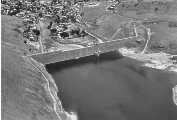
FIGURE 20.2 Willow Creek Dam in Colorado, which was the world's first major all RCC dam and used mostly 80 lb of cement and 32 lb of ash per cubic yard. (Photograph courtesy of Ernest K. Schrader.)
