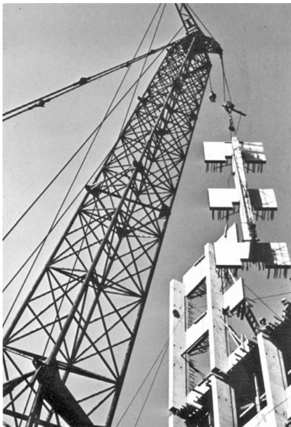
FIGURE 11.14 Two-way pretensioned concrete wall units serve both structural and architectural purposes in the construction of new university building.
