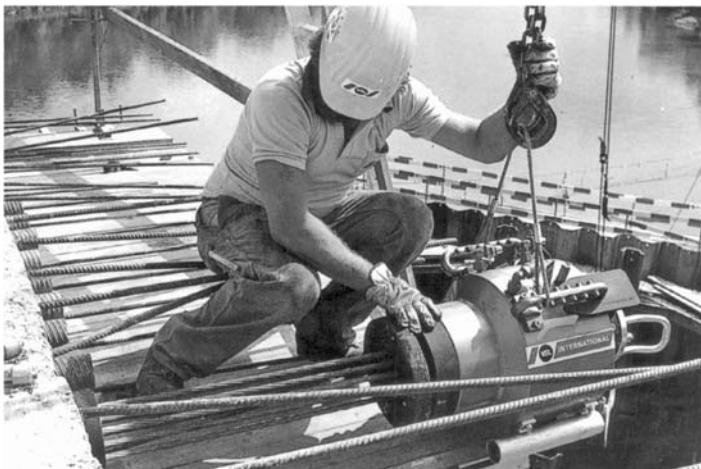
FIGURE 11.18 The stressing operation. (Photograph courtesy of VSL Corporation, Campbell, CA.)
