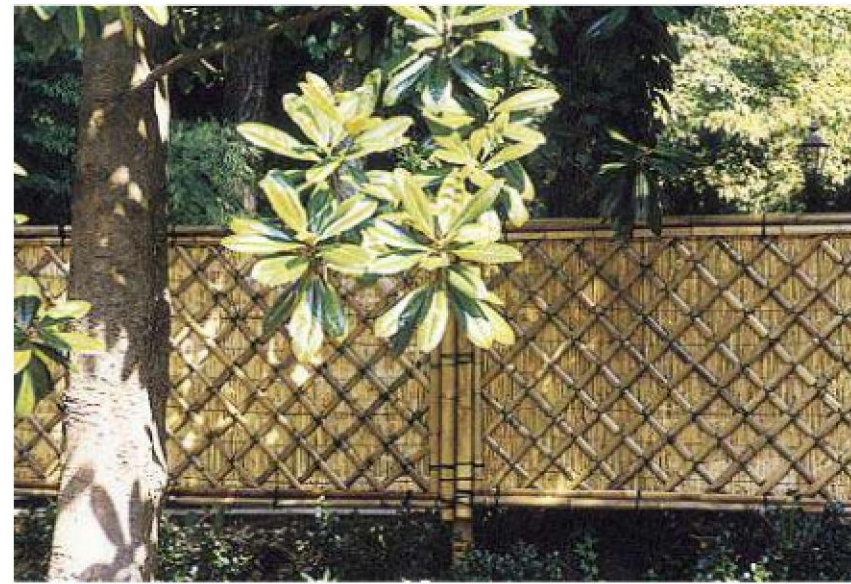
Split bamboo creates diamond patterns over panels of reed fencing.
