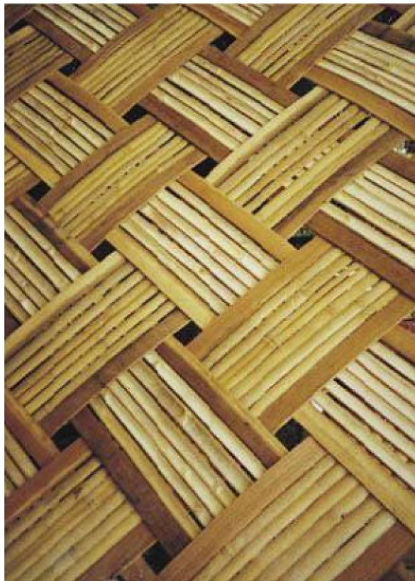
Detail of a split and woven bamboo fence panel. DESIGN AND PHOTO BY THE BAMBOO-SMITHS
