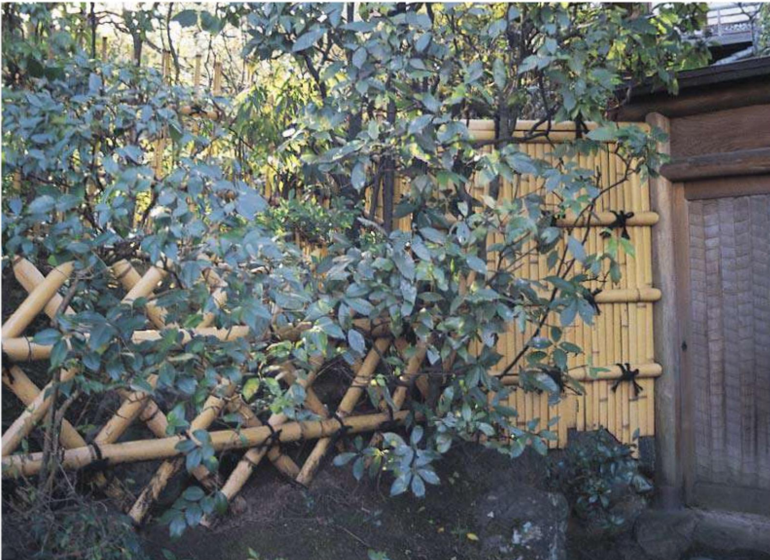
Clockwise from top: Bamboo poles are attached on the diagonal to create this fence at the Bamboo Farm near Savannah, Georgia.
