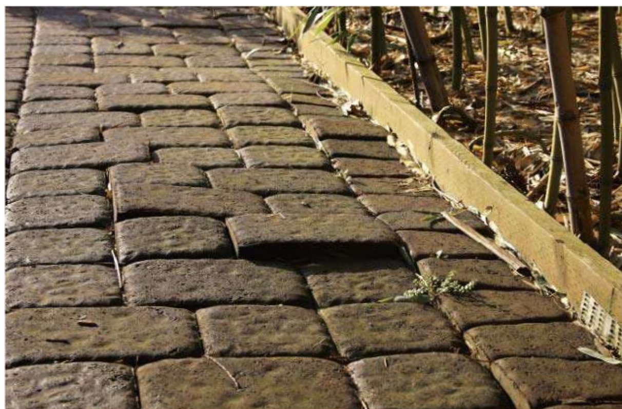
A thin wooden edging along a path will not deter bamboo from running. Here, rhizomes trying to grow new culms push up a brick.
