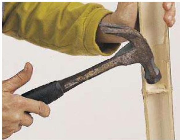
You can use a hammer to knock out diaphragms.
