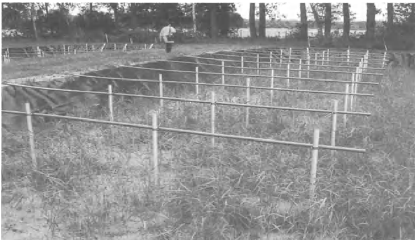
Fig. 7. 7. Sludge Composting Plant at Wienhausen before Commencement of Operation
