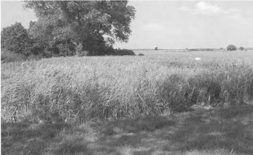
Fig. 7.11. Multistage Planted Soil Filter at Konau
