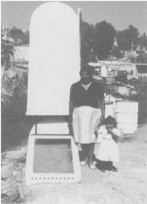
Fig. 8.11. Prefabricated Dry SIRDO - Type 6M
