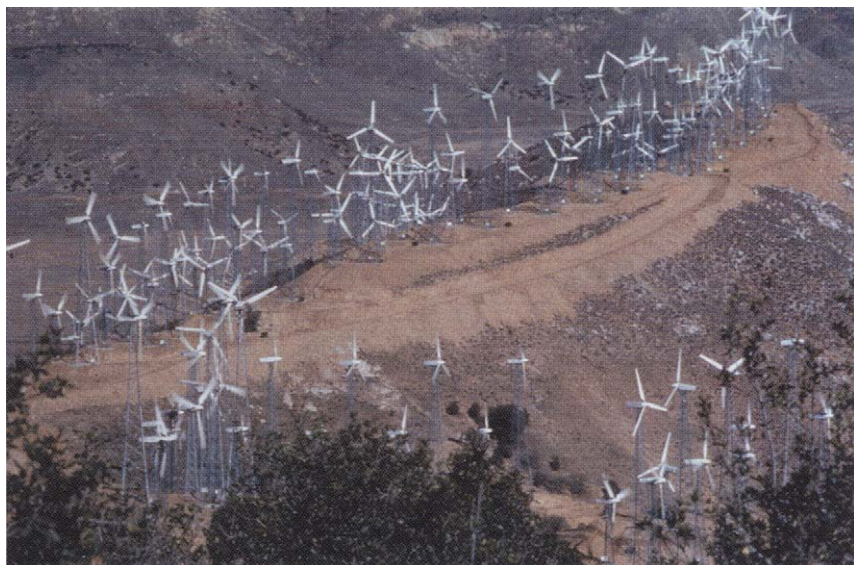
FIGURE 9.18 Mountaintop removal? Construction on this steep ridge at Zond's Victory Garden site required blasting and bulldozing pads for erecting the wind turbines. This photo, taken in 1986, is reminiscent of the "mountaintop removal" method of mining found in the coal fields of Appalachia. The wind turbines on the right have since been removed because of poor wind conditions. As of 1998 the foundations had not yet been removed. (Courtesy Paul Gipe.)
