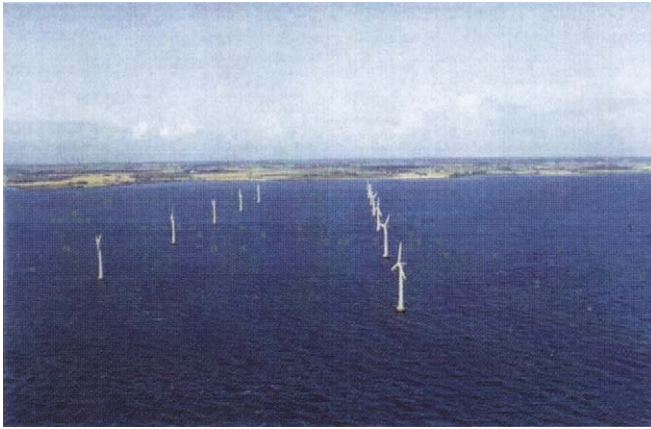
FIGURE 6.6 Vindeby: 11 (4.95-MW installation) turbines. The world's first offshore wind farm was commissioned 2 kilometers off the north coast of Lolland in September 1991. The 11 wind turbines stand in shallow waters 3 to 5 meters (10–20 feet) deep and are oriented in two parallel rows trending in a northwest to southeast direction, transverse to the prevailing winds. This simple pattern is easy to perceive from all angles, and the perspective corridor created by the two rows of columns appears dramatic as you pass by. The wind turbines form part of an intimate visual interplay with the coastal landscape. In bright sun, the wind turbines are easy to see from the shore, appearing white. In overcast weather, however, they assume a grayish cast, which significantly reduces their visual dominance.
