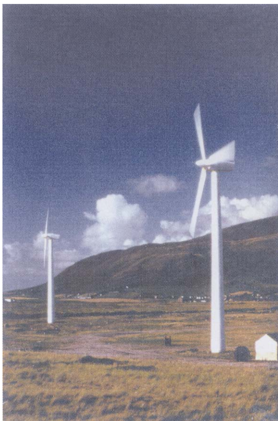
FIGURE 2.3 Some of the five Vestas 225-kW wind turbines at the former Haverigg air base, southwest Cumbria. The turbines are 27 meters (90 feet) in diameter and stand atop towers 30 meters (110 feet) tall. The turbines are located near the shore of the Irish Sea. Black Combe rises to the northwest and a prison borders the site to the east. Across Duddon Sands to the east, the turbines of Kirkby Moor are sometimes visible. The Lake District National Park is less than 40 kilometers (25 miles) to the north. (Courtesy Paul Gipe.)
