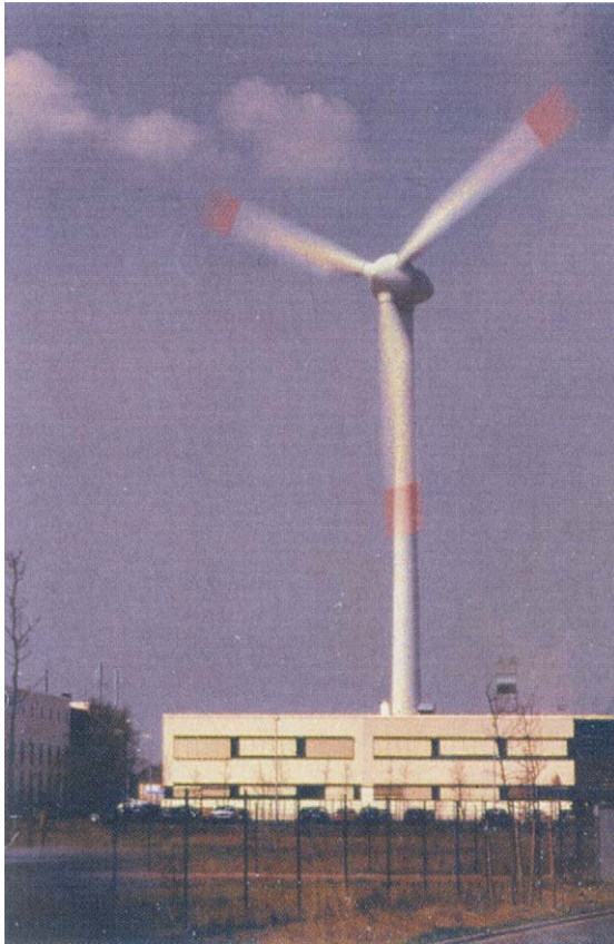
FIGURE 7.7 Lower Saxony, Northern Germany. Enercon is one of Germany's leading manufacturer's of 1.5-MW wind turbines. Here is one of Enercon's E66s outfitted in anticollision markings looming over Enercon's blade assembly hall in an industrial suburb of Aurich in Östfriesland province. The E66 uses a rotor 66 meters (215 feet) in diameter on a tower of equivalent height. (Courtesy Paul Gipe.)
