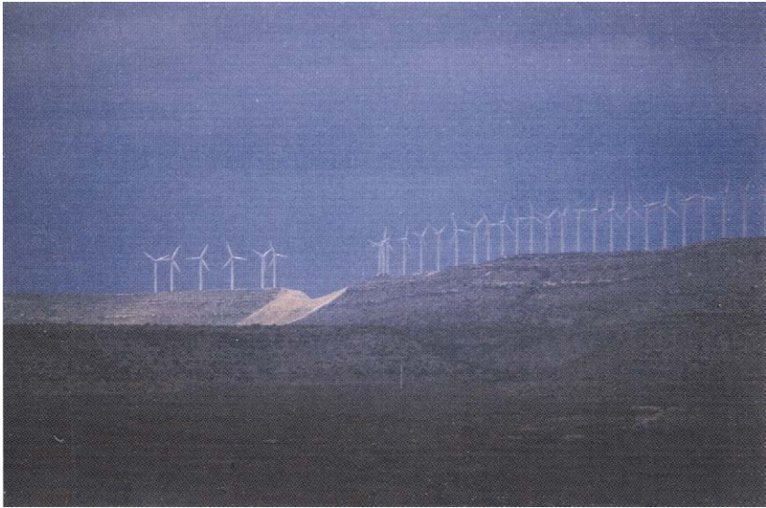
FIGURE 1.7 Part of an array of 107 wind turbines installed at the Southwest Mesa Wind Project, near McCamey, in West Texas, dedicated June 1999 by Governor George W. Bush. Together the 700-kW NEG-Micon generators have a capacity of 75 megawatts, making it at the time the largest wind power installation in Texas. It is located amid one of the most productive, but now largely spent, west Texas oil fields. (Courtesy Martin Pasqualetti.)
