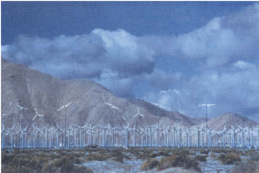
FIGURE 9.8 Inconsistent tower heights. Carter wind turbines on the White-water Wash near Palm Springs stuck out "like a sore thumb" above the mass of turbines on the dry riverbed. Worse, the Carter turbines seldom operated, drawing attention to themselves. These photos were taken 10 years after the turbines had been installed. All have since been removed and sold for scrap. (Courtesy Paul Gipe.)
