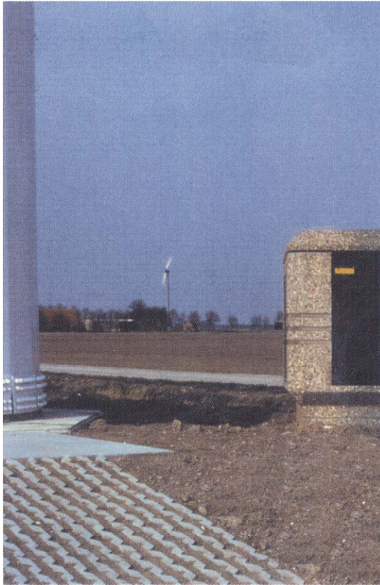
FIGURE 9.14 Hardened vehicle access. Hardening the access tract is also used at a small wind plant of six turbines along a canal in the Wieringermeer polder in north Holland. The prefabricated concrete blocks are designed to permit water percolation (a common feature of sidewalks and parking lots in lowland Europe) while supporting wheeled traffic. Nearby pad-mounted transformer is shrouded with a pleasing stone finish. (Courtesy Paul Gipe.)
