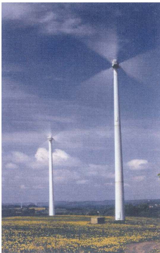
FIGURE 7.1 Hessen (Hesse), Mittlegebirge. Two turbines in a mixed cluster of machines on a hilltop in the Hoher Westerwald of Germany's central highlands. The Vestas turbine on the left is in the 500–600 kW class and was made in Denmark. The Fuhrländer on the right is about the same size and was built within the region. The turbines use rotors about 40 meters (130 feet) in diameter and stand atop towers of about the same height. Other turbines may be seen in the distance. (Courtesy Paul Gipe.)
