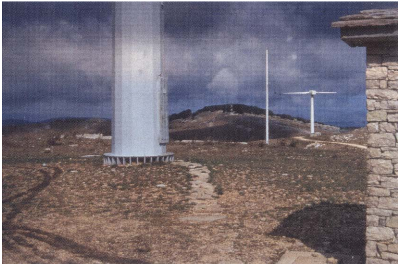
FIGURE 9.13 Hardened pedestrian access. The "Appian Way" of wind energy at ENEL's Acqua Spruzza test field in Italy's central Apennines. The façades and roofs of the control buildings use native stone, and the footpaths to the turbines are paved with flag stones. The flagstones "harden" the walkway, limiting erosion from foot traffic. (Courtesy Paul Gipe.)
