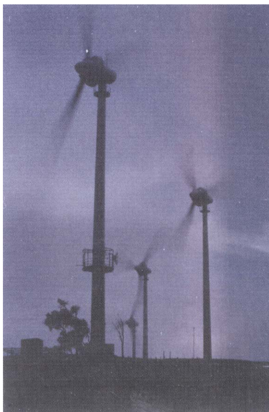
FIGURE 9.15 Telecom antennas. Awkward installation of a telecommunications antenna on an Enercon E40 tower at Wairarapa, New Zealand's first wind power plant. The E40, with its large ring generator, is ungainly enough on its own, but the antenna platform accentuates its industrial appearance. (Courtesy Paul Gipe.)
