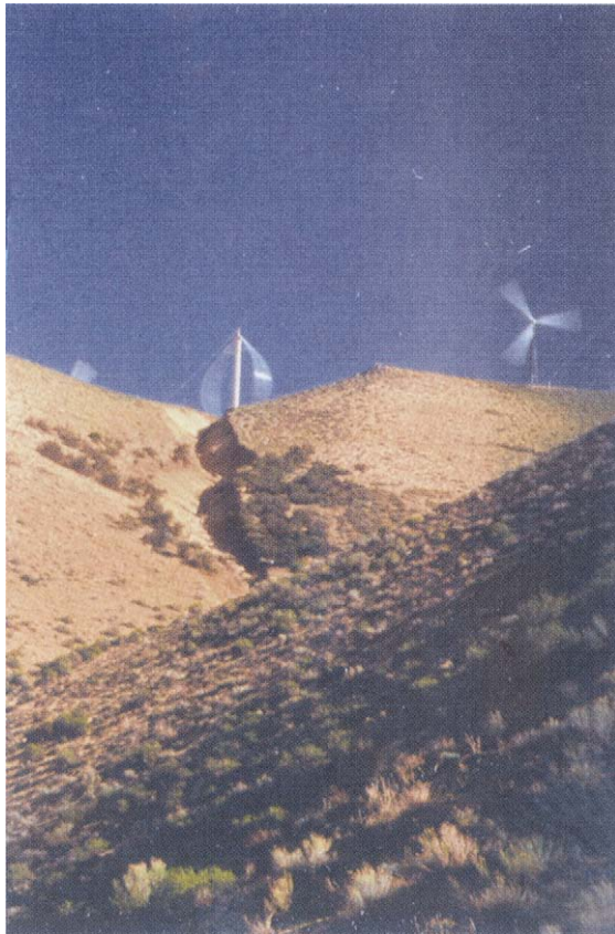
FIGURE 9.16 Tehachapi Pass erosion scar. Gully cutting into steep slope on Cameron Ridge below the former FloWind site in 1995. After this photo was taken, the Darrieus turbines were removed and new turbines installed. The new owners brought in British engineers to manage redevelopment. Local activists found the British engineers more sensitive to environmental concerns than domestic wind companies. (Courtesy Paul Gipe.)
