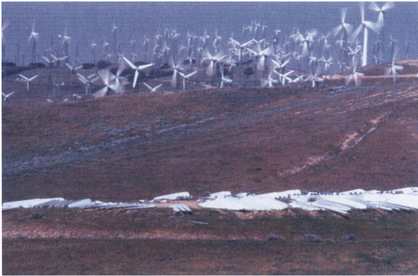
FIGURE 9.24 Bone yard II. Improper disposal of scrap wind turbine blades on Enron's (formerly Zond Systems) Victory Garden site in the Tehachapi Pass. There was at least one other large bone yard on the Enron site in spring 1998. (Courtesy Paul Gipe.)
