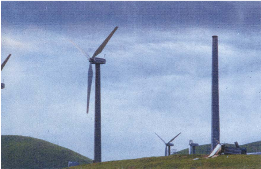
FIGURE 9.9 Headless horseman. Crumpled nacelle of a WindMaster turbine lies at the base of its headless tower in The Altamont Pass during spring 1997. In the background, another WindMaster stands idle with a broken and dangling blade. (Courtesy Paul Gipe.)
