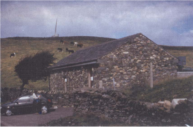
FIGURE 9.12 Harmonizing ancillary structures. National Windpower's transformer building at Kirkby Moor in Cumbria, northwest England. The façade uses native stone and the roof is covered with slate. Note windswept tree at left and wind turbine protruding just above the crest of the hill. (Courtesy Paul Gipe.)
