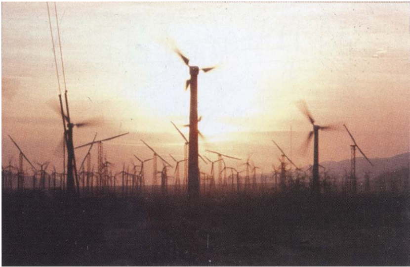
FIGURE 9.4 Visual clutter. Whitewater Wash, spring 1997. Visually disturbing mixture of two- and three-bladed turbines, truss and tubular towers, working and nonworking wind turbines. Many of these turbines, 13 years after the problem was first identified, were finally removed in 1998. (Telephoto lens foreshortens distance.) (Courtesy Paul Gipe.)
