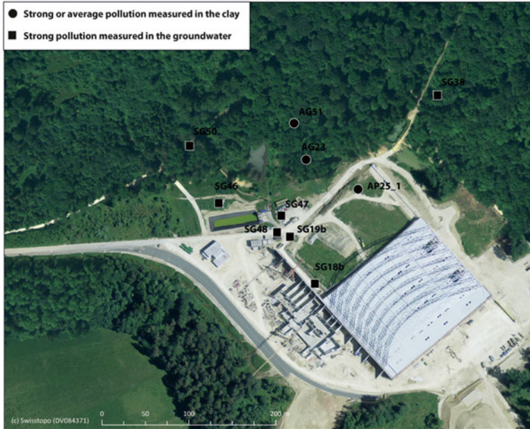
Fig. 8.3 Impacts of the Bonfol landfill on the groundwater as measured in 2003 (Satellite image of the site (2007) reproduced by permission of Swisstopo (DV084371). Data from (CSD Ingénieurs et Géologues SA & Mireco, 2003))
