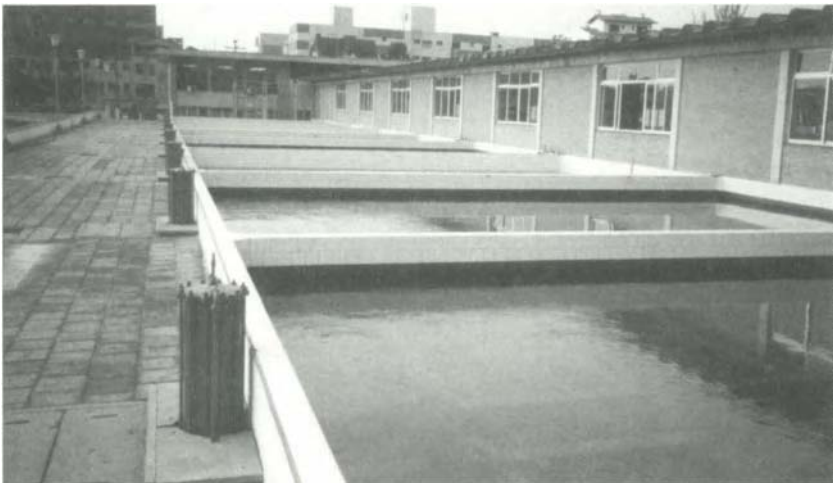
Figure 3.2 Photograph of deep bed filter units
