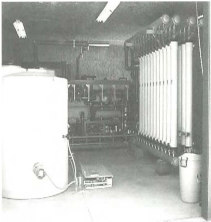
Figure 4.39 A modular MF system
