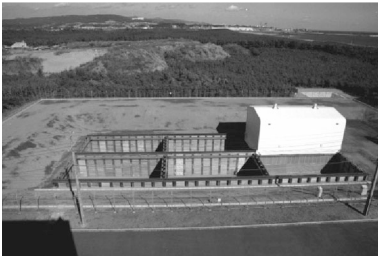
Fig. 6.2 General view of JAEA's waste burial field test facility ( http://www.enecho.meti.go.jp/rw/gaiyo/gaiyo03-1.html )
