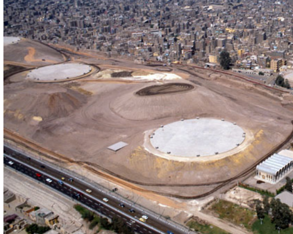
FIG. 3. The existing potable water tanks
