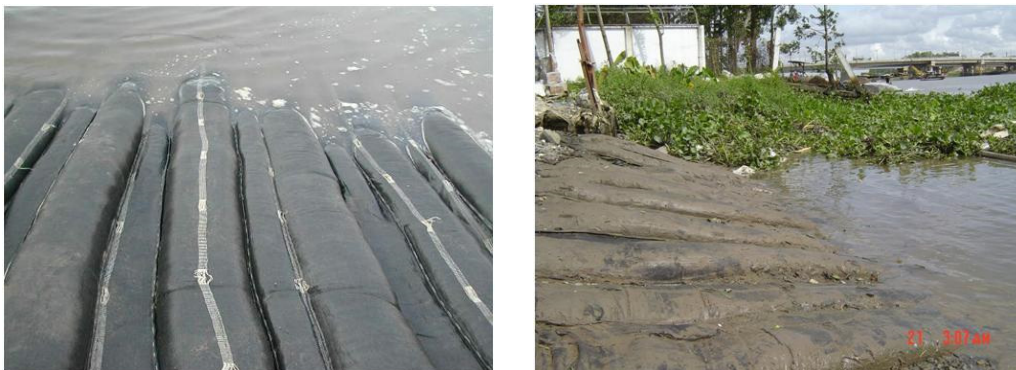
FIG.8 Sand mattresses installation (left) and after 18 months (right)
