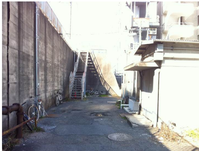
FIG. 9 Retaining Wall and Adjacent Buildings Prior to Construction
