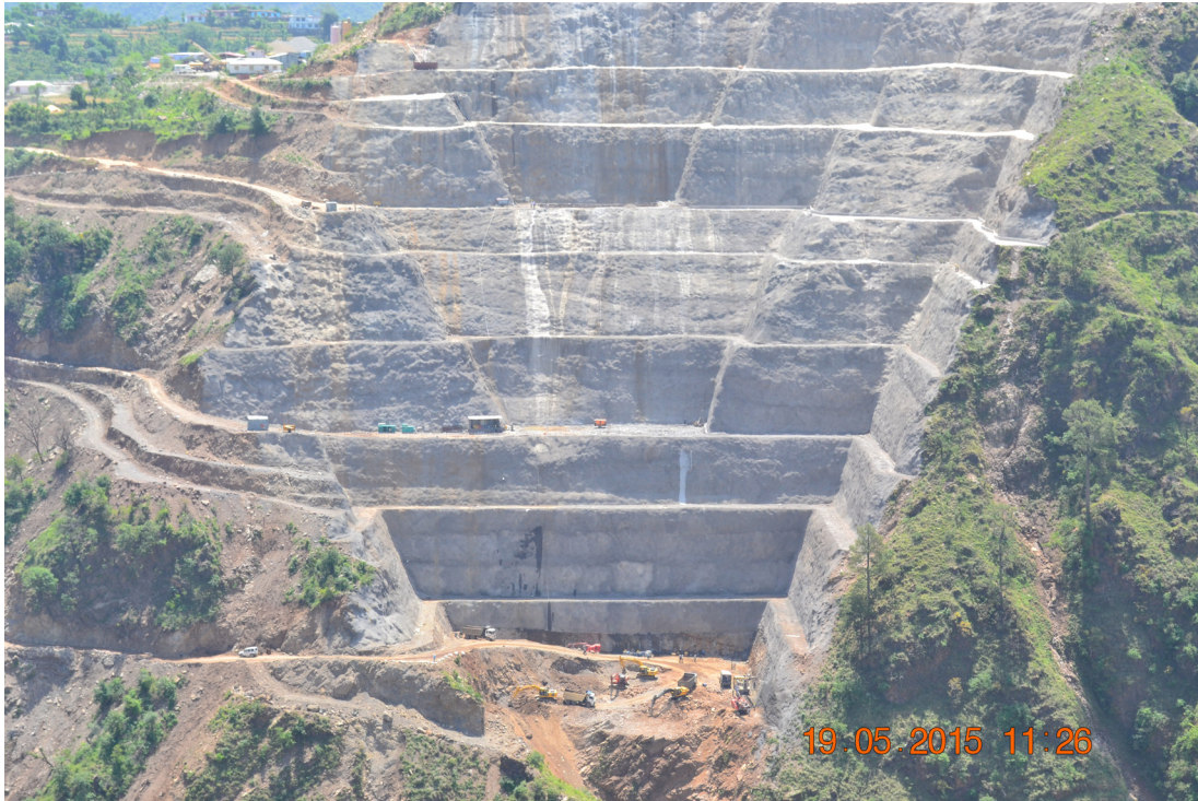
FIG. 6. Completed slope S2
