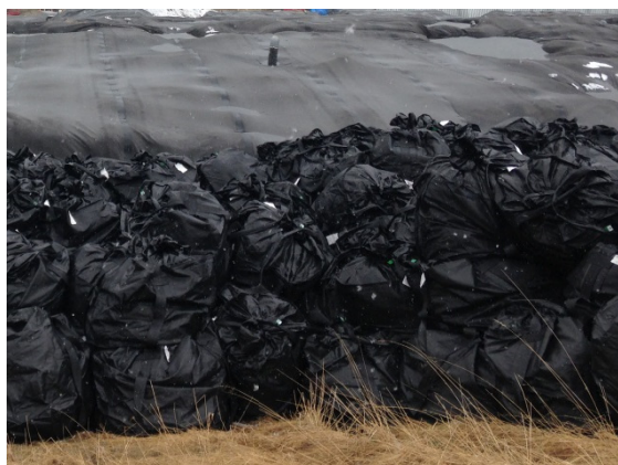
FIG. 1. Soil Bags Containing Radioactively Polluted Wastes and Soils Piled at a Temporary Storage Yard in Fukushima (March 2015).
