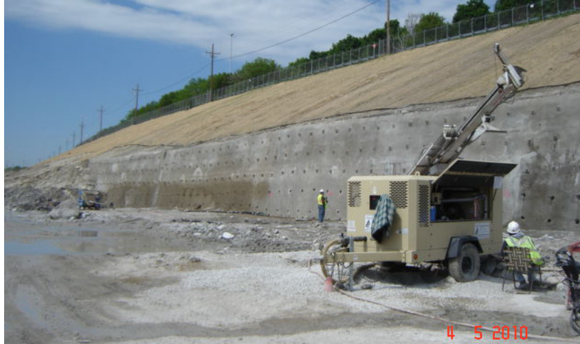
Figure 5: Photo of Soil Nail Wall installation
