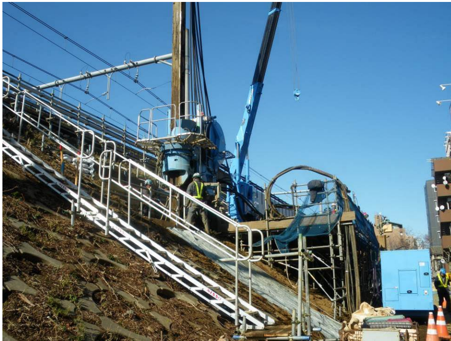
FIG. 8 Sheet Pile Installation by the Press-in Driver with GRB System
