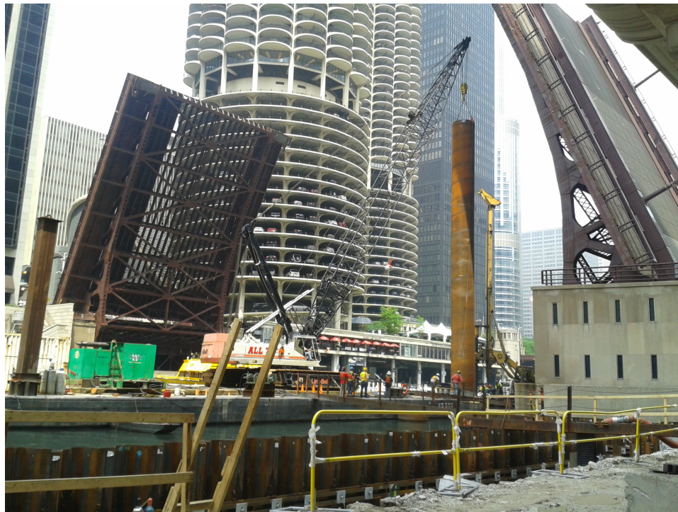
Figure 8 – Permanent Casing Installation for the Dearborn Street Underbridge
