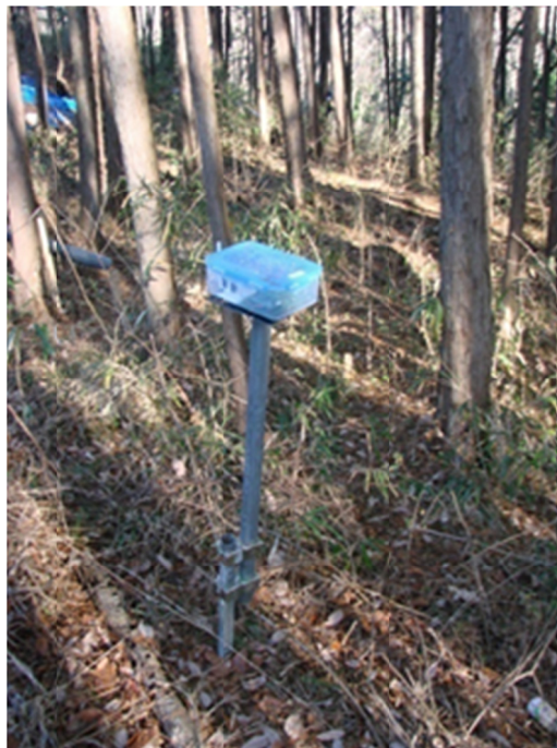
FIG.5. Set up of ZigBee router with sensing device on stands with piles.
