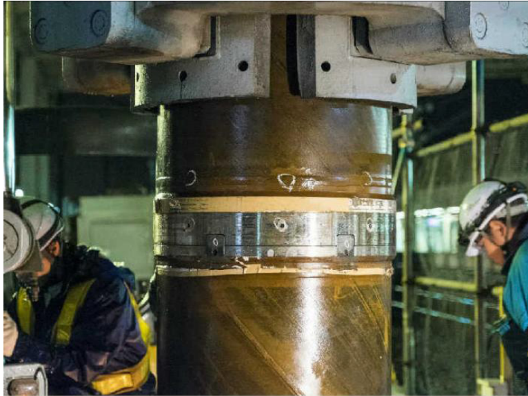
FIG. 12 Mechanically-spliced Tubular Pile
