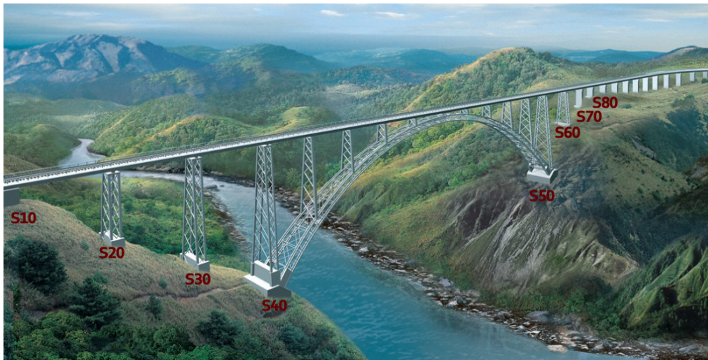
FIG. 2. Designer's view of the Chenab railway bridge
