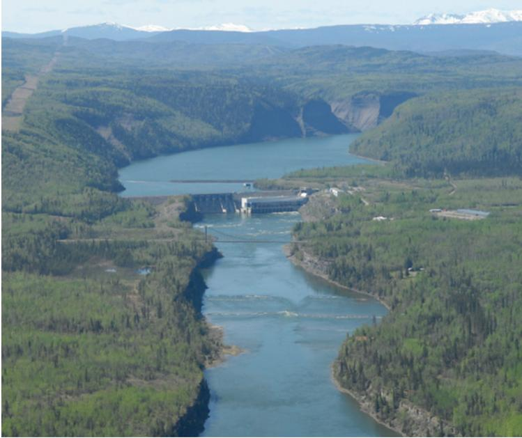
**Figure 1.3** Peace Canyon Dam, in the front ridge of the Rocky Mountains, northeastern British Columbia, Dinosaur Lake beyond. The dam is 20.4 km downstream from W.A.C. Bennett Dam, which impounds the reservoir known as Lake Williston. The white water immediately below the dam is formed by rock ridges on the channel bed. River flow is  $970 \text{ m}^3\text{s}^{-1}$  (Photo courtesy of M. J. Miles).
