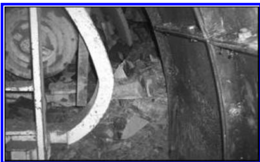
Figure 7. Material fall inside the tunnel.
