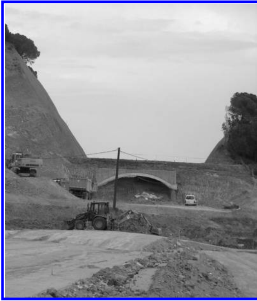
Figure 11. Construction of the Barcelona portal side of the Telleda Tunnel.
