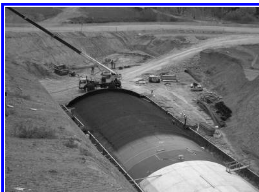
Figure 10. Construction of the reinforced vault.
