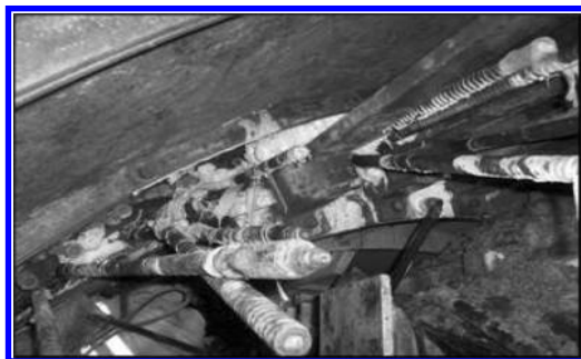
Figure 11. Injected selfdrilling rock bolts.
