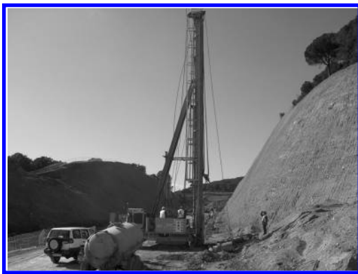
Figure 9. Construction of the pile walls.
