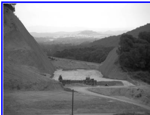
Figure 7. Trench excavated for building the Telleda Tunnel.
