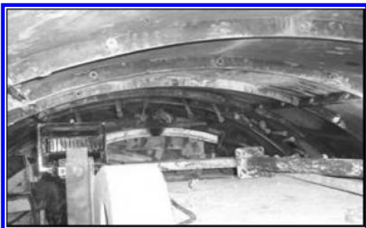
Figure 8. Rock bolts umbrella to the advance.
