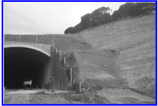
Figure 13. Construction of the portal on the French side.
