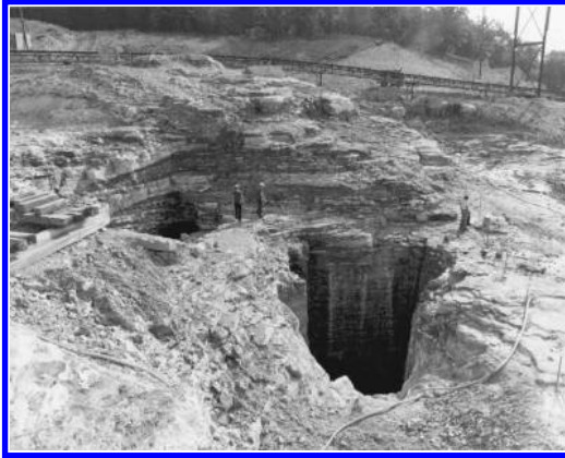
Figure 2. Large solution features discovered during the construction of the Mark Twain Lake's Clarence Cannon Dam on the Salt River near Hannibal, MO, USA, from Watkins (2006).
